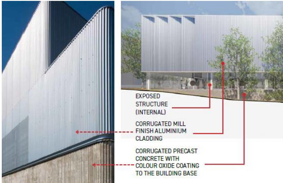
Figure 18: Description of external materials and finishes (west, north, south and east building elevations) Source: Lahznimmo Architects
