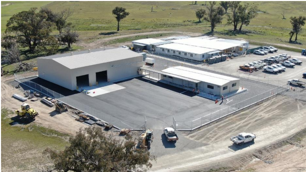
FIGURE 16 EXAMPLE O&M FACILITY
