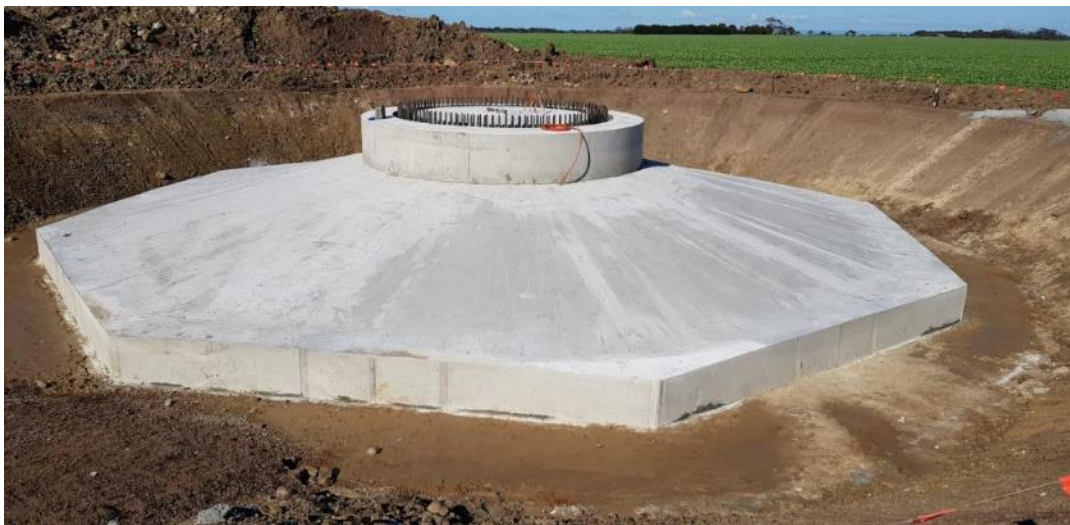
FIGURE 10 TYPICAL FOUNDATION IN CONSTRUCTION
