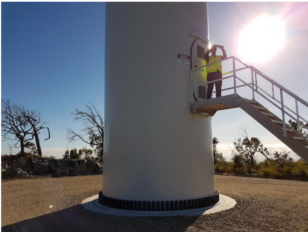
FIGURE 11 TYPICAL FOUNDATION POST-CONSTRUCTION
