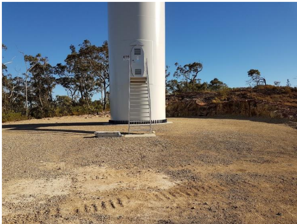
FIGURE 12 TYPICAL HARDSTAND AREA
