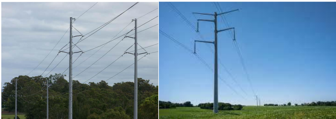
FIGURE 14 TYPICAL STEEL POLE STRUCTURES
