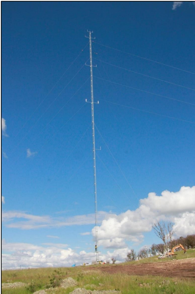
Figure 13 WMT 1 installed onsite
