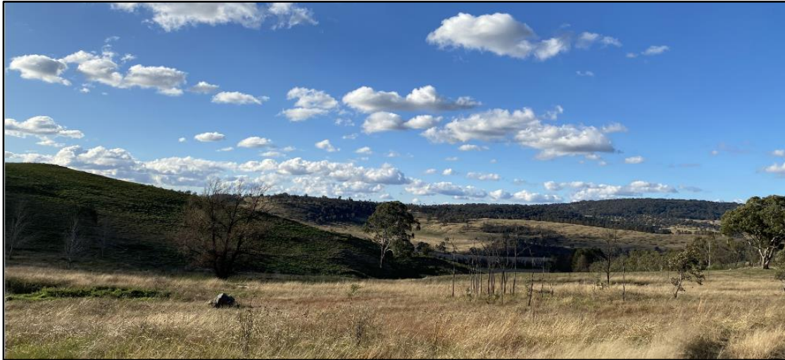
Figure 9 Oxley Highway looking to the north-east at WWF site
