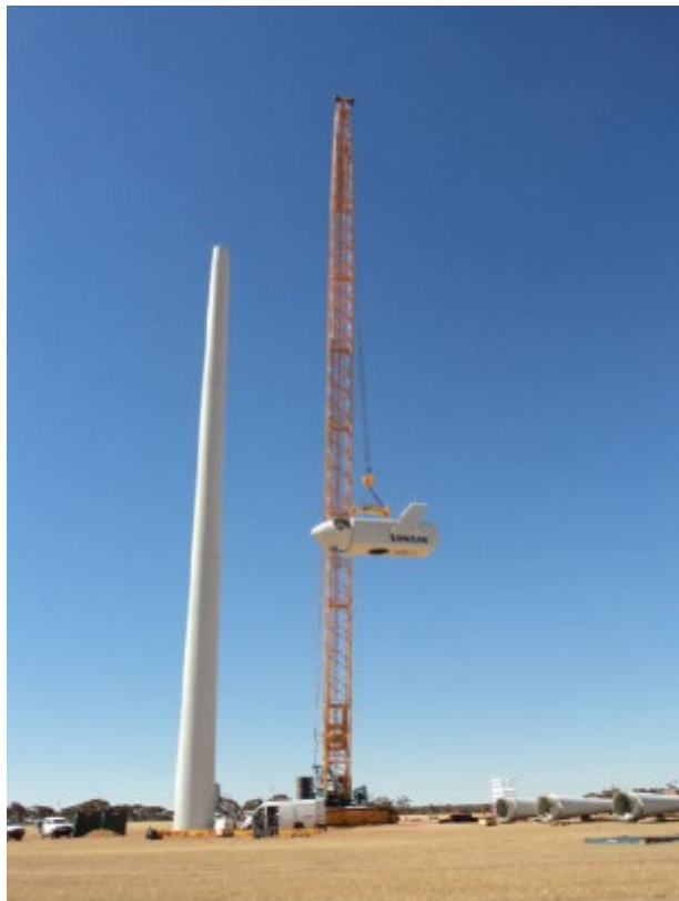
Figure 20 | Wind Turbine Nacelle dismantling
