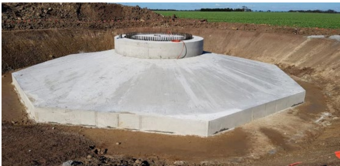
Figure 4 | Typical gravity wind turbine reinforced concrete foundation
