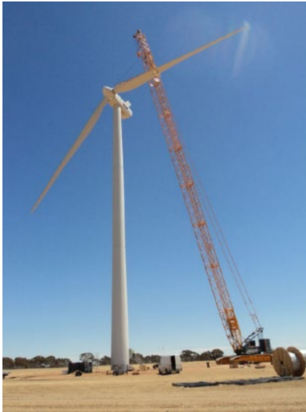
Figure 19 | Wind Turbine Blade dismantling
