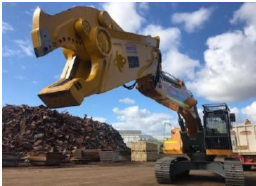
Figure 27 | Hydraulic excavator with shear attachment
