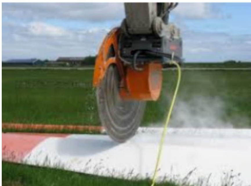
Figure 25 | Wind turbine blade cutting
