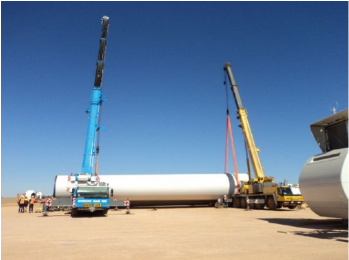
Figure 23 | Tower sections loaded onto over dimensional transport
