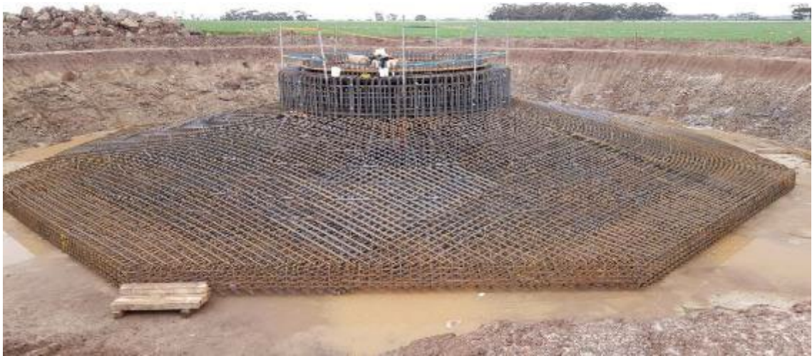
Figure 3 | Typical gravity wind turbine foundation reinforcement
