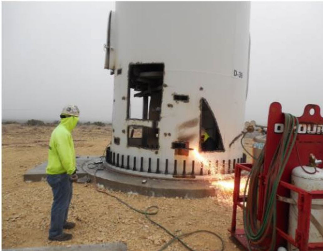
Figure 24 | Oxy-acetylene cutting preparation of tower base
