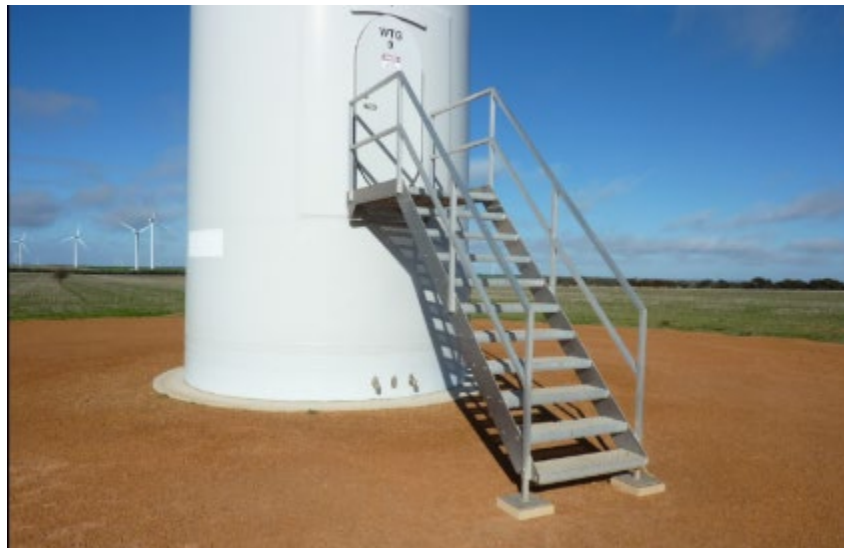
Figure 6 | Wind turbine tower base and access stairs
