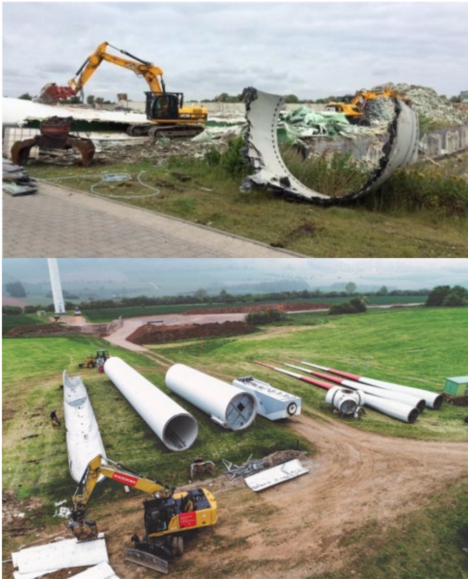
Figure 26 | Wind turbine components processing for scrap recycling
