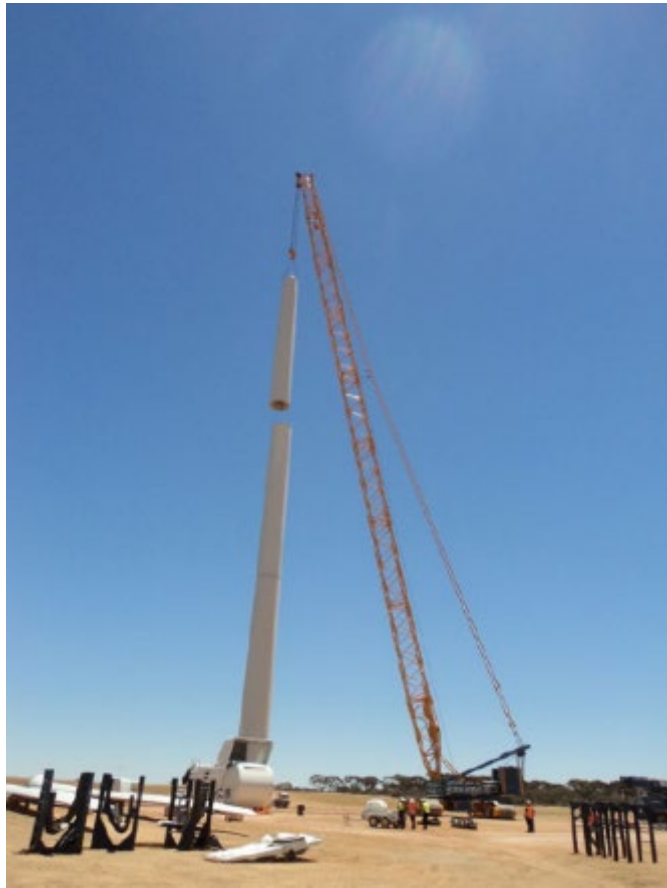
Figure 21 | Wind turbine tower dismantling
