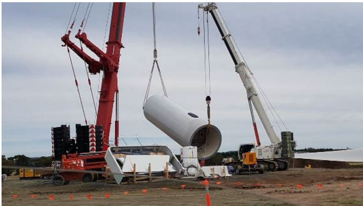
Figure 22 | Cranage of wind turbine components
