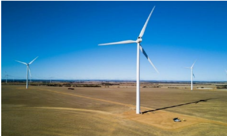
Figure 7 | Typical wind farm access road and crane hardstand
