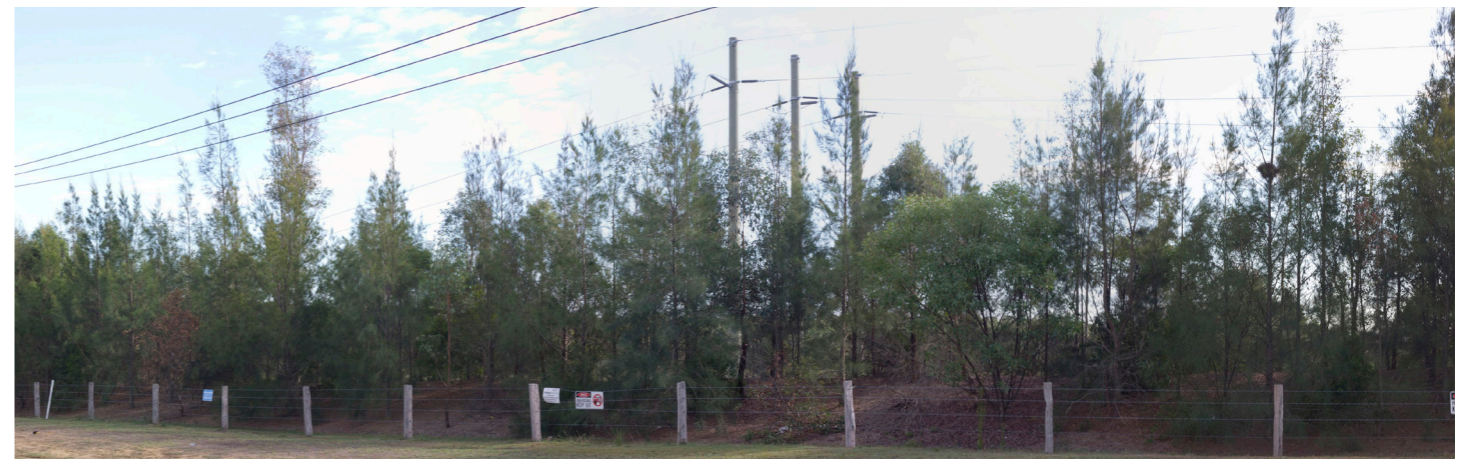
Image 35: Example of landscape screening along the boundary of a substation - Rothbury NSW
