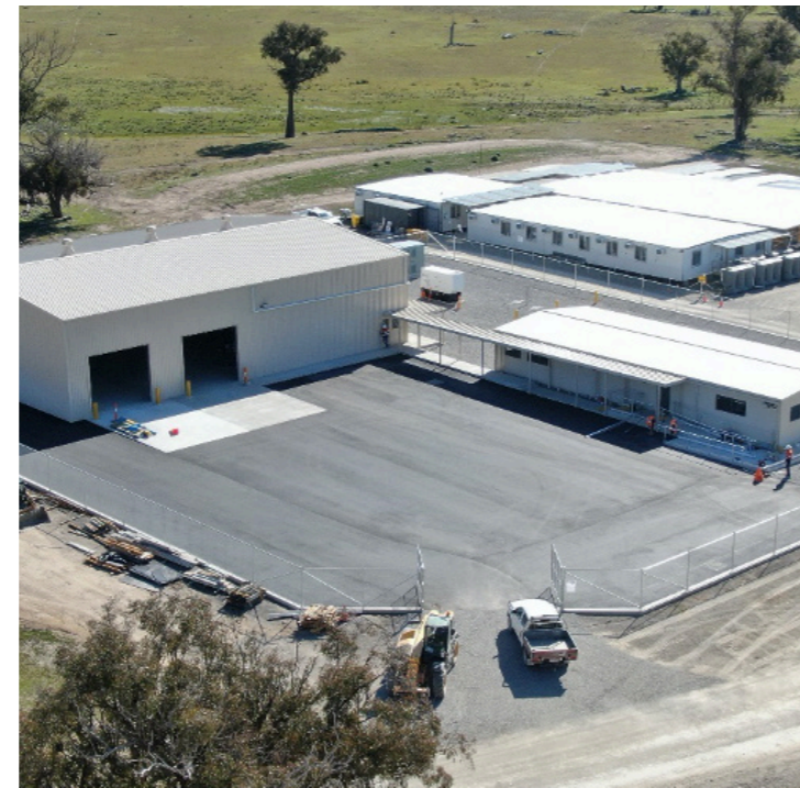
Image 5: Operations and Maintenance Facility (Source: Vestas)
