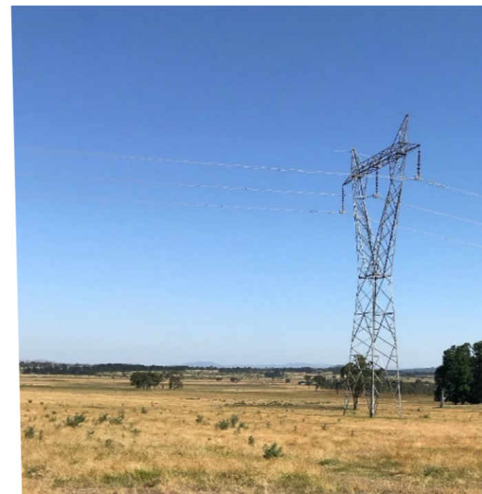
Image 3: Transmission Line (Source: Vestas)
