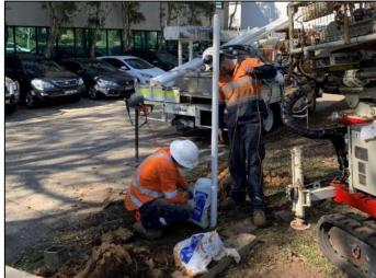
Plate 22 – Installation of MW121 on 15 Percy Street.
