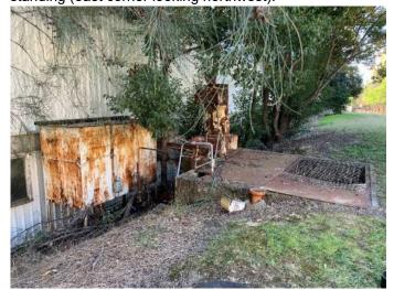
Plate 6 – Former lime dosing unit (south corner).
