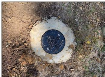
Plate 24 – Finished monitoring well.
