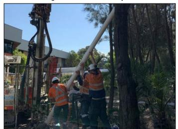
Plate 23 – Installation of casing for air hammer drilling at MW205 on 15 Percy Street.
