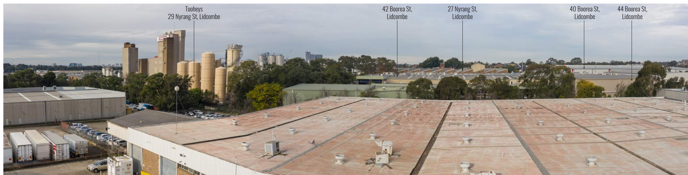
Figure 4: Drone at RL 24.65m - Looking East
