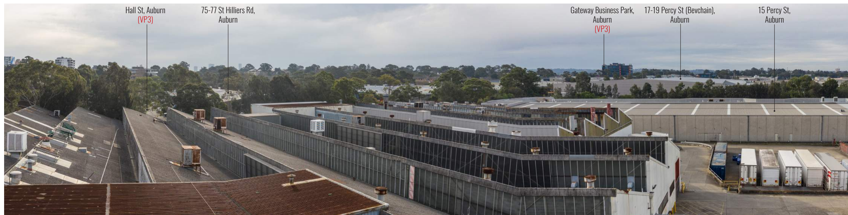
Figure 3: Drone at RL 24.65m - Looking North
