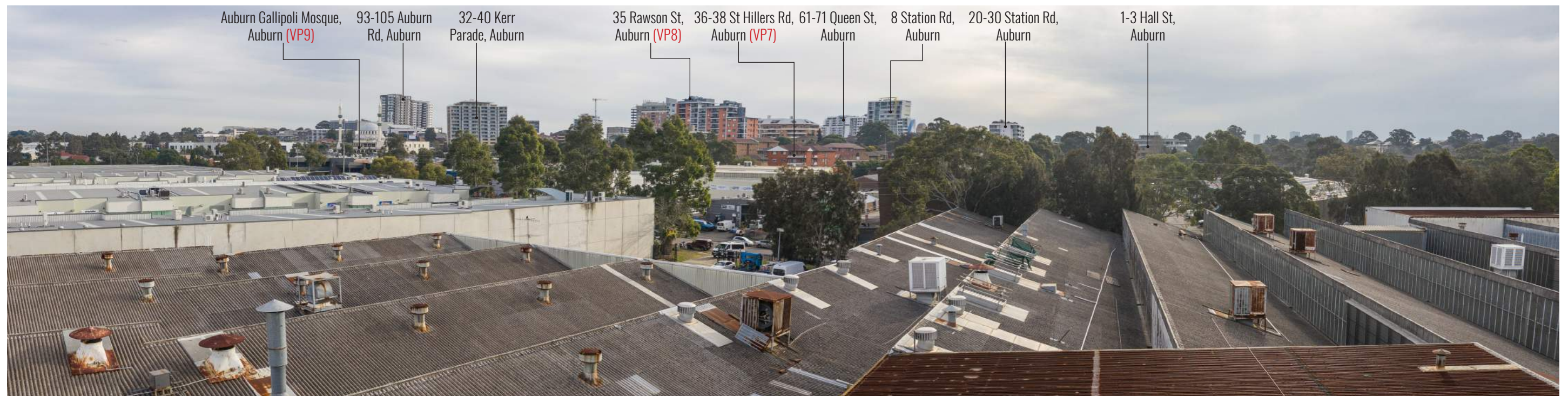
Figure 6: Drone at RL 24.65m - Looking West
