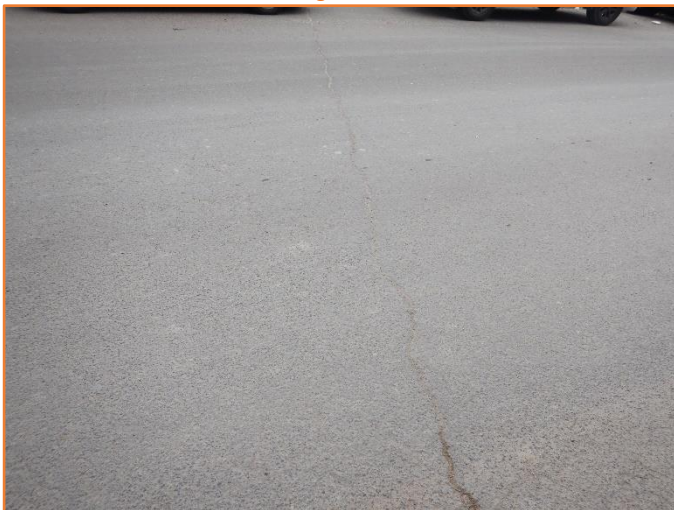
Figure 208: Reasonable - General condition of flexible pavement. Major cracking observed.
