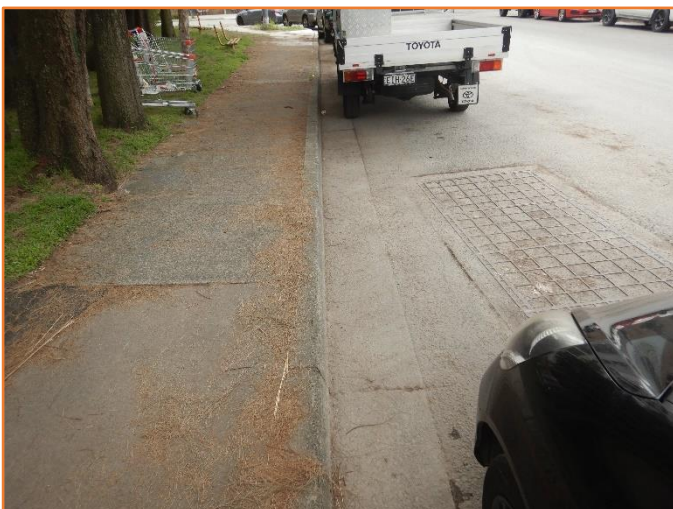
Figure 362: Reasonable - General condition of kerb and gutter. Minor cracking observed.
