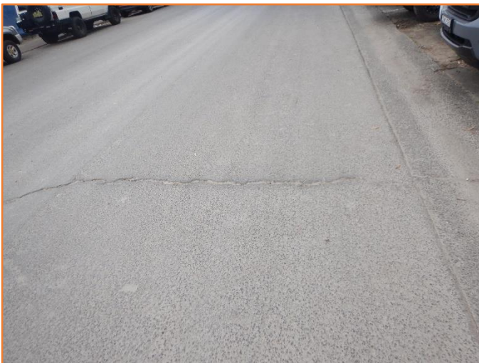
Figure 250: Reasonable - General condition of flexible pavement. Major cracking observed.
