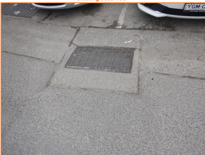
Figure 275: Reasonable - General condition of service pit. Minor cracking observed.
