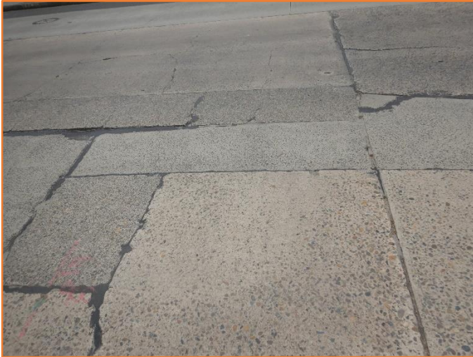
Figure 100: Reasonable - General condition of rigid pavement. Extensive cracking observed.
