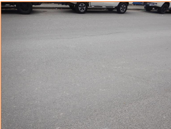
Figure 245: Reasonable - General condition of flexible pavement. Minor cracking observed.
