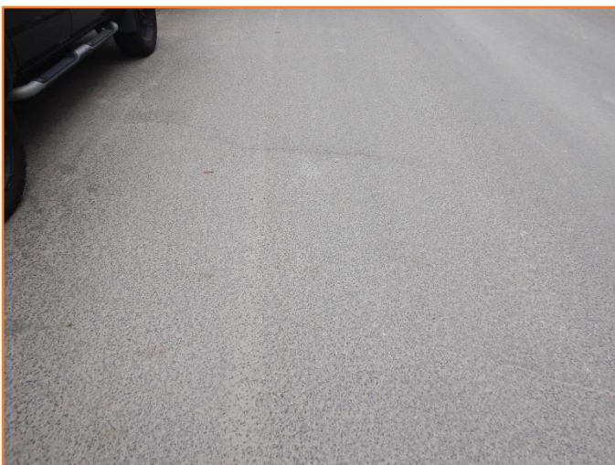
Figure 242: Reasonable - General condition of flexible pavement. Minor cracking observed.
