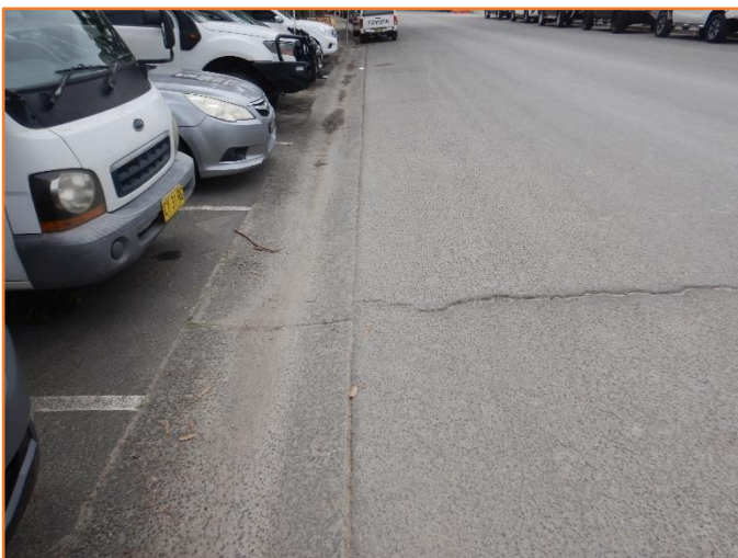
Figure 323: Reasonable - General condition of kerb and gutter. Minor cracking observed.
