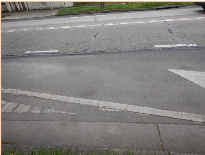
Figure 89: Reasonable - General condition of flexible and rigid pavement.
