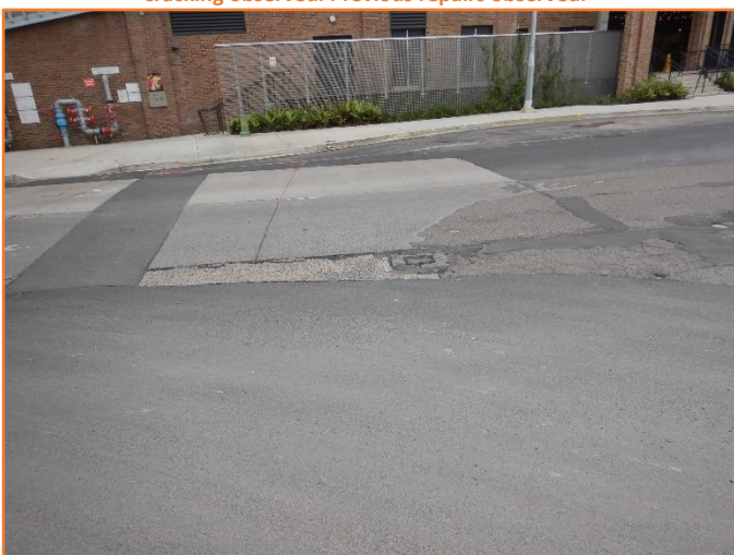
Figure 51: Reasonable - General condition of flexible pavement. Minor cracking observed.
