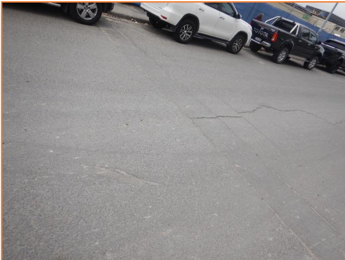
Figure 235: Reasonable - General condition of flexible pavement. Major cracking observed.
