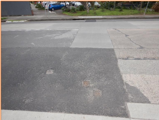
Figure 104: Reasonable - General condition of flexible and rigid pavement. Minor cracking observed.
