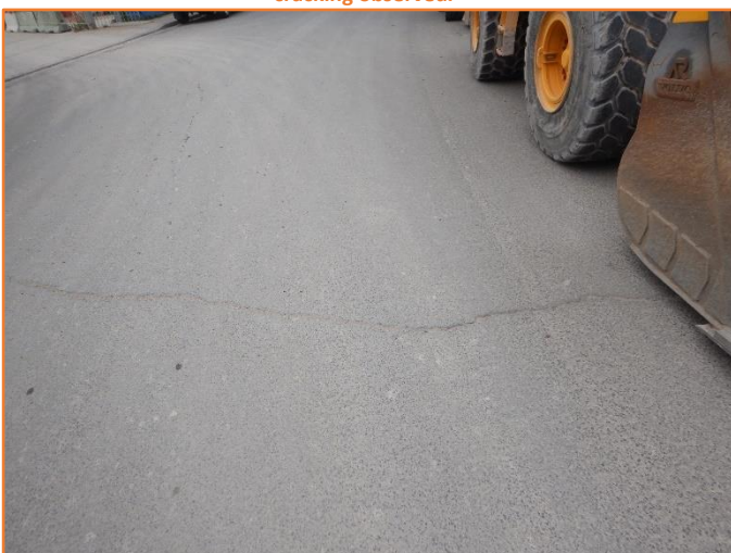
Figure 221: Reasonable - General condition of flexible pavement. Major cracking observed.
