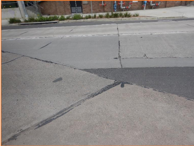
Figure 58: Reasonable - General condition of rigid pavement. Minor cracking observed.
