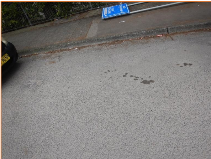
Figure 211: Reasonable - General condition of flexible pavement. Minor cracking observed.
