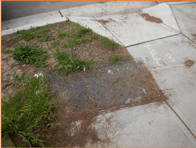
Figure 381: Reasonable - General condition of service pit.
