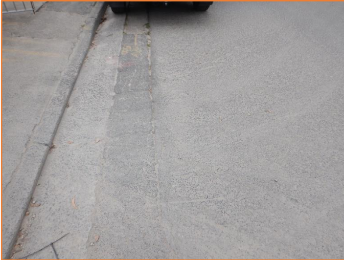
Figure 228: Reasonable - General condition of flexible pavement. Extensive cracking observed. Previous repairs observed.
