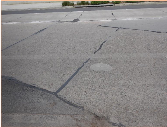
Figure 61: Reasonable - General condition of rigid pavement. Minor cracking observed.
