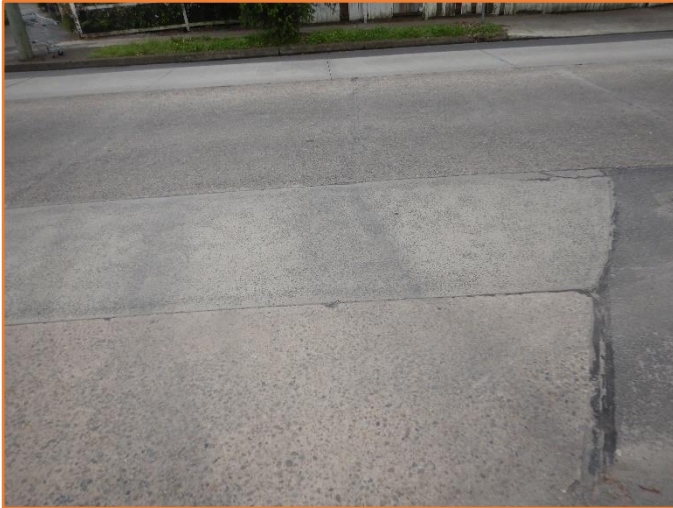
Figure 97: Reasonable - General condition of rigid pavement. Minor cracking observed.
