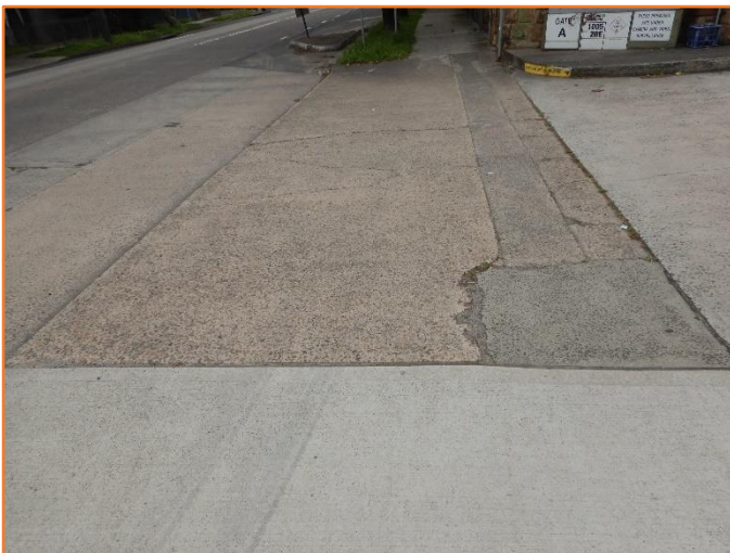
Figure 122: Reasonable - General condition of driveway crossover. Major cracking observed.
