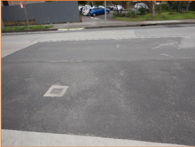
Figure 106: Reasonable - General condition of flexible pavement.
