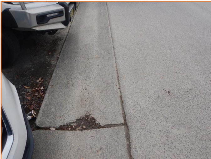
Figure 316: Reasonable - General condition of kerb and gutter. Minor spalling observed.
