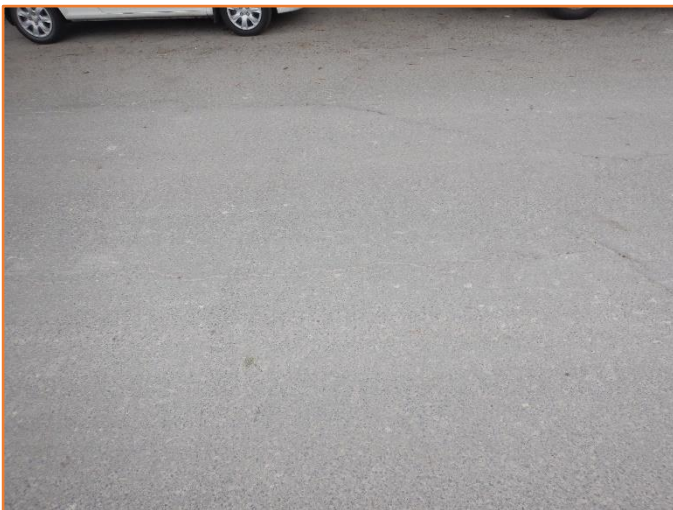
Figure 238: Reasonable - General condition of flexible pavement. Minor cracking observed.
