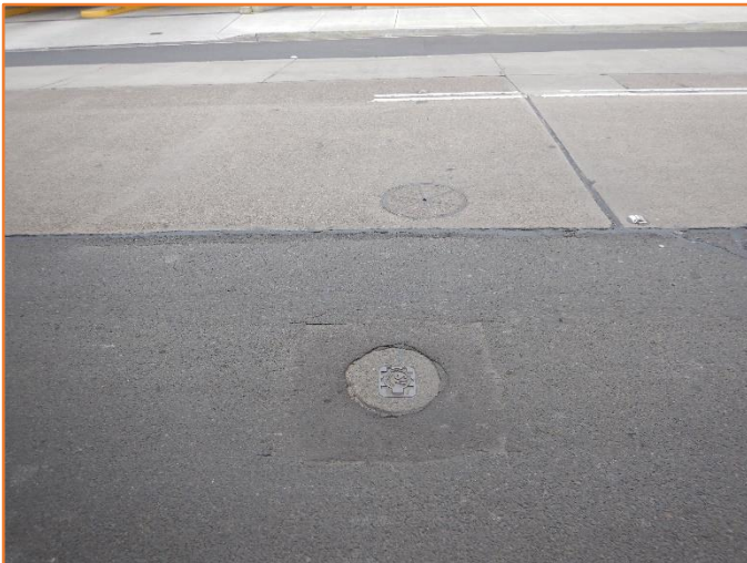
Figure 68: Reasonable - General condition of service pit.
