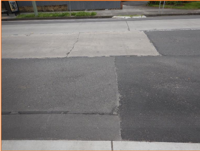
Figure 109: Reasonable - General condition of flexible and rigid pavement. Minor cracking observed.
