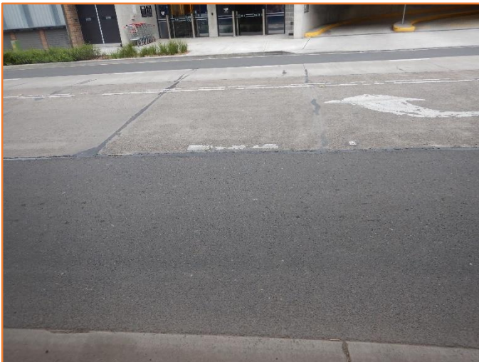
Figure 72: Reasonable - General condition of flexible and rigid pavement.
