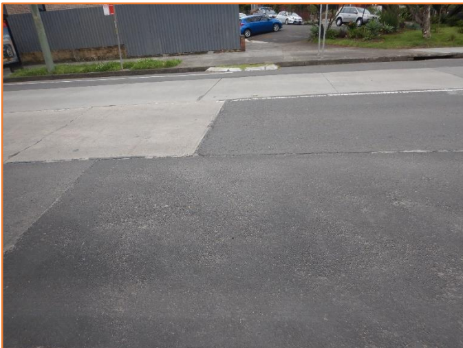
Figure 108: Reasonable - General condition of flexible and rigid pavement.
