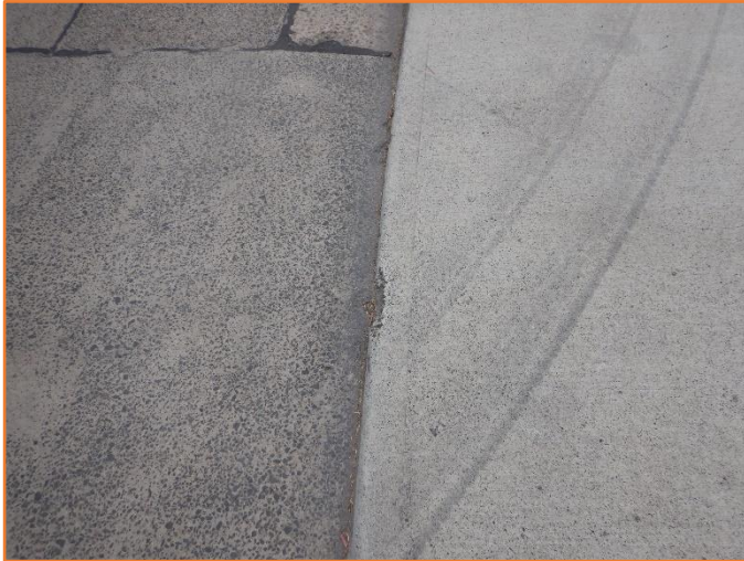
Figure 7: Reasonable - General condition of driveway layback. Minor spalling observed.
