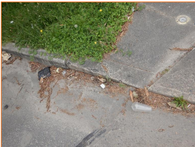
Figure 9: Reasonable - General condition of driveway splay. Minor cracking and spalling observed.
