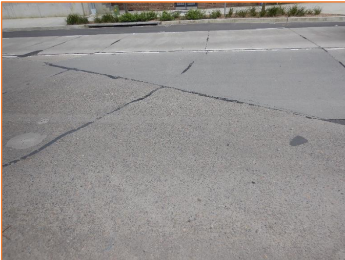
Figure 59: Reasonable - General condition of rigid pavement. Minor cracking observed.
