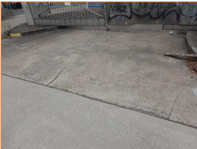
Figure 119: Reasonable - General condition of driveway crossover. Minor cracking observed.
