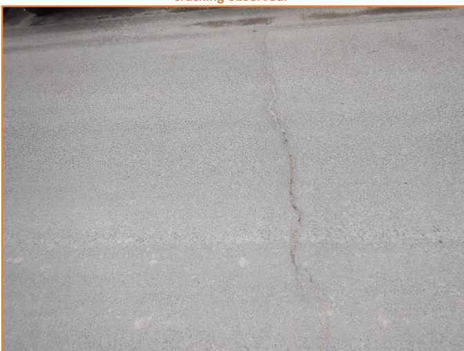
Figure 260: Reasonable - General condition of flexible pavement. Major cracking observed.
