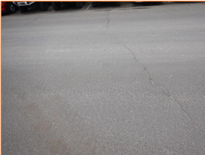
Figure 259: Reasonable - General condition of flexible pavement. Major cracking observed.
