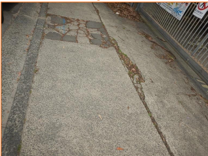
Figure 416: Reasonable - General condition of driveway crossover. Extensive cracking observed.
