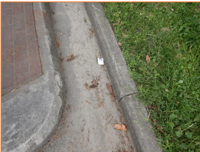
Figure 11: Reasonable - General condition of kerb and gutter. Minor cracking observed.
