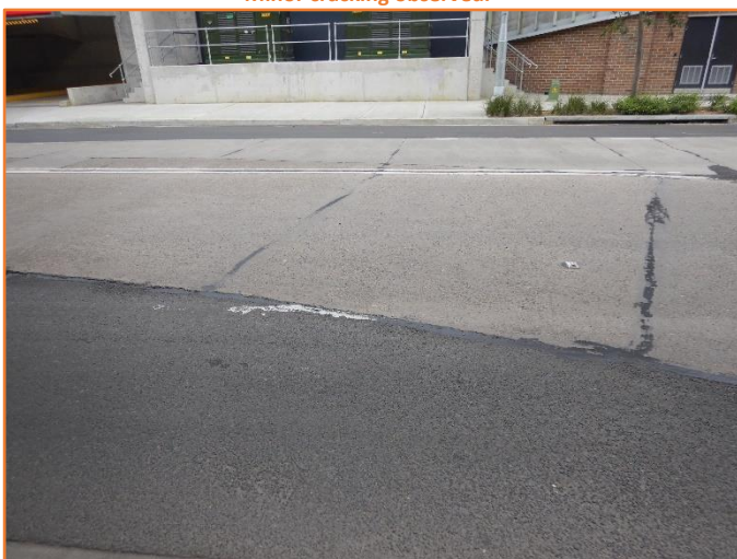
Figure 63: Reasonable - General condition of flexible and rigid pavement. Minor cracking observed.
