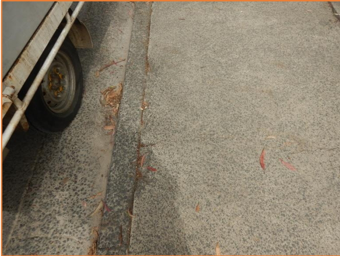
Figure 420: Reasonable - General condition of footpath. Minor cracking observed.
