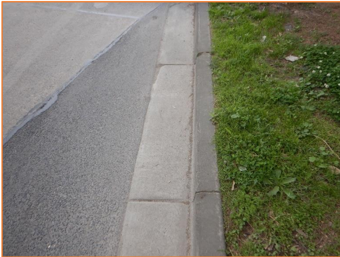
Figure 40: Reasonable - General condition of kerb and gutter. Minor cracking observed.
