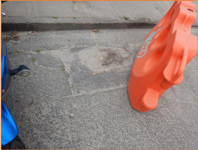
Figure 225: Reasonable - General condition of flexible pavement. Minor cracking observed. Previous repairs observed.
