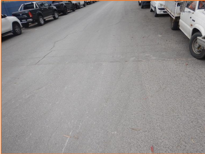
Figure 234: Reasonable - General condition of flexible pavement. Major cracking observed.
