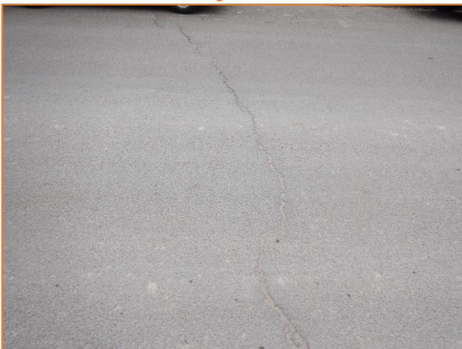
Figure 251: Reasonable - General condition of flexible pavement. Major cracking observed.
