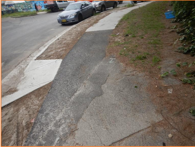
Figure 186: Reasonable - General condition of footpath. Minor cracking observed. Previous repairs observed.
