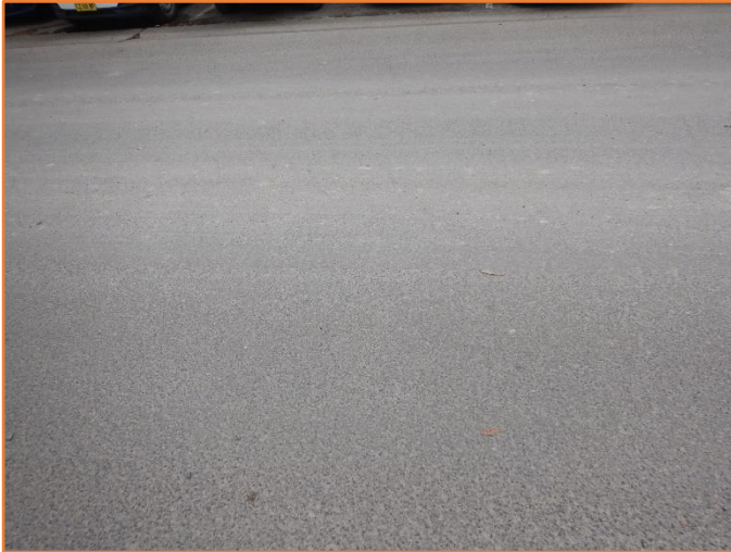
Figure 264: Reasonable - General condition of flexible pavement.
