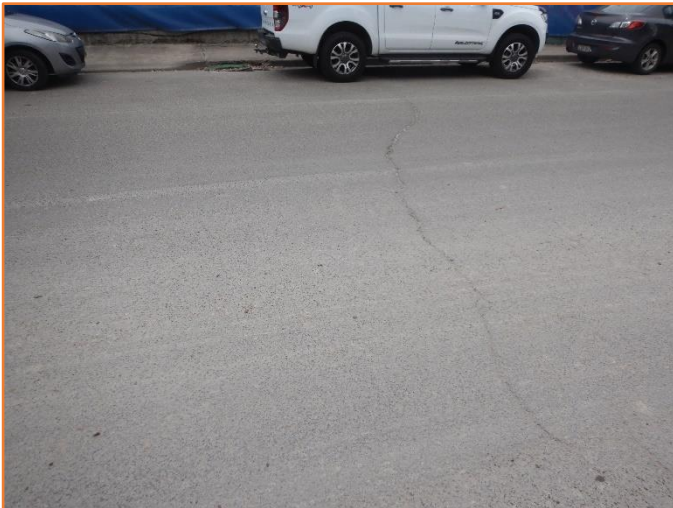
Figure 274: Reasonable - General condition of flexible pavement. Major cracking observed.
