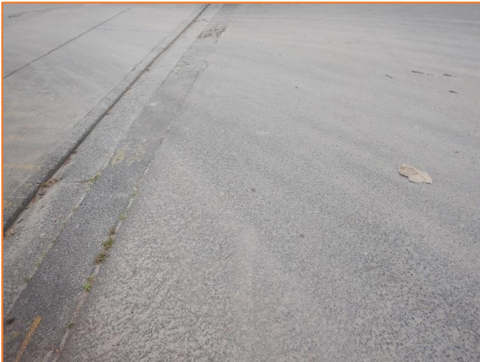
Figure 226: Reasonable - General condition of flexible pavement. Minor cracking observed. Previous repairs observed.
