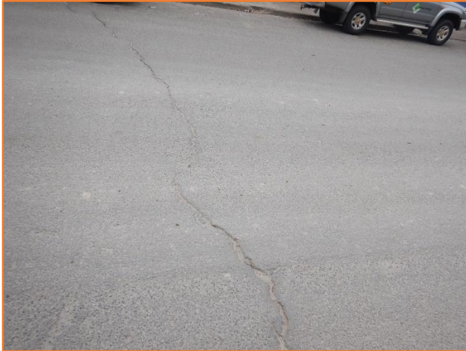
Figure 252: Reasonable - General condition of flexible pavement. Major cracking observed.
