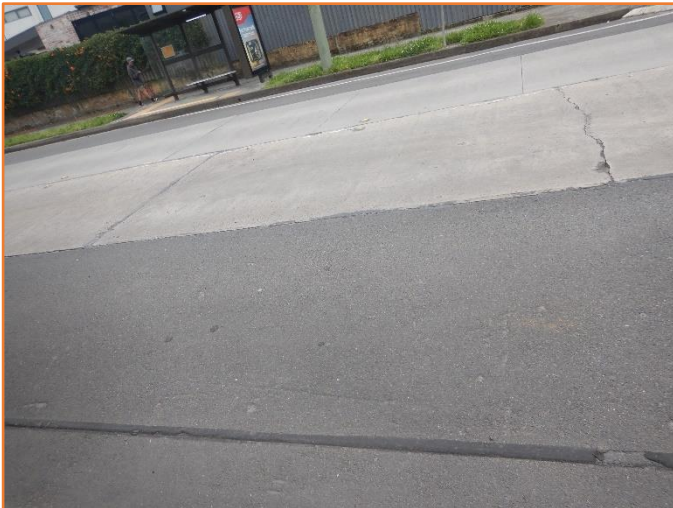
Figure 110: Reasonable - General condition of flexible and rigid pavement. Minor cracking observed.
