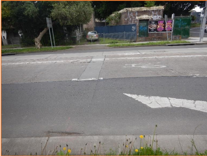
Figure 85: Reasonable - General condition of flexible and rigid pavement.
