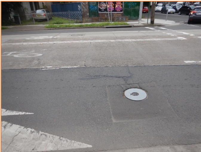
Figure 83: Reasonable - General condition of flexible and rigid pavement. Minor cracking observed.
