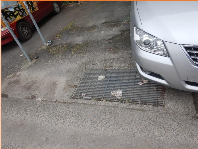
Figure 276: Reasonable - General condition of service pit. Minor cracking observed.
