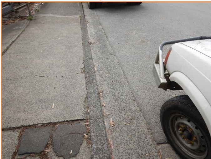
Figure 343: Reasonable - General condition of kerb and gutter. Minor cracking observed.
