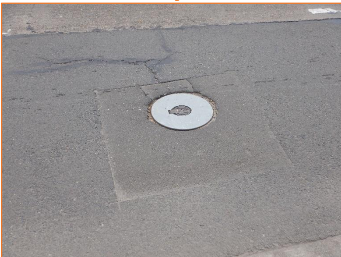
Figure 84: Reasonable - General condition of service pit. Minor cracking observed.
