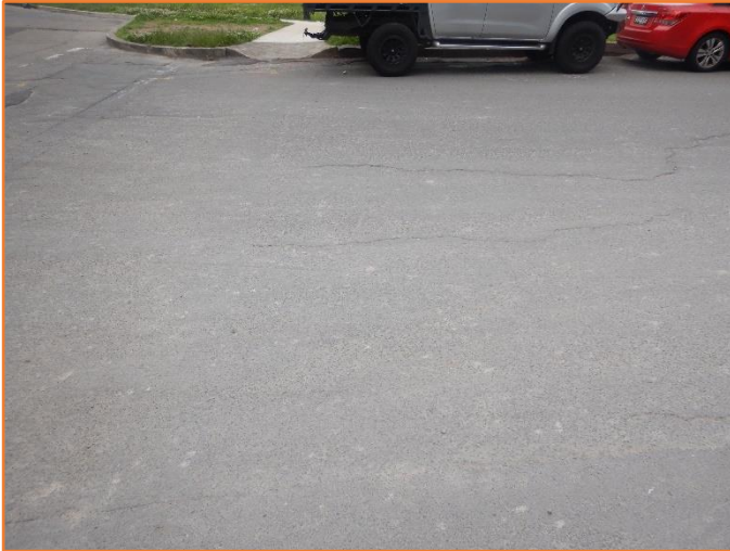
Figure 192: Reasonable - General condition of flexible pavement. Minor cracking observed.
