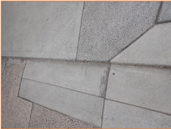
Figure 5: Reasonable - General condition of driveway layback. Minor cracking observed.
