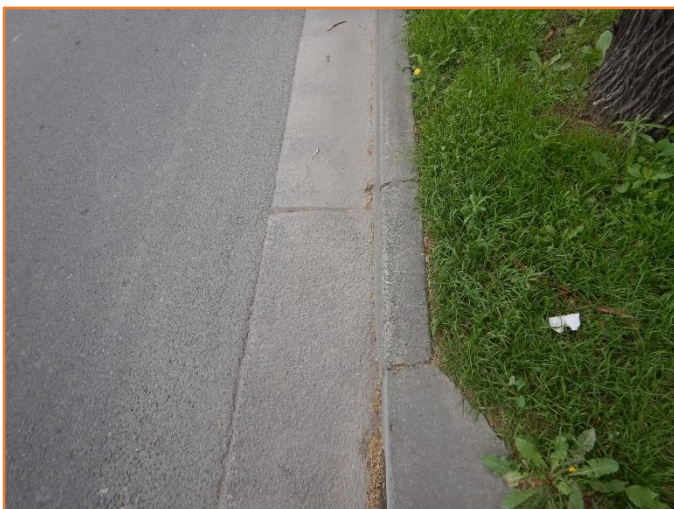
Figure 33: Reasonable - General condition of kerb and gutter. Minor cracking observed.
