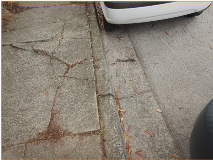
Figure 339: Reasonable - General condition of kerb and gutter. Minor cracking observed.
