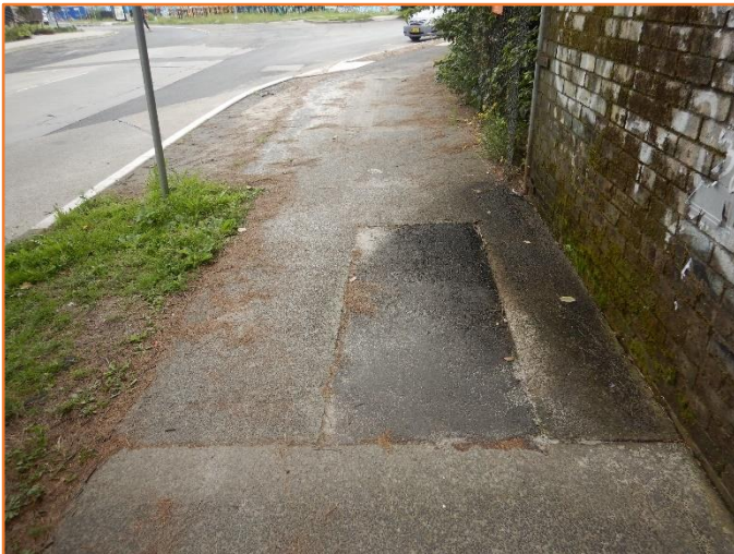
Figure 182: Reasonable - General condition of footpath. Previous repairs observed.
