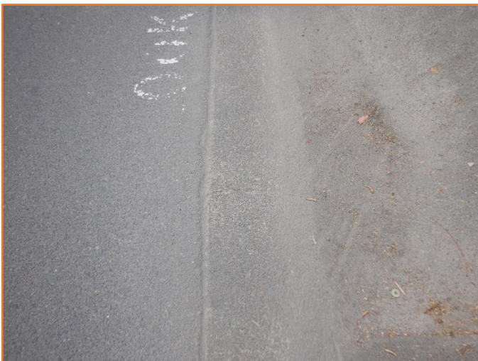
Figure 21: Reasonable - General condition of flexible pavement. Minor physical damage observed.
