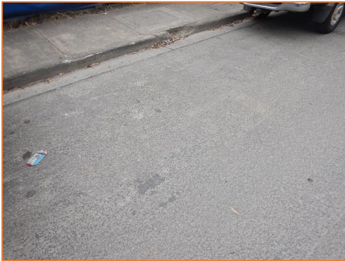
Figure 253: Reasonable - General condition of flexible pavement. Minor physical damage observed.
