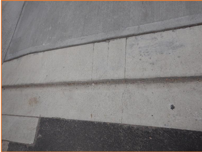
Figure 4: Reasonable - General condition of driveway layback. Minor cracking observed.
