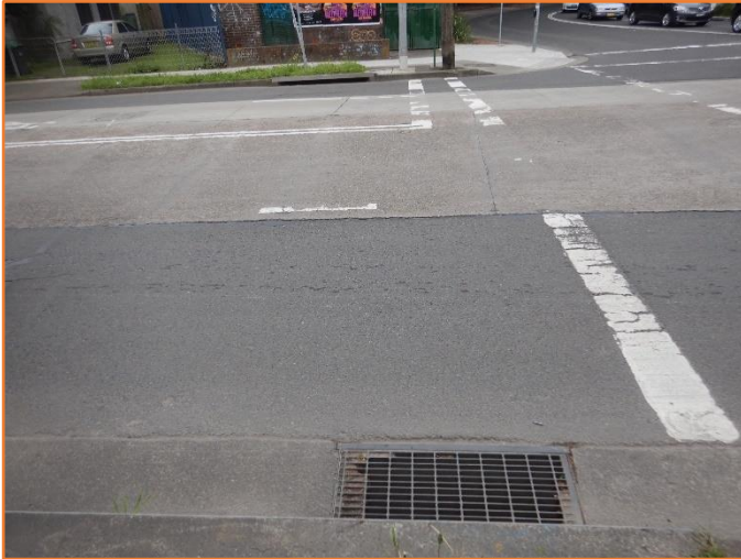
Figure 82: Reasonable - General condition of flexible and rigid pavement.
