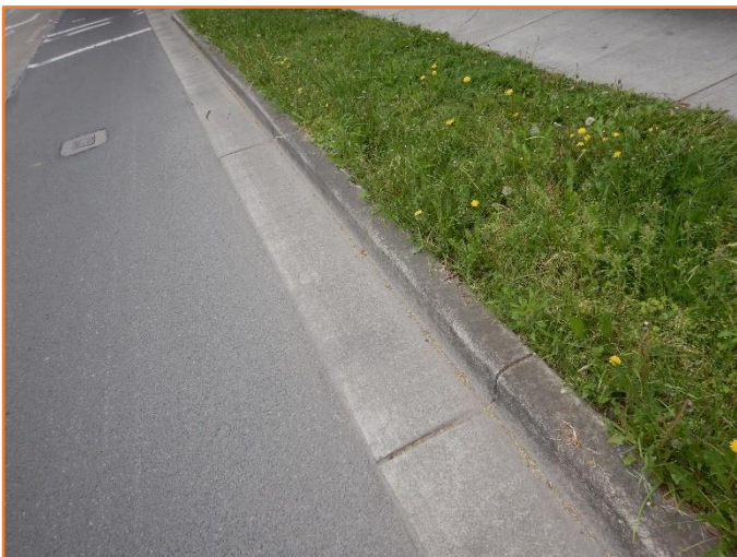
Figure 24: Reasonable - General condition of kerb and gutter. Minor spalling observed.
