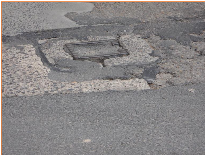
Figure 53: Reasonable - General condition of service pit. Minor cracking observed.
