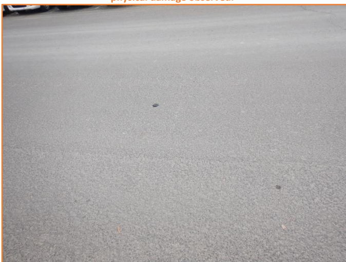
Figure 254: Reasonable - General condition of flexible pavement.
