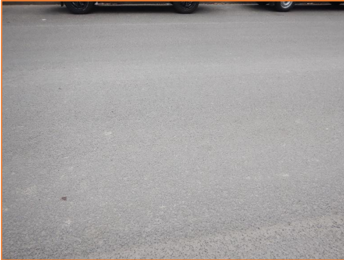
Figure 249: Reasonable - General condition of flexible pavement.
