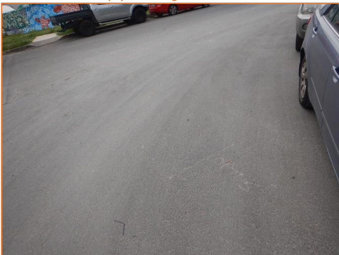
Figure 191: Reasonable - General condition of flexible pavement. Minor physical damage observed.
