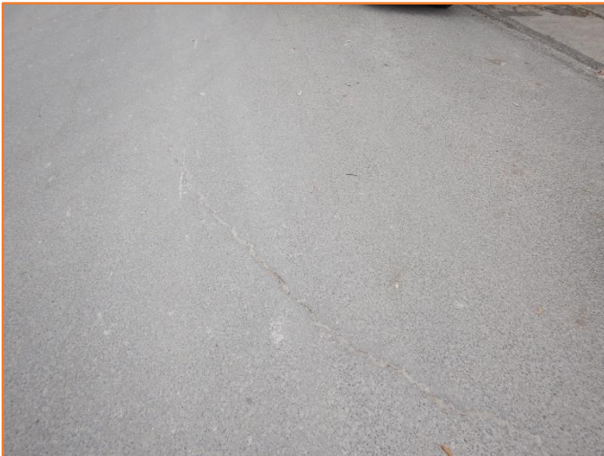
Figure 232: Reasonable - General condition of flexible pavement. Minor cracking observed.
