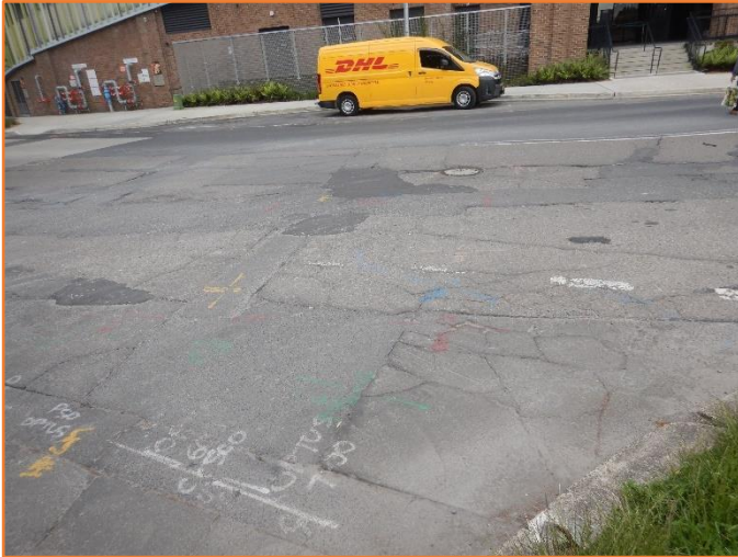
Figure 46: Poor - General condition of flexible pavement. Extensive cracking observed. Previous repairs observed.
