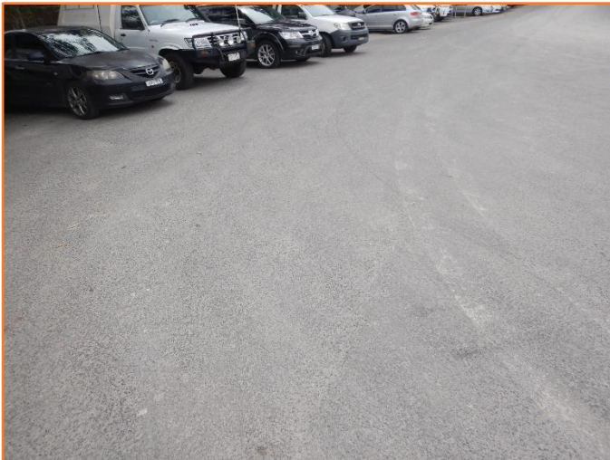
Figure 292: Reasonable - General condition of flexible pavement.
