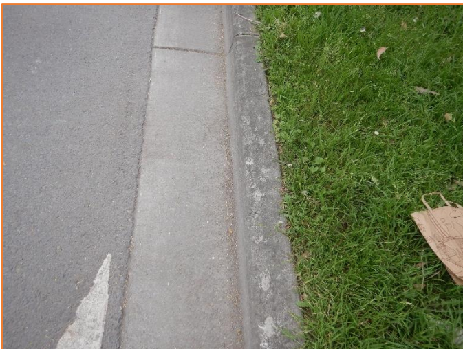
Figure 15: Reasonable - General condition of kerb and gutter. Minor spalling observed.
