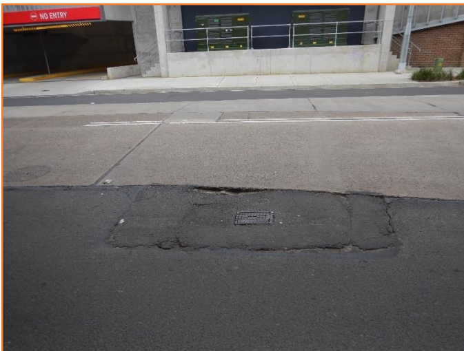
Figure 65: Reasonable - General condition of flexible and rigid pavement. Minor cracking observed.
