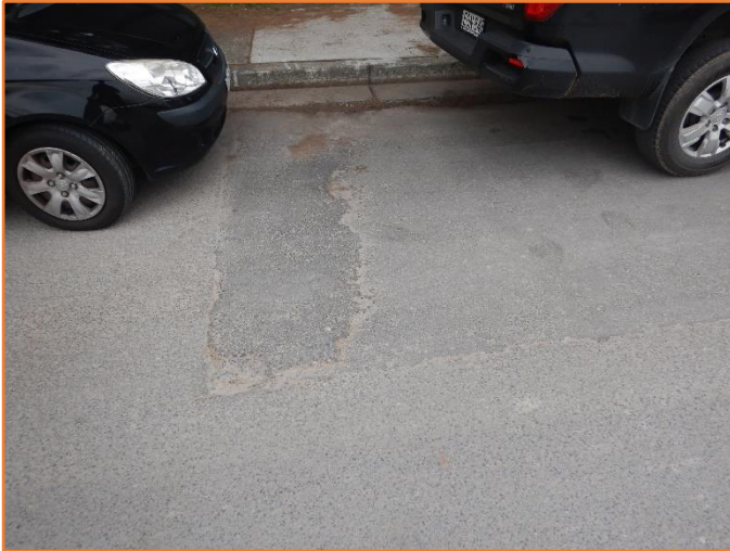
Figure 201: Reasonable - General condition of flexible pavement. Minor cracking observed. Previous repairs observed.
