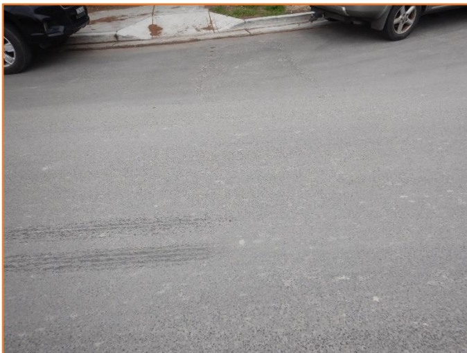
Figure 196: Reasonable - General condition of flexible pavement. Minor cracking observed.
