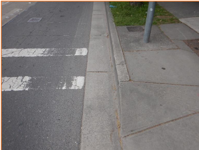
Figure 29: Reasonable - General condition of kerb and gutter. Minor cracking observed.
