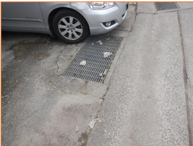
Figure 307: Reasonable - General condition of kerb and gutter. Minor cracking observed.
