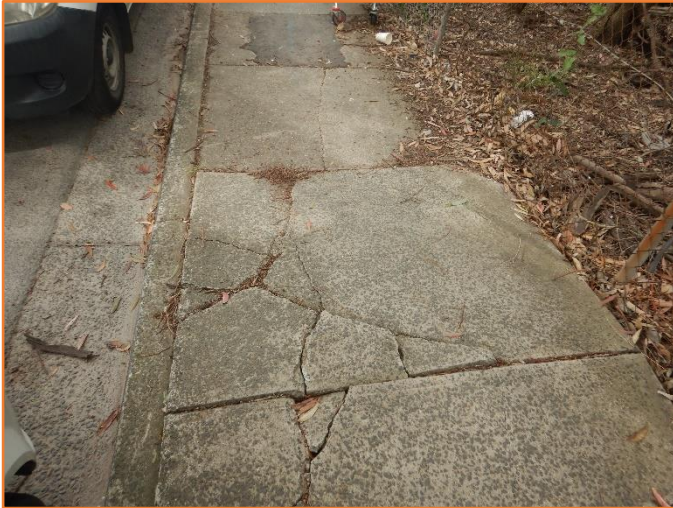
Figure 423: Poor - General condition of footpath. Extensive cracking observed.
