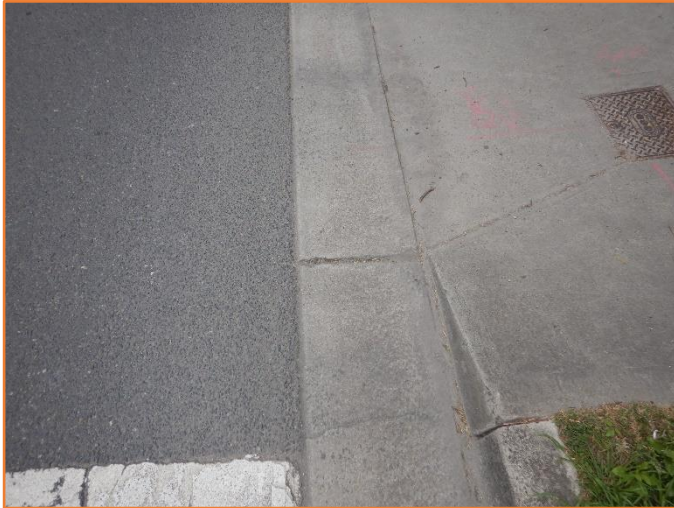
Figure 28: Reasonable - General condition of driveway layback. Minor cracking observed.
