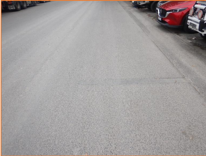
Figure 261: Reasonable - General condition of flexible pavement. Previous repairs observed.
