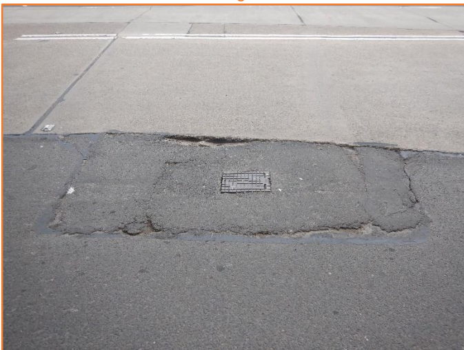
Figure 66: Reasonable - General condition of service pit. Minor cracking observed.
