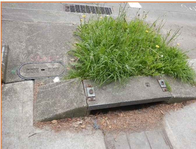
Figure 140: Reasonable - General condition of inlet pit and service pit.
