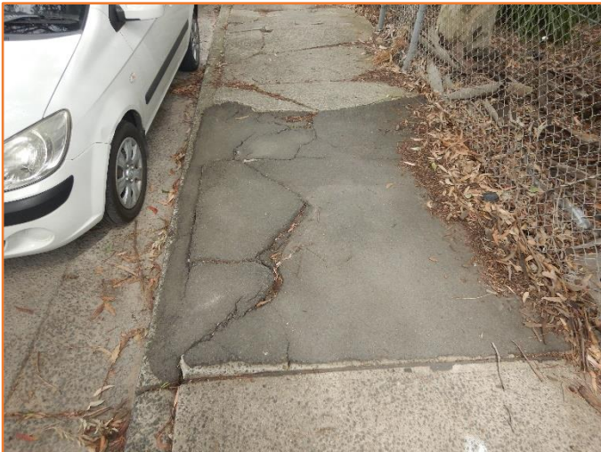
Figure 421: Poor - General condition of footpath. Extensive cracking and differential settlement observed.
