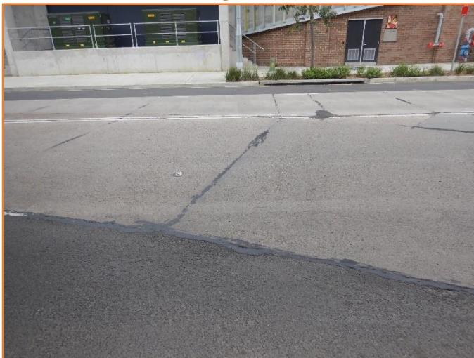
Figure 62: Reasonable - General condition of flexible and rigid pavement. Minor cracking observed.
