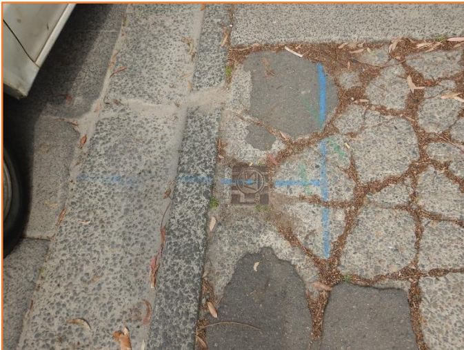
Figure 418: Reasonable - General condition of service pit. Extensive cracking observed.
