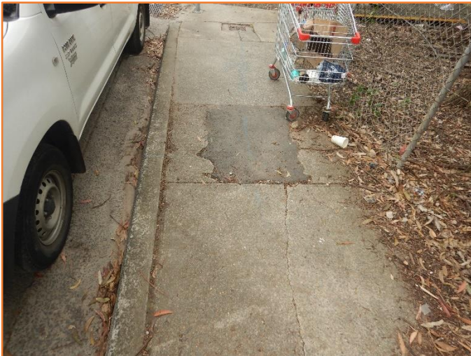
Figure 424: Reasonable - General condition of footpath. Major cracking observed. Previous repairs observed.
