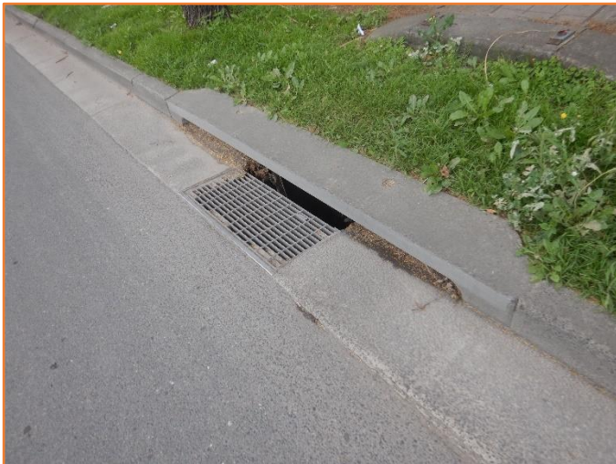
Figure 32: Reasonable - General condition of kerb inlet pit.
