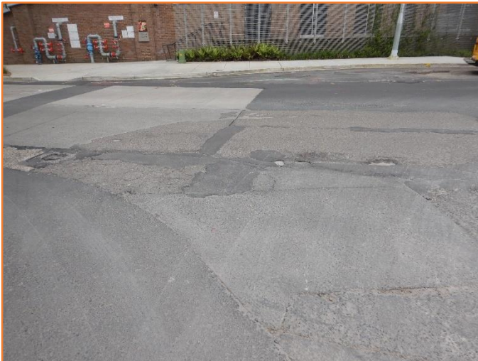
Figure 50: Poor - General condition of flexible pavement. Extensive cracking observed. Previous repairs observed.
