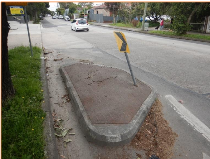
Figure 92: Reasonable - General condition of traffic island and signage. Minor rotation observed.
