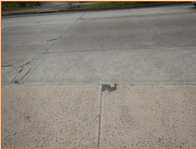
Figure 98: Reasonable - General condition of rigid pavement. Minor cracking observed.
