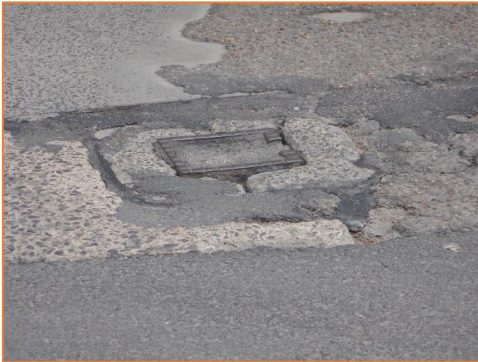
Figure 52: Reasonable - General condition of service pit. Minor cracking observed.
