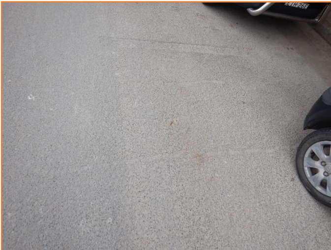
Figure 202: Reasonable - General condition of flexible pavement. Minor physical damage observed.
