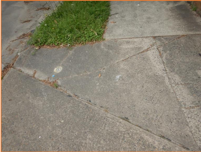
Figure 124: Reasonable - General condition of footpath. Major cracking observed.
