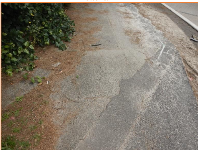
Figure 440: Reasonable - General condition of footpath. Minor cracking observed. Previous repairs observed.
