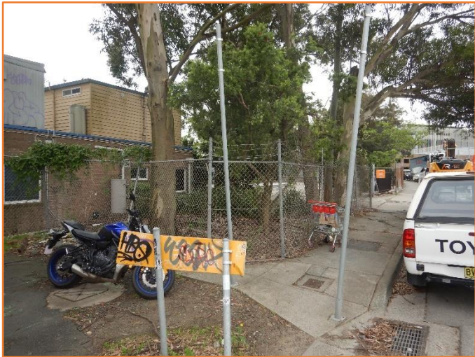
Figure 333: Reasonable - General condition of signage. Minor rotation observed.
