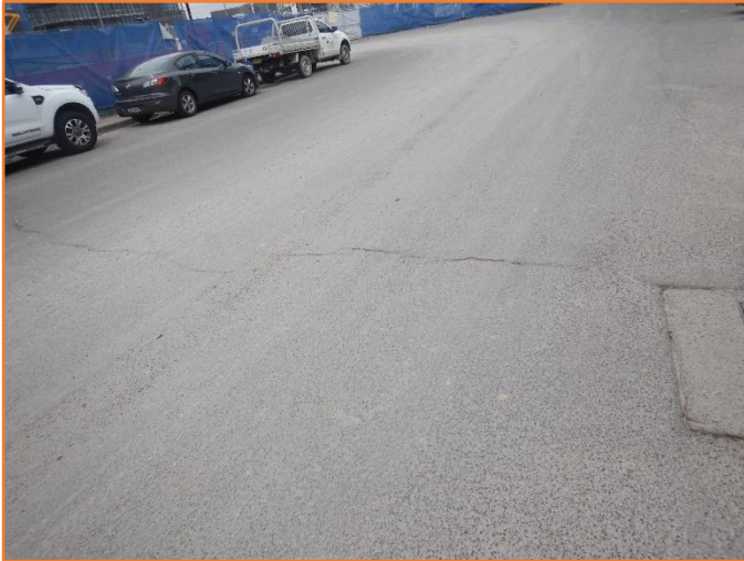
Figure 273: Reasonable - General condition of flexible pavement. Major cracking observed.
