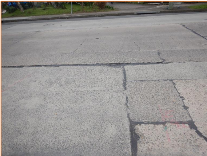
Figure 101: Reasonable - General condition of rigid pavement. Extensive cracking observed.
