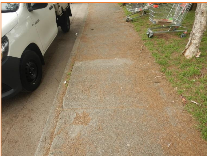
Figure 395: Reasonable - General condition of footpath. Minor cracking observed.
