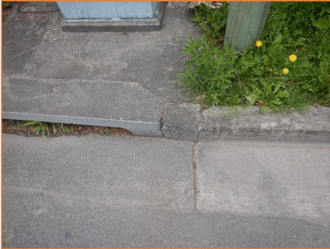
Figure 19: Reasonable - General condition of kerb inlet pit. Minor cracking observed.
