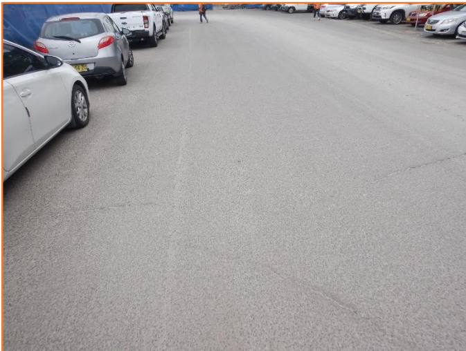
Figure 268: Reasonable - General condition of flexible pavement. Minor cracking observed.
