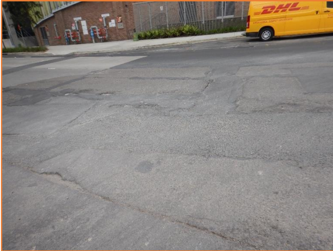
Figure 49: Poor - General condition of flexible pavement. Extensive cracking observed. Previous repairs observed.
