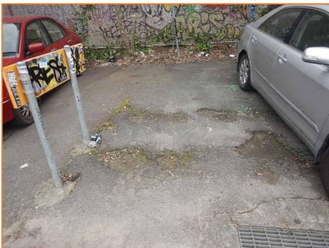
Figure 305: Reasonable - General condition of flexible pavement and signage. Moderate potholes and cracking observed.
