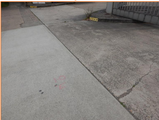
Figure 120: Reasonable - General condition of driveway crossover. Minor cracking observed.
