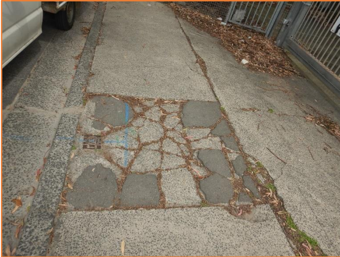
Figure 417: Reasonable - General condition of driveway crossover. Extensive cracking observed.
