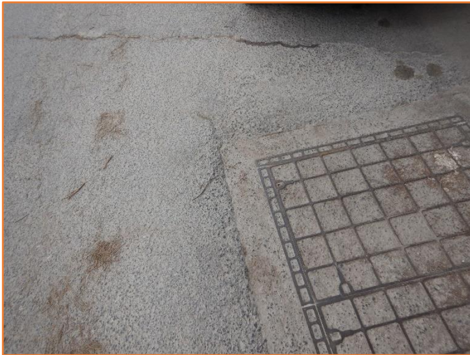
Figure 207: Reasonable - General condition of flexible pavement. Minor cracking observed.
