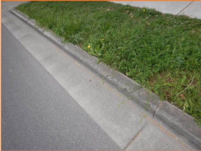
Figure 25: Reasonable - General condition of kerb and gutter. Minor spalling observed.
