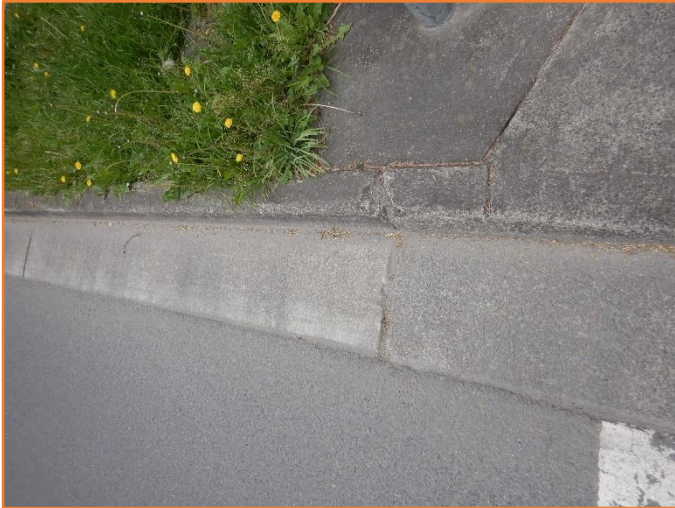
Figure 22: Reasonable - General condition of kerb and gutter. Major spalling observed.
