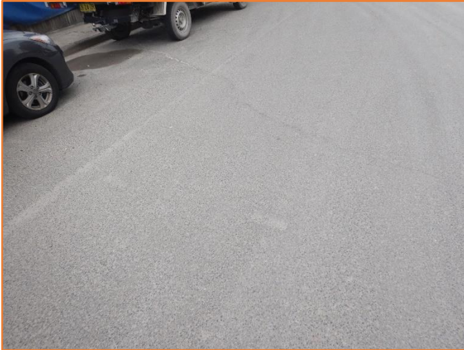
Figure 279: Reasonable - General condition of flexible pavement. Minor cracking observed.
