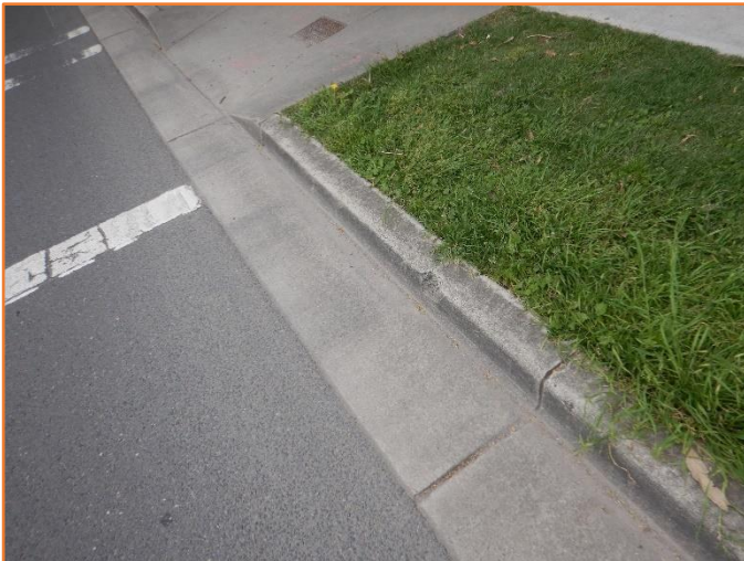
Figure 26: Reasonable - General condition of kerb and gutter. Minor spalling observed.
