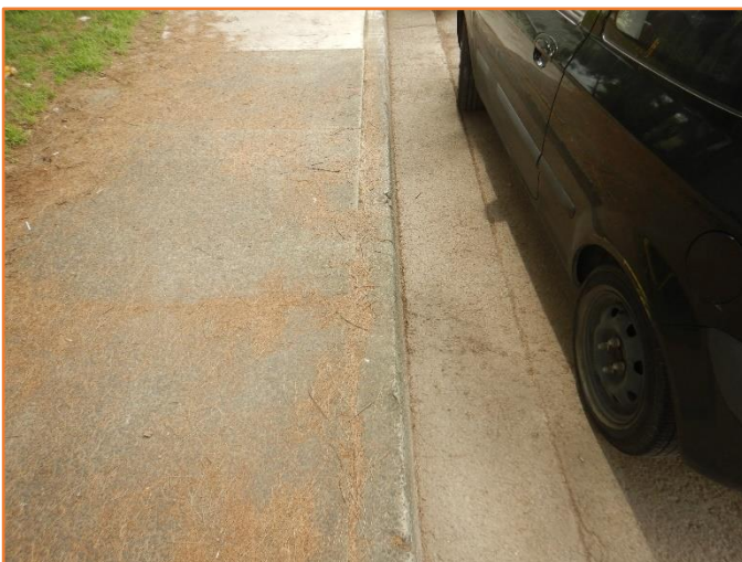
Figure 368: Reasonable - General condition of kerb and gutter. Minor spalling observed.
