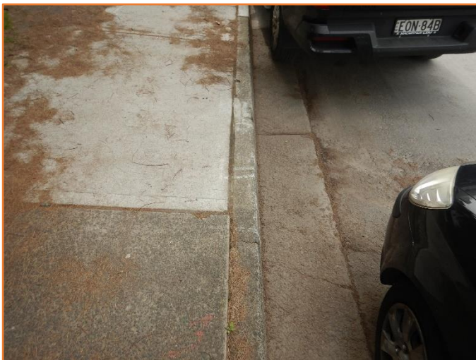
Figure 370: Reasonable - General condition of kerb and gutter. Minor cracking observed.
