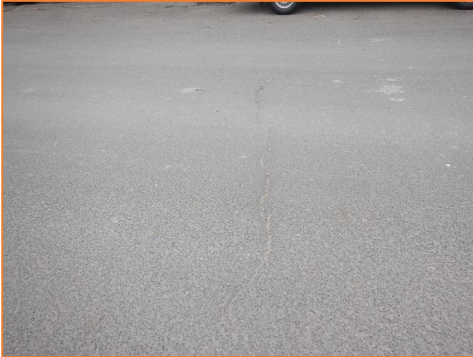
Figure 243: Reasonable - General condition of flexible pavement. Minor cracking observed.
