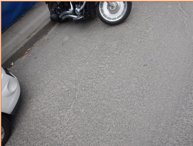
Figure 223: Reasonable - General condition of flexible pavement. Minor cracking observed.
