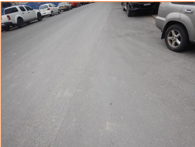
Figure 193: Reasonable - General condition of flexible pavement. Minor cracking observed.
