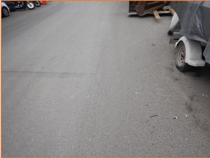
Figure 219: Reasonable - General condition of flexible pavement. Minor cracking observed.
