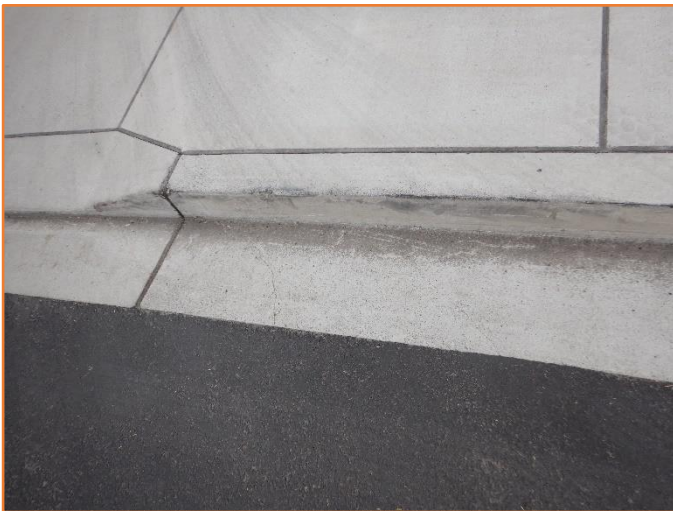
Figure 2: Reasonable - General condition of kerb and gutter. Minor spalling observed.
