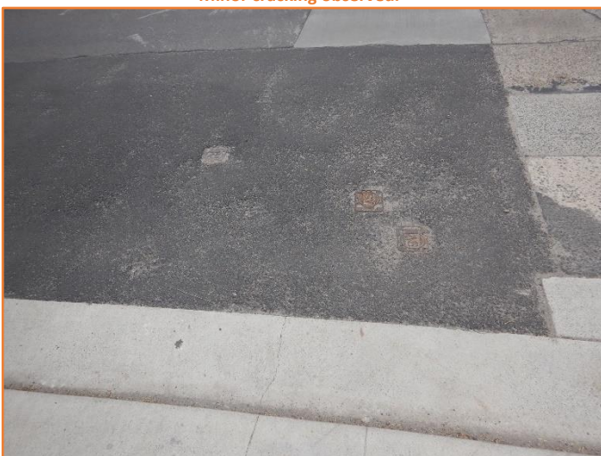
Figure 105: Reasonable - General condition of flexible pavement.
