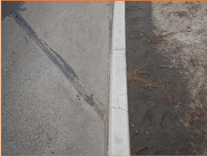
Figure 43: Reasonable - General condition of kerb and gutter. Minor hairline cracking observed.
