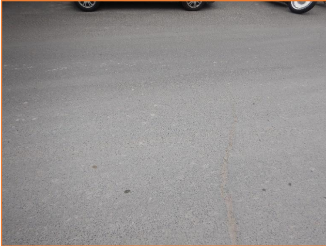
Figure 222: Reasonable - General condition of flexible pavement. Minor cracking observed.
