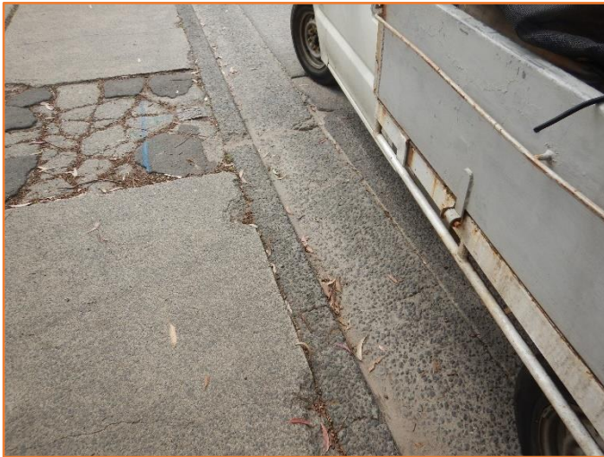
Figure 342: Reasonable - General condition of kerb and gutter. Minor cracking observed.
