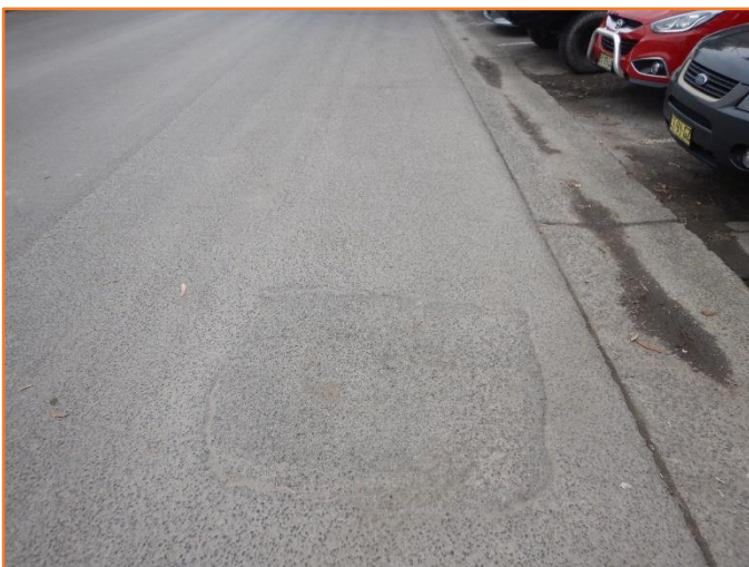
Figure 248: Reasonable - General condition of flexible pavement. Previous repairs observed.
