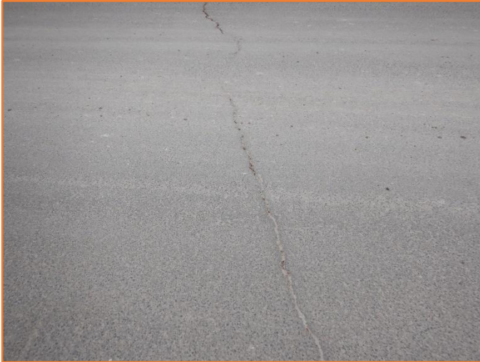
Figure 270: Reasonable - General condition of flexible pavement. Major cracking observed.
