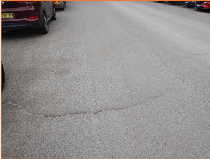
Figure 258: Reasonable - General condition of flexible pavement. Major cracking observed.
