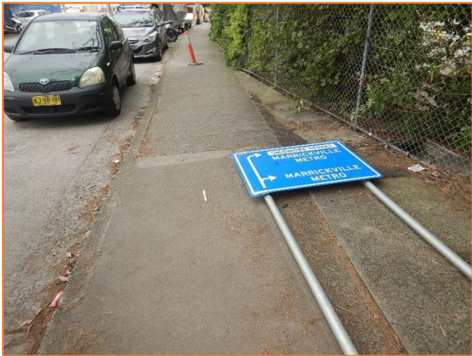
Figure 403: Reasonable - General condition of footpath and signage. Major physical damage observed.
