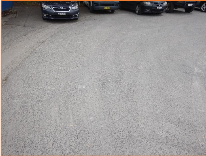
Figure 291: Reasonable - General condition of flexible pavement. Minor physical damage observed.
