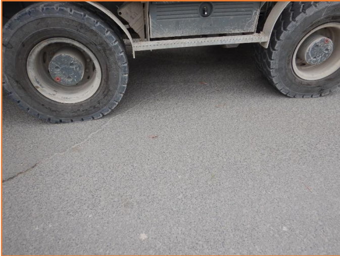
Figure 231: Reasonable - General condition of flexible pavement. Minor cracking observed.
