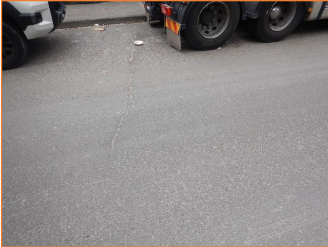
Figure 213: Reasonable - General condition of flexible pavement. Minor cracking observed.
