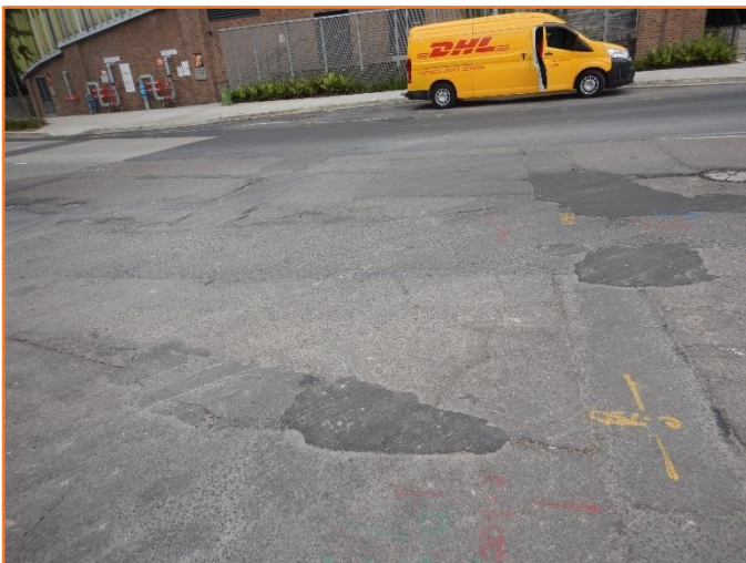
Figure 48: Poor - General condition of flexible pavement. Extensive cracking observed. Previous repairs observed.
