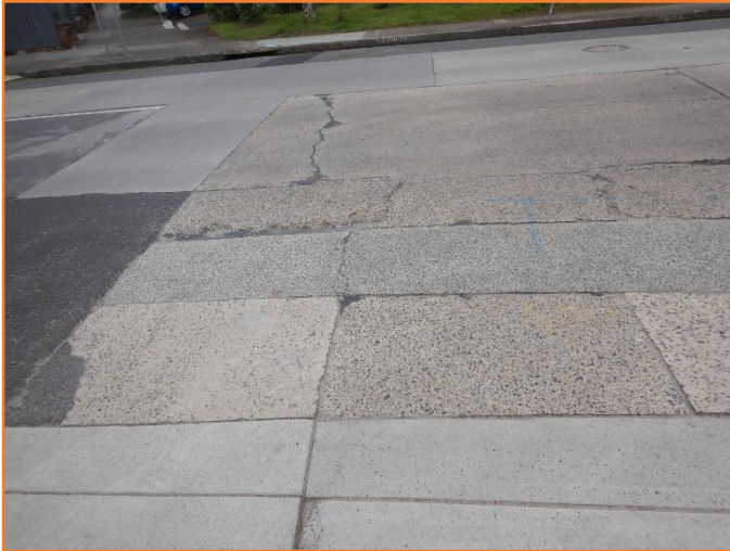
Figure 103: Reasonable - General condition of rigid pavement. Extensive cracking observed.
