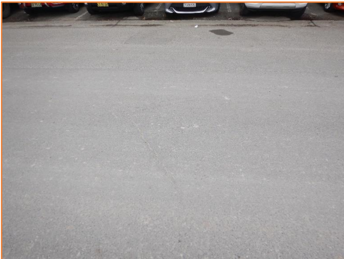
Figure 247: Reasonable - General condition of flexible pavement.
