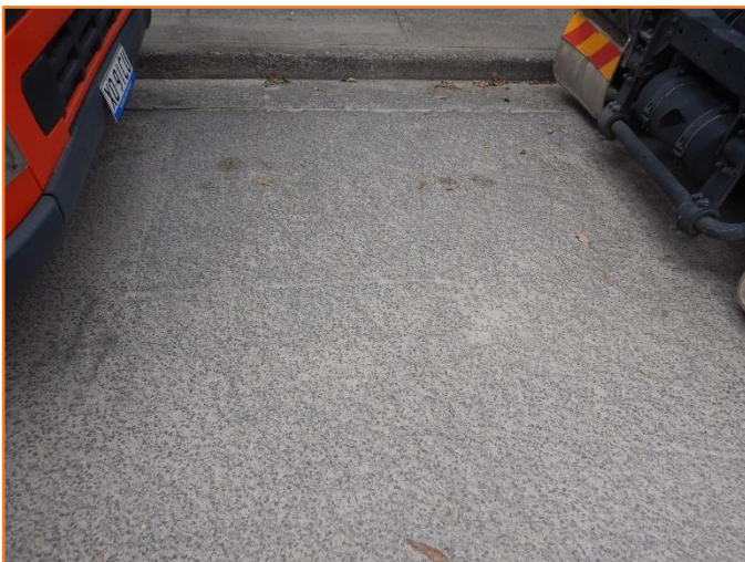
Figure 215: Reasonable - General condition of flexible pavement. Minor physical damage observed.
