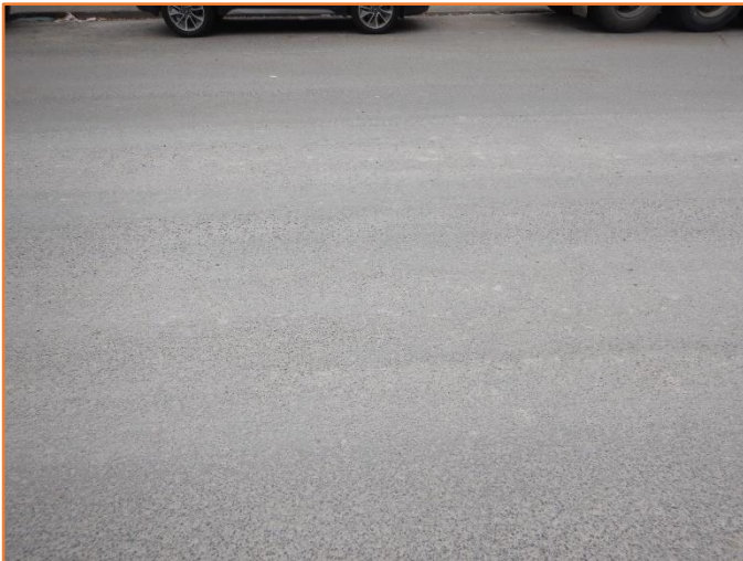
Figure 262: Reasonable - General condition of flexible pavement.
