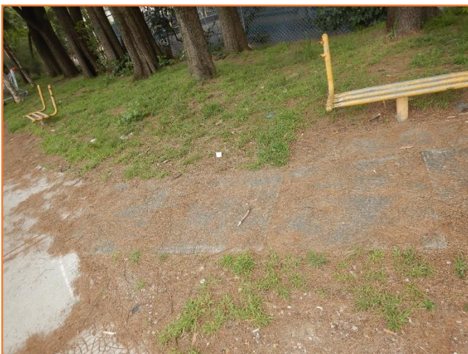
Figure 386: Reasonable - General condition of footpath. Minor cracking observed.
