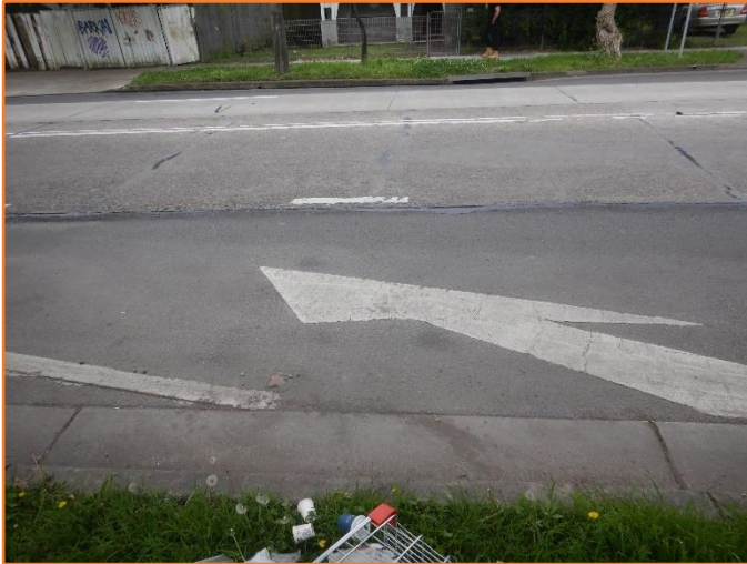
Figure 88: Reasonable - General condition of flexible and rigid pavement.
