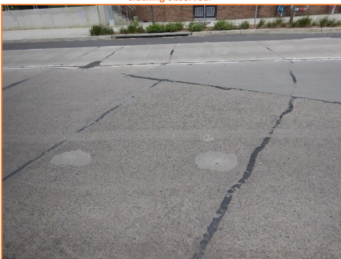
Figure 60: Reasonable - General condition of rigid pavement. Minor cracking observed.
