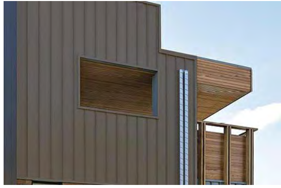
2. Metal Wall Sheeting Enseam - Jasper
