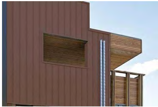
1. Metal Wall Sheeting Enseam - Terrain
