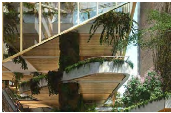
13. Timber Soffit to External Recreation Area
