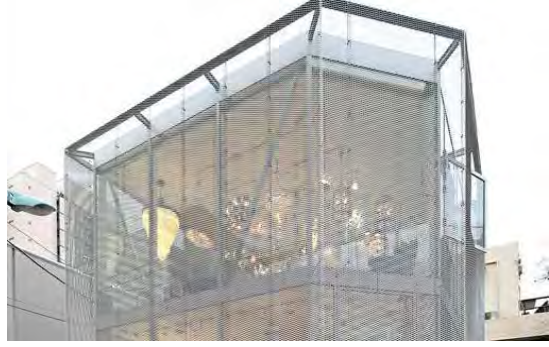
5. Wire Mesh Screen/ Perforated Screen - Stainless Steel with Black Reveal
