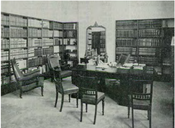
Judge's Chamber in former Department of Public Works Building Source: NSW Department of Public Works Annual Report Year ended 30 June 1969
