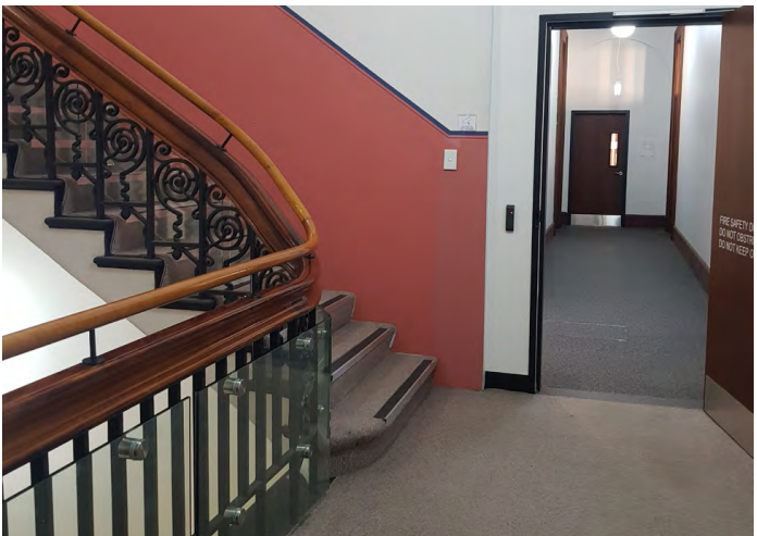
The central stair. The wall on the northern side of the staircase was constructed to compartmentalise each floor from the spread of smoke in case of fire. Source: GBA Heritage, 2020
