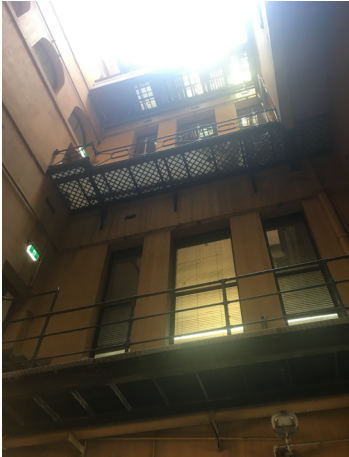
iii. Phillip Lane Light Well
