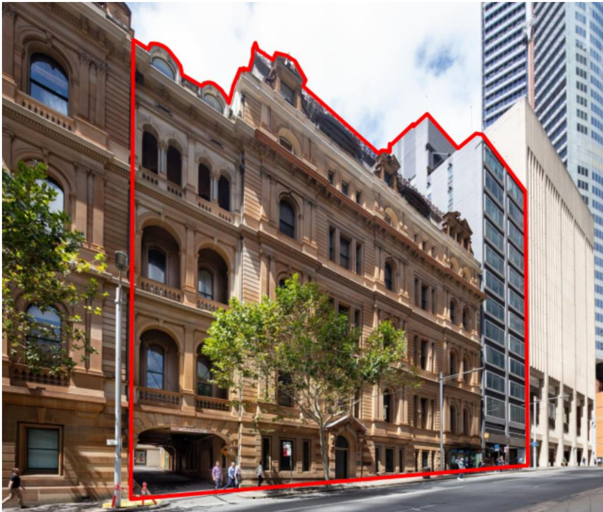
Figure 1.2: Existing frontages of 50-52 Phillip Street outlined in red (Source: Built 2020)
