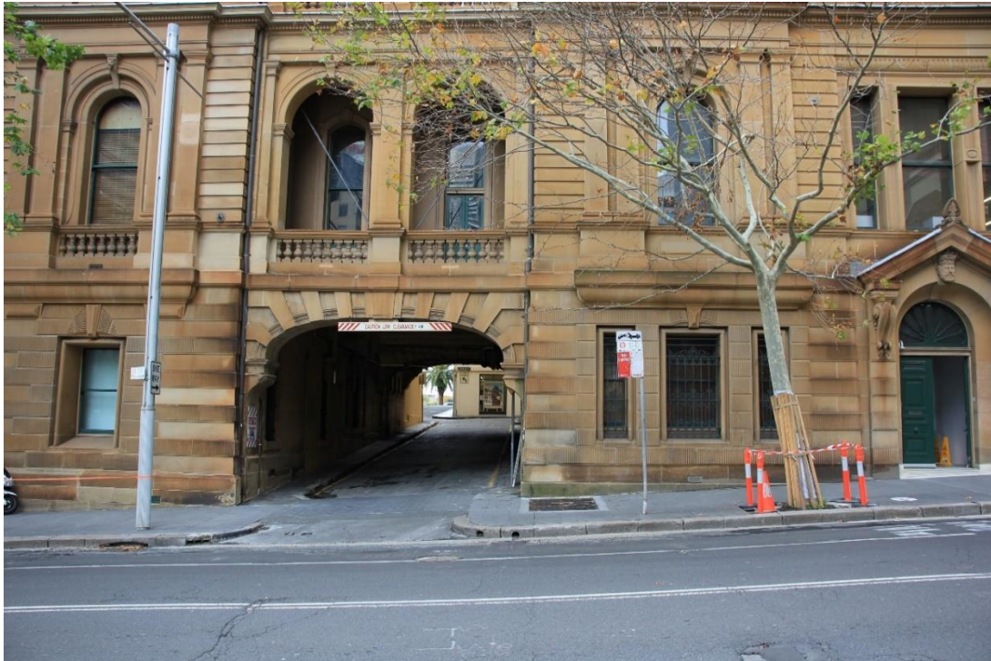
Figure 4.13: 50 Phillip Street facade with Phillip Lane underpass (Source: Curio 2020)
