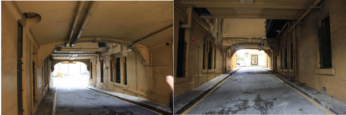
Figure 4.15: Phillip Lane underpass with Chief Secretary's Building & 50 Phillip Street on either side (Source: Curio 2020)
