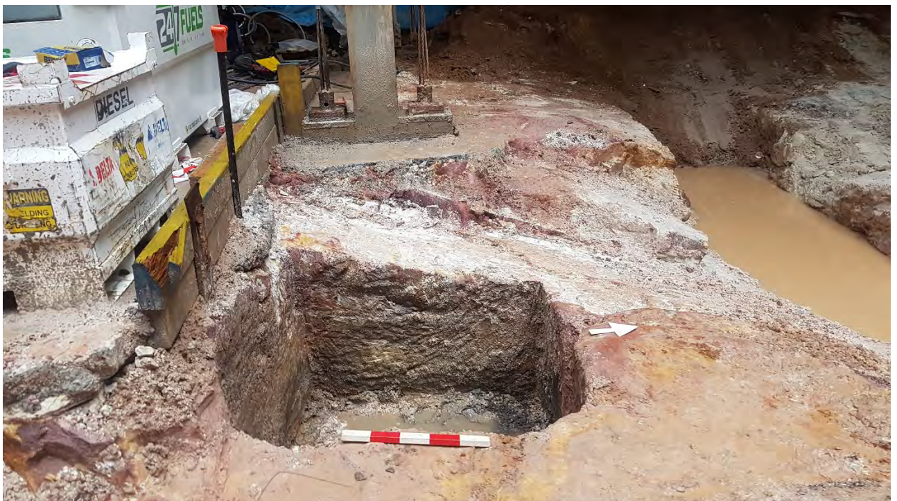
Figure 5-2 Rock cut cistern/cess pit, Education Building, south west, looking west. (Source: Curio 2020)
