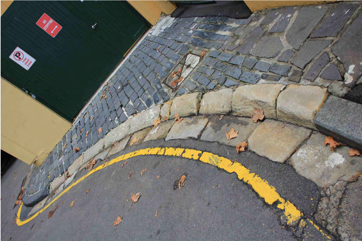
Figure 4-5 Remnant stone kerbing at the elbow of Phillip Lane. (Source: Curio 2020)
