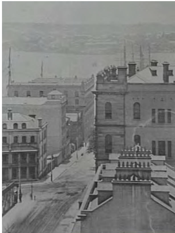
Figure 3-13: 1890 Photograph of Phillip Street 'View showing ships moored at Circular Quay in Sydney Cove. Chief Secretary's Department building behind terraces at R. Goldsborough Mort wool store building (Farmers & Graziers) L at bottom of street.' (Source: City of Sydney SRC9899)
