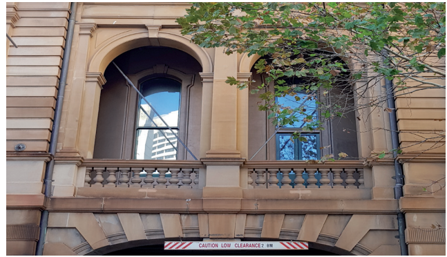
Figure 3.14 structural bracing to the first floor balcony spanning over Phillip Lane Source: GBA Heritage, 2020
