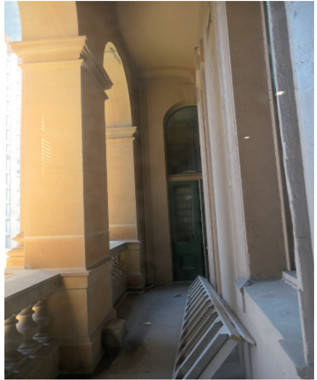
Figure 3.28 Access to the Chief Secretary's Building via the octagonal room, and balcony on levels 2-5. Source: GBA Heritage, 2020
