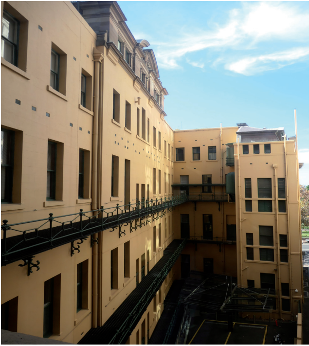
Figure 3.35 The floor covering the walkway on level 4 is a mix of glass panels and timber boards Source: GBA Heritage, 2020
