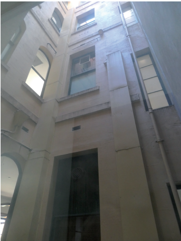
Figure 3.37 Views looking up from the central light well Source: GBA Heritage, 2020
