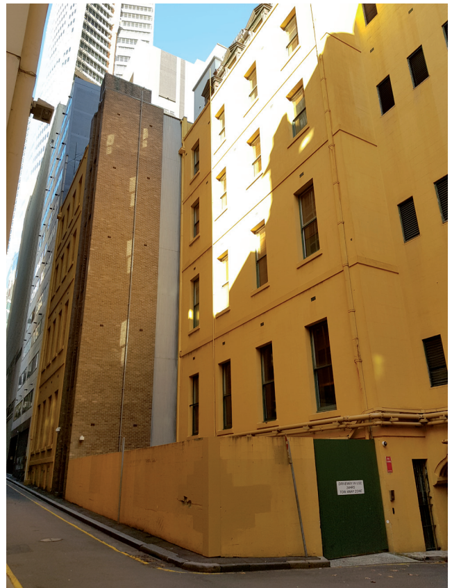
Figure 3.38 The east facade of 50 Phillip Street in cement-rendered brickwork. The fire stairs in a new brick wall is attached to the building. Source: GBA Heritage, 2020
