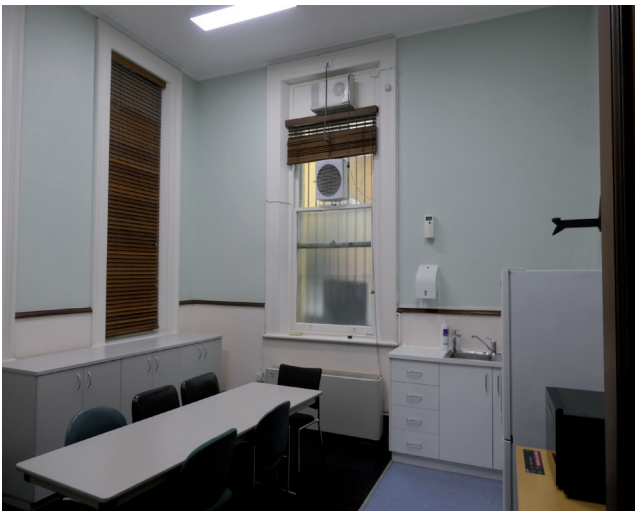
Figure 3.88 Vents and mechanical fans installed within the window sashes on ground level. Source: GBA Heritage, 2020
