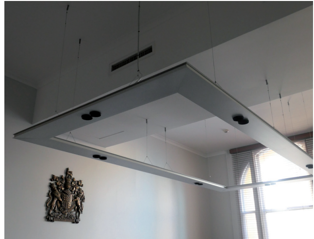
Figure 3.68 Suspended ceiling in an office room on level 5. Typical Coat of Arms (Some significance) - late 20 th century. Source: GBA Heritage, 2020
