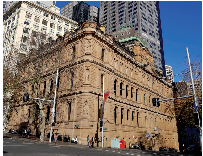
Figure4.1 Chief Secretary's Building Source: GBA Heritage, 2020
