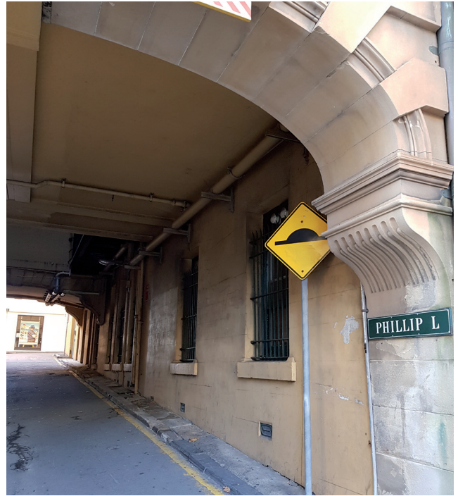
Figure 3.25 The north facade of the building over Phillip Lane. Source: GBA Heritage, 2020
