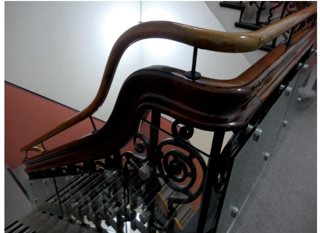
Figure 3.91 Central open stair. A second handrail was installed to increase balustrade height. The glass balustrade was installed for safety reasons. Source: GBA Heritage, 2020
