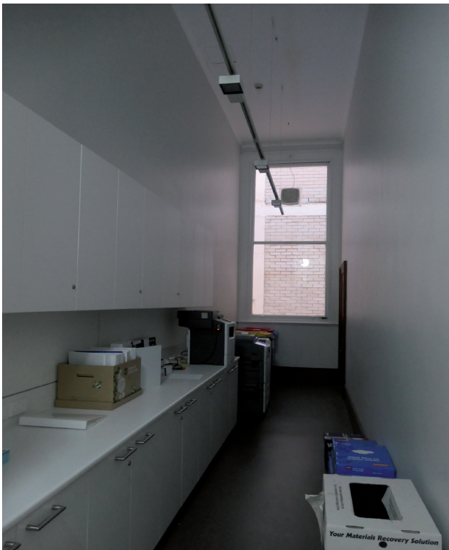
Figure 3.98 Renovated kitchen on level 3. A mechanical fan installed within the window sashes. Source: GBA Heritage, 2020
