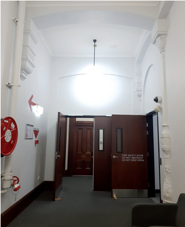
Figure 3.96 Main hall on ground level Source: GBA Heritage, 2020
