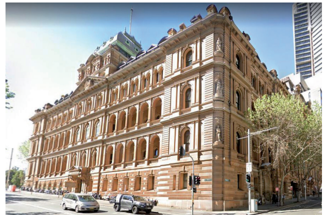
Figure 3.20 The Chief Secretary's Building located on the northern side of the subject site, adjacent to the former Department of Public Works building Source: Google Map, 2020
