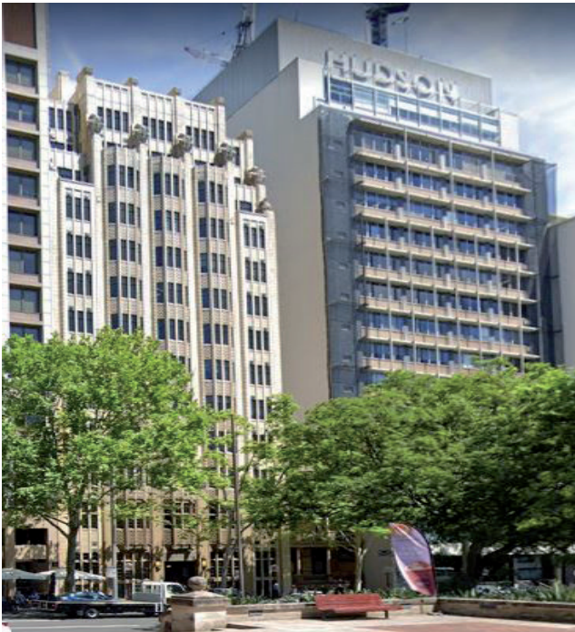
Figure 3.26 Looking to BMA House from the Royal Botanic Garden Source: Google Map, 2020
