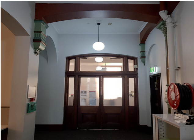
Figure 3.43 Level 5, looking across existing corridor Source: GBA Heritage, 2020
