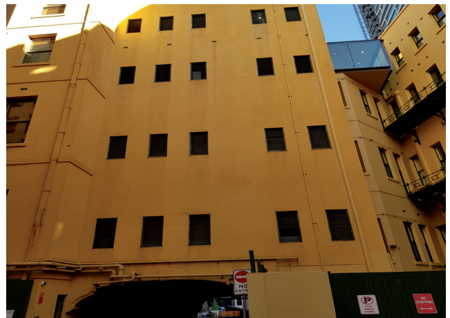
Figure 3.34 The rear facade of the building over Phillip lane. Source: GBA Heritage, 2020
