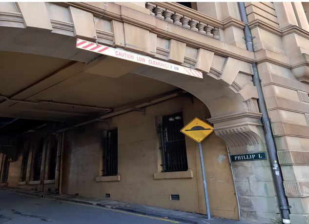
Figure 3.31 North side of the building over Phillip Lane Source: GBA Heritage, 2020
