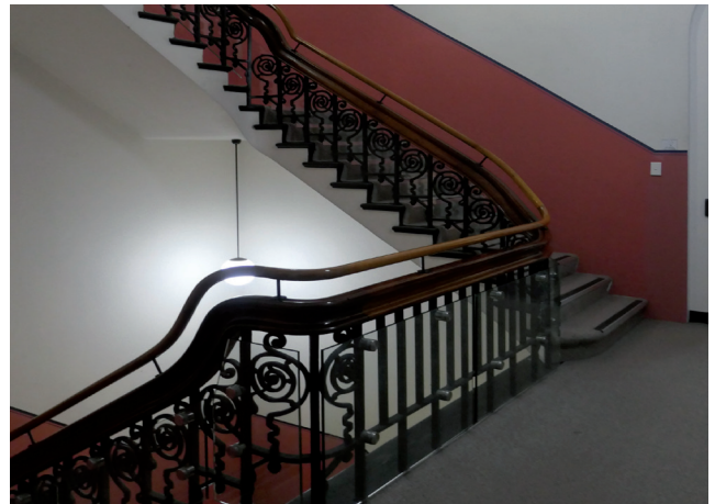
Figure 3.38 Main central staircase Source: GBA Heritage, 2020
