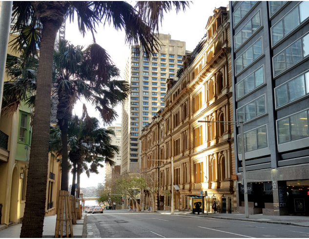
Figure 3.29 Looking north towards the former Department of Public Works building at 50 Phillip Street. Source: GBA Heritage, 2020
