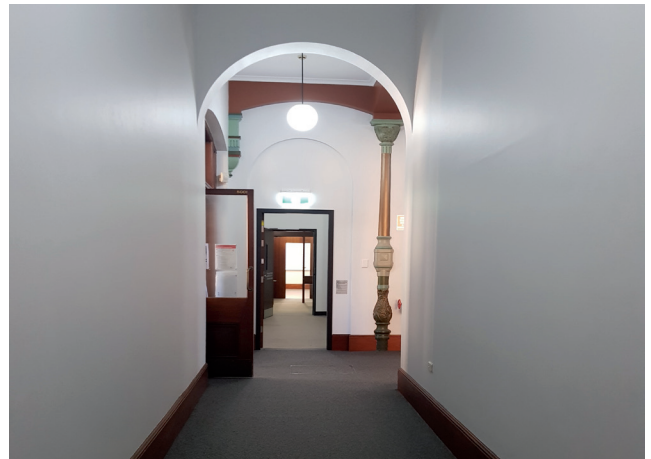
Figure 3.44 Level 5, looking through the central staircase, showing the cast iron column partially enclosed Source: GBA Heritage, 2020
