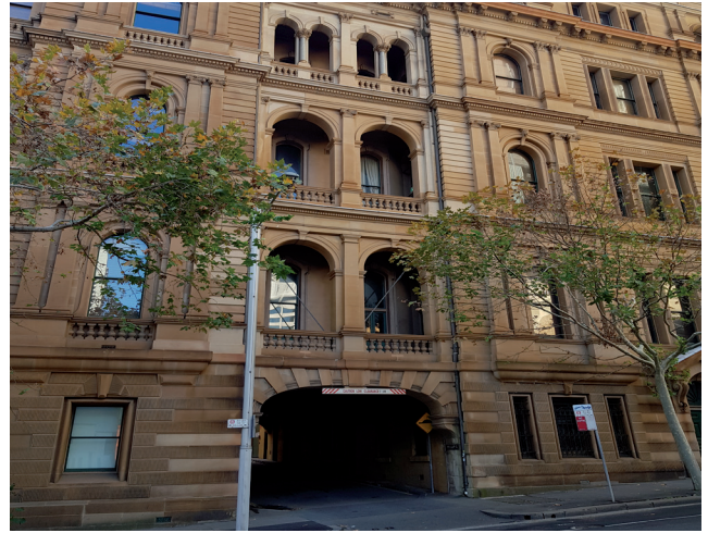
Figure 3.30 The connection between the former Department of Public Works building and Chief Secretary's Building over Phillip Lane. Source: GBA Heritage, 2020
