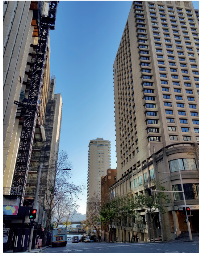
Figure 3.16 Looking northward to Phillip Street from the intersection of Bridge and Phillip Streets Source: GBA Heritage, 2020
