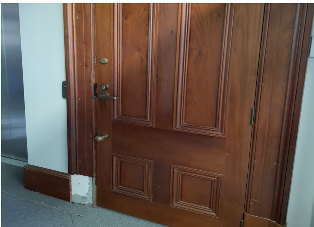
Figure 3.39 A broken door architrave on level 6, showing an original brass knob and a new lever door handle Source: GBA Heritage, 2020
