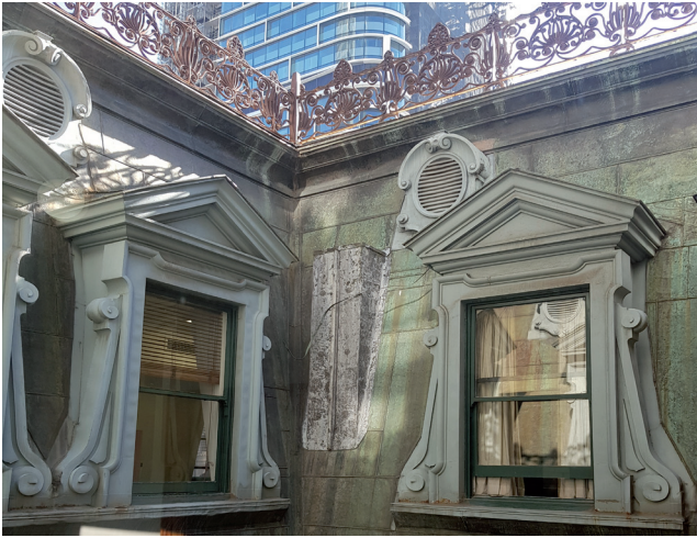
Figure 3.35 Mansard roof and dormer windows within the lightwell, decorative iron balustrade around the perimeter of the light well, and metal louvred vents. Source: GBA Heritage, 2020
