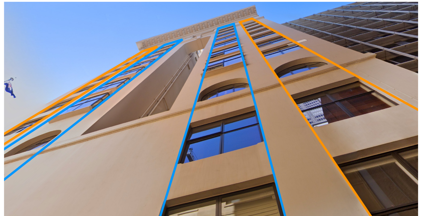
Astor Apartments - Phillip Lane Facade
