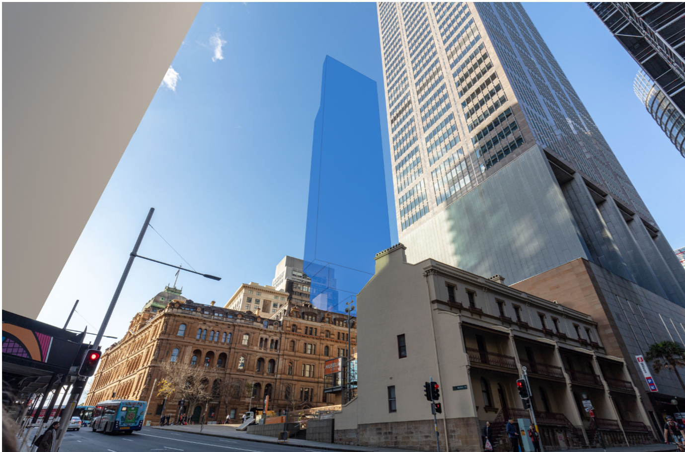
Bridge Street View 2
