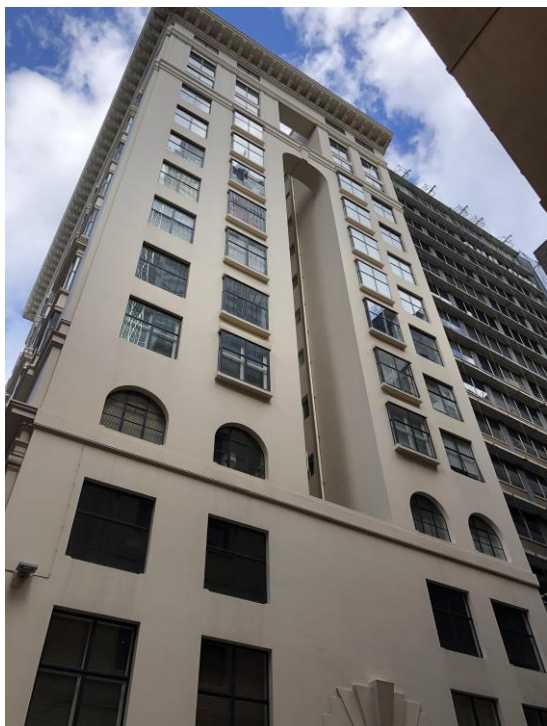
Rear of 123-125 Macquarie Street, "The Astor"
