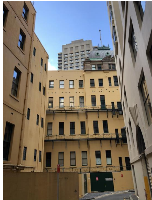
Rear of Former Chief Secretary's Building fronting Phillip Lane
