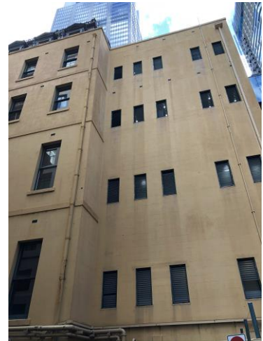
Rear of the heritage-listed sandstone building fronting Phillip Lane
