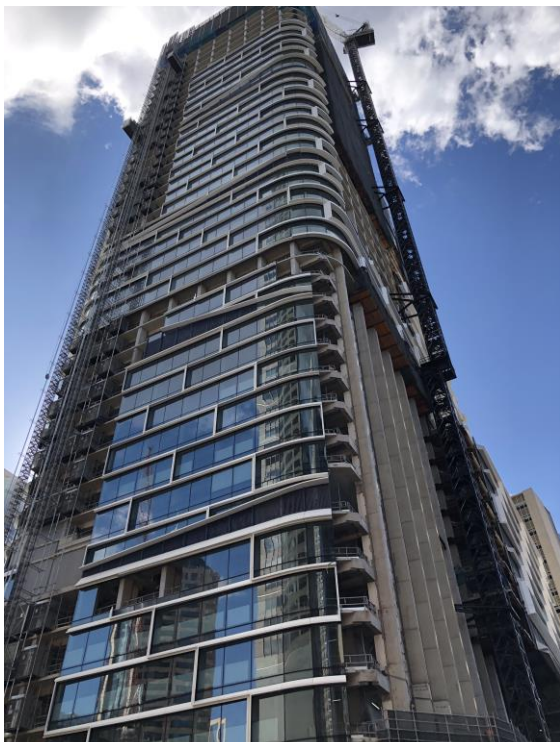
50 storey Quay Quarter Tower development under construction
