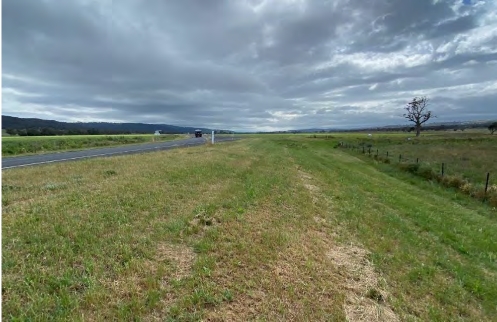
Plate 1: Degraded and managed roadside
