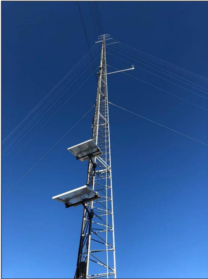
Figure A-9: Example of a meteorological mast
