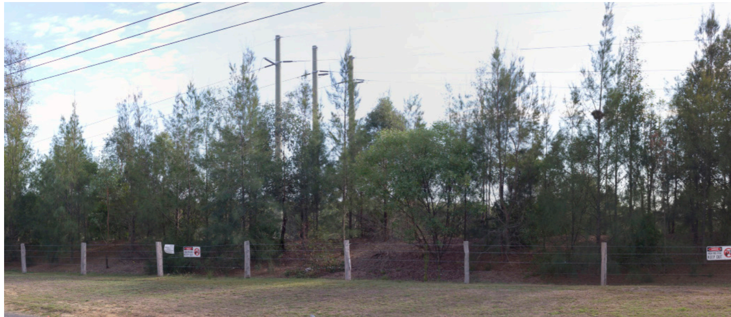
Image 30. Example of landscape screening along the boundary of a substation - Rothbury NSW
