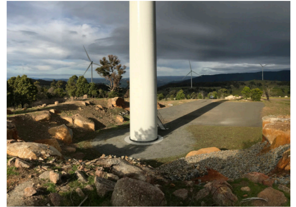
Image 3 Crane Hardstand Area (Source: NGH)
