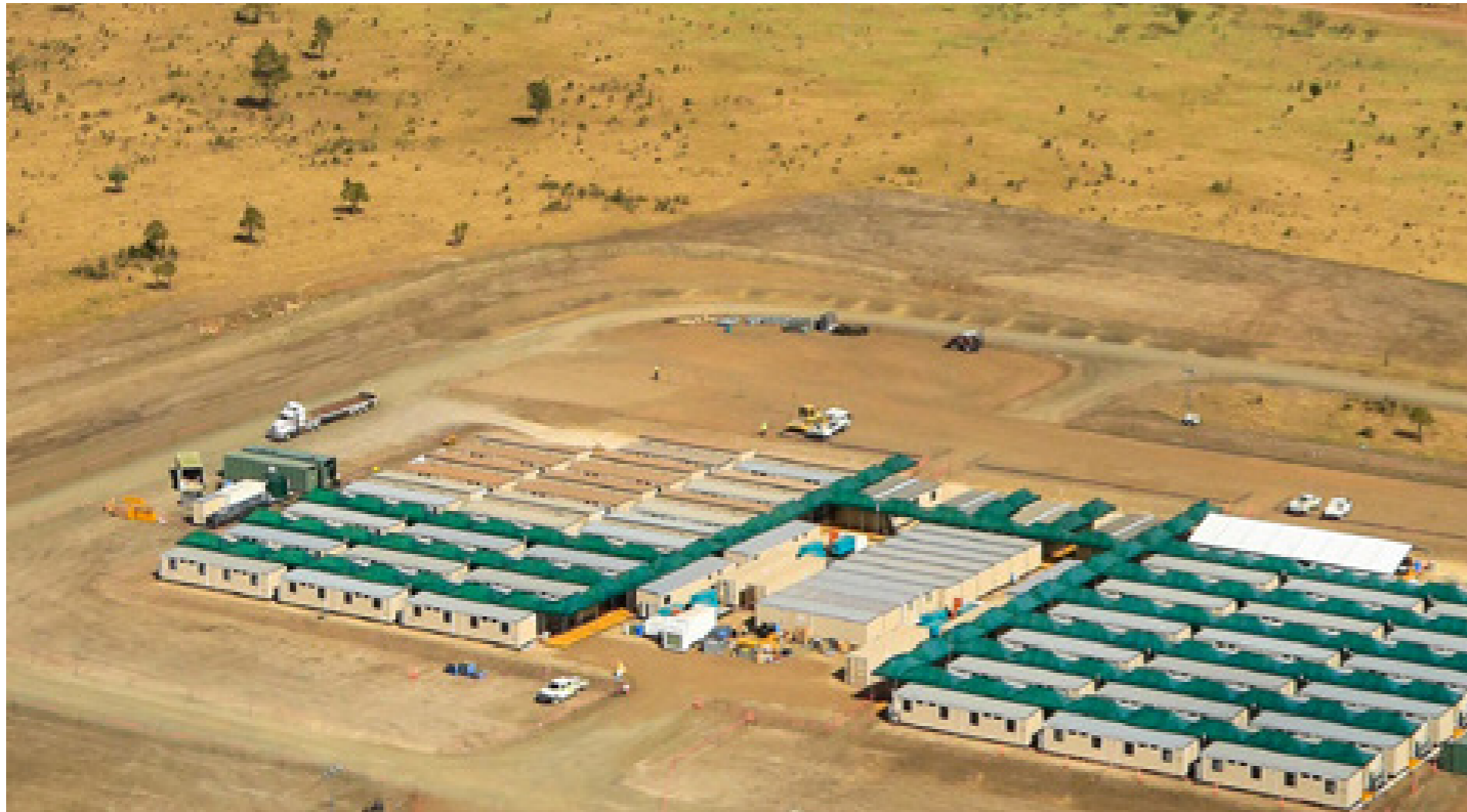
Image 31 Typical aerial view of temporary workers accommodation (Source: Ausco Modular Pty Ltd)
