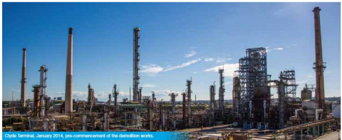
FIGURE 4-2: HISTORIC IMAGE OF PREVIOUS CLYDE TERMINAL, JANUARY 2014 5
