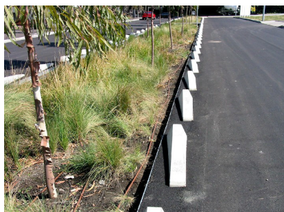
Figure 30: Water sensitive parking areas are required for parking layouts 100 cars or greater.
