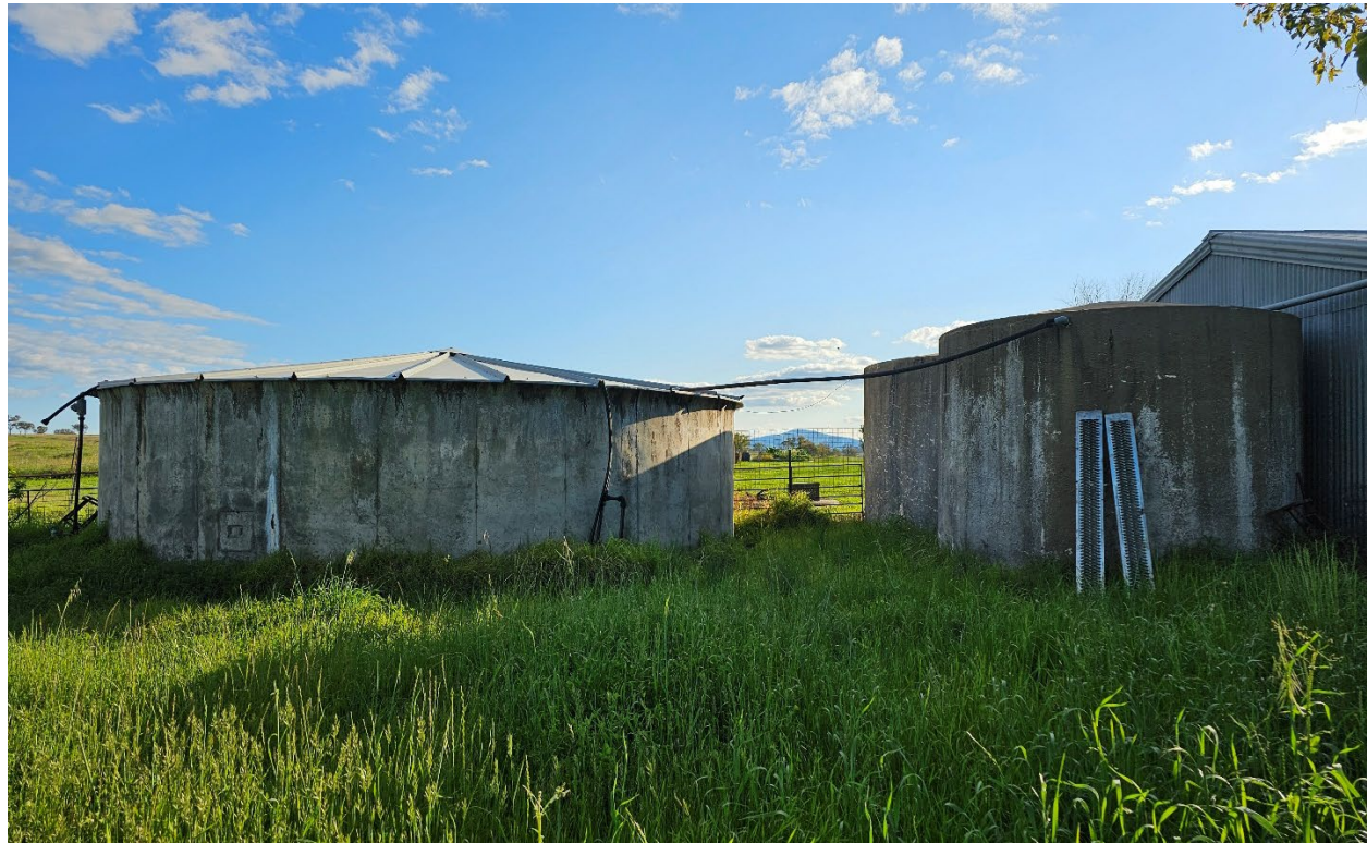
Figure 2-11 Change 1a – Water tanks occurring within proximity to the shed
