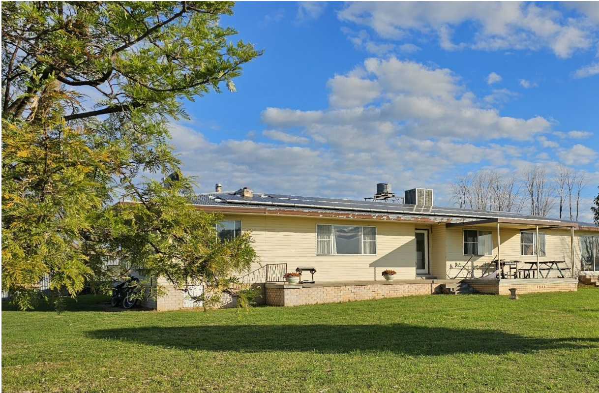
Figure 2-10 Change 1a – Residence – proposed for demolition
