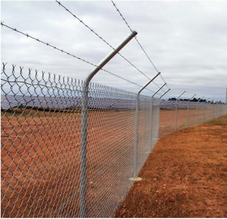
Figure 3-3 Example of security fencing with barbed wire.
