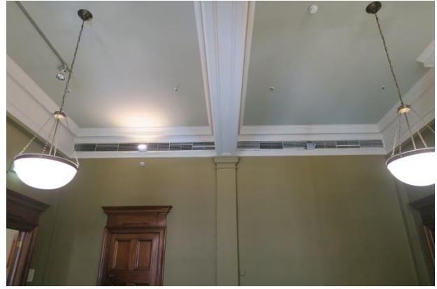
Figure 131 – Ceiling in S3.20 showing insertion of services around corning
