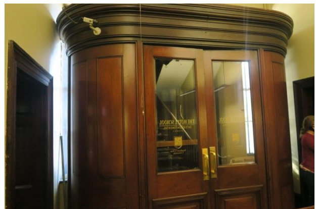
Figure 41 – D17A – later air-lock enclosure in stair hall
