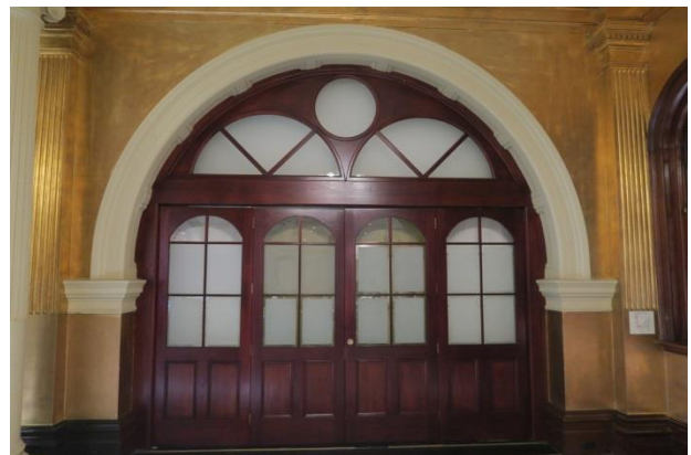
Figure 73 – S2.17 – later timber partitions between S2.17 and S2.18 Source: Urbis
