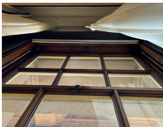
Figure 5 Existing hardware to centre of top sash to be retained.
