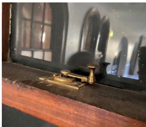
Figure 6 Existing sash fastener to S.17
