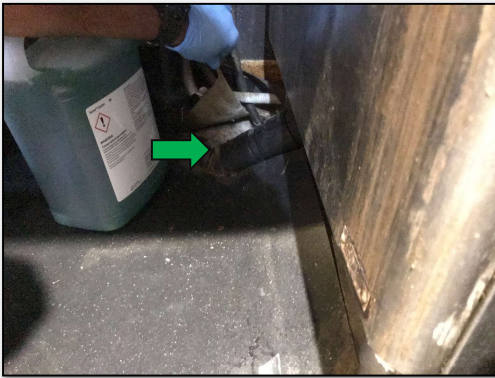
Photo 3: Level 32, internal, back of house flooring under vinyl - non-asbestos compressed cement sheet.
