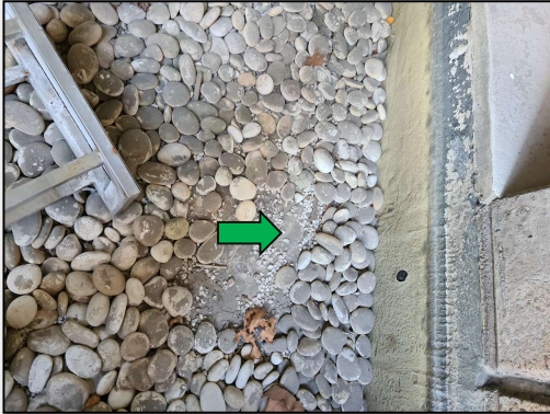
Photo 13: Level 5, external, northern water feature flooring membrane - non-asbestos bituminous membrane.
