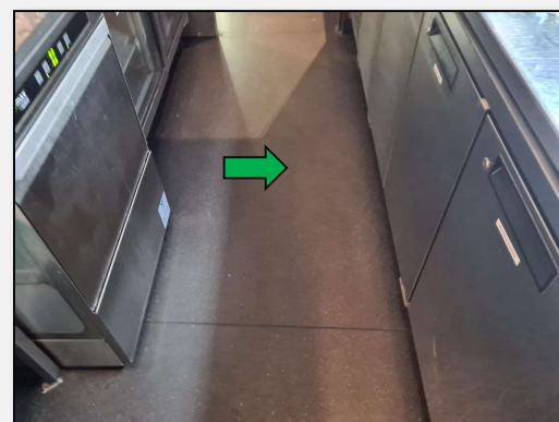
Photo 10: Level 5, internal, bar flooring - non-asbestos sheet vinyl.
