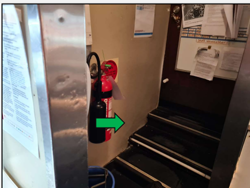
Photo 11: Level 5, internal, kitchenette adjacent bar, wall lining - non-asbestos fibre cement sheet.
