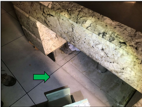
Photo 9: Level 6, internal, along floor joints between floor tiles, Bain Marie - non-asbestos mastic sealant.
