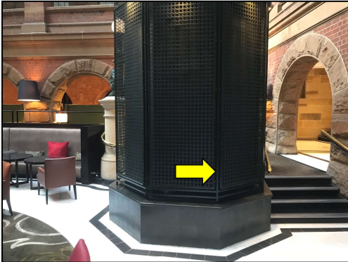
Photo 19: Level 5, internal, metal enclosure in lobby area - Lead-containing dark green coloured paint system.
