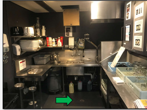
Photo 4: Level 32, internal, back of house flooring - non-asbestos sheet vinyl.
