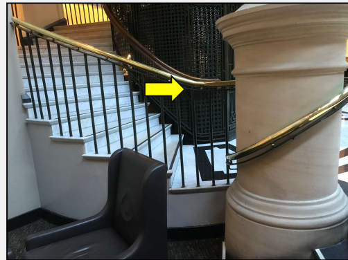
Photo 18: Level 5, internal, balustrade and railings in lobby area - Lead-containing dark green coloured paint system.
