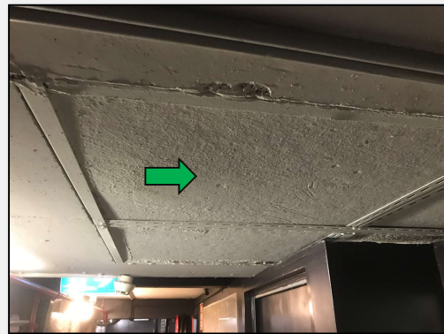
Photo 6: Level 32, internal, bar sitting area under flooring - non-asbestos bituminous membrane.
