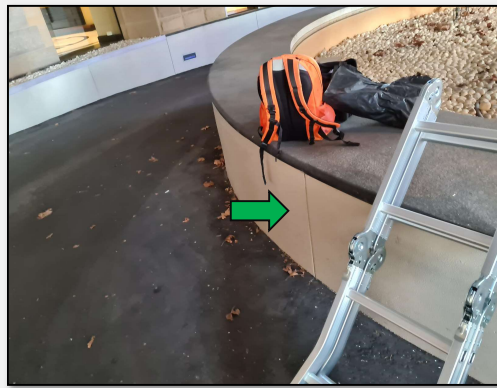
Photo 22: Level 5, external, outer wall of water feature - Non-lead containing beige coloured paint system.
