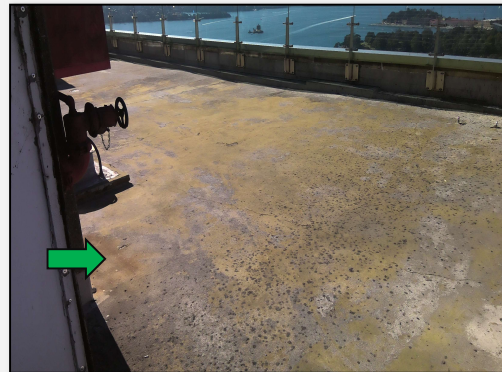
Photo 2: Level 32, internal, lower layer rooftop floor - non-asbestos bituminous membrane.
