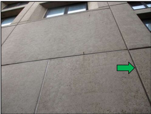
Photo 15: Level 8, external, eastern lower face - non-asbestos mastic sealant.
