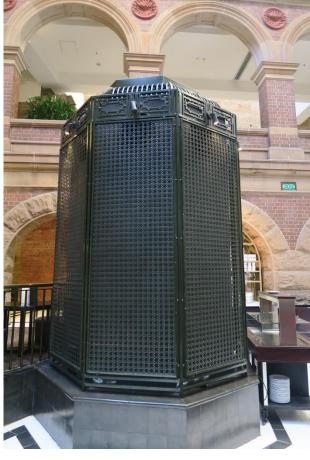
Figure 162 – Decorative vent cage referential to the caged lift (1980s' replica fabric)
