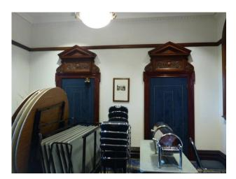
Figure 90 – Refurbished baize doors (D74 & D75) in S3.13
