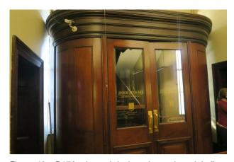
Figure 43 - D17A - later air-lock enclosure in stair hall
