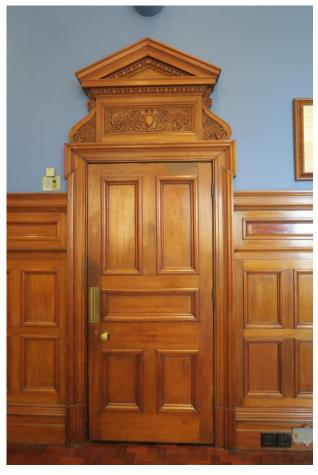
Figure 84 - D84 original door in S.3.14 – the Premier's Room (function space)
