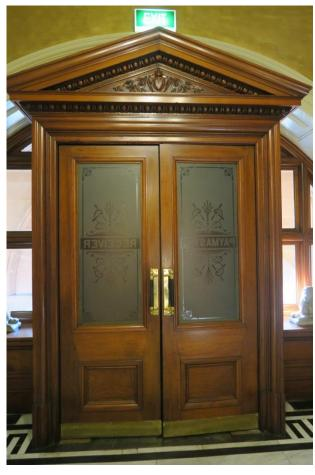
Figure 76 – D66 – lobby timber doors with "Paymaster" and "Receiver" etched glass
