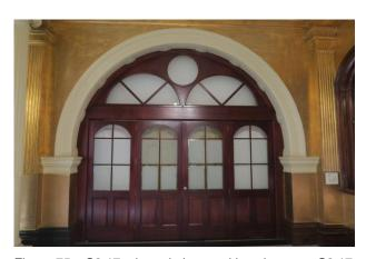
Figure 75 – S2.17 – later timber partitions between S2.17 and S2.18  $\,$
