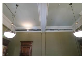
Figure 133 – Ceiling in S3.20 showing insertion of services around cornicing
