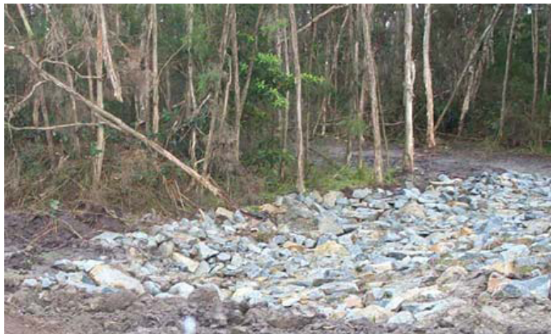
Rock Armouring, (EPA, 2004)
