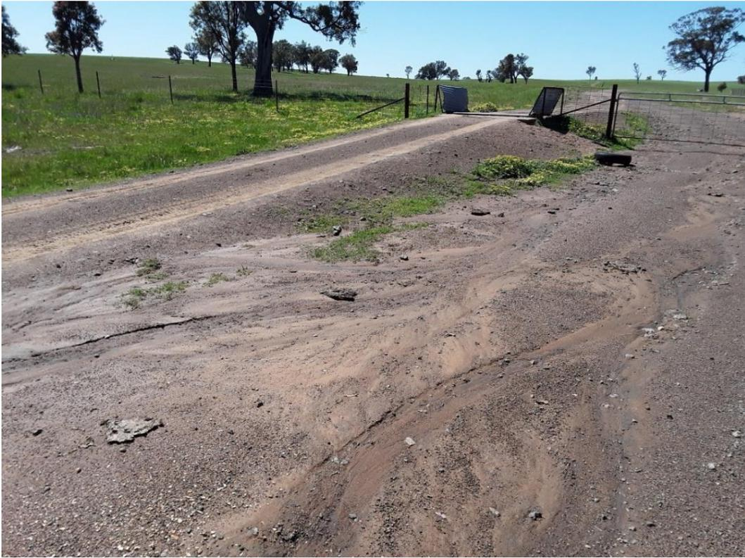
Photo 9-5: Washout and drainage rills on road and adjacent track, on unvegetated soils in the north east of the study area
