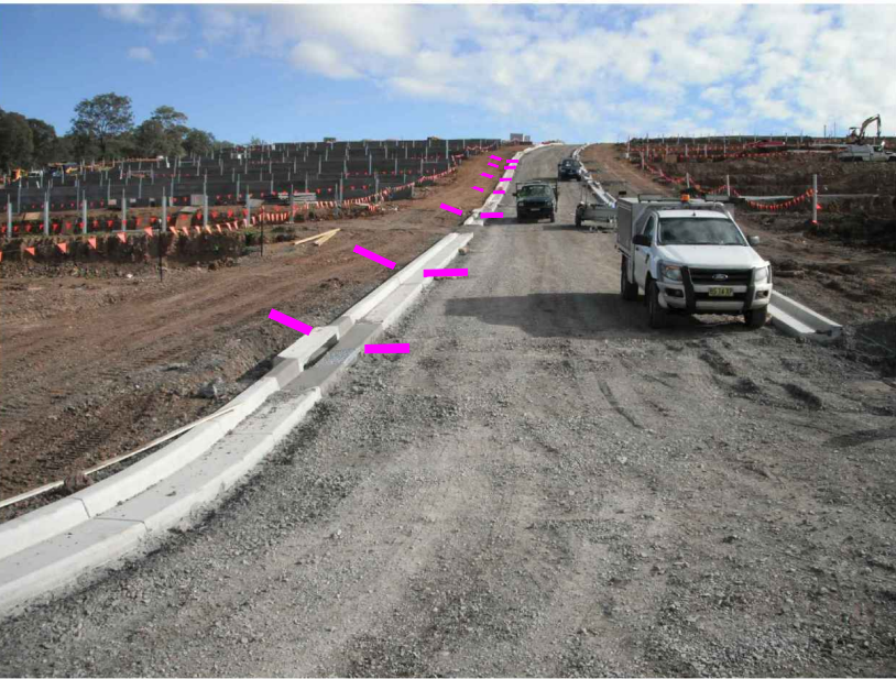
PHOTO 1: SANDBAGS INSTALLED ALONG NEW KERB AND GUTTER TO MINIMISE THE RISK OF SCOUR AND DIVERT FLOWS INTO KERBS.
