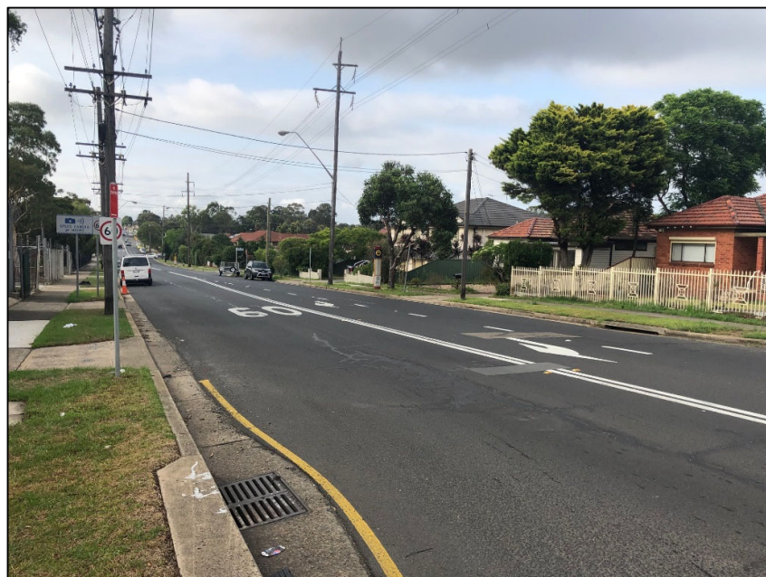
Figure 6: Gibson Avenue facing South
