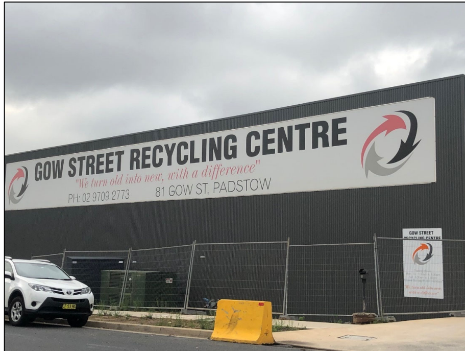
Figure 3: Development Site (81 Gow Street in Padstow)
