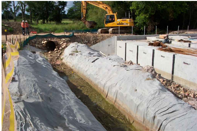
PHOTO 1 - EXAMPLE OF OFFSITE (CLEAN) WATER DIVERSION
