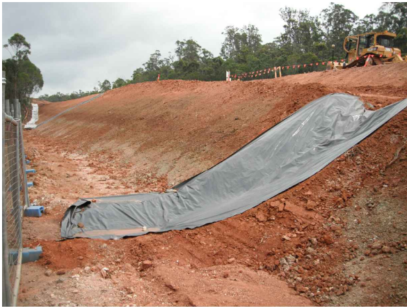
PHOTO 6 - EXAMPLE OF BATTER CHUTE
