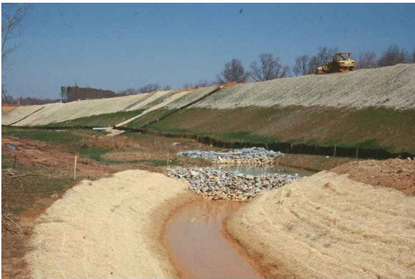
PHOTO 2 - PROGRESSIVE STABILISATION OF BATTERS AS WORKS PROGRESS
