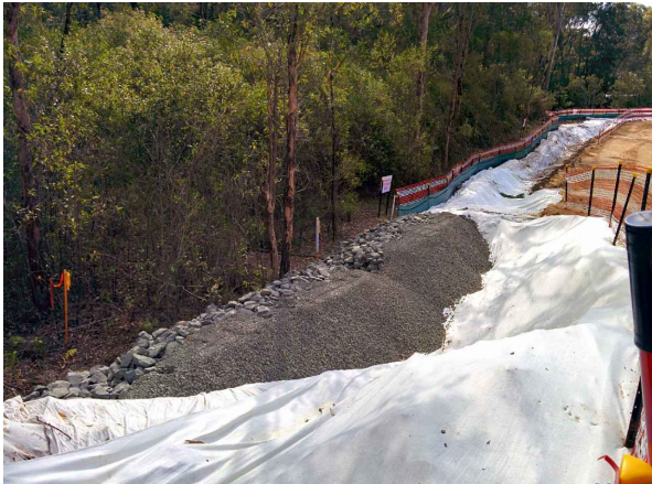
PHOTO 5 - EXAMPLE OF ROCK FILTER DAM AND SUMP
