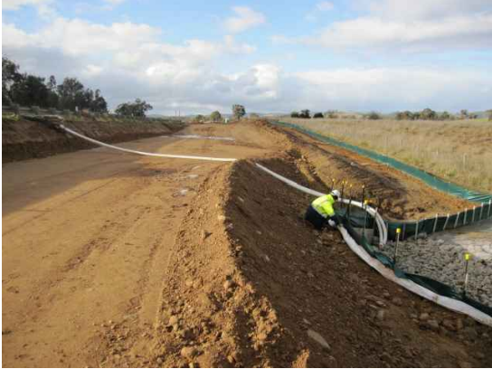
PHOTO 4 - EXAMPLE OF TEMPORARY PIPED (CLEAN) WATER DIVERSION INSTALLED PRIOR TO RAINFALL
