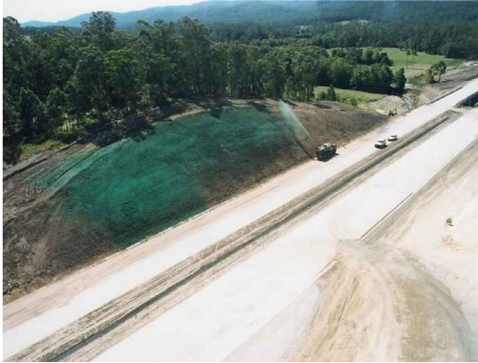
PHOTO 3 - TEMPORARY STABILISATION OF BATTERS WITH POLYMER
