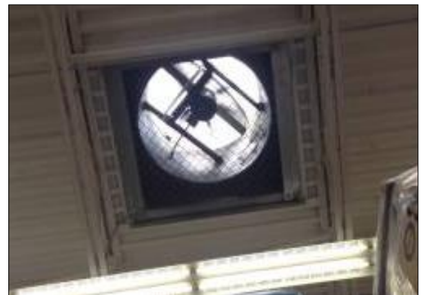
Figure 11 - Motorised smoke exhaust fans can enable hot air to escape through roof, facilitating air ventilation.
