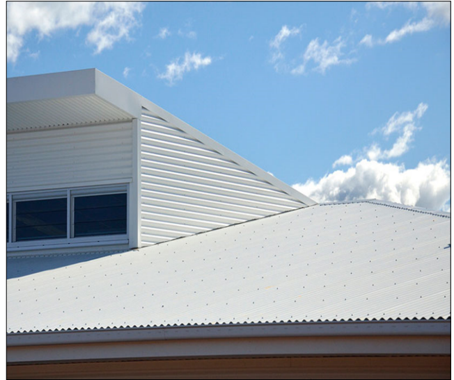
Figure 8 - Illustration of a light coloured (reflective) roof sheeting.
