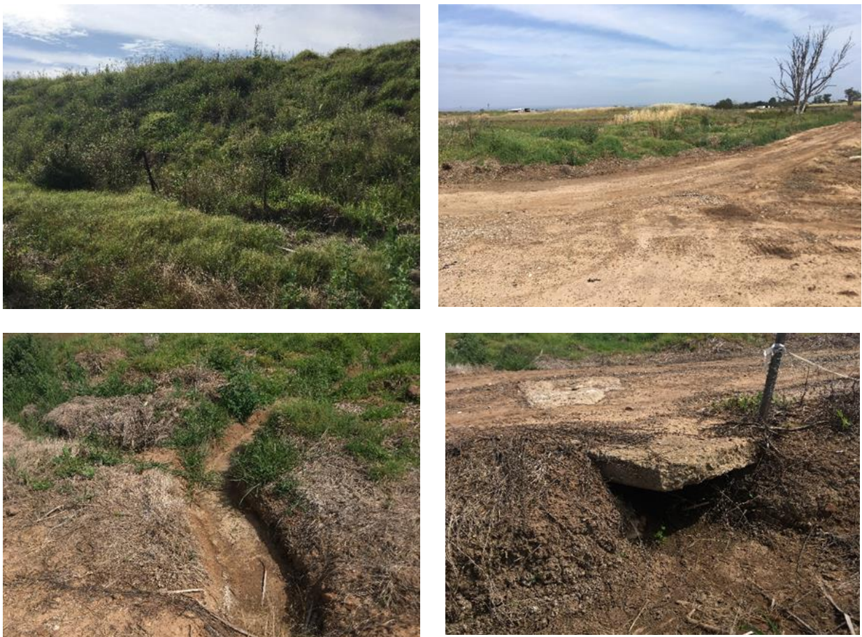
Figure 10: Photo point 2: Top left: looking upstream at downstream wall of the 2 nd dam; top right: looking downstream towards 3 rd dam in Lot 55, no defined channel; bottom left: dug out drainage channel to convey uphill runoff; bottom right: drainage culvert under unformed road.
