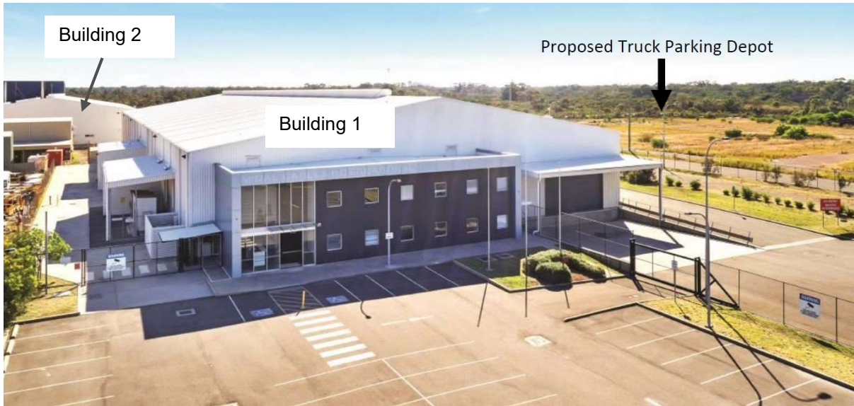
Figure 3 | Existing Buildings on the Site
