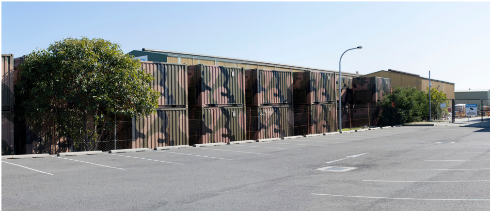
Photo 6. View north west along towards the boundary of Lot 21D. Containers in the fore-ground and large warehouse in the background part of the neighbouring business operations. Source: Moir LA 2020
