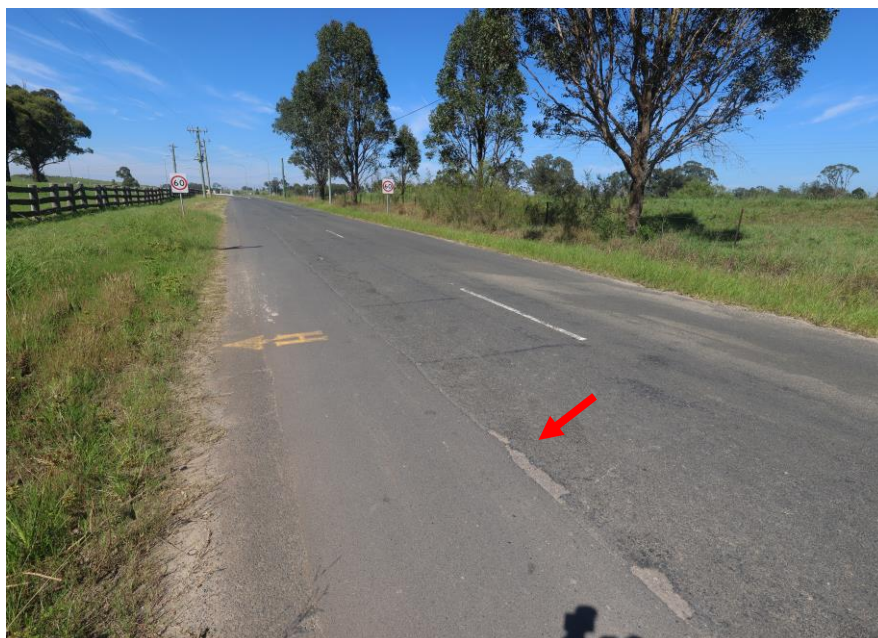
General view of the roadway on Adams Road. Showing chipping.
