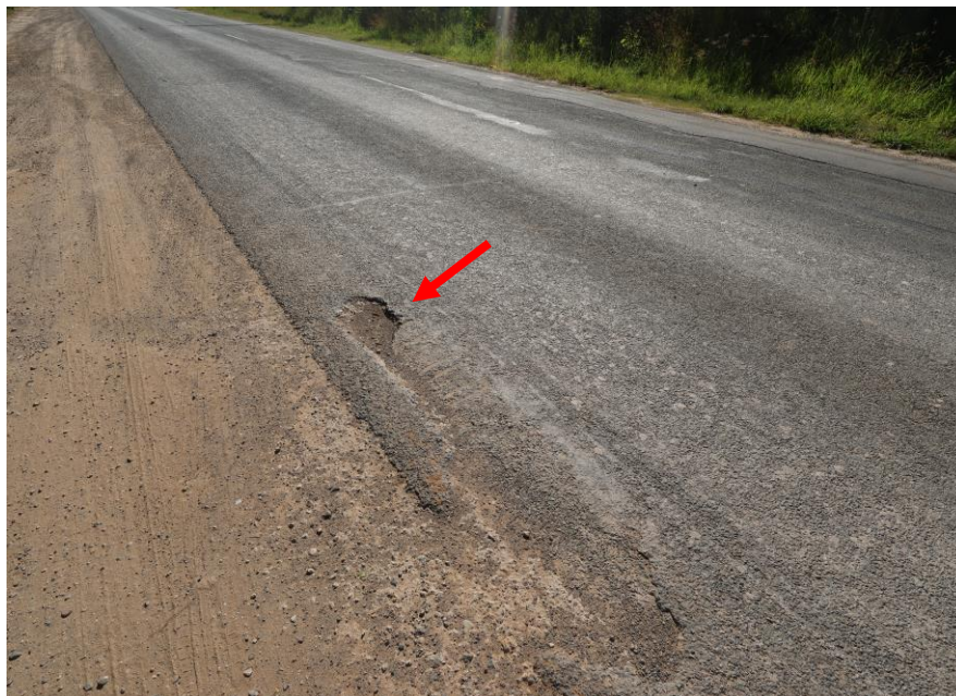
Pothole in the roadway on Adams Road.
