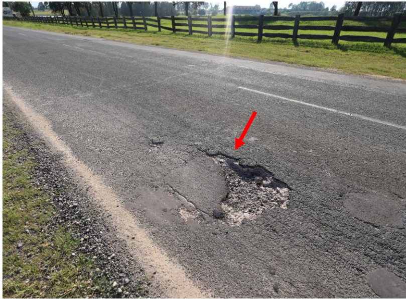
Pothole in the roadway on Adams Road.
