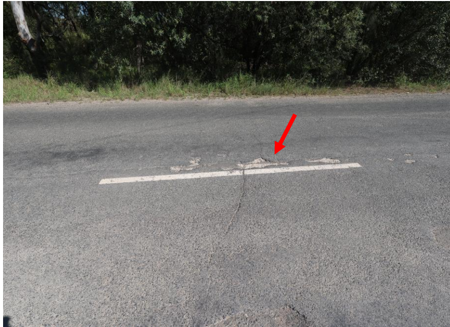
Spalling in the roadway on Adams Road.
