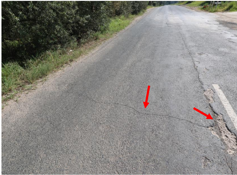
Fine cracking and damage in the roadway on Adams Road.
