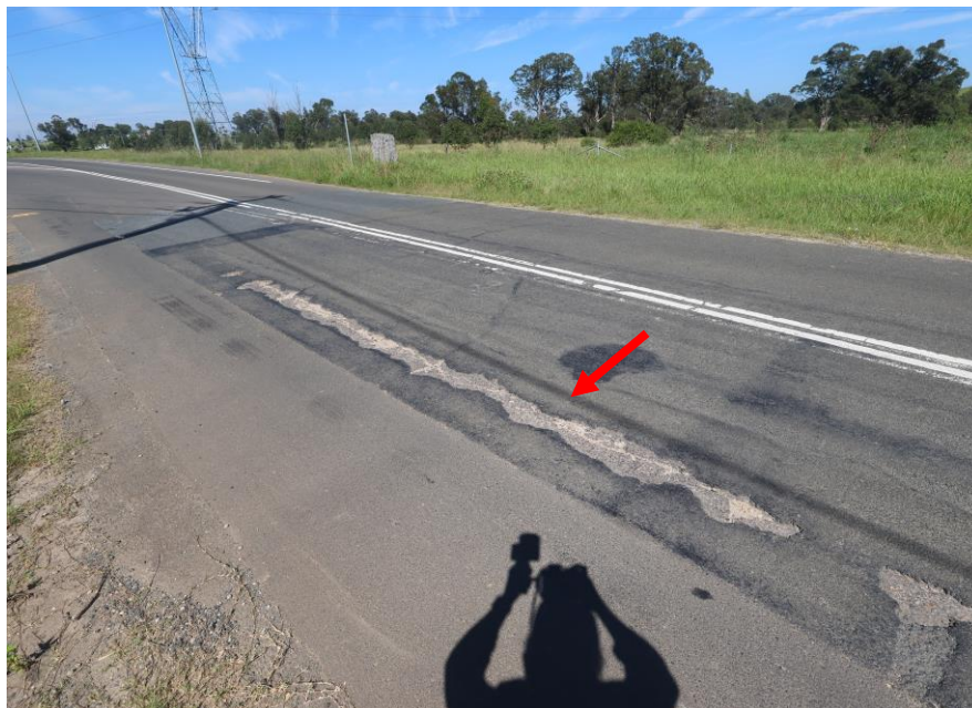
Spalling in the roadway on Adams Road.
