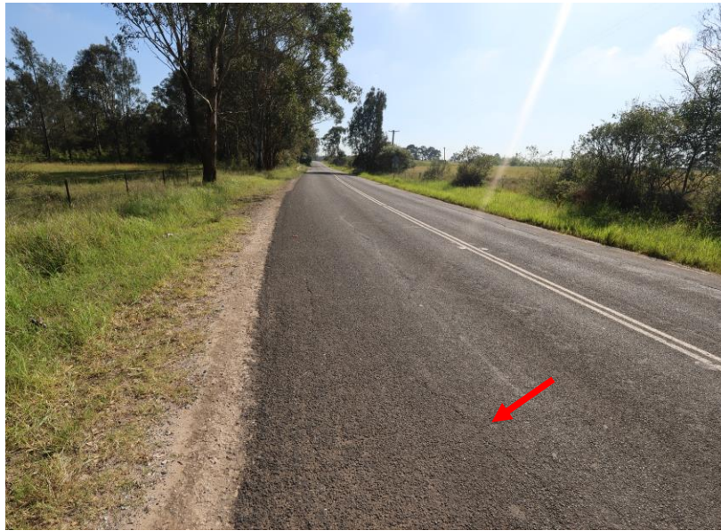
General view of the roadway showing fine cracking.
