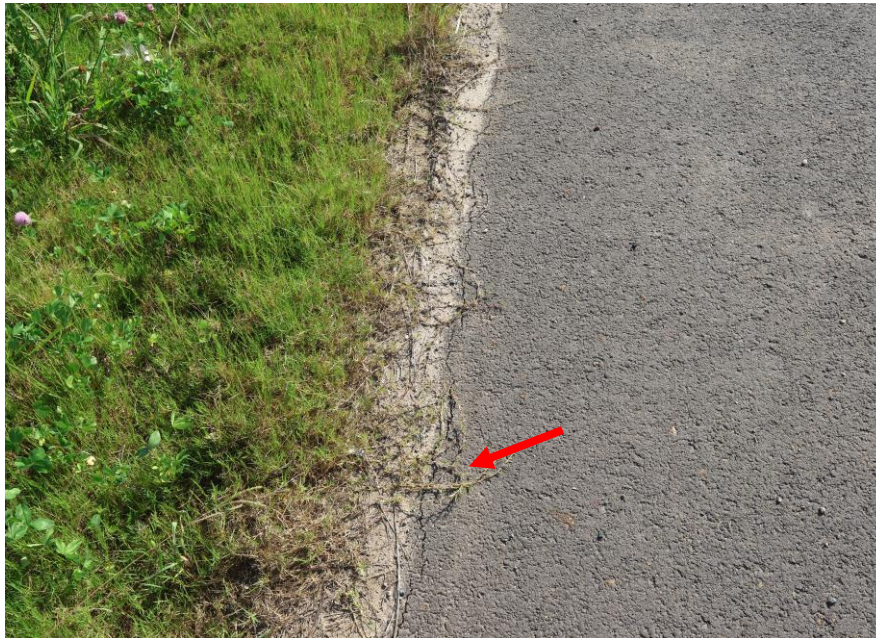
Fine cracking in the roadway on Adams Road.
