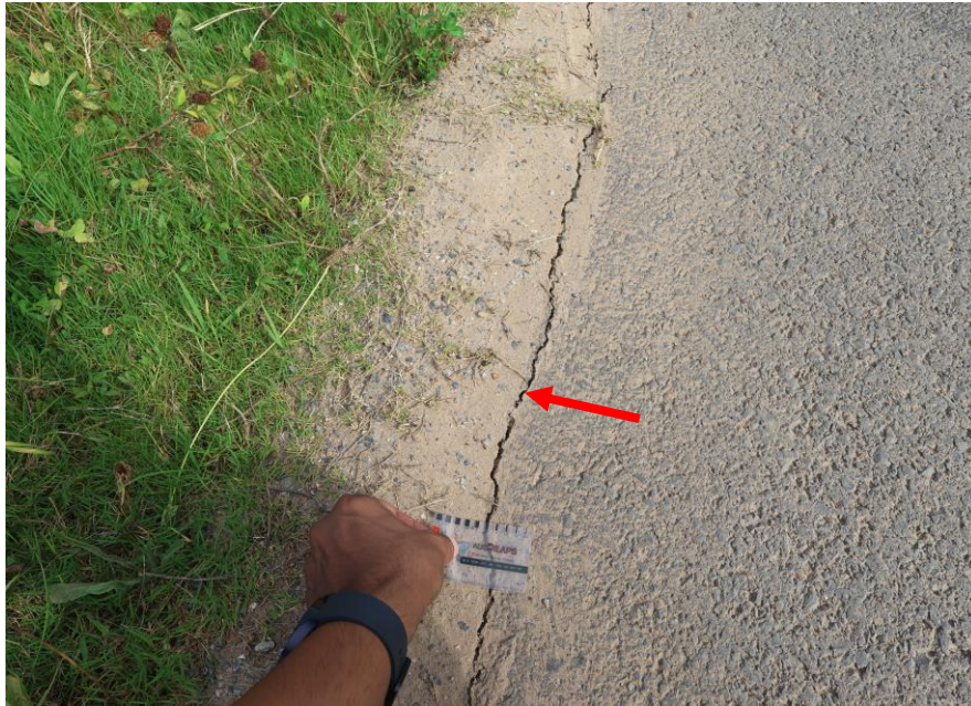
Slight cracking in the roadway on Anton Road.
