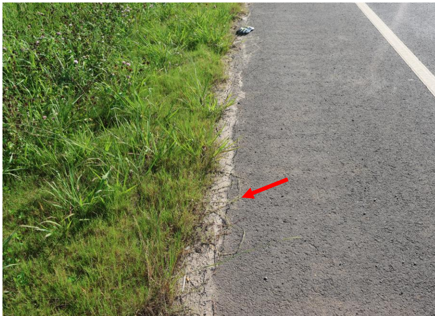
Fine cracking in the roadway on Adams Road.
