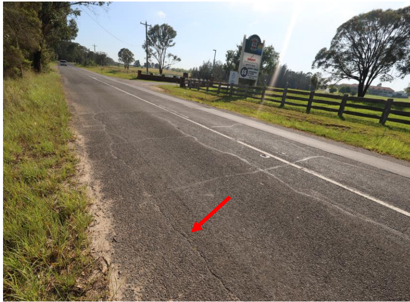
General view of the roadway on Adams Road. Showing fine cracking.
