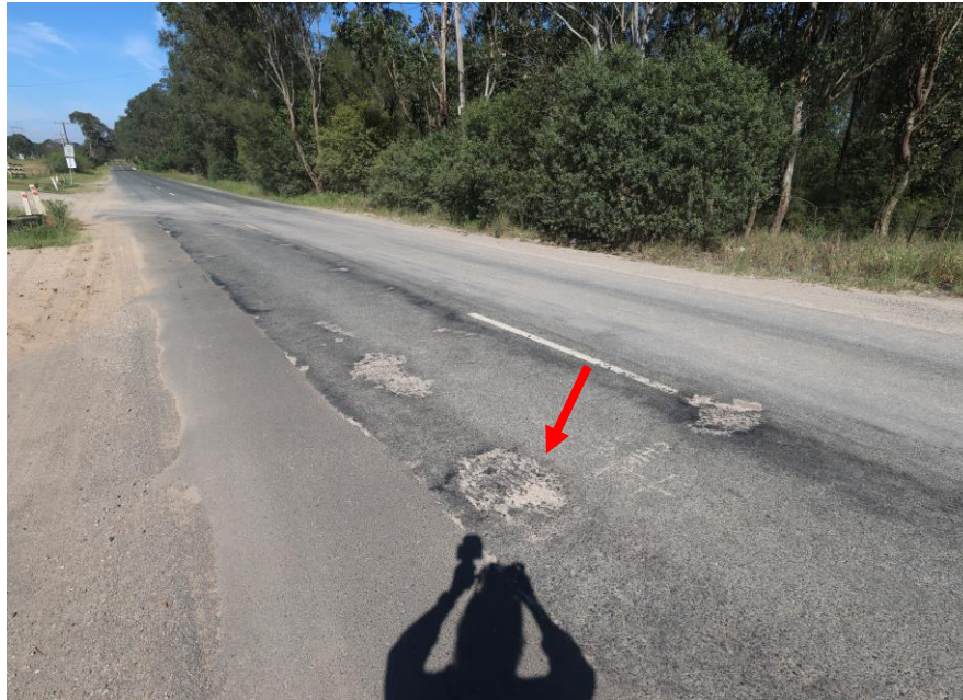
Spalling in the roadway on Adams Road.
