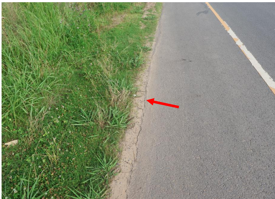
Slight cracking in the roadway on Anton Road.
