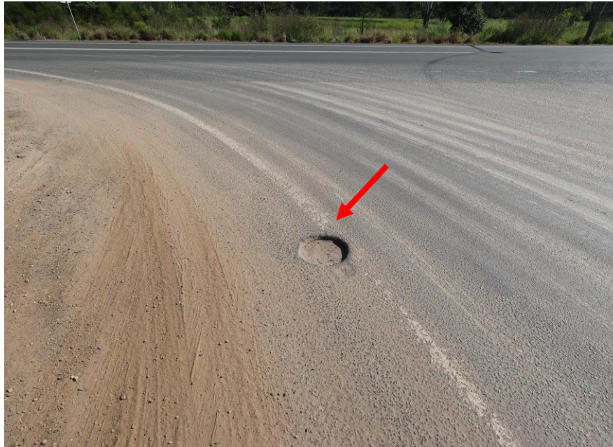
Pothole in the roadway on Adams Road.
