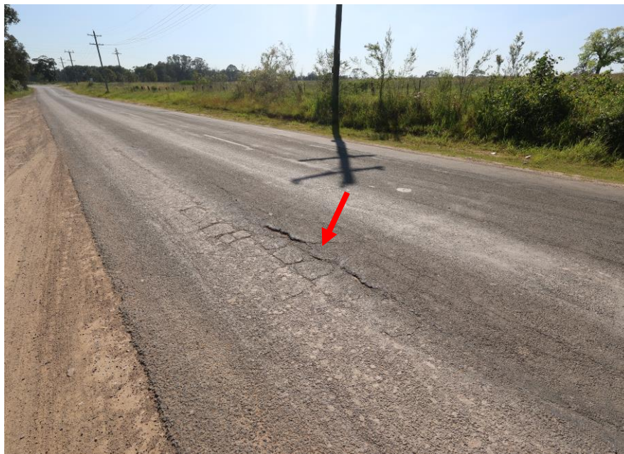
General view of the roadway on Adams Road. Showing alligator cracking.
