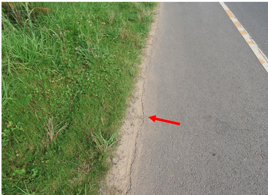
Slight cracking in the roadway on Anton Road.
