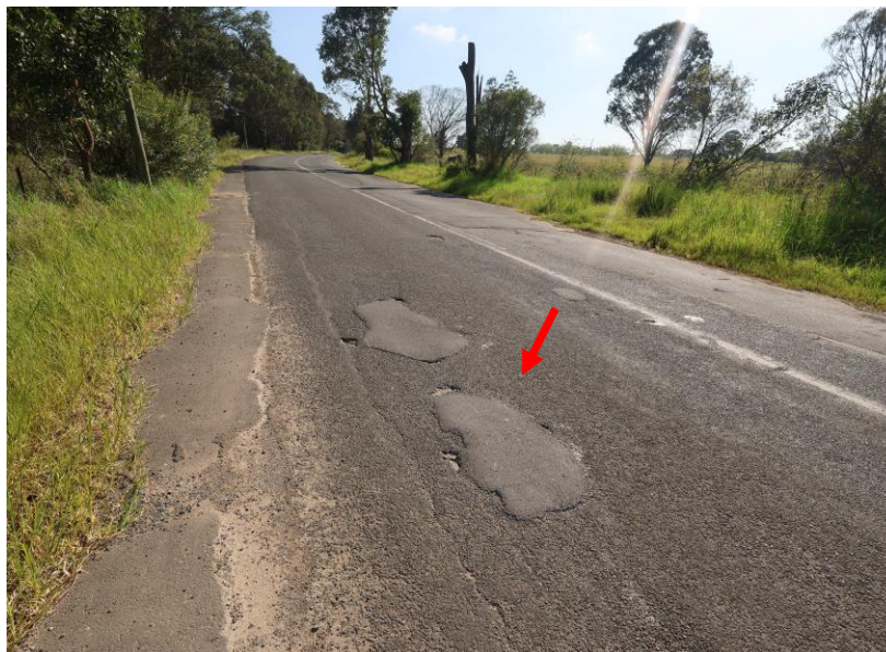
General view of the roadway on Adams Road. Showing patching.
