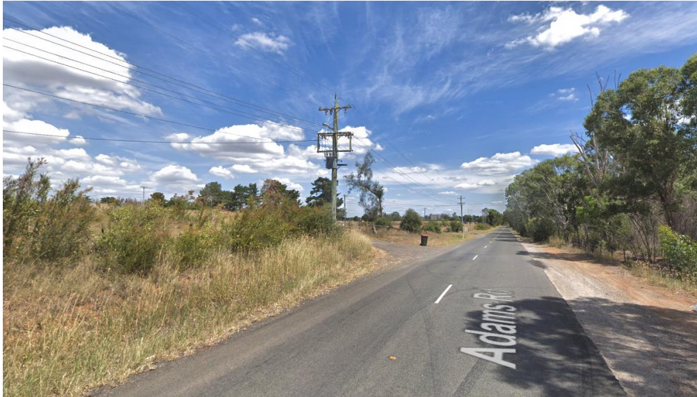
Figure 5 An image showing the Aerial low Voltage Network and Pole Mounted Transformer on Adams Rd
