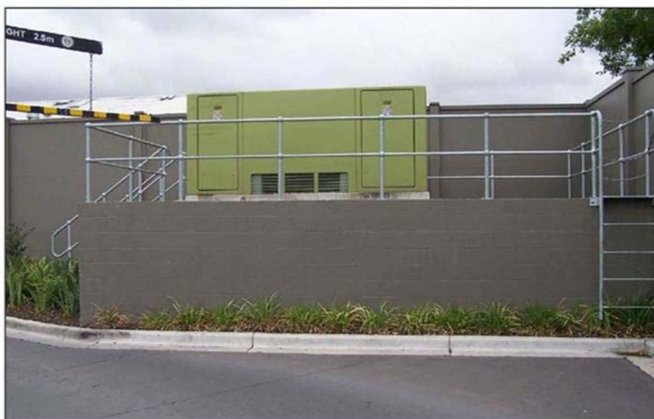
Figure 51 - Example substation raised above 1:100 flood level
