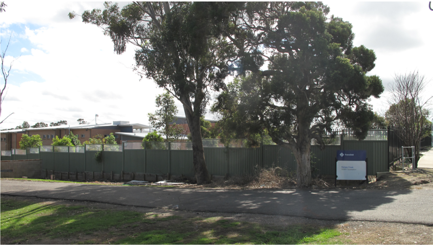
BEFORE: Street view from the intersection of Fourth and Gurner Avenue
