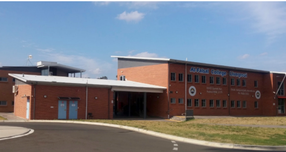
Existing Primary structures
