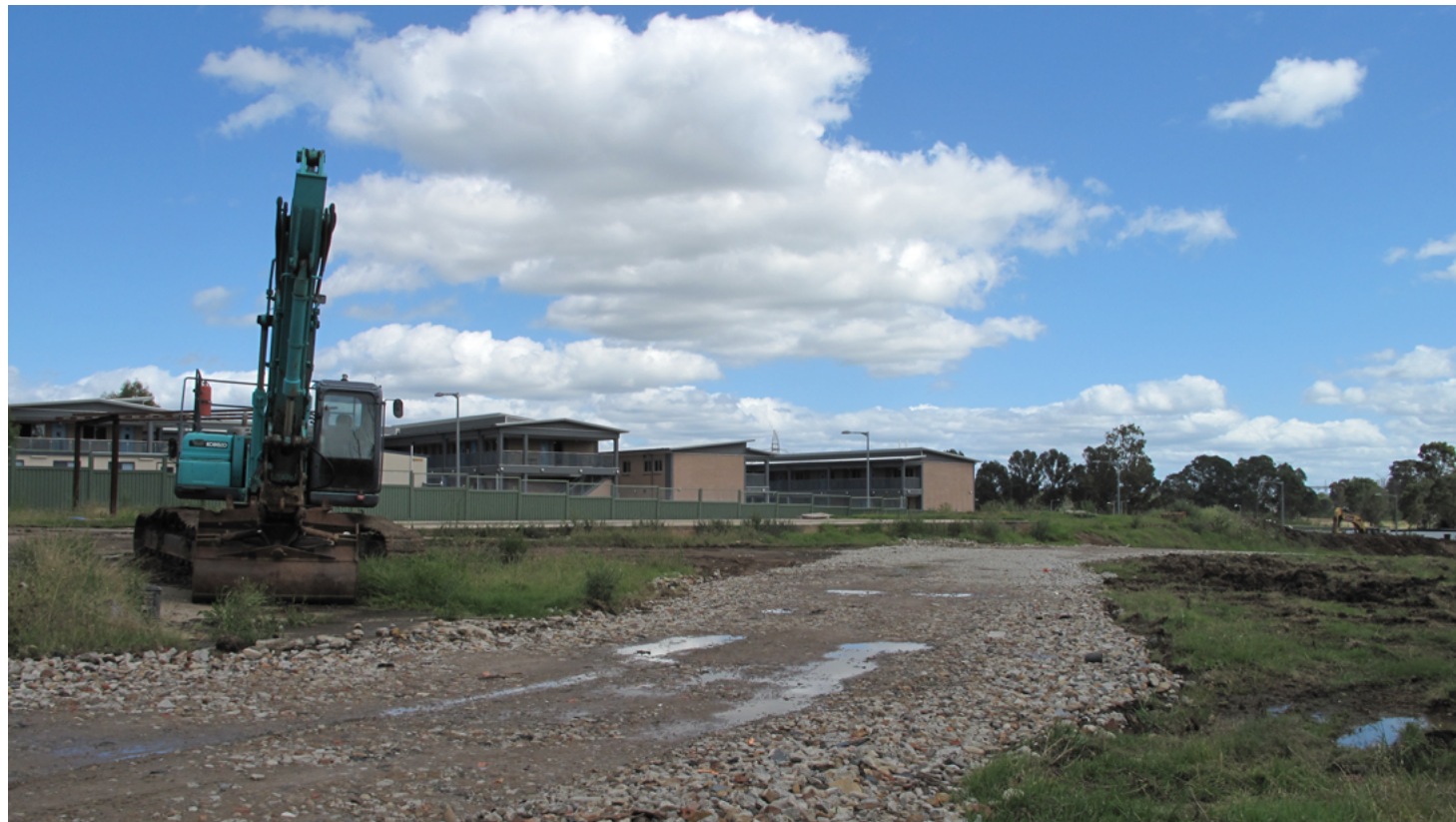
BEFORE: Street view from the green area
