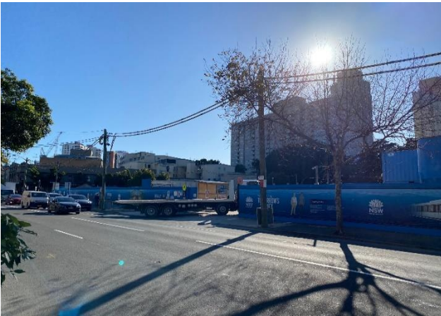
Picture 3 North western corner of site, looking north east illustrating station construction vehicular entrance
