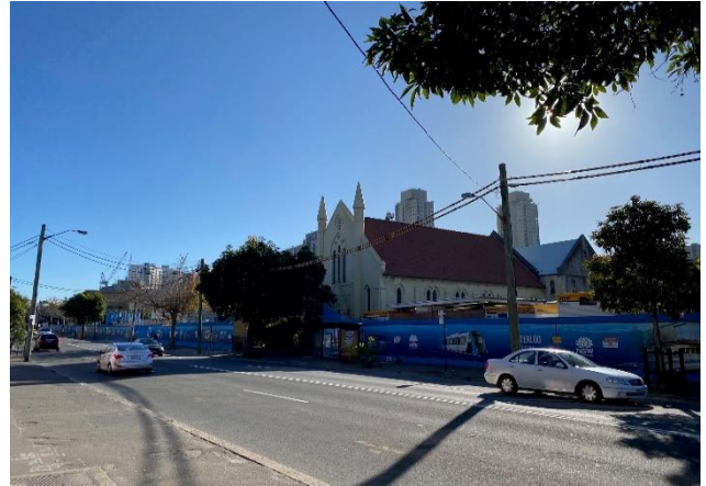
Picture 2 Botany Road street frontage, looking north east
