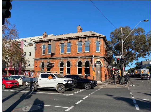
Picture 12 Locally heritage listed Former CBC Bank, including Interior located at 60 Botany Road
