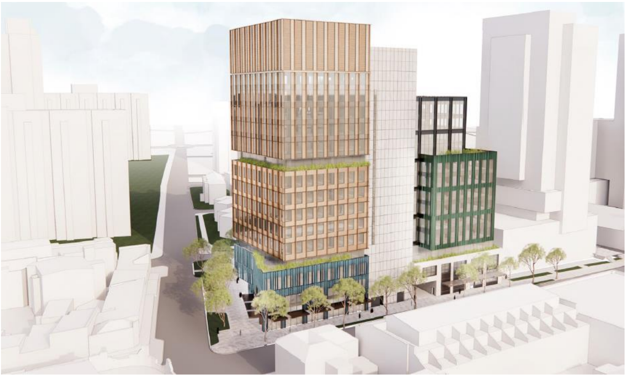
Picture 21 View of building 1 from the north-west
