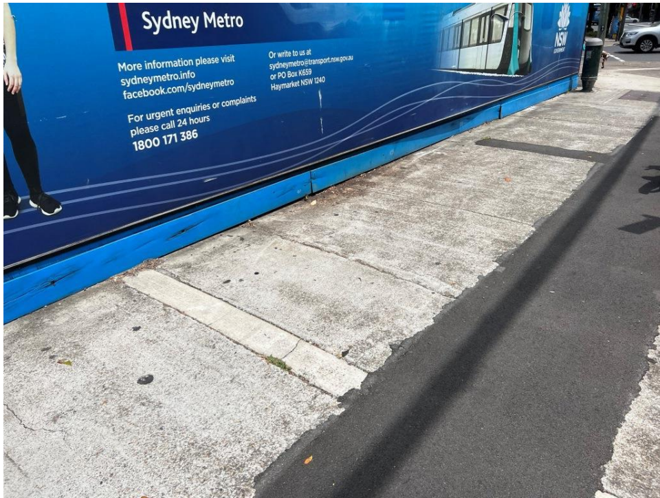
PHOTO 115 (Overview of footpath – Raglan Street)
