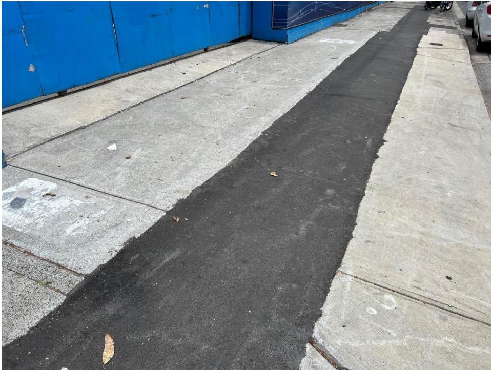
PHOTO 79 (Overview of truck driveway – Raglan Street)
