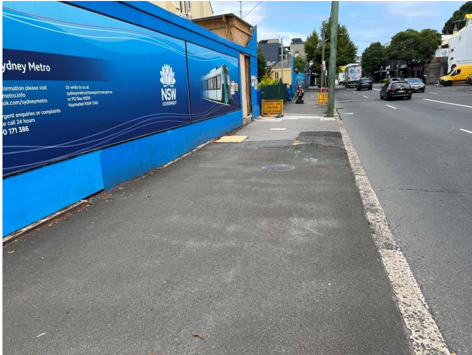
PHOTO 329 (Overview of footpath – Botany Road)
