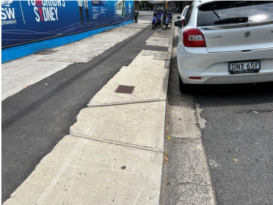
PHOTO 93 (Overview of footpath – Raglan Street)
