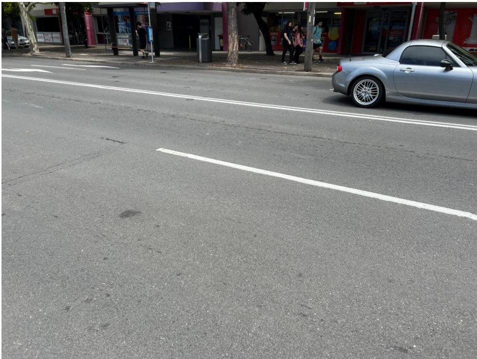
PHOTO 188 (Overview of roadway – Botany Road)
