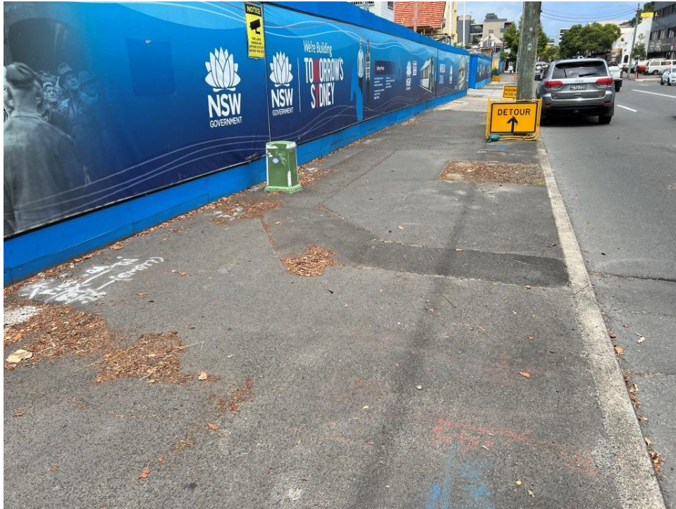
PHOTO 281 (Overview of footpath – Botany Road)
