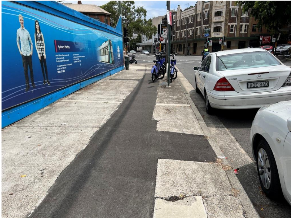
PHOTO 99 (Overview of footpath – Raglan Street)
