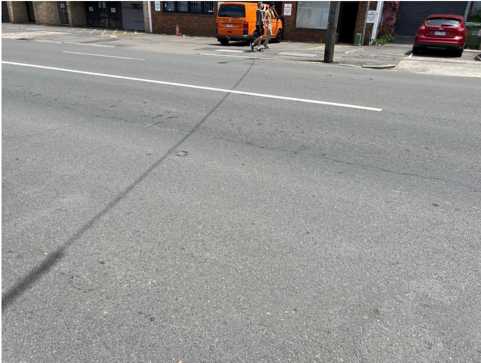
PHOTO 295 (Overview of roadway – Botany Road)
