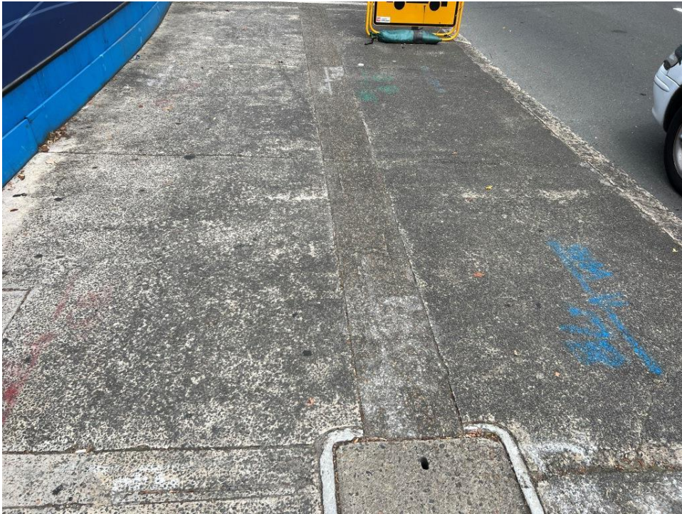
PHOTO 183 (Overview of footpath – Botany Road)
