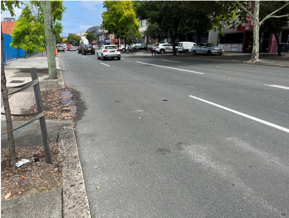
PHOTO 205 (Overview of roadway – Botany Road)
