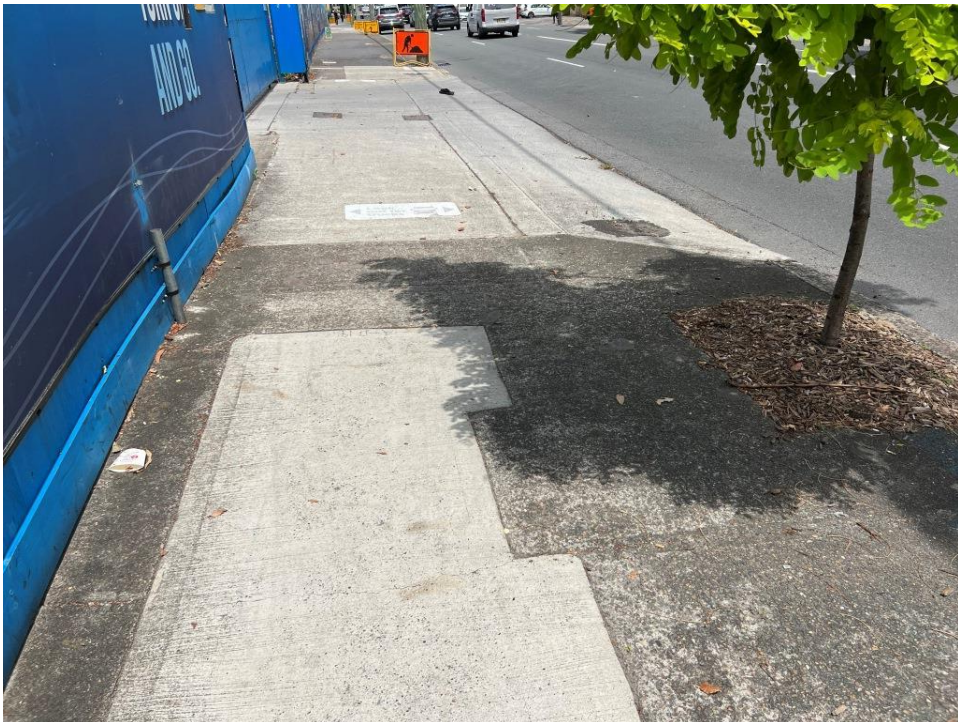
PHOTO 222 (Overview of footpath and tree – Botany Road)
