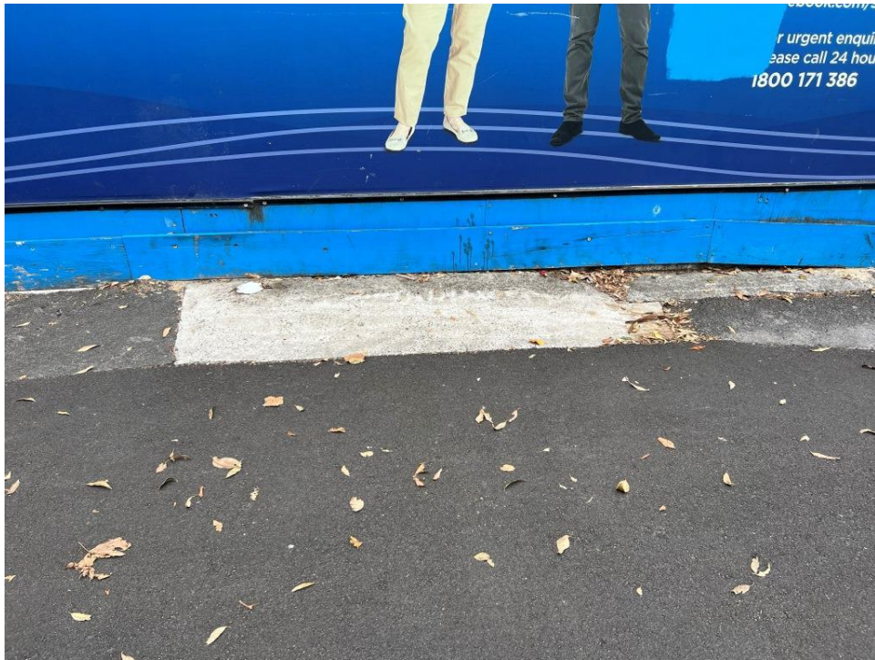
PHOTO 27 (Overview of footpath – Raglan Street)
