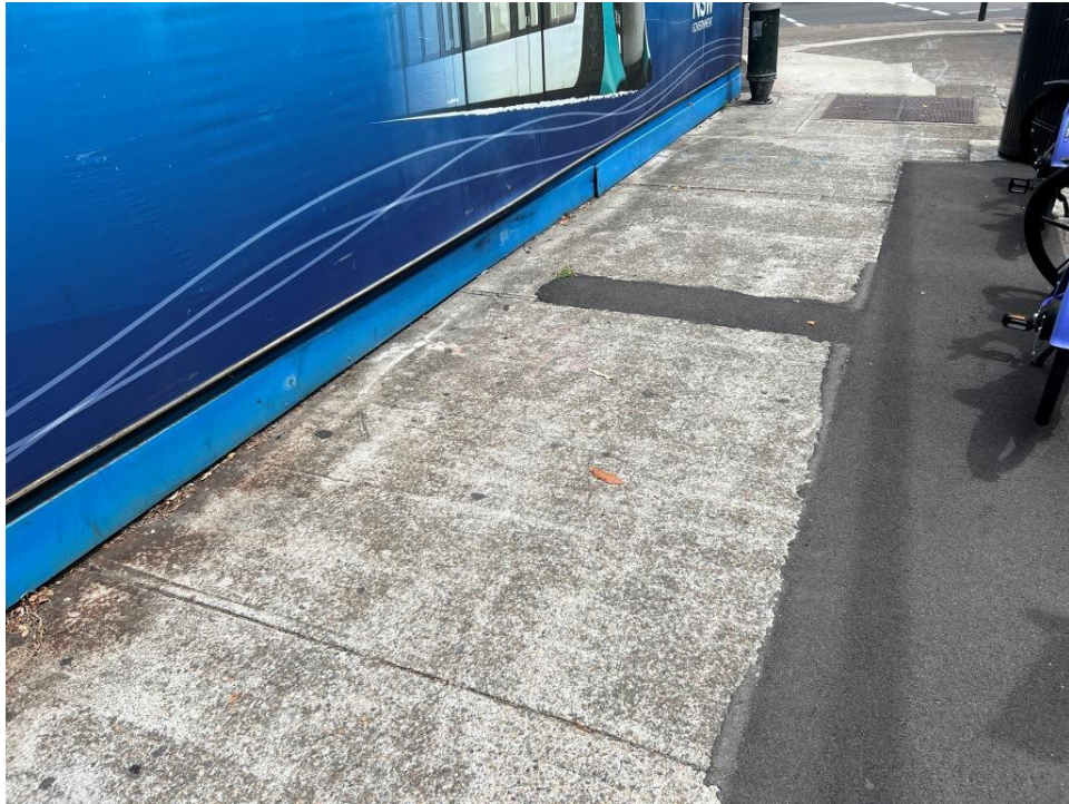
PHOTO 123 (Overview of footpath – Raglan Street)
