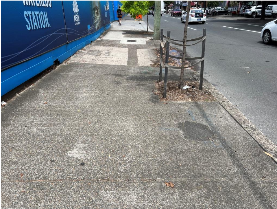
PHOTO 203 (Overview of footpath – Botany Road)
