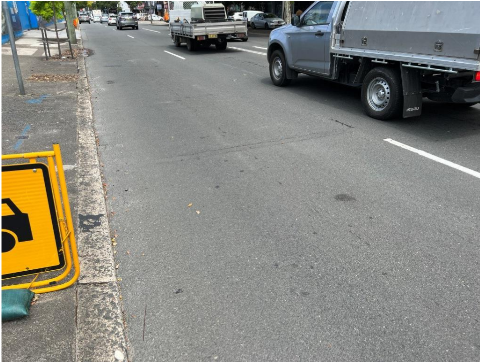
PHOTO 187 (Overview of roadway – Botany Road)
