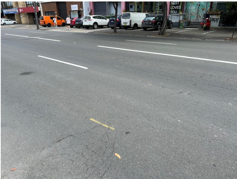
PHOTO 270 (Overview of roadway – Botany Road)
