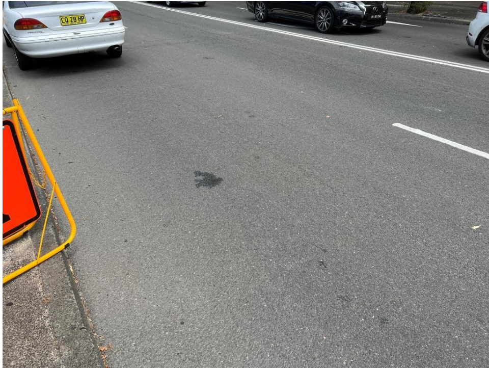
PHOTO 169 (Overview of roadway – Botany Road)
