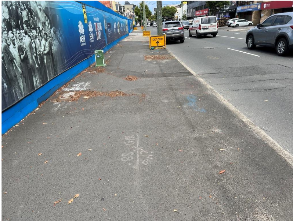
PHOTO 279 (Overview of footpath – Botany Road)
