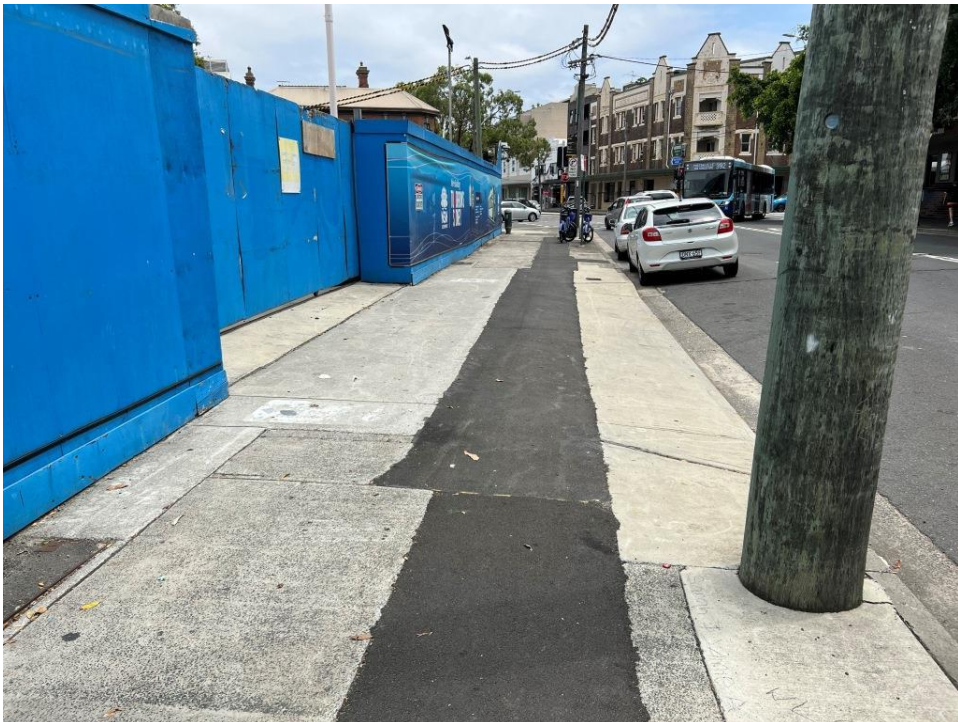
PHOTO 72 (Overview of footpath – Raglan Street)
