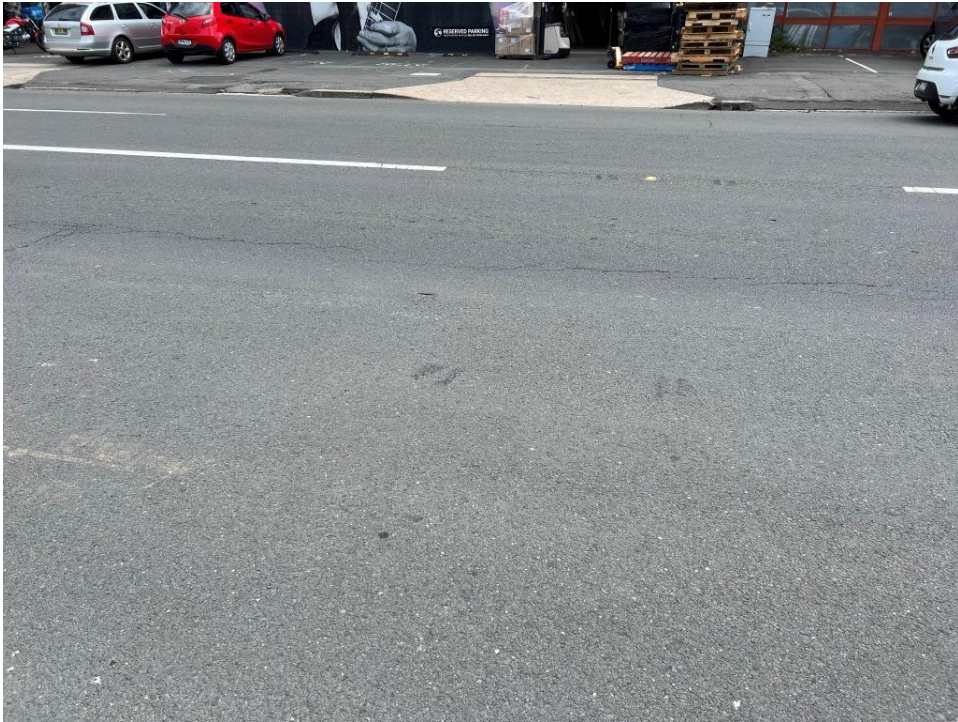
PHOTO 331 (Overview of roadway – Botany Road)
