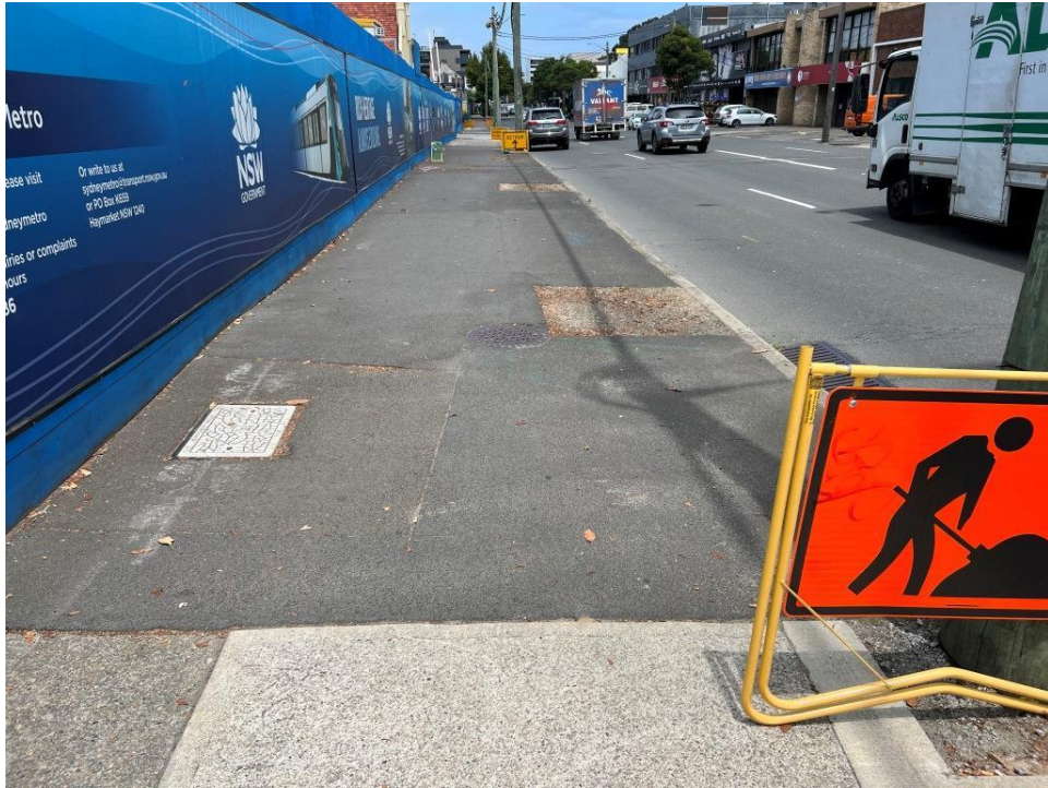
PHOTO 251 (Overview of footpath – Botany Road)
