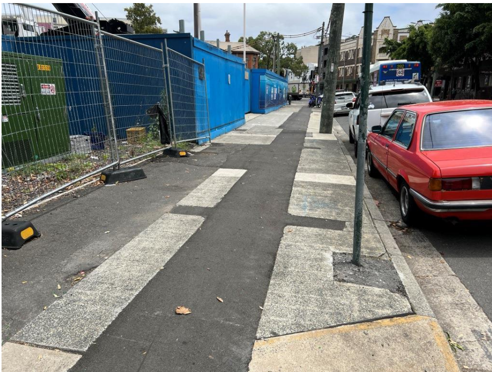
PHOTO 42 (Overview of footpath – Raglan Street)
