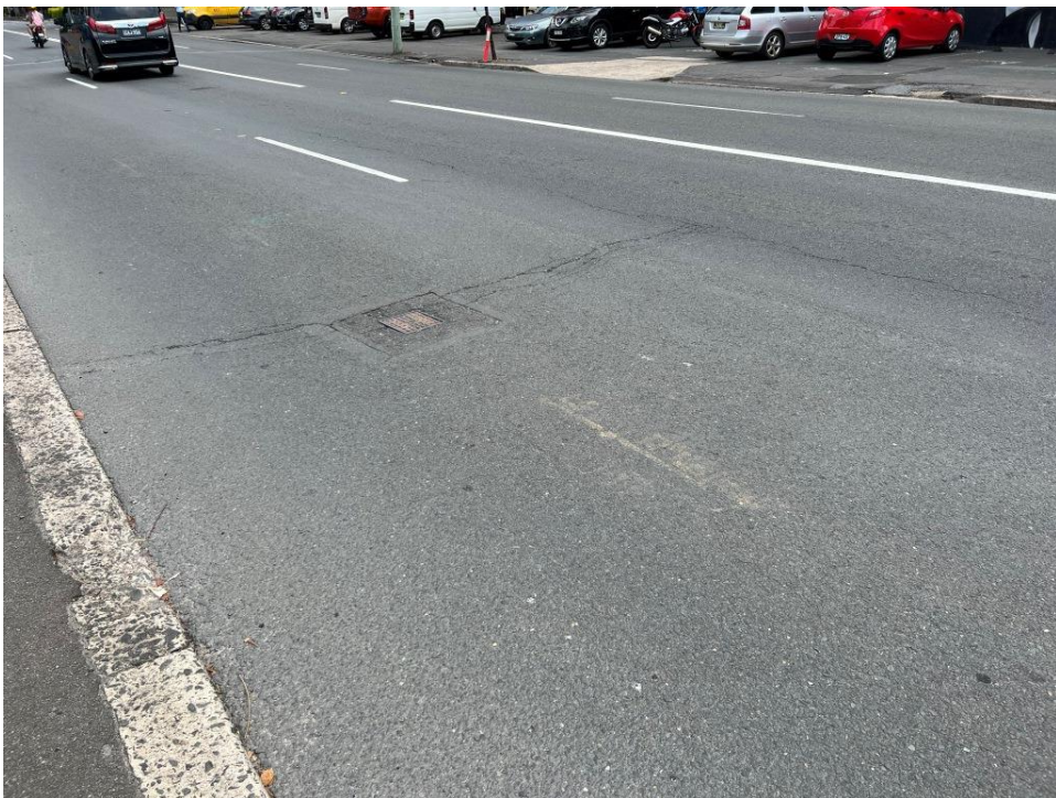
PHOTO 332 (Overview of roadway – Botany Road)
