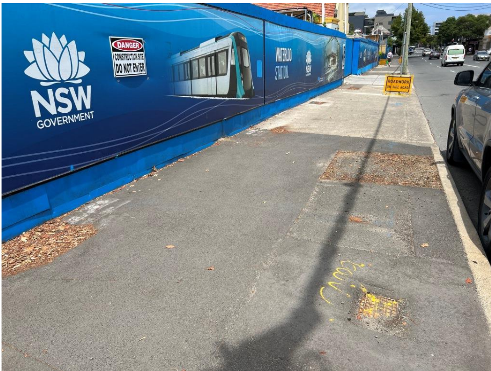
PHOTO 296 (Overview of footpath – Botany Road)
