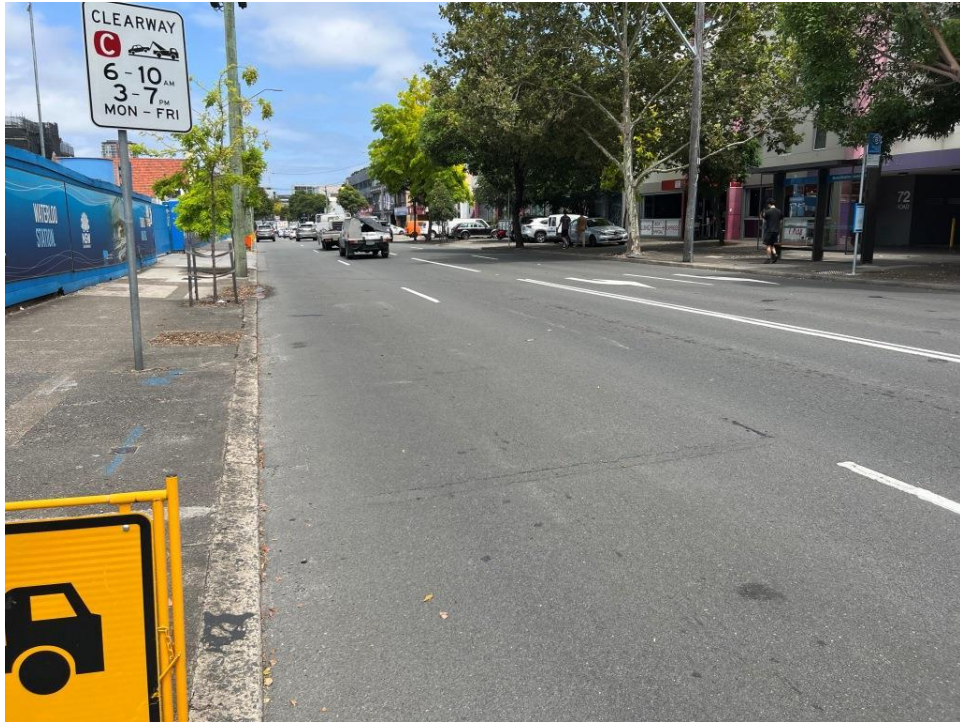
PHOTO 189 (Overview of roadway – Botany Road)
