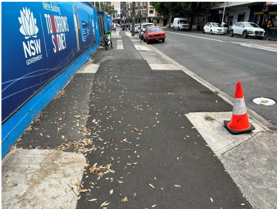
PHOTO 14 (Overview of footpath – Raglan Street)
