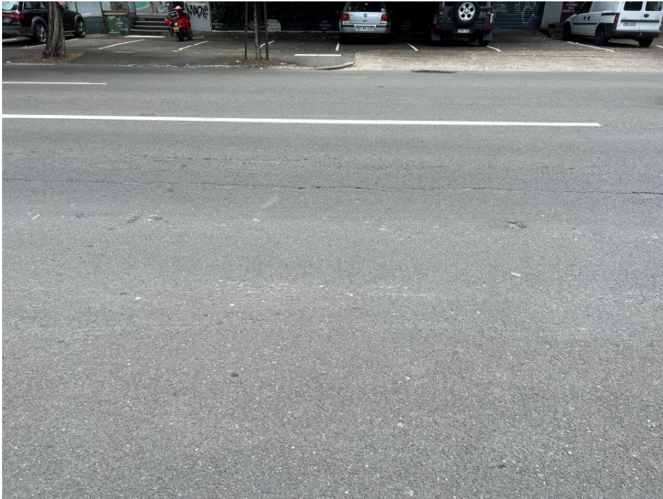
PHOTO 269 (Overview of roadway – Botany Road)
