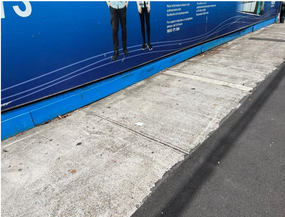
PHOTO 107 (Overview of footpath – Raglan Street)
