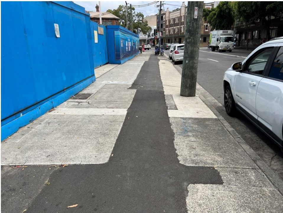
PHOTO 66 (Overview of footpath – Raglan Street)
