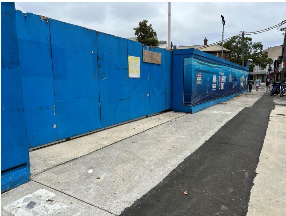
PHOTO 80 (Overview of truck driveway – Raglan Street)
