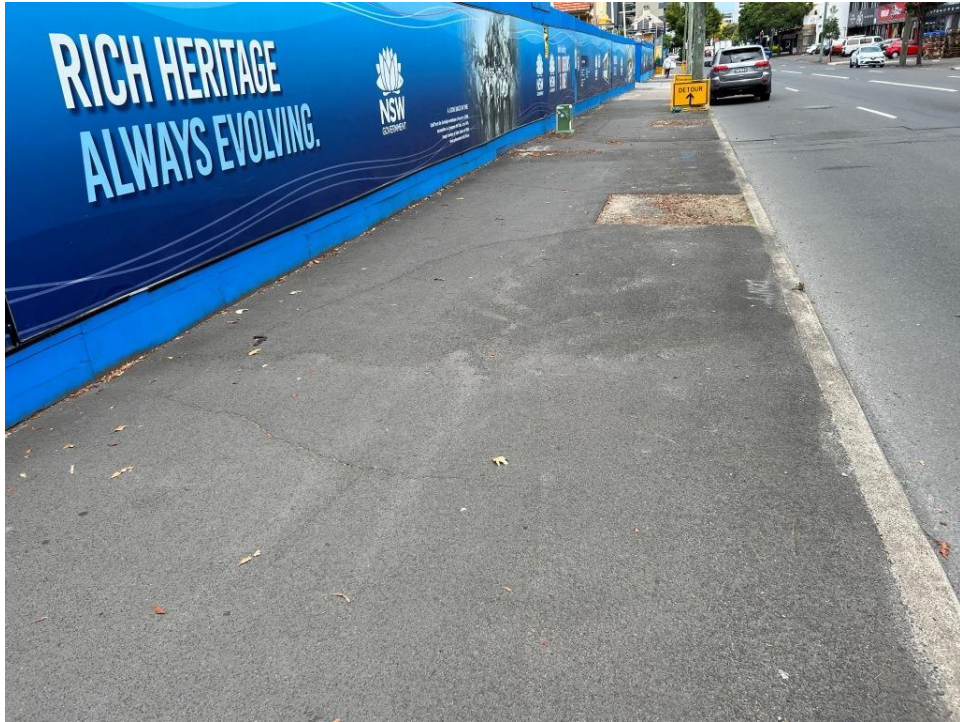
PHOTO 273 (Overview of footpath – Botany Road)
