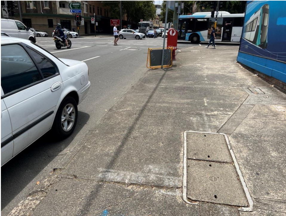
PHOTO 191 (Overview of footpath – Botany Road)
