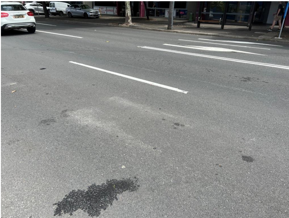
PHOTO 204 (Overview of roadway – Botany Road)
