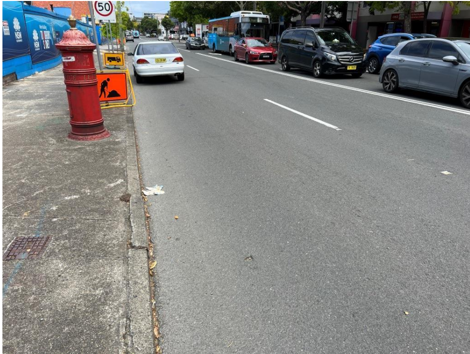
PHOTO 157 (Overview of roadway – Botany Road)
