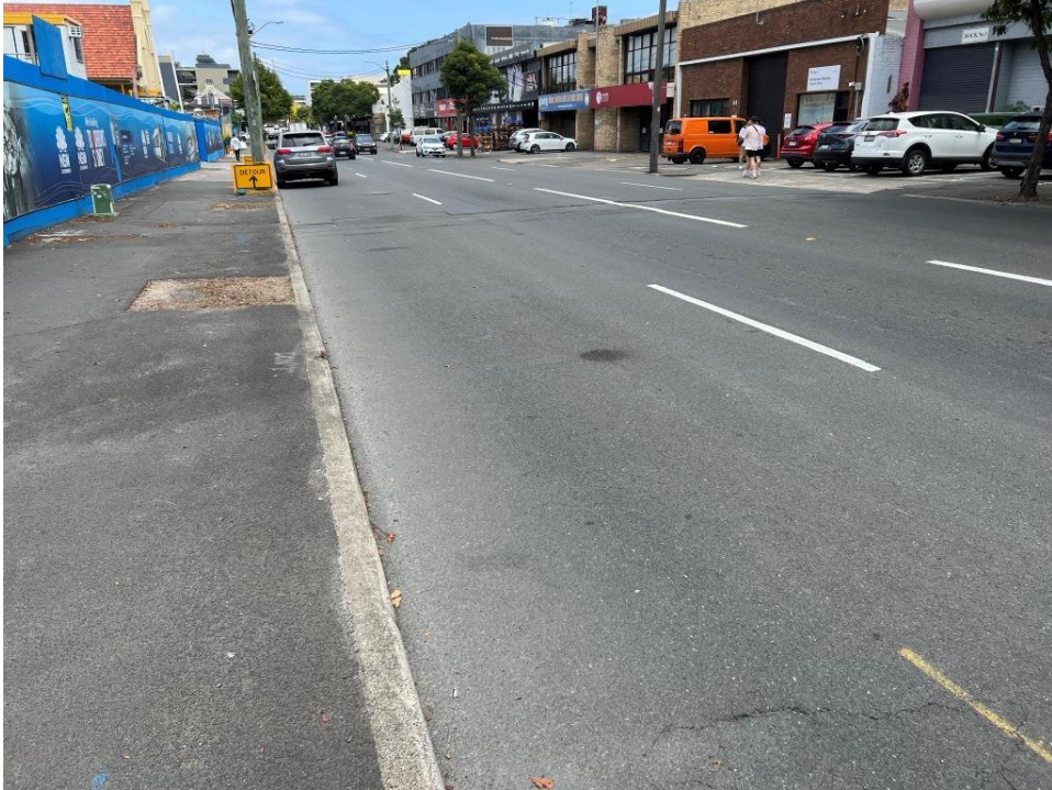
PHOTO 271 (Overview of roadway – Botany Road)
