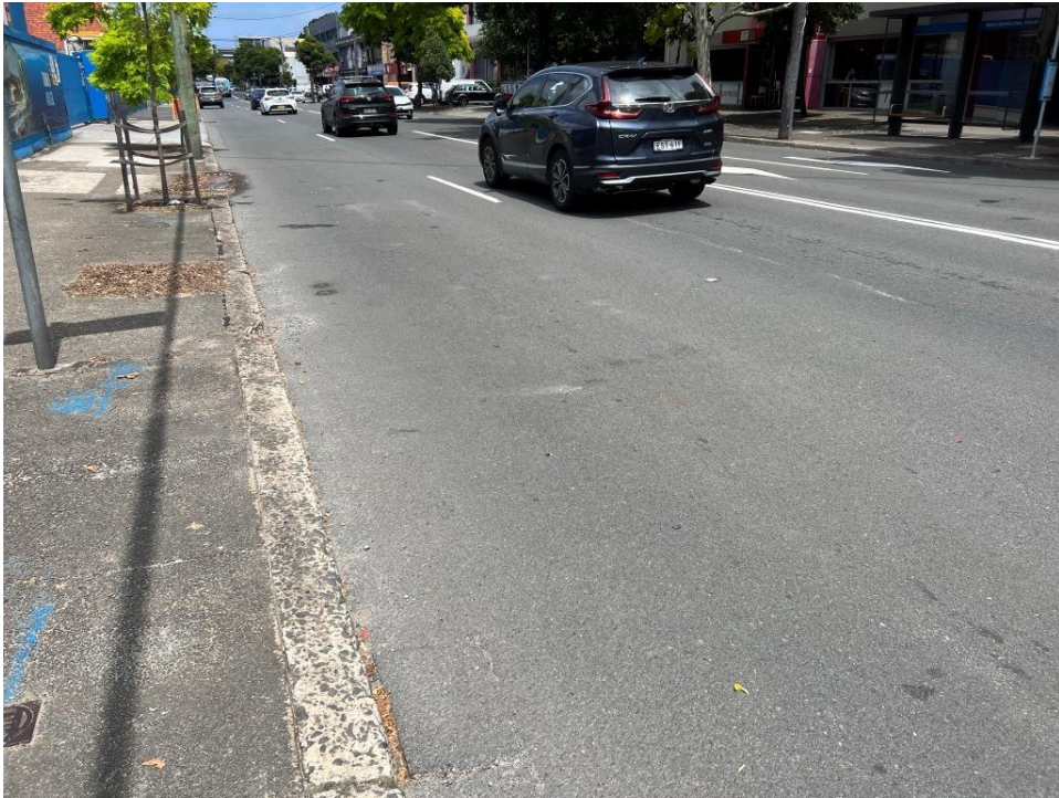
PHOTO 195 (Overview of roadway – Botany Road)
