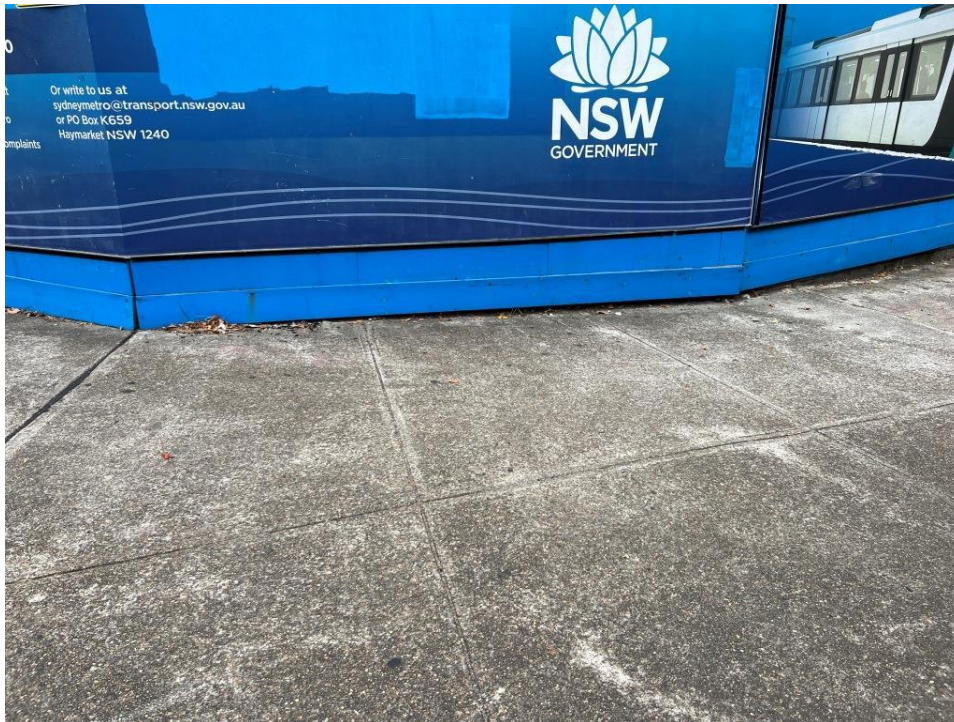
PHOTO 165 (Overview of footpath – Botany Road)
