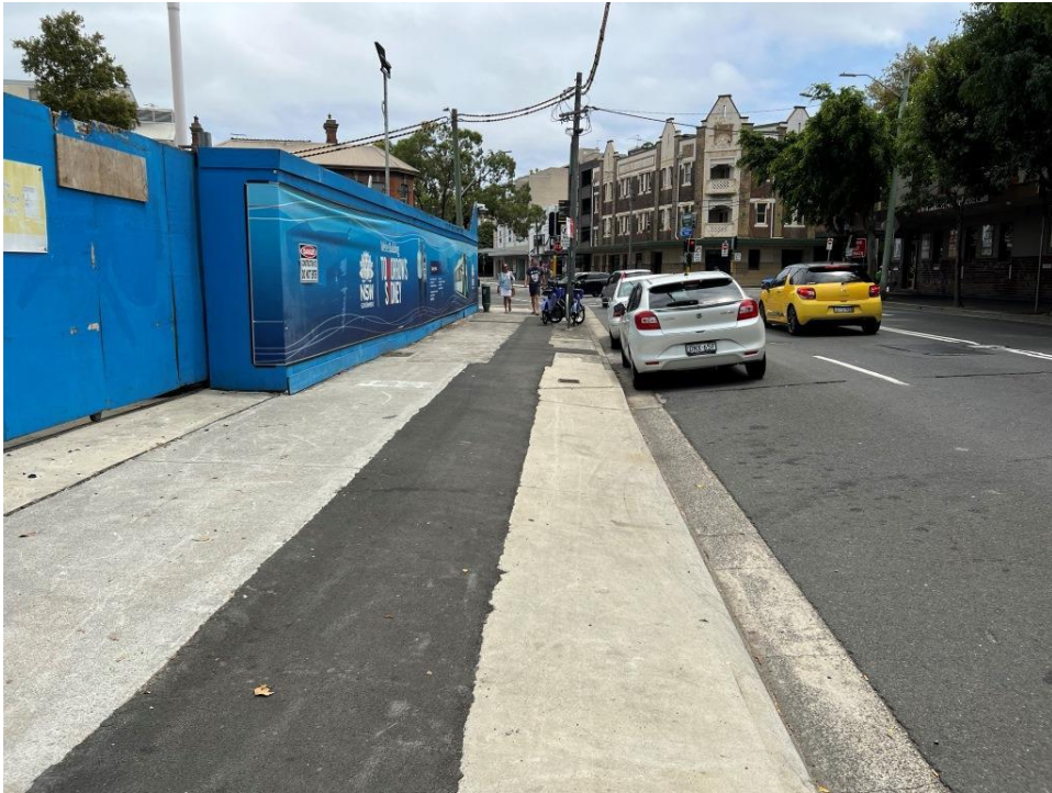
PHOTO 81 (Overview of truck driveway – Raglan Street)
