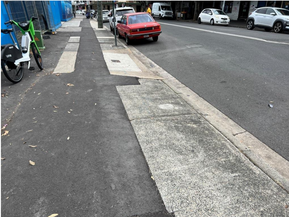
PHOTO 29 (Overview of footpath – Raglan Street)
