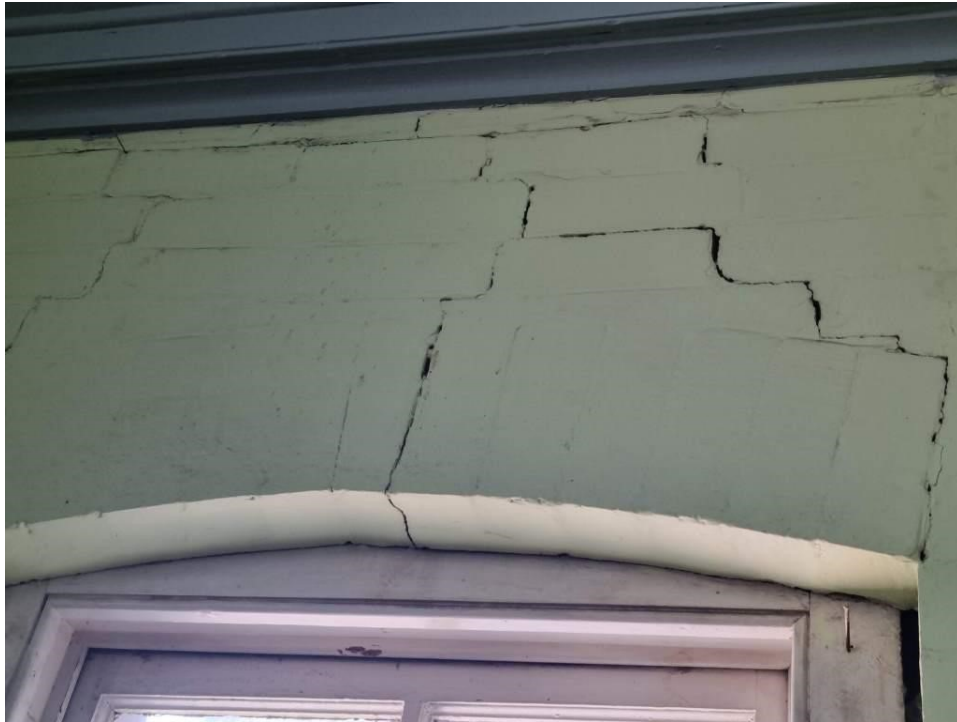
PHOTO 69 (Close up of brickwork crack above window)
