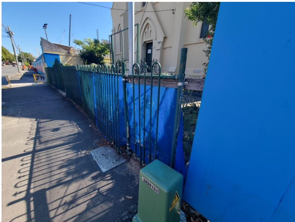
PHOTO 4 (Photo showing leaning fence with break of the fence railing creating a gap)
