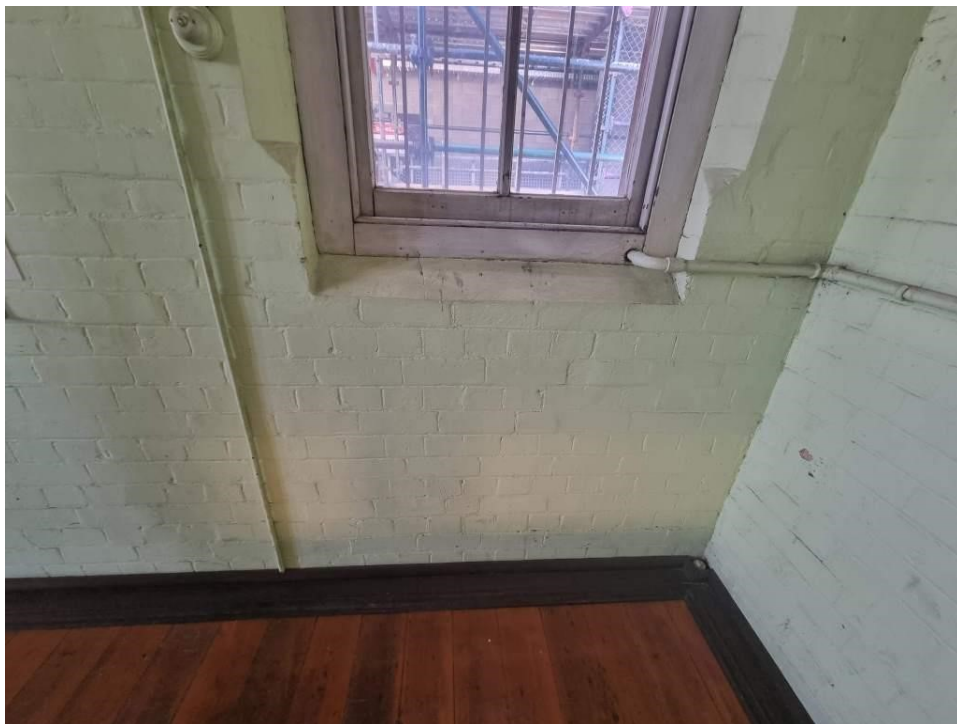
PHOTO 60 (Photo showing cracking below the window adjacent to the stairs on level 2)
