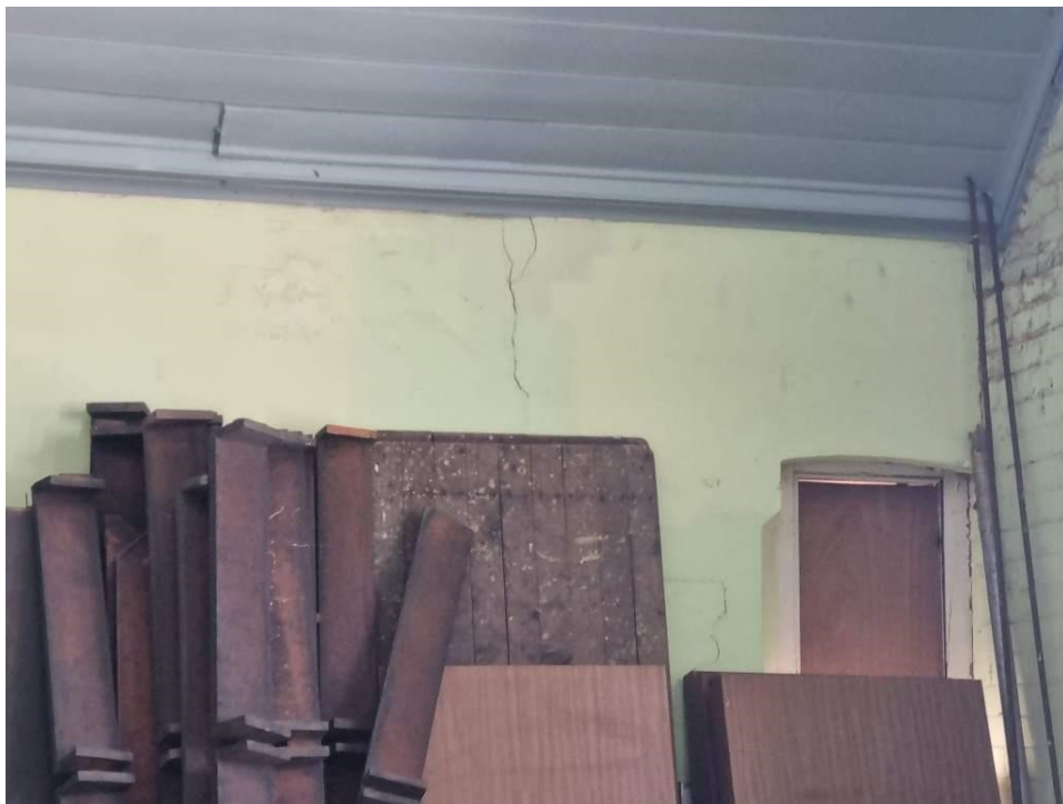
PHOTO 70 (Photo showing brickwork crack to top of wall on Level 2. Unable to reach and measure with of cracks)
