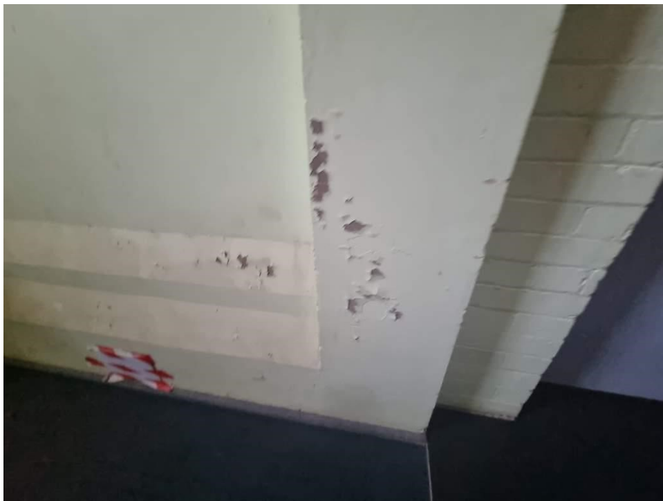
PHOTO 54 (Photo showing paint peeling on wall on level 1)
