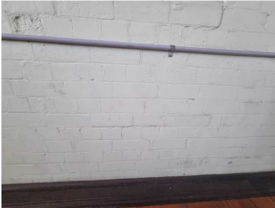
PHOTO 71 (Cracking to brick wall below the windows on level 2)
