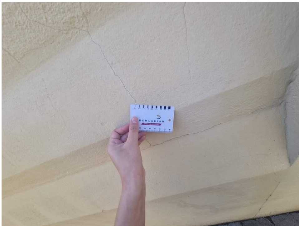
PHOTO 42 (Photo showing cracks with a width of 0.1mm)
