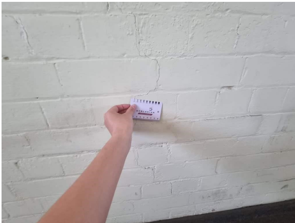
PHOTO 72 (Photo showing cracks are 0.1mm in width)
