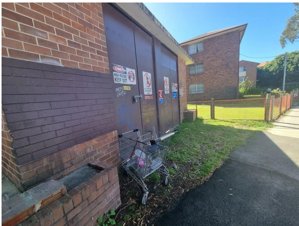
PHOTO 12 (Overview of footpath and street facing façade of 215 Cope Street)
