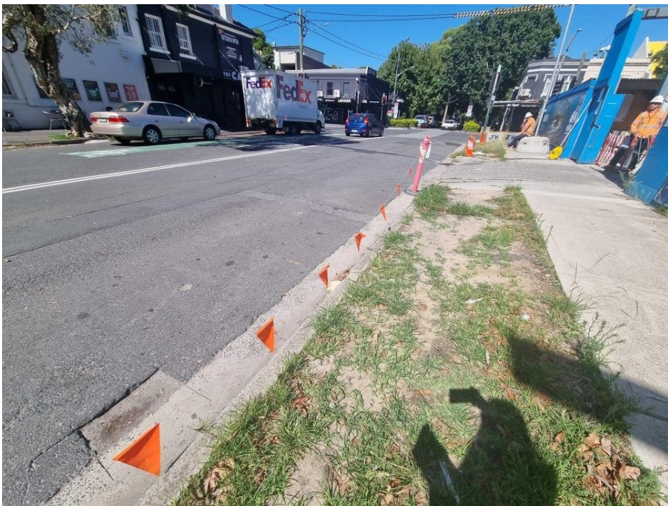
PHOTO 80 (Overview of footpath and road on Wellington Street)
