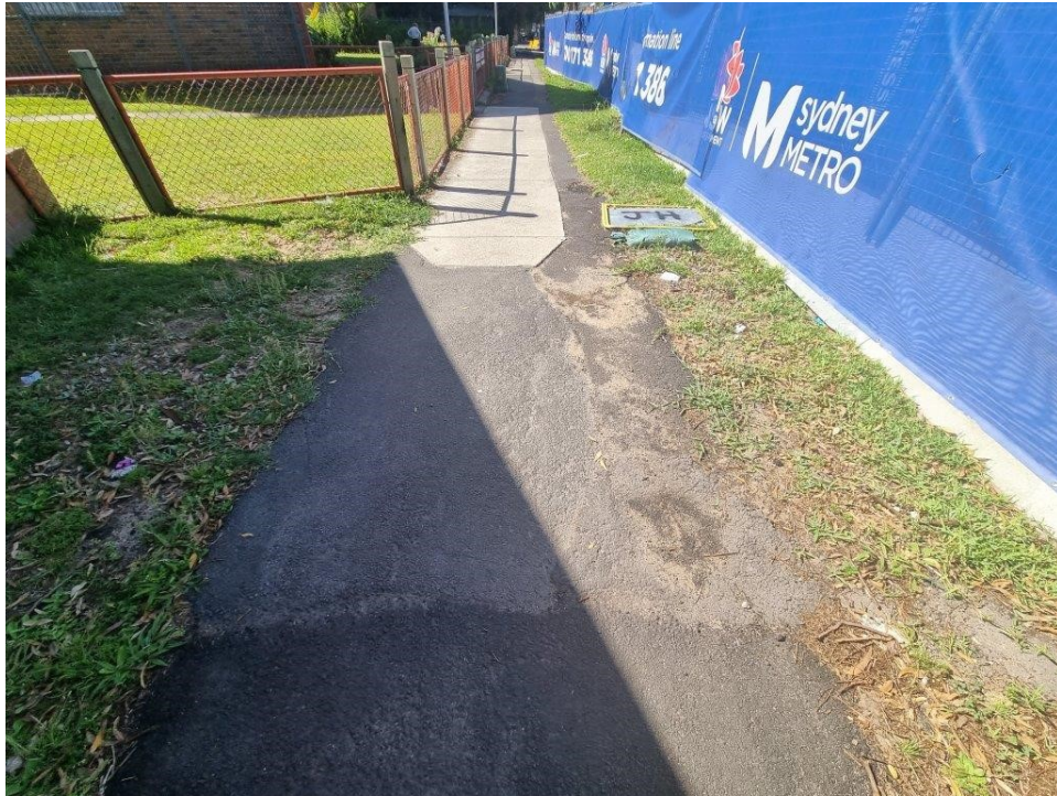
PHOTO 13 (Overview of footpath adjacent 215 Cope Street)
