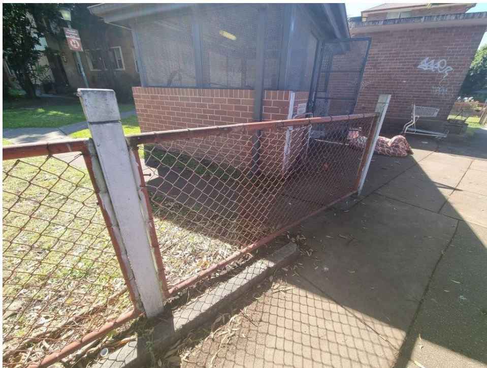
PHOTO 4 (Photo showing condition of boundary fence of 213-215 Cope Street)
