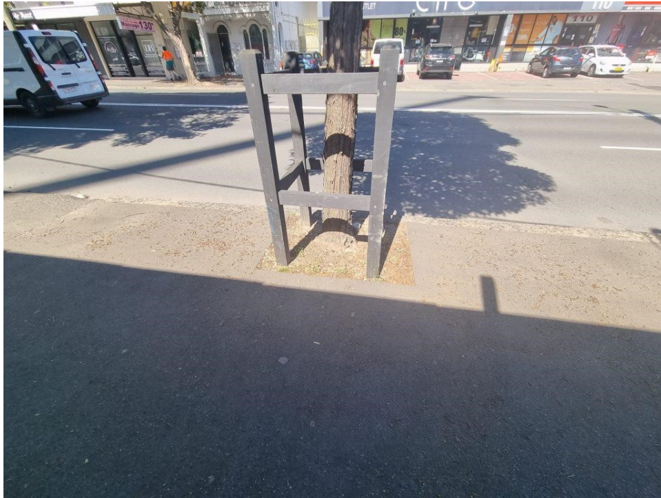
PHOTO 121 (Overview of footpath, kerb and tree along Botany Road)
