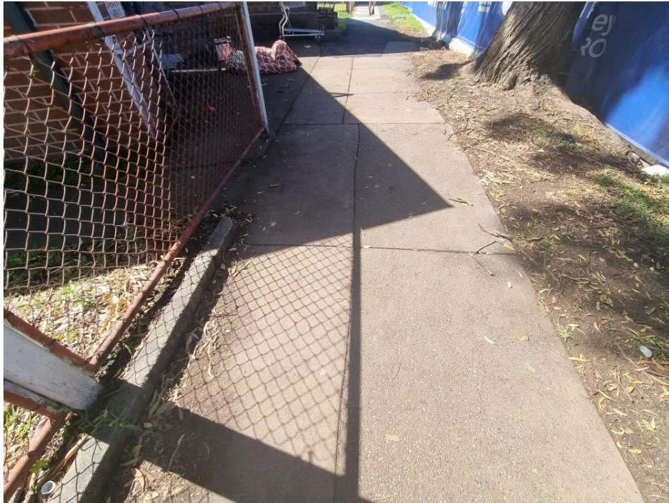
PHOTO 3 (Overview of footpath adjacent 213-215 Cope Street)
