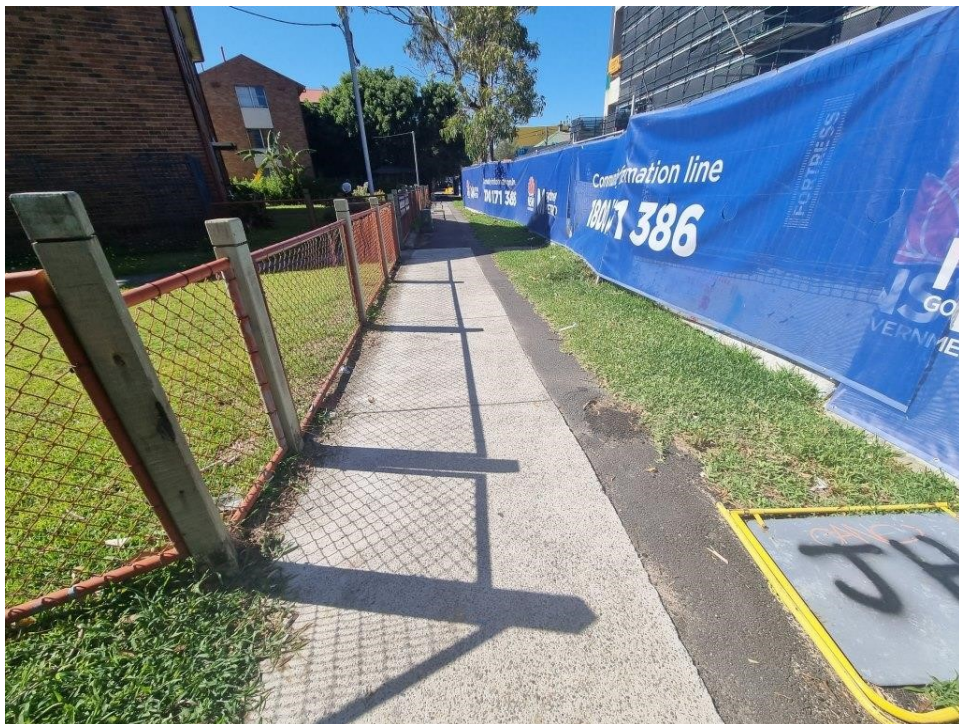
PHOTO 14 (Overview of footpath adjacent 215 Cope Street)
