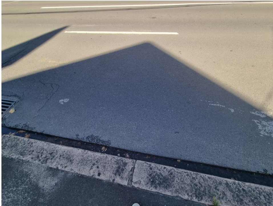
PHOTO 153 (Overview of road adjacent church)
