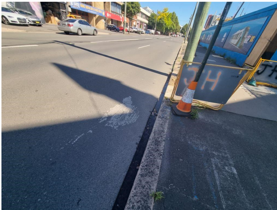
PHOTO 154 (Overview of road, kerb and footpath adjacent church facing North)
