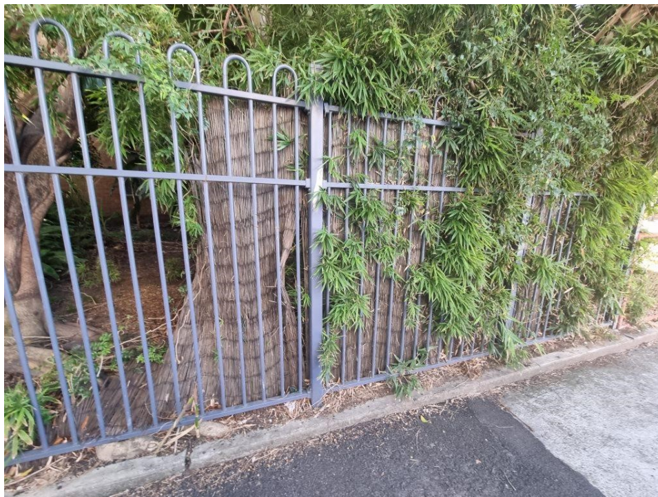
PHOTO 43 (Overview of boundary fence of 113 Wellington Street)
