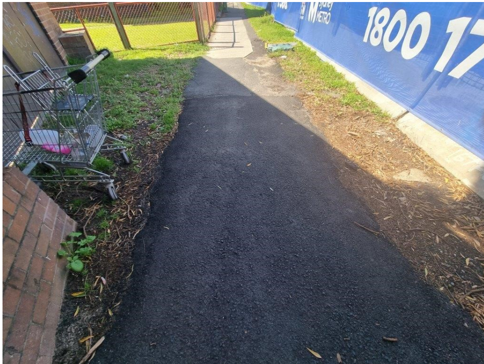
PHOTO 11 (Overview of footpath adjacent 215 Cope Street)
