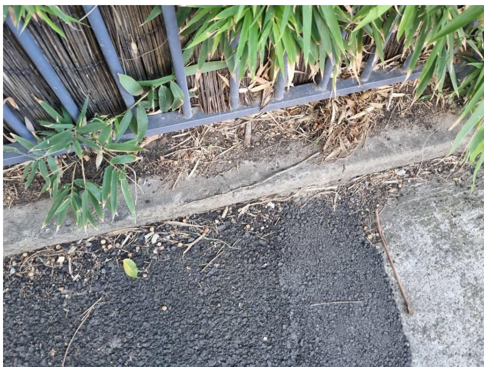
PHOTO 44 (Overview of boundary fence of 113 Wellington Street)
