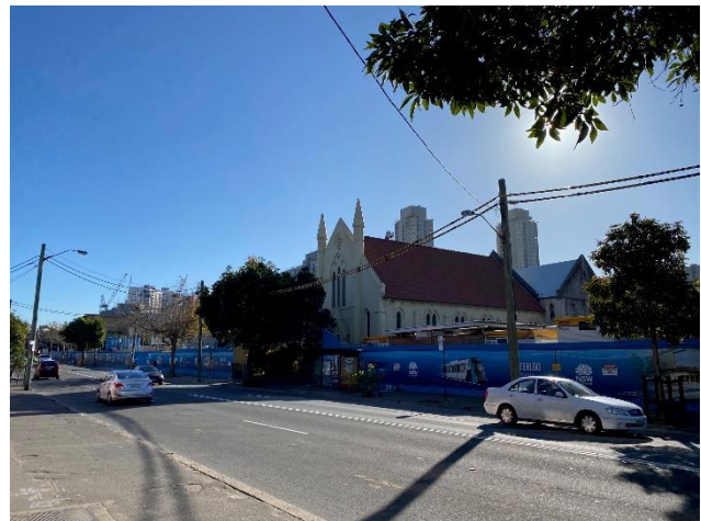
Picture 12 Botany Road street frontage, looking north east
