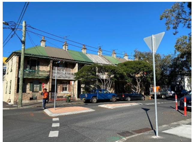
Picture 22 Terrace housing on Wellington Street, south of the site, looking south
