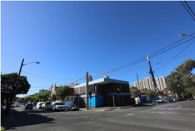
Picture 27 Previous site development (prior to site clearing)
