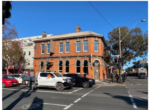
Picture 20 Locally heritage listed Former CBC Bank, including Interior located at 60 Botany Road
