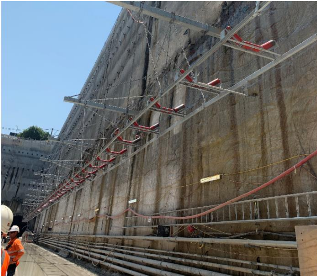
Figure 7 - Exposed face of the excavation, depicting the Hawkesbury Sandstone formation
