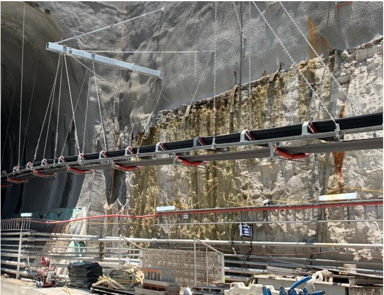
Figure 8 - Section of exposed Hawkesbury Sandstone underneath the proposed BLD 3
