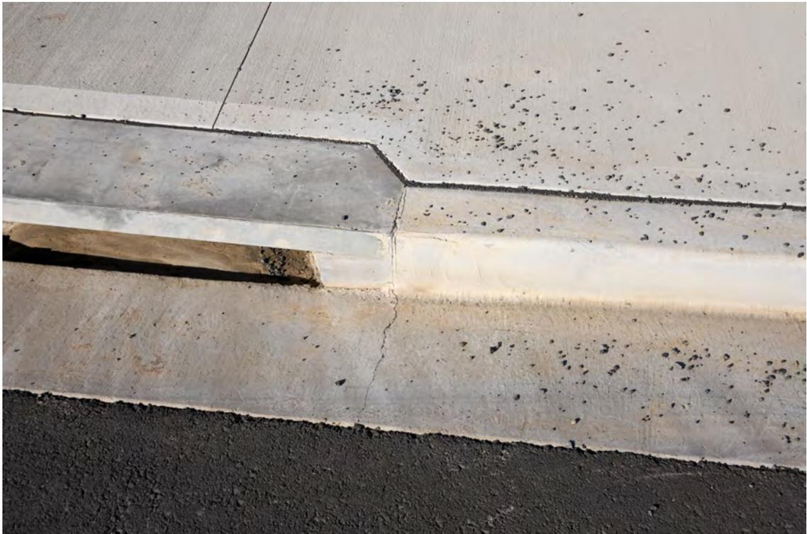
Johnston Crescent. Area adjacent to 6 Johnston Crescent (to the north of the site). Heading south along the eastern side of the Crescent. Area between light pole ID 957686 and 957687. Storm water drain. Cracked gutter.
