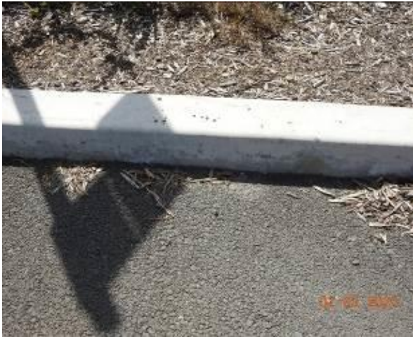
Figure 2111 – Crack propagation through kerb
