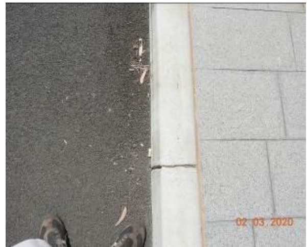
Figure 2102 – Crack propagation through kerb
