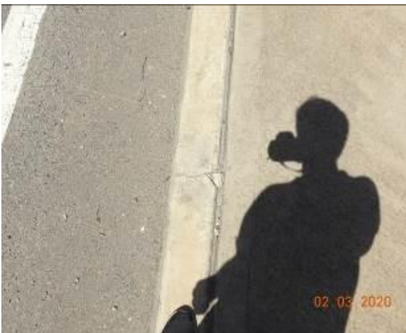
Figure 1532 – Crack propagation and loss of material through kerb
