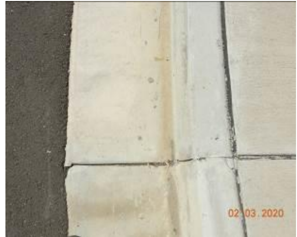
Figure 2046 – Loss of material through kerb and gutter
