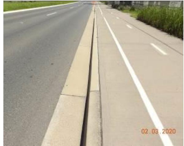
Figure 1619 – General Condition of kerb and gutter
