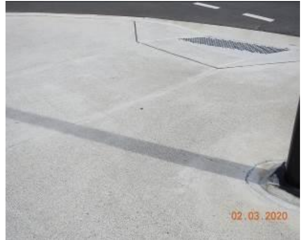
Figure 1920 – Crack propagation through footpath pavement
