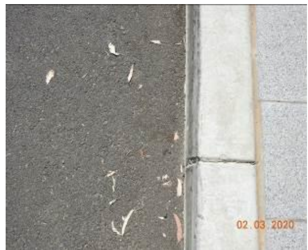
Figure 2138 – Crack propagation through kerb
