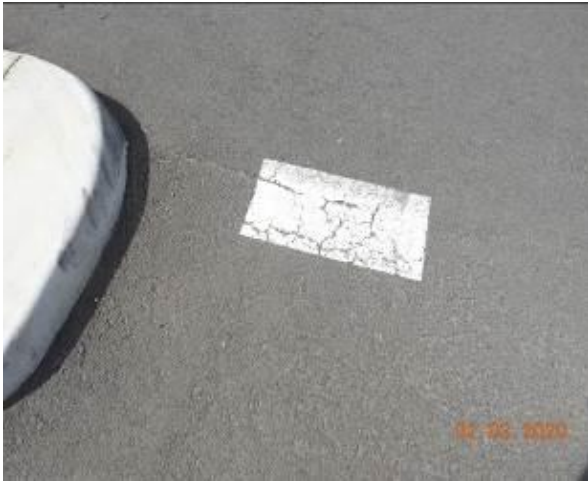
Figure 2654 – Crack propagation through carpark pavement
