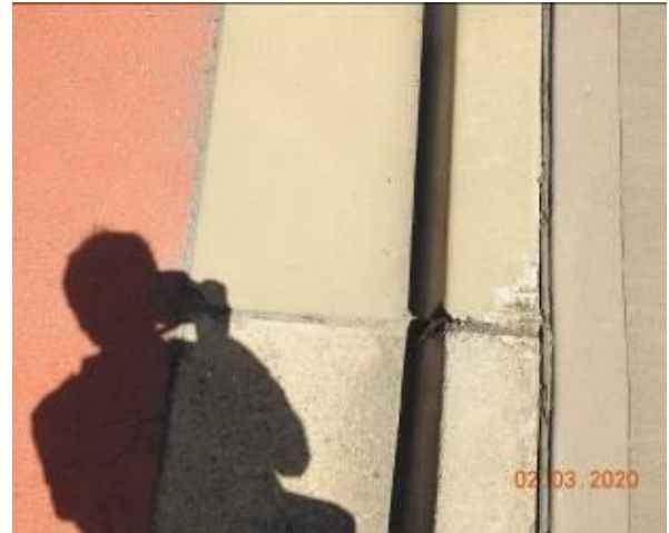
Figure 1655 – Loss of material through kerb and gutter
