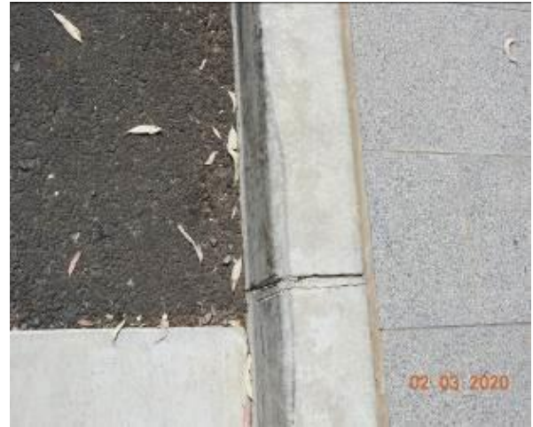
Figure 2136 – Crack propagation through kerb
