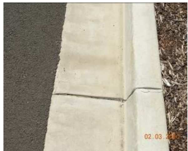
Figure 2116 – Crack propagation through kerb and gutter
