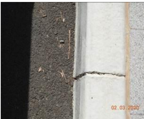
Figure 2085 – Crack propagation through kerb
