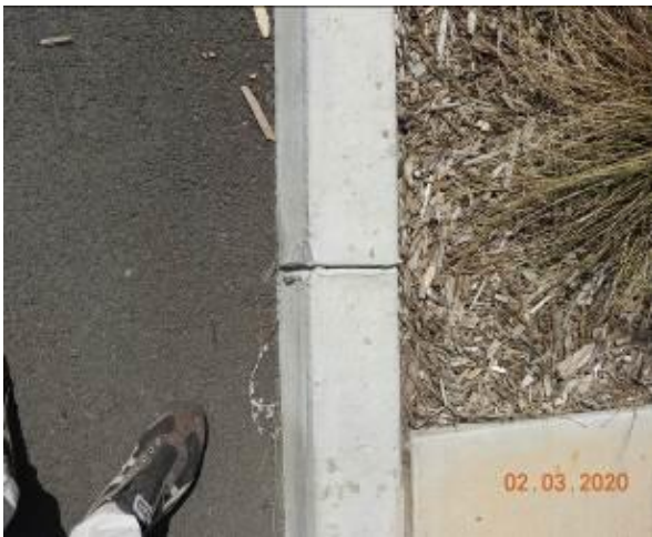
Figure 2011 – Crack propagation through kerb
