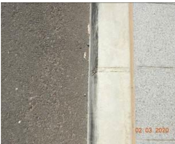
Figure 2145 – Crack propagation through kerb
