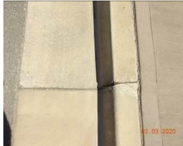
Figure 1499 – Crack propagation through kerb
