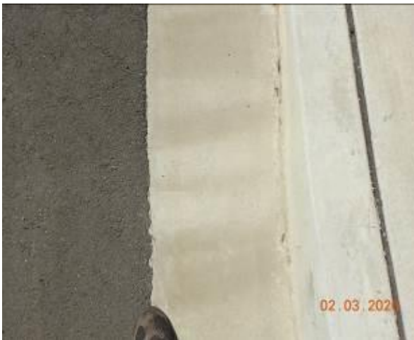
Figure 2041 – Crack propagation through layback and gutter
