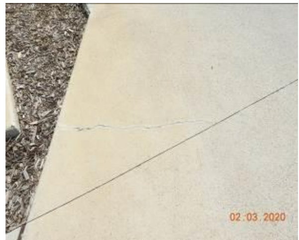
Figure 2515 – Crack propagation through driveway pavement
