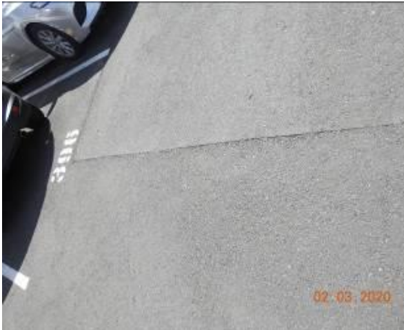
Figure 3018 – Crack propagation through carpark pavement
