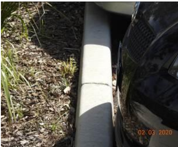
Figure 3104 – Crack propagation through kerb
