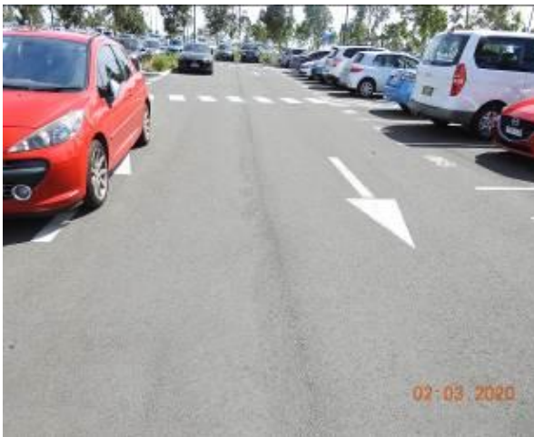
Figure 2996 – Loss of material through carpark pavement
