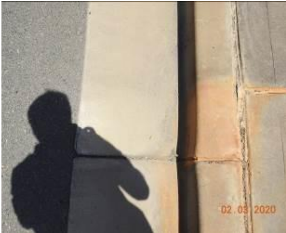
Figure 1594 – Loss of material through gutter
