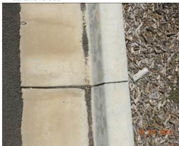
Figure 1997 – Loss of material through kerb and gutter
