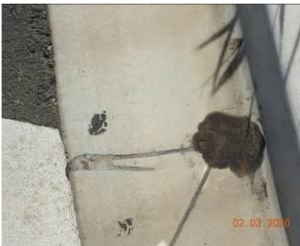
Figure 1953 – Loss of material through gutter
