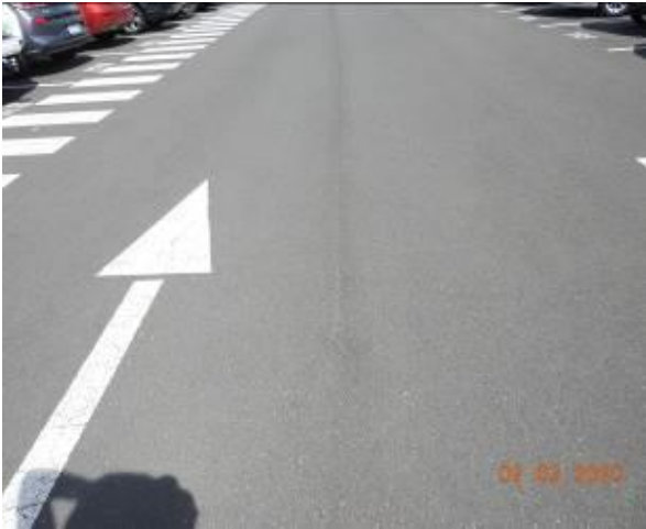
Figure 2958 – Crack propagation through carpark pavement
