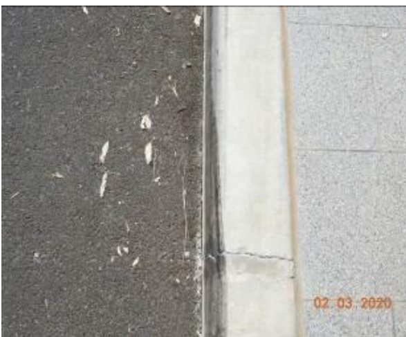
Figure 2137 – Crack propagation through kerb
