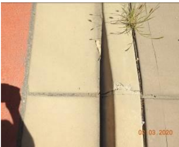
Figure 1698 – Loss of material through kerb
