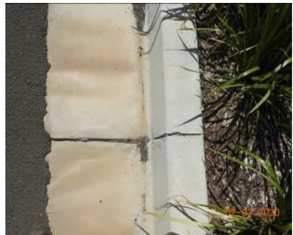
Figure 1984 – Crack propagation through kerb
