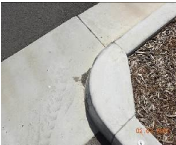
Figure 2151 – Crack propagation through kerb
