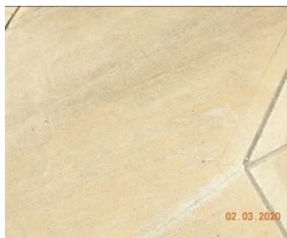
Figure 1471 – Crack propagation through footpath pavement
