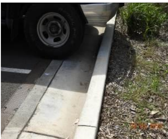
Figure 2462 – General Condition of kerb and gutter
