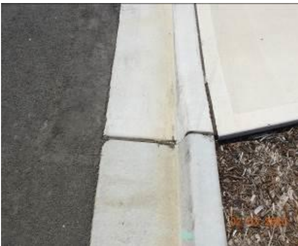
Figure 2181 – Crack propagation and loss of material through kerb and gutter
