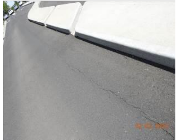
Figure 2887 – Crack propagation through carpark pavement
