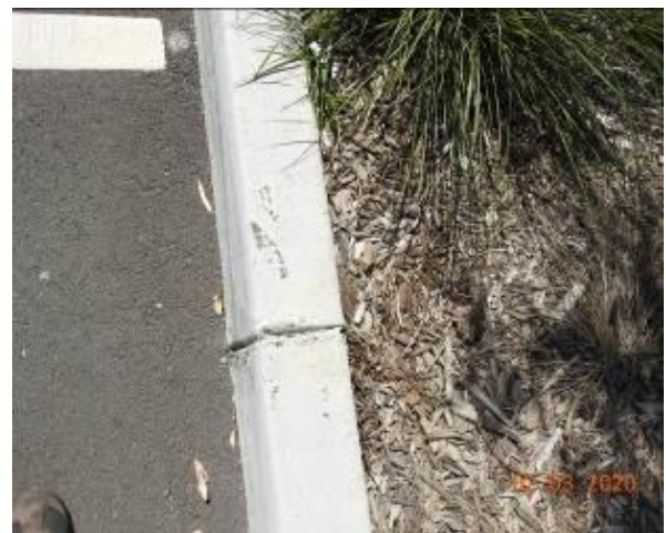
Figure 2020 – Loss of material through kerb
