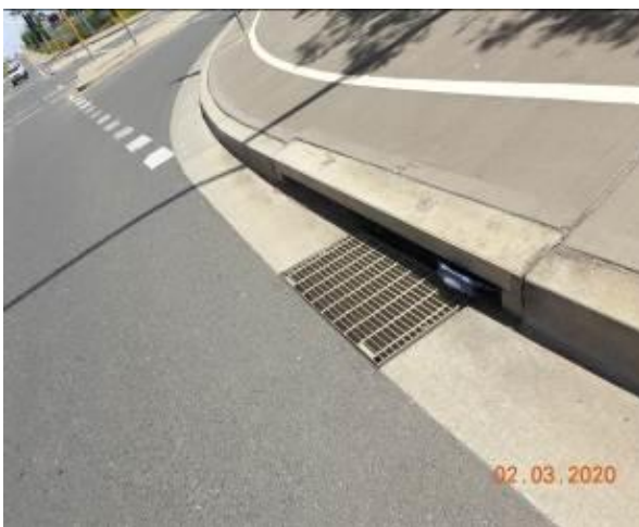
Figure 1500 – General Condition of stormwater inlet pit
