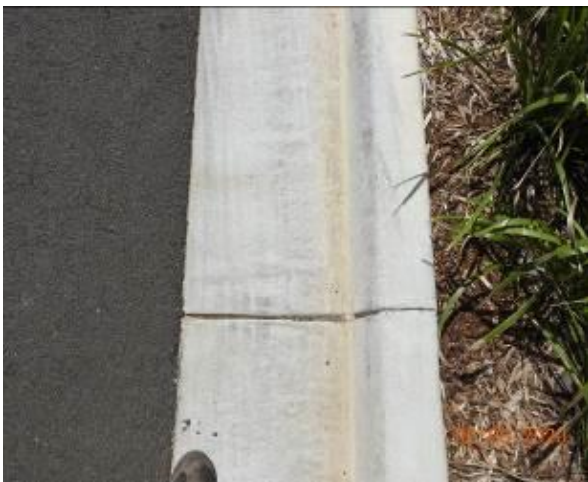
Figure 2175 – Crack propagation through kerb and gutter
