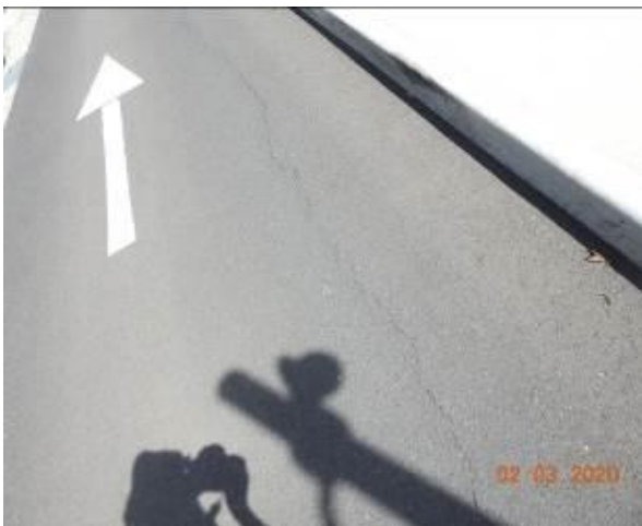
Figure 2884 – Crack propagation through carpark pavement
