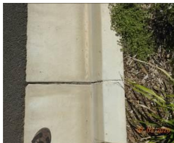
Figure 1972 – Crack propagation and loss of material through kerb and gutter
