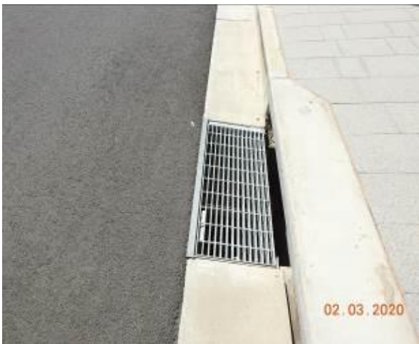
Figure 2167 – General Condition of stormwater inlet pit
