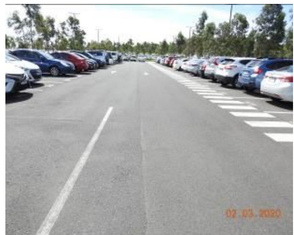
Figure 3017 – Crack propagation through carpark pavement
