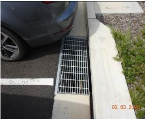
Figure 2490 – General Condition of stormwater inlet pit
