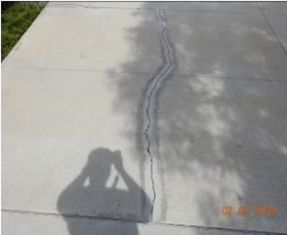
Figure 1931 – Crack propagation and loss of material through footpath pavement
