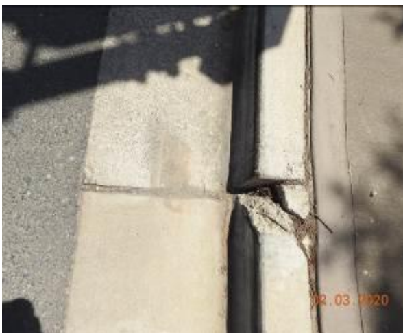
Figure 1506 – Loss of material through kerb
