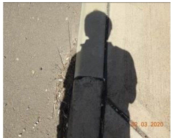
Figure 1537 – Loss of material through kerb
