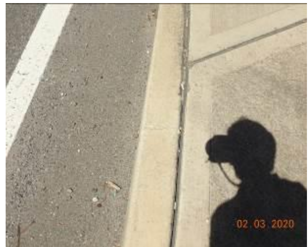
Figure 1533 – Crack propagation through kerb
