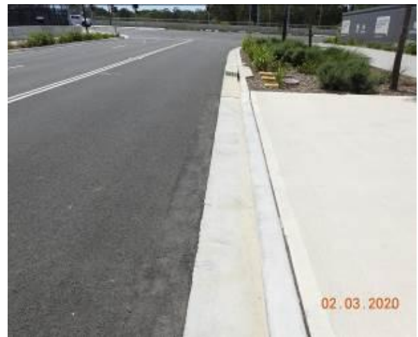
Figure 2182 – General Condition of layback and gutter
