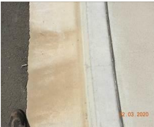
Figure 2047 – Crack propagation through kerb and gutter
