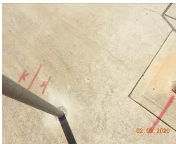
Figure 1468 – Crack propagation through footpath pavement
