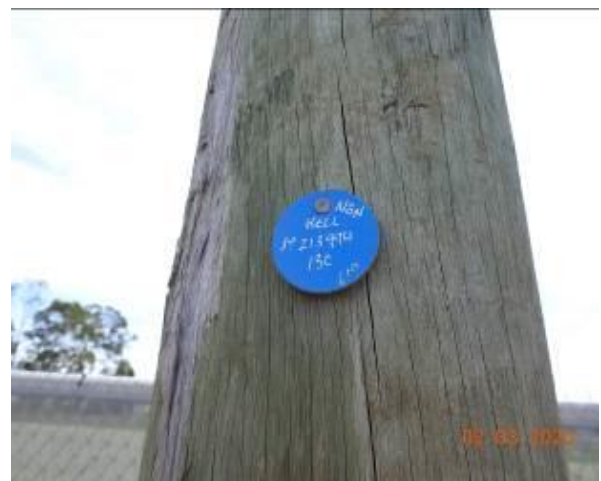
Figure 1827 – General Condition of telegraph pole Identification No.213994/130
