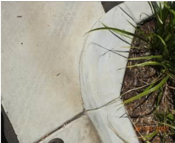
Figure 2059 – Crack propagation through kerb and gutter
