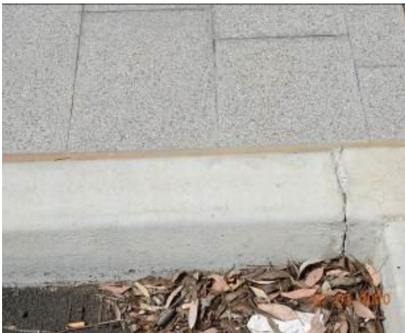
Figure 2083 – Separation through kerb
