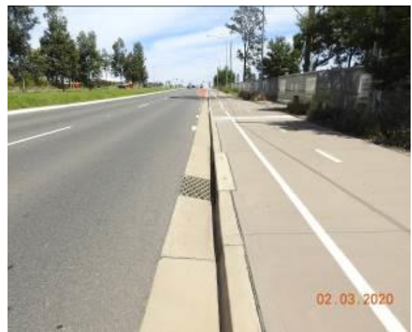
Figure 1627 – General Condition of kerb and gutter
