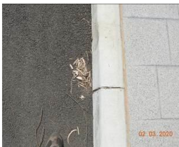
Figure 2073 – Crack propagation through kerb
