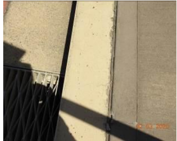
Figure 1667 – Crack propagation through stormwater inlet pit
