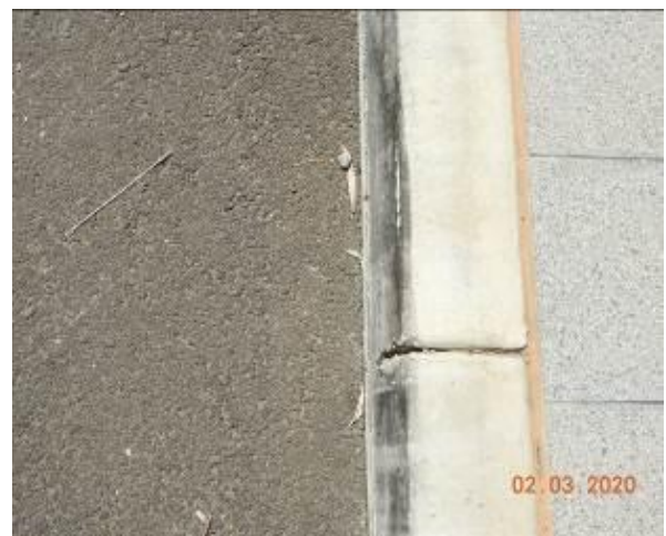
Figure 2146 – Crack propagation and loss of material through kerb
