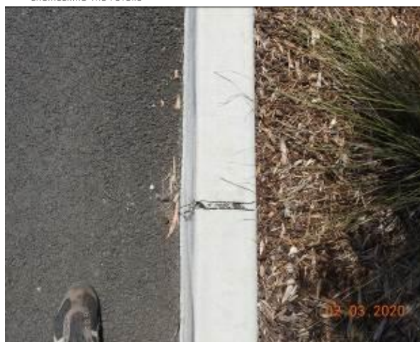
Figure 2069 – Crack propagation and loss of material through kerb
