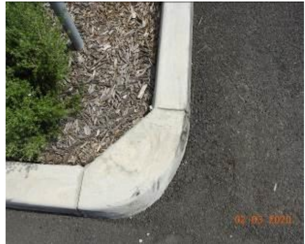
Figure 2509 – Crack propagation through kerb
