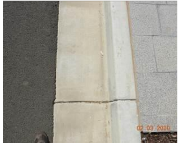
Figure 2154 – Crack propagation through kerb and gutter
