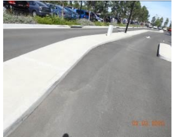
Figure 2863 – Evidence of patchwork through carpark pavement
