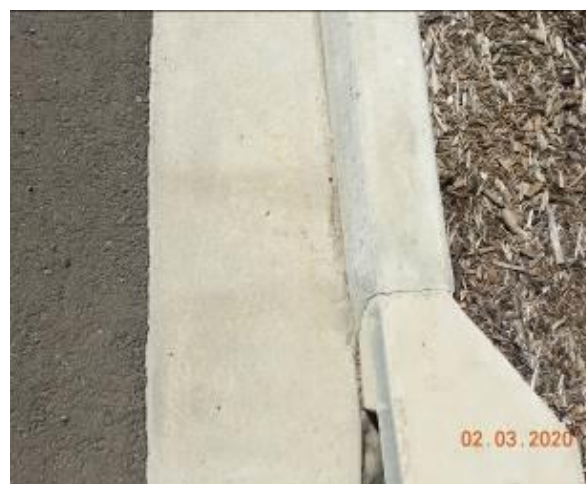
Figure 2038 – Crack propagation through stormwater inlet pit
