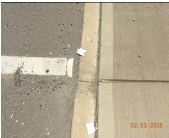
Figure 1520 – Crack propagation through layback
