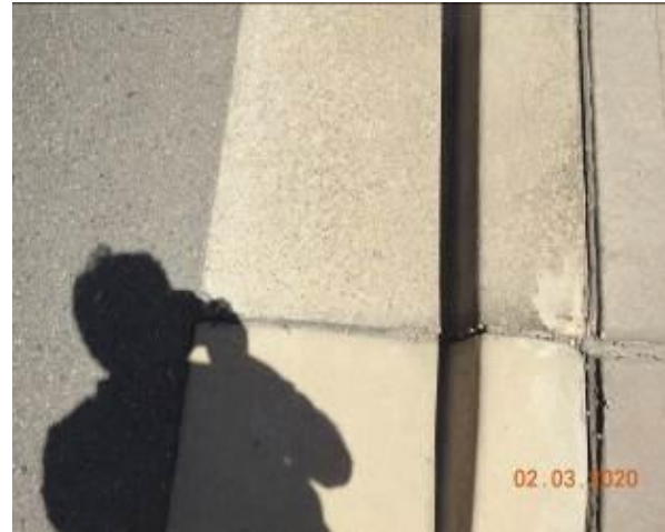
Figure 1607 – Loss of material through kerb
