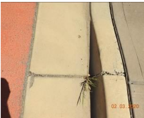
Figure 1686 – Loss of material through kerb and gutter
