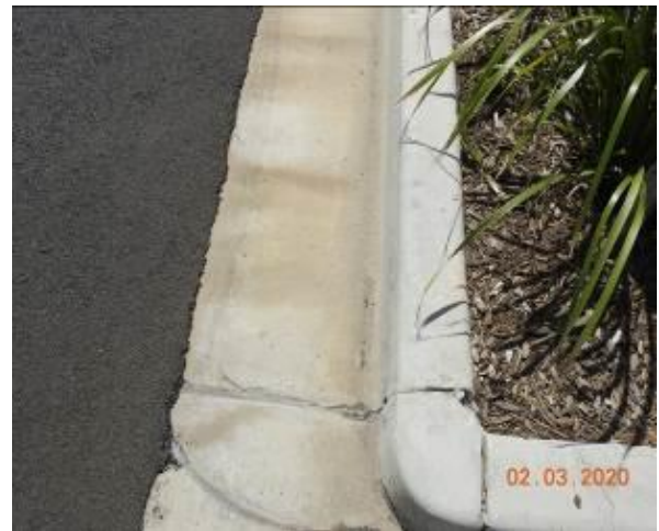
Figure 2030 – Loss of material through kerb
