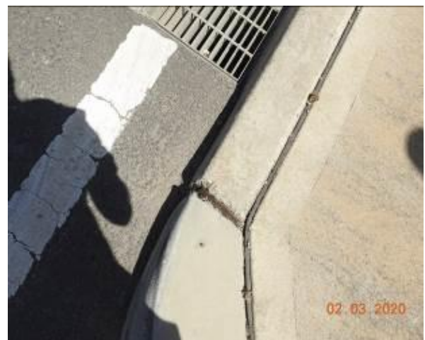
Figure 1539 – Loss of material through kerb
