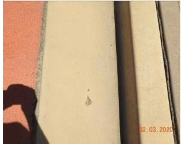
Figure 1685 – Loss of material through gutter
