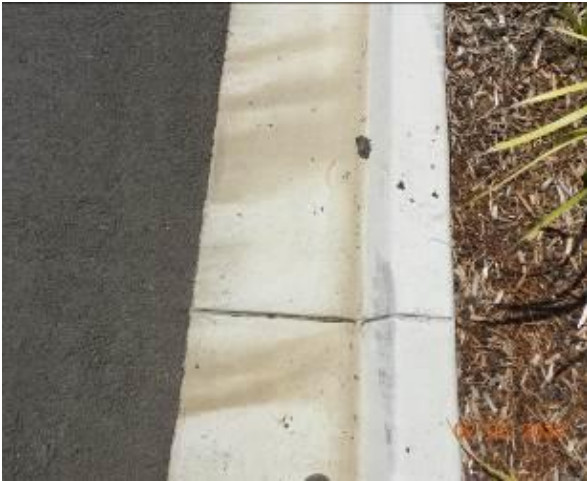
Figure 2189 – Crack propagation through kerb and gutter
