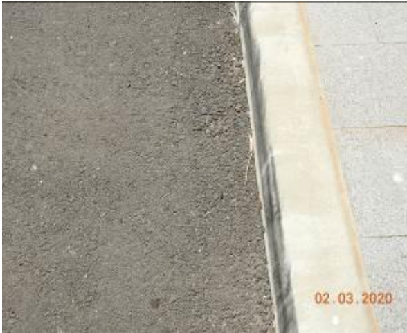
Figure 2147 – Crack propagation through kerb
