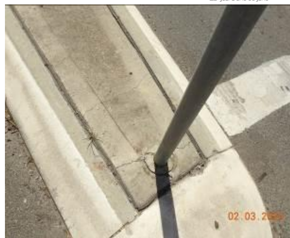
Figure 1475 – Crack propagation through traffic island footpath pavement
