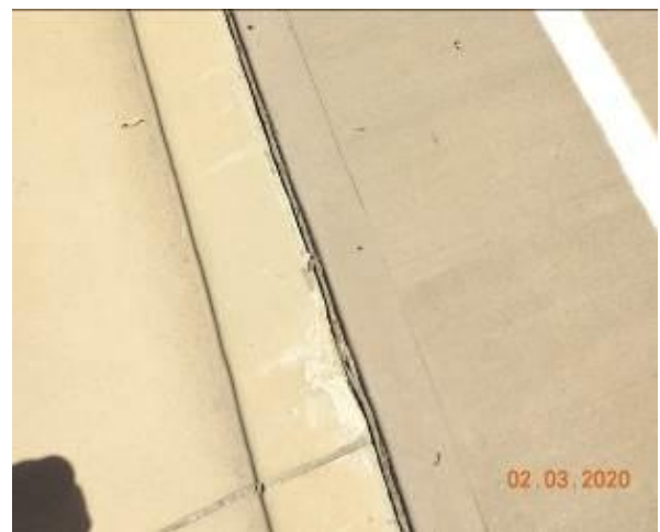
Figure 1687 – Loss of material through layback
