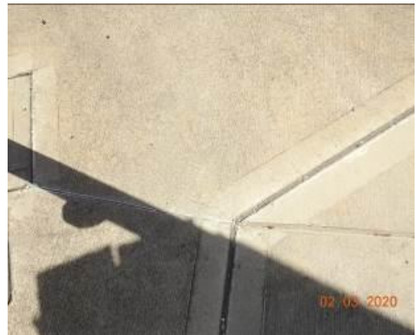
Figure 1483 – Crack propagation through footpath pavement
