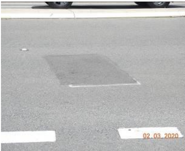
Figure 1794 – Evidence of patchwork through road surface
