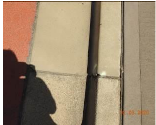
Figure 1669 – Loss of material through kerb
