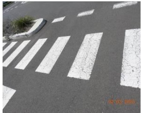
Figure 2651 – Crack propagation through carpark pavement
