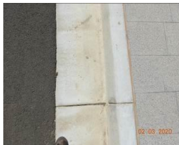
Figure 2164 – Crack propagation through kerb and gutter
