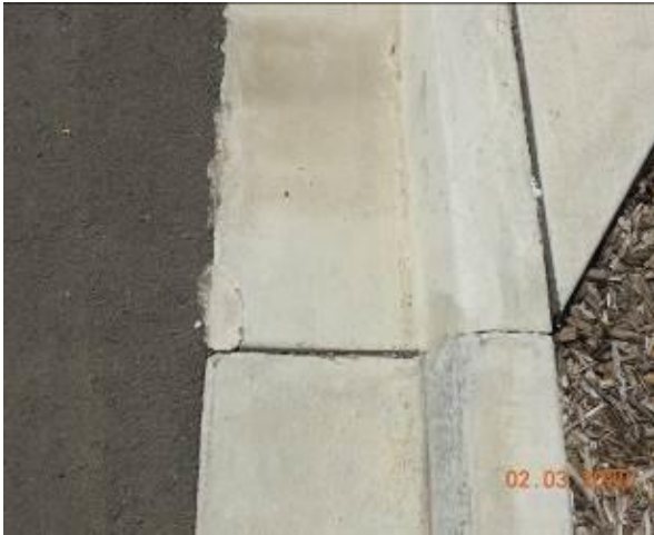
Figure 2039 – Crack propagation through gutter
