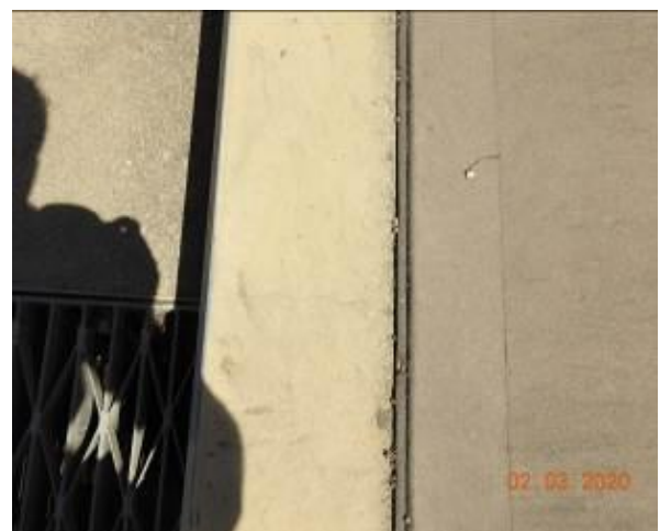
Figure 1575 – Crack propagation through stormwater inlet pit
