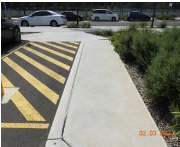
Figure 2468 – Crack propagation through footpath pavement
