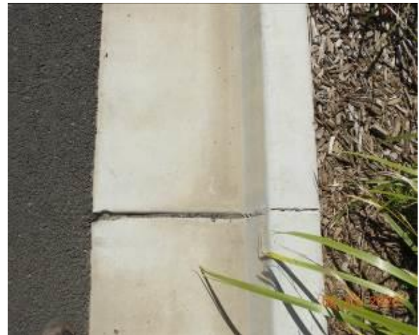
Figure 1976 – Crack propagation through kerb and gutter
