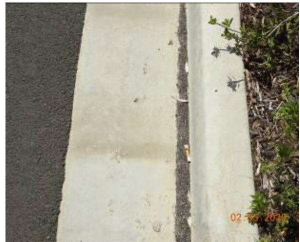
Figure 2114 – Crack propagation through kerb
