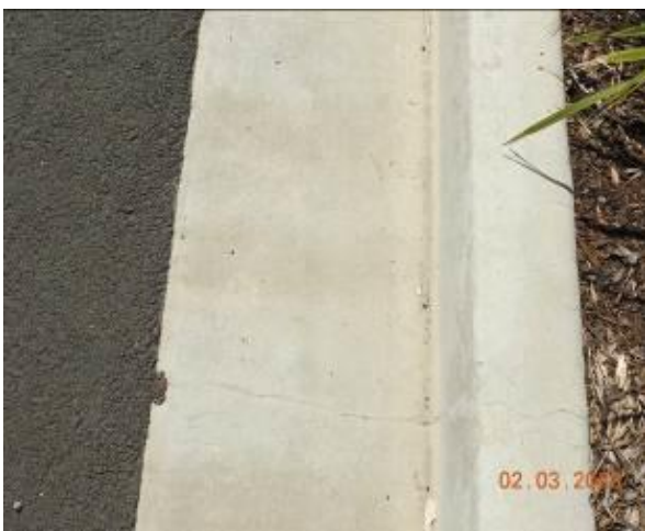
Figure 2115 – Crack propagation through kerb and gutter
