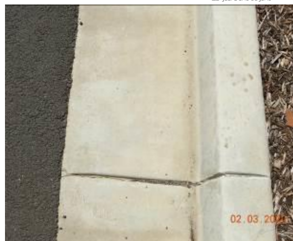
Figure 2118 – Crack propagation through kerb and gutter
