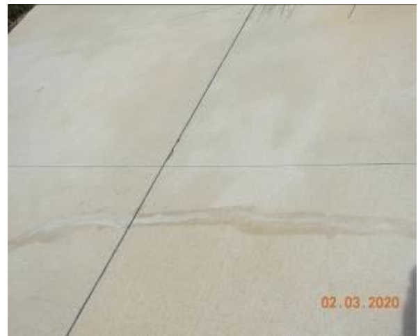
Figure 1940 – Loss of material through footpath pavement
