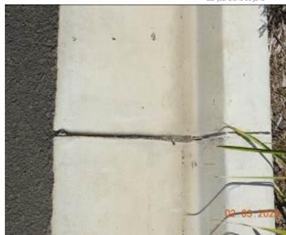
Figure 1968 – Crack propagation and loss of material through kerb and gutter
