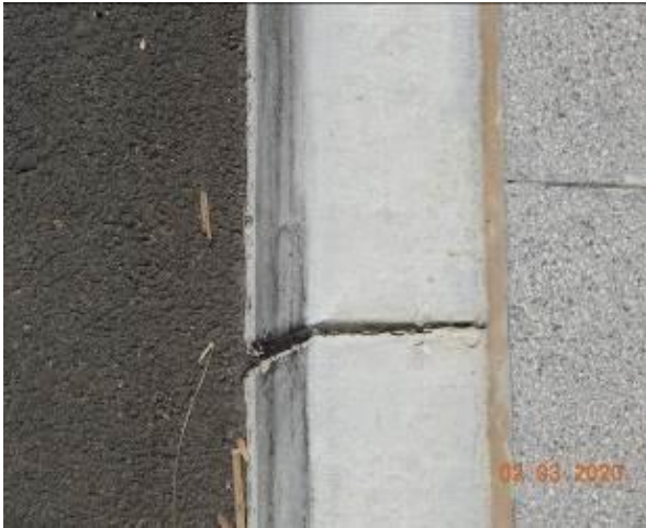
Figure 2087 – Crack propagation and loss of material through kerb
