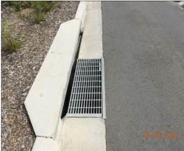
Figure 2786 – General Condition of stormwater inlet pit
