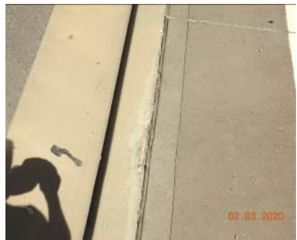
Figure 1639 – Loss of material through kerb
