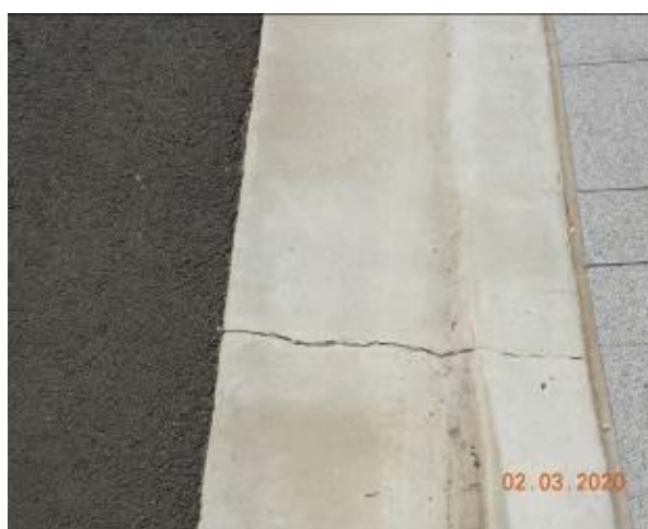
Figure 2121 – Crack propagation through layback and gutter
