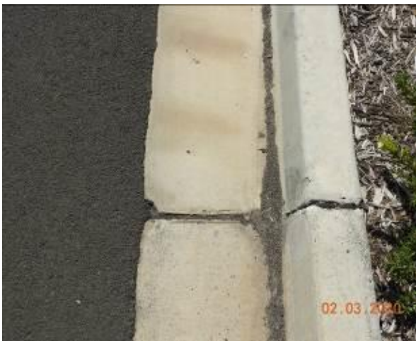
Figure 1983 – Loss of material through kerb and gutter
