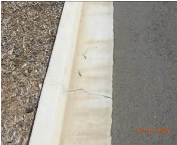
Figure 2788 – Crack propagation through kerb and gutter
