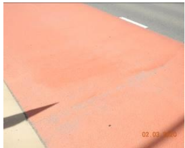
Figure 1713 – Crack propagation through road surface
