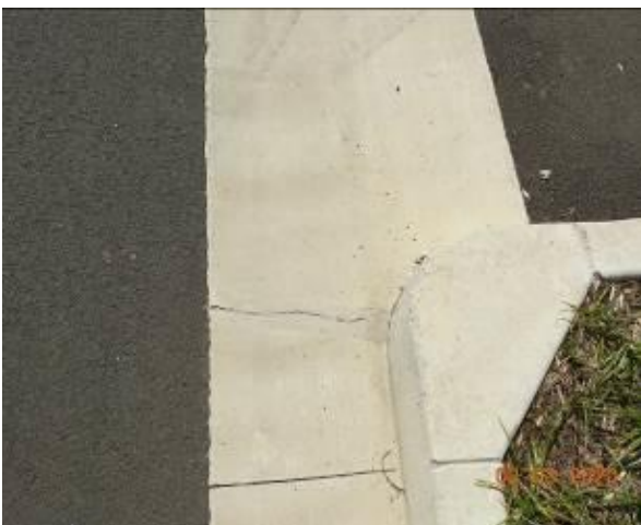
Figure 2097 – Crack propagation through gutter
