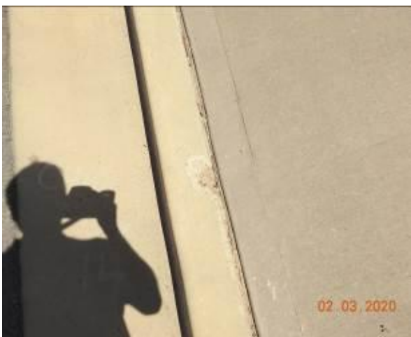
Figure 1562 – Loss of material through kerb
