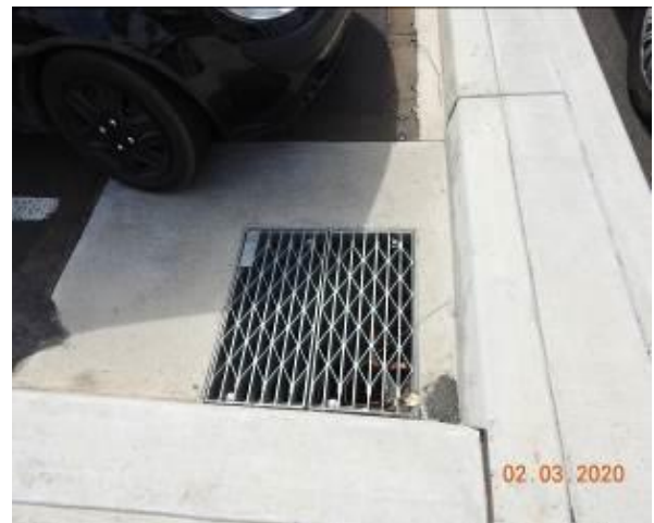
Figure 2493 – General Condition of stormwater inlet pit
