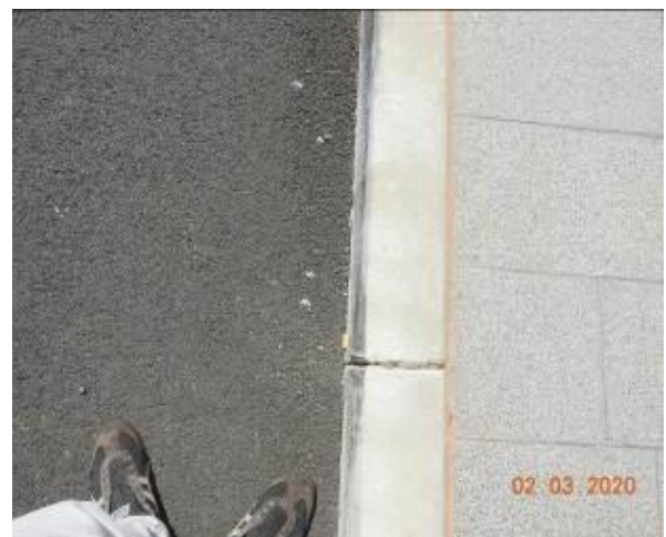
Figure 2104 – Crack propagation through kerb
