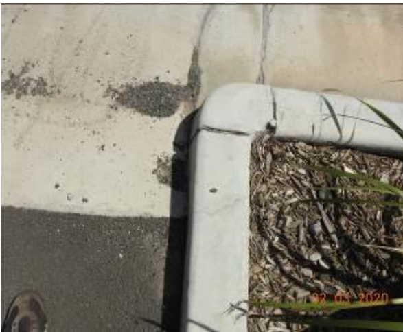
Figure 2029 – Crack propagation through kerb
