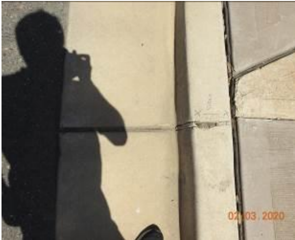
Figure 1558 – Crack propagation through kerb and gutter
