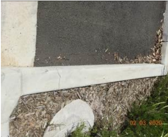
Figure 2003 – Crack propagation through curb
