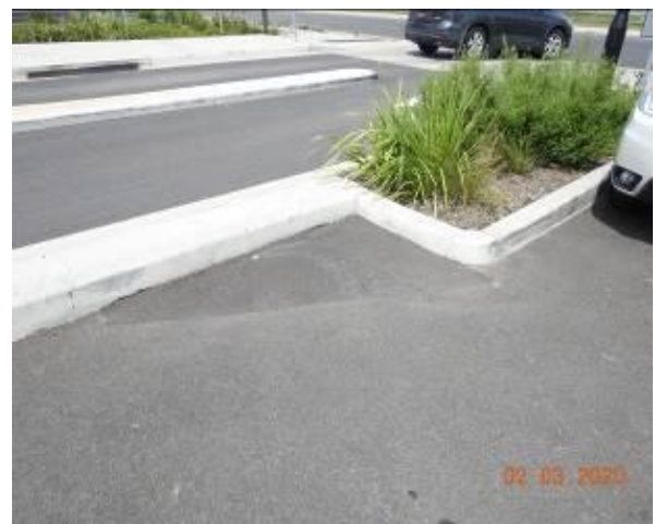
Figure 2361 – Crack propagation through carpark pavement
