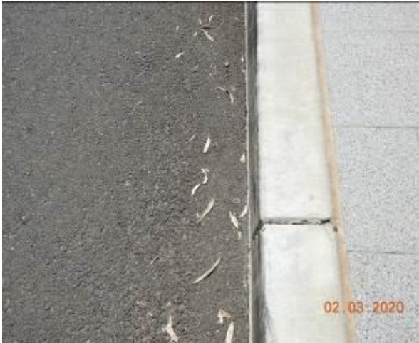
Figure 2141 – Crack propagation through kerb
