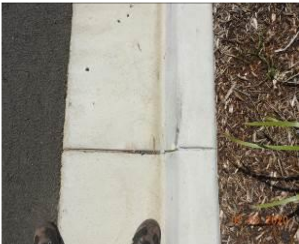
Figure 2187 – Crack propagation through kerb and gutter
