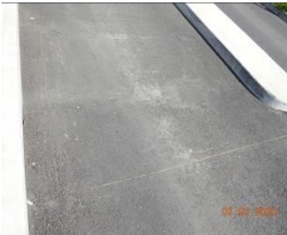
Figure 2870 – Crack propagation through carpark pavement
