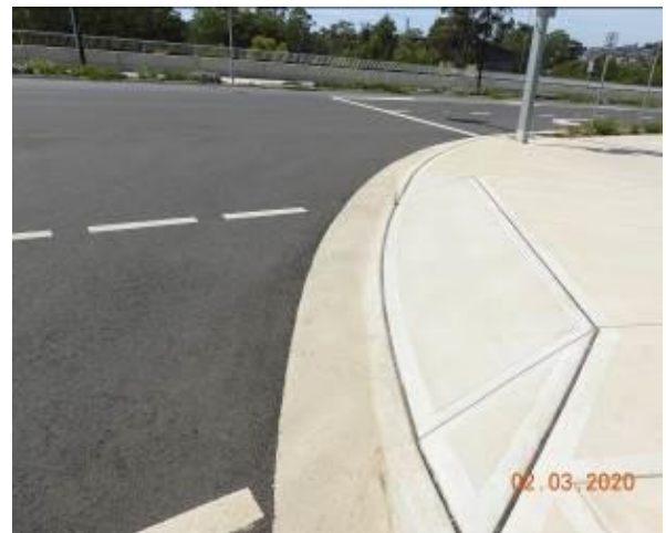
Figure 2194 – General Condition of layback and gutter
