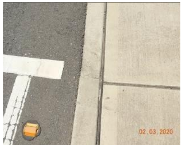
Figure 1551 – Crack propagation through kerb
