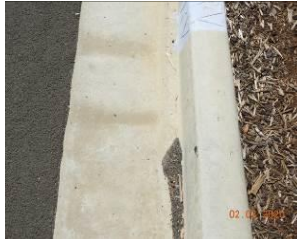
Figure 2124 – Crack propagation through kerb and gutter
