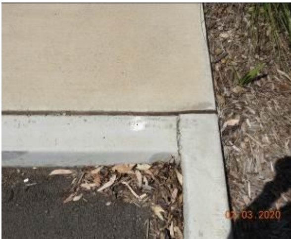
Figure 2017 – Crack propagation and loss of material through kerb
