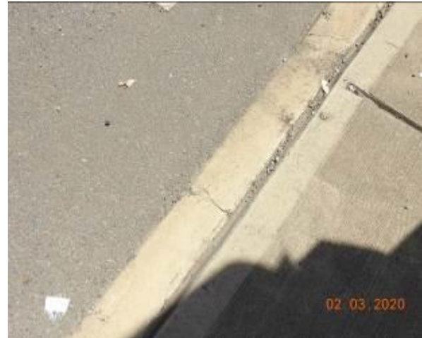
Figure 1523 – Crack propagation through layback
