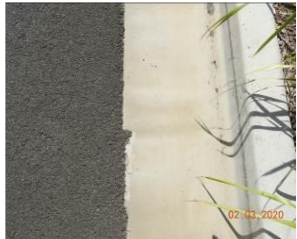
Figure 1964 – Loss of material through gutter
