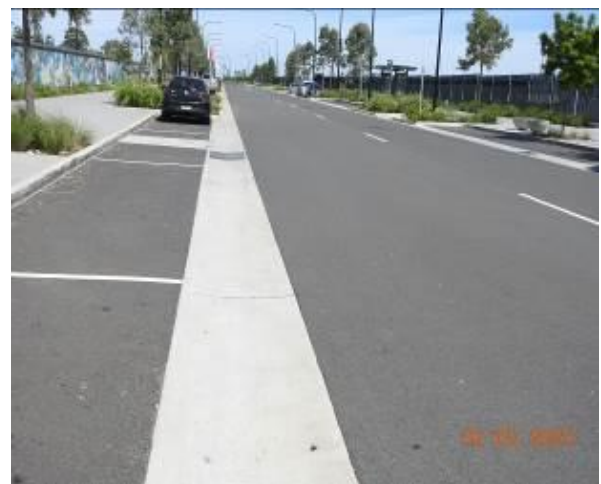
Figure 2212 – General Condition of road surface
