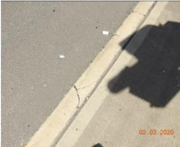
Figure 1522 – Crack propagation and loss of material through layback
