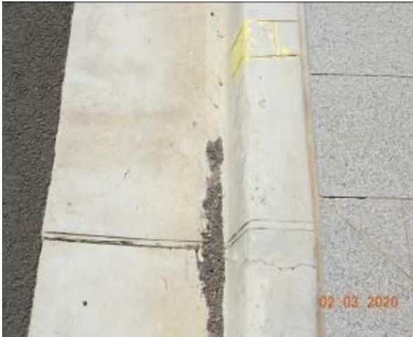
Figure 2123 – Crack propagation through kerb and gutter
