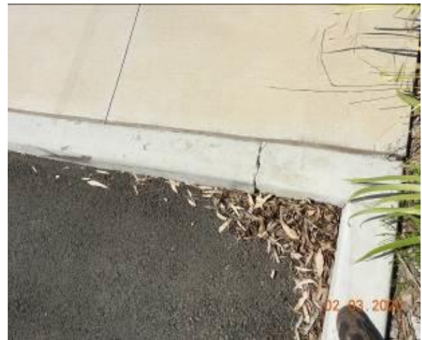
Figure 2006 – Crack propagation through curb
