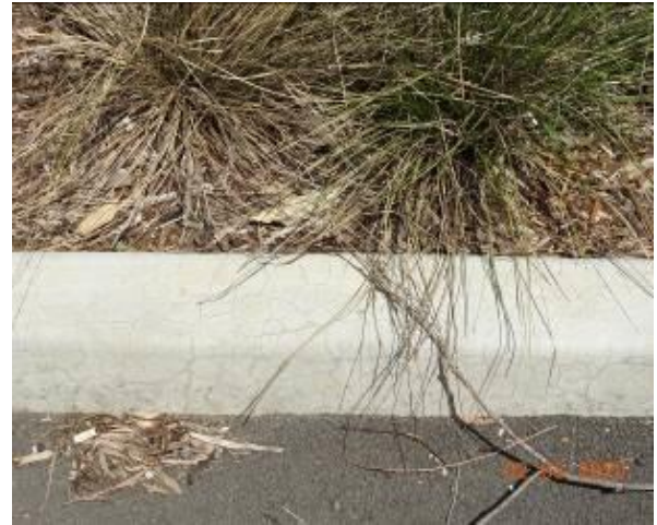
Figure 2082 – Crack propagation through kerb
