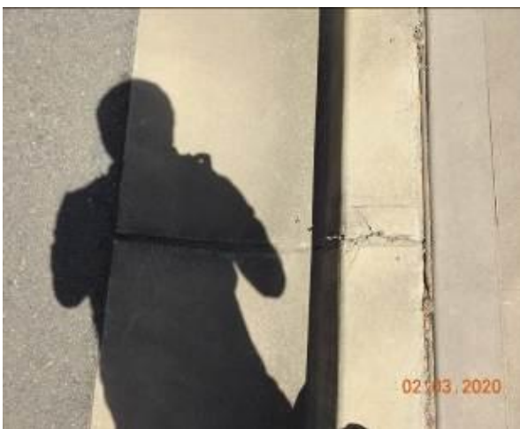
Figure 1566 – Loss of material through kerb
