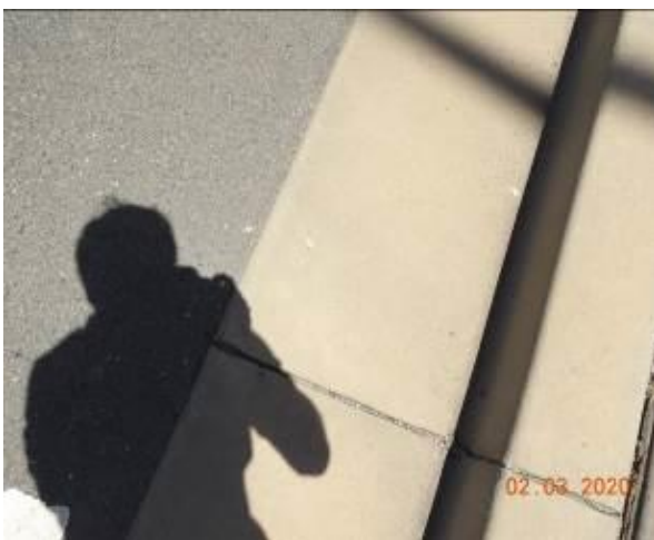
Figure 1638 – Crack propagation through kerb
