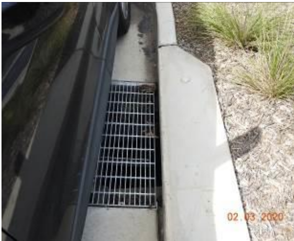
Figure 2812 – General Condition of stormwater inlet pit
