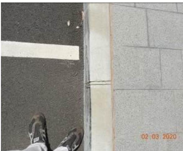
Figure 2103 – Crack propagation through kerb
