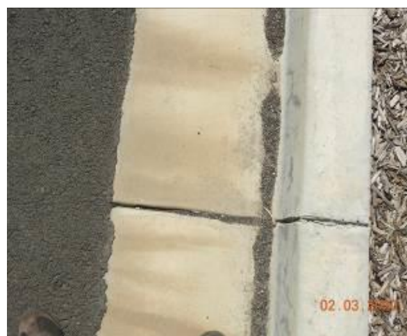
Figure 2000 – Crack propagation through kerb and gutter
