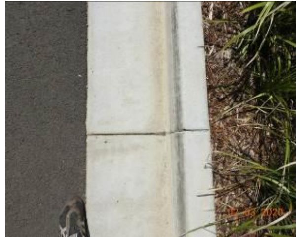
Figure 2172 – Crack propagation through kerb and gutter
