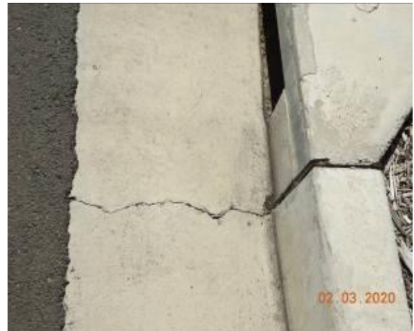
Figure 1958 – Crack propagation through gutter
