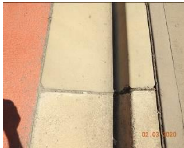
Figure 1695 – Loss of material through kerb and gutter
