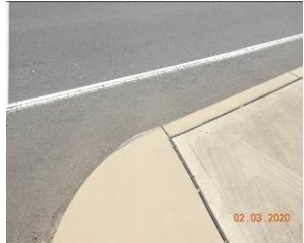
Figure 1547 – Crack propagation through kerb
