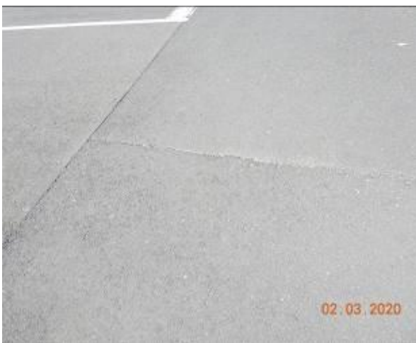
Figure 2912 – Crack propagation through carpark pavement
