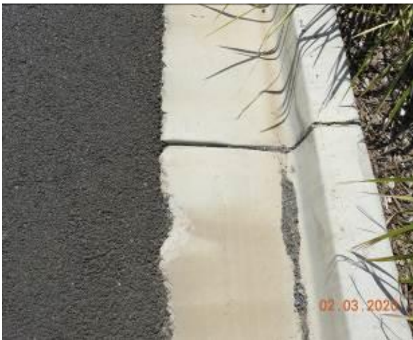
Figure 1963 – Loss of material through gutter
