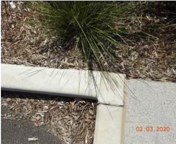
Figure 2075 – Crack propagation through kerb
