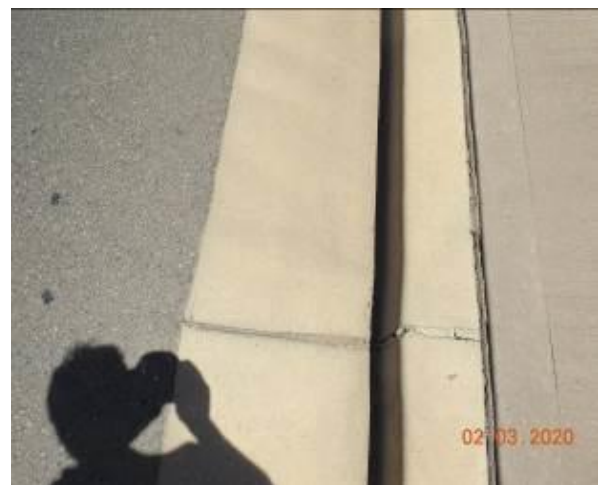
Figure 1615 – Crack propagation through kerb and gutter
