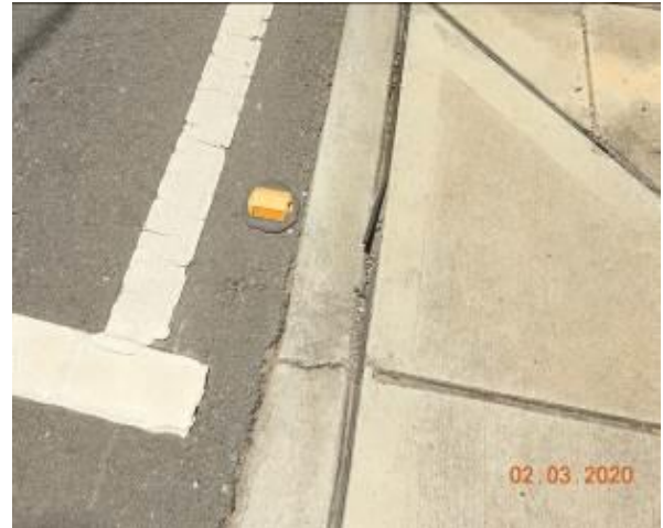
Figure 1553 – Crack propagation through kerb
