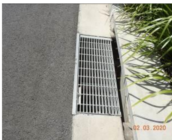
Figure 2053 – General Condition of stormwater inlet pit
