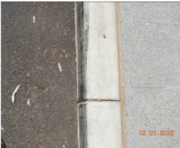
Figure 2143 – Crack propagation through kerb
