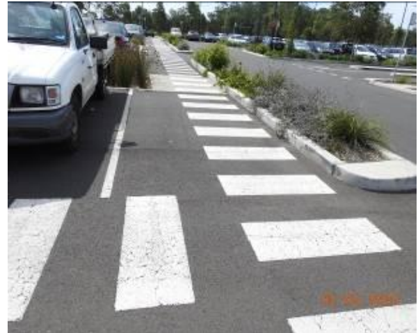
Figure 2649 – Crack propagation through carpark pavement
