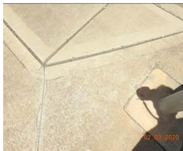
Figure 1479 – Crack propagation through footpath pavement
