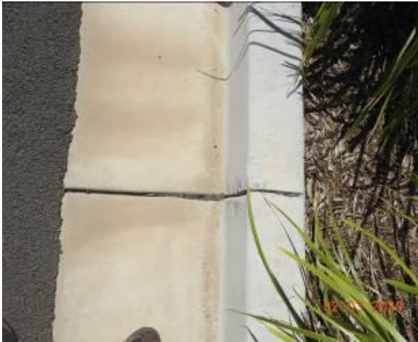
Figure 1985 – Crack propagation through kerb
