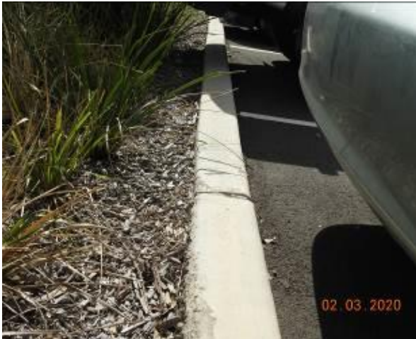
Figure 2834 – Loss of material through kerb
