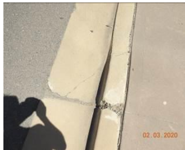
Figure 1633 – Crack propagation and loss of material through kerb and gutter
