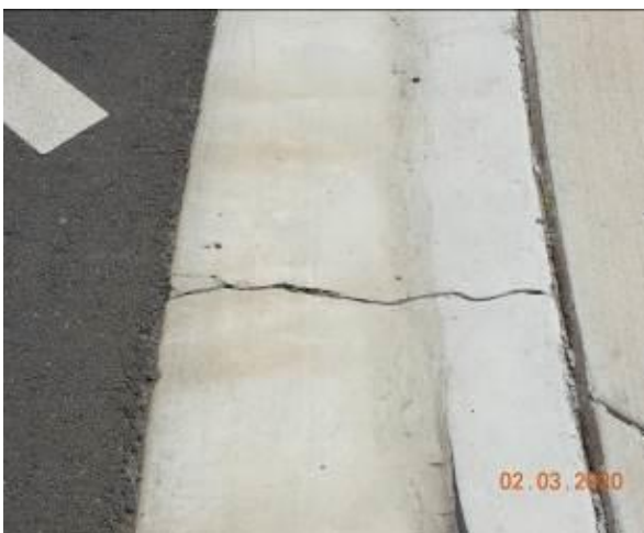
Figure 1951 – Crack propagation through kerb and gutter
