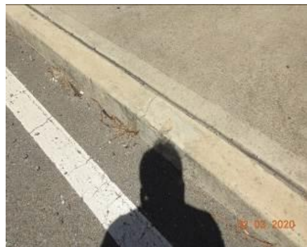
Figure 1509 – Crack propagation through kerb
