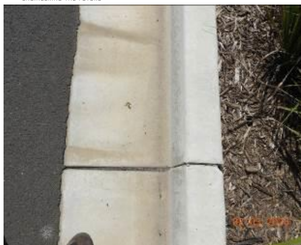
Figure 2033 – Crack propagation through kerb
