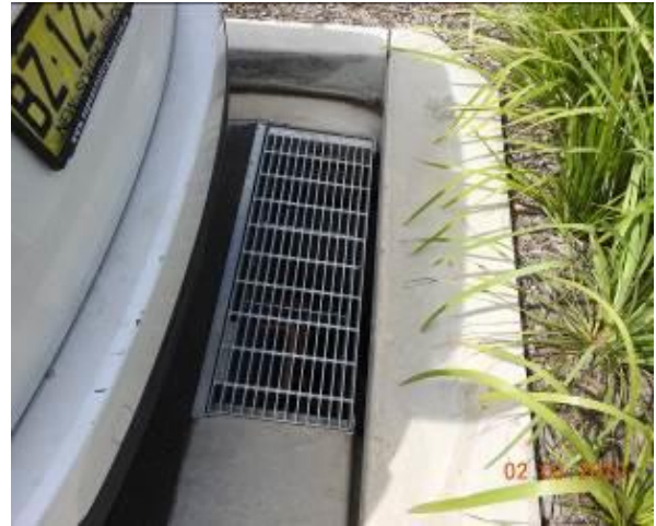
Figure 2501 – General Condition of stormwater inlet pit
