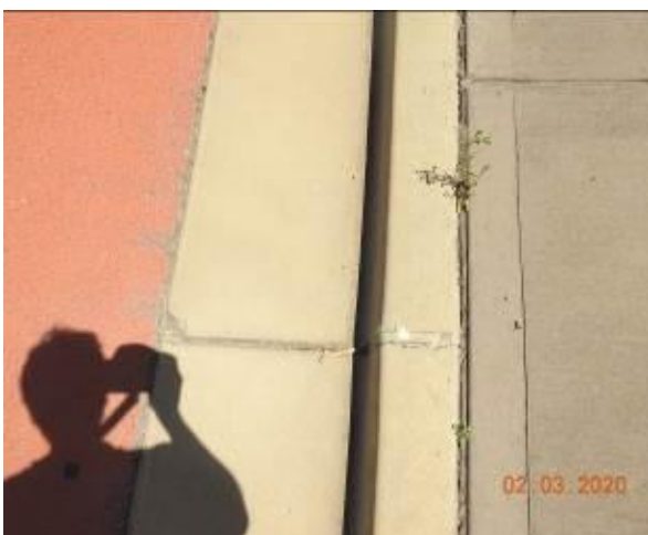
Figure 1658 – Crack propagation and loss of material through kerb and gutter
