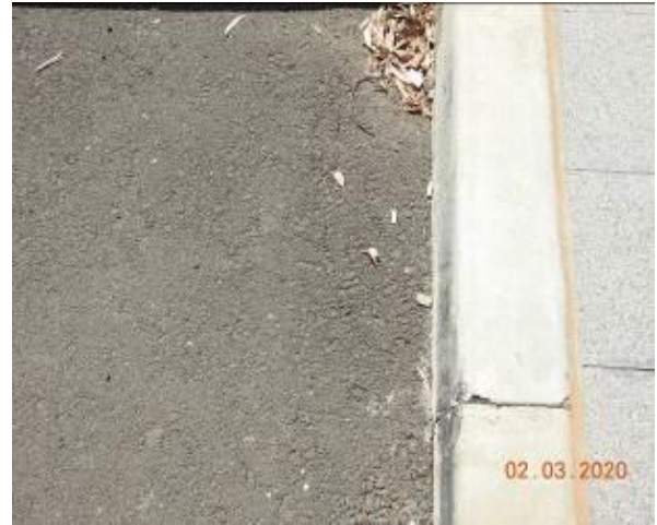
Figure 2148 – Crack propagation through kerb
