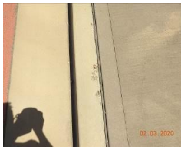
Figure 1677 – Loss of material through kerb
