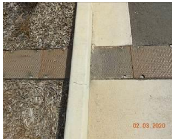
Figure 2785 – Crack propagation through kerb
