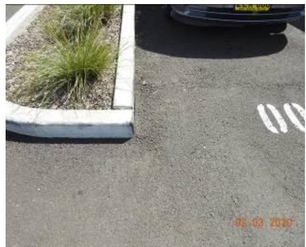
Figure 2919 – Loss of material through carpark pavement
