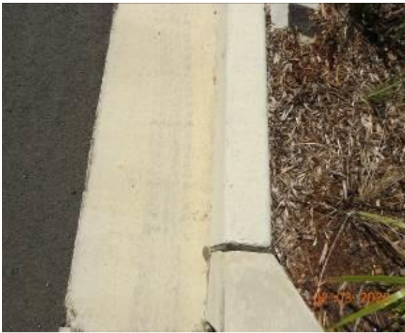
Figure 2185 – Crack propagation through kerb
