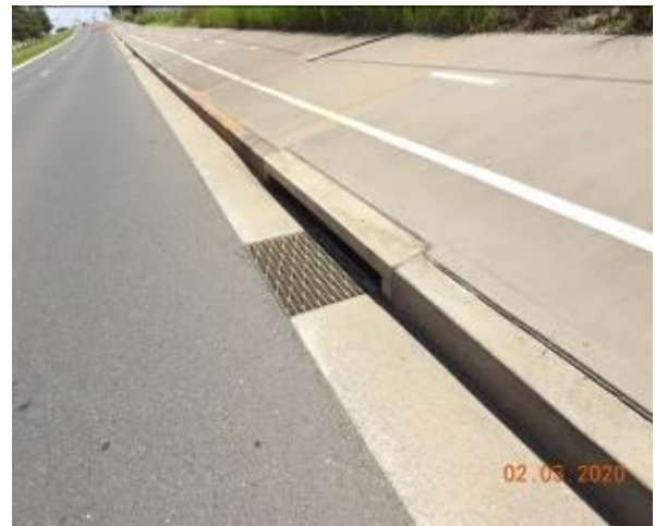
Figure 1591 – General Condition of stormwater inlet pit
