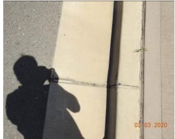
Figure 1589 – Crack propagation and loss of material through kerb and gutter
