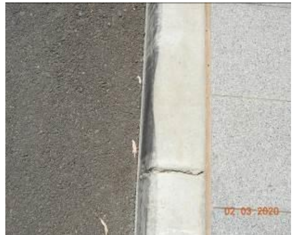
Figure 2144 – Crack propagation through kerb
