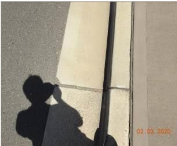
Figure 1584 – Loss of material through gutter
