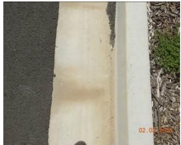
Figure 1988 – Crack propagation through kerb and gutter
