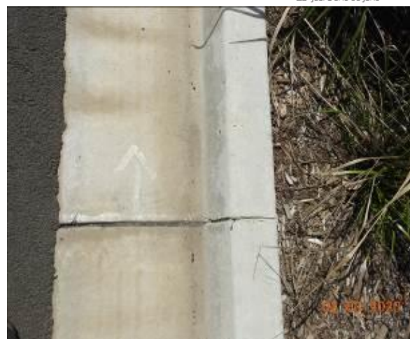
Figure 2034 – Crack propagation through kerb
