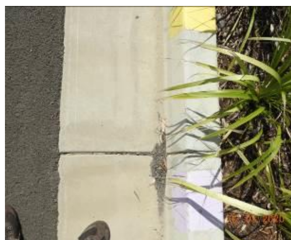
Figure 2056 – Crack propagation through kerb and gutter
