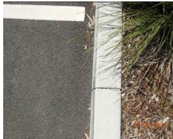
Figure 2066 – Crack propagation through kerb
