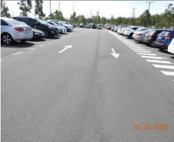
Figure 3048 – Loss of material through carpark pavement
