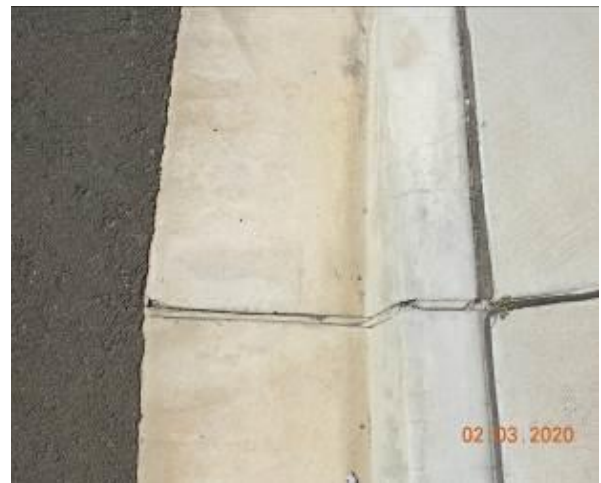
Figure 2048 – Loss of material through kerb and gutter
