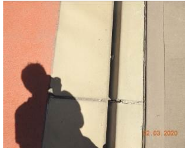
Figure 1673 – Crack propagation and loss of material through kerb and gutter
