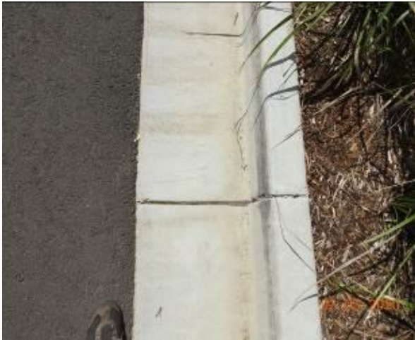
Figure 2171 – Crack propagation through kerb
