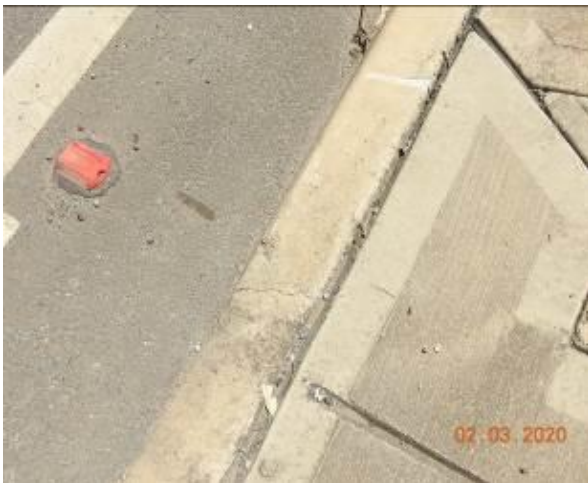
Figure 1524 – Crack propagation through layback
