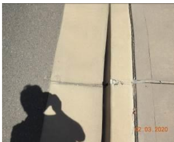
Figure 1604 – Loss of material through kerb and gutter
