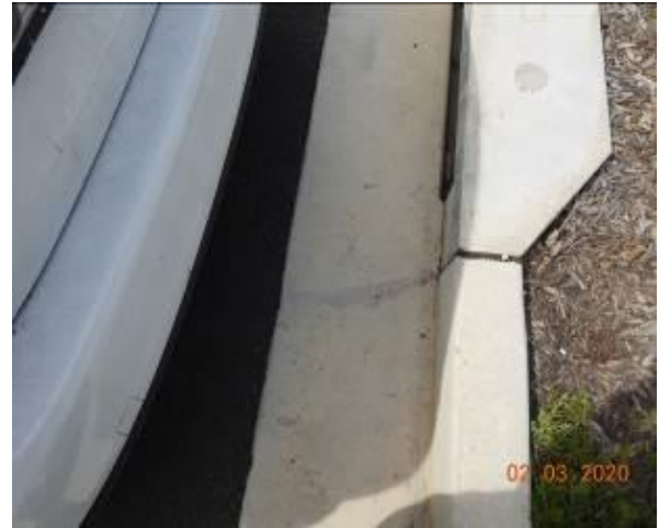
Figure 2489 – Crack propagation through gutter
