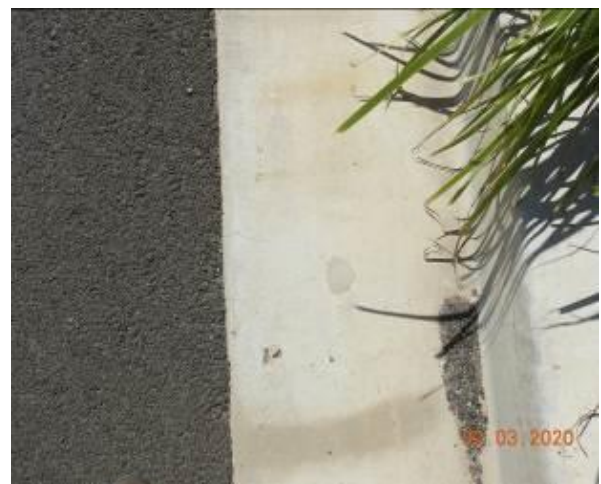
Figure 1966 – Crack propagation and Evidence of patchwork through gutter
