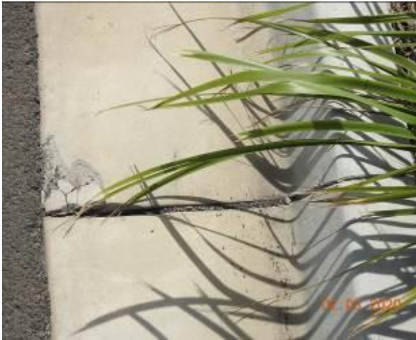
Figure 1955 – Crack propagation and loss of material through kerb and gutter
