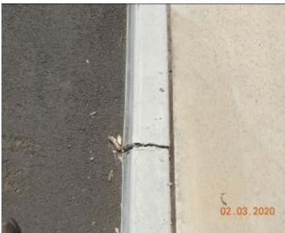
Figure 2019 – Loss of material through kerb
