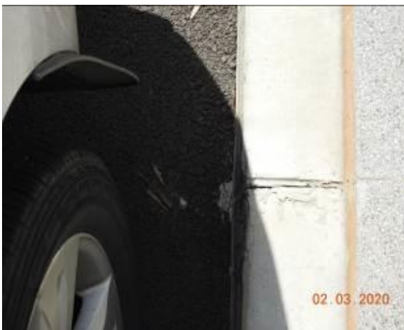
Figure 2091 – Crack propagation through kerb
