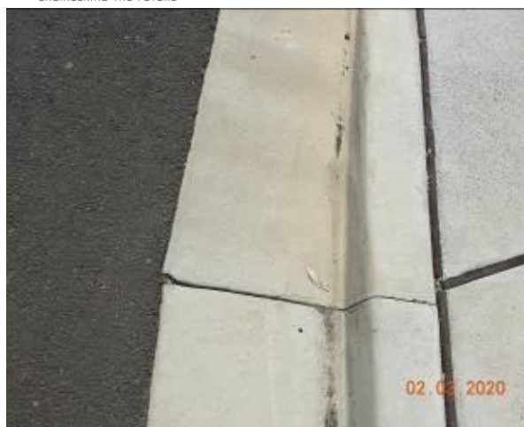
Figure 2051 – Loss of material through gutter
