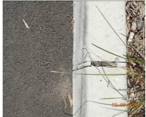
Figure 2088 – Crack propagation through kerb
