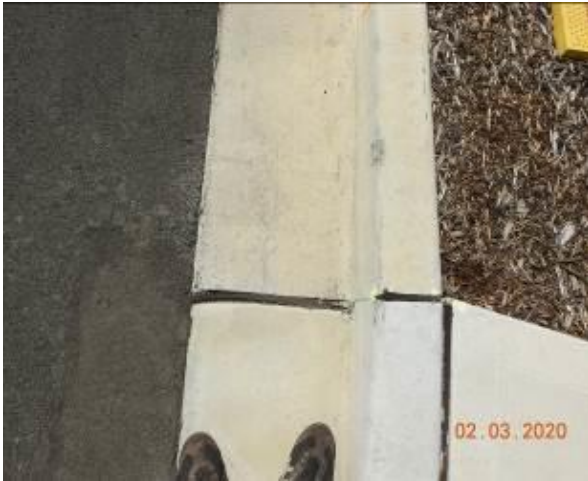
Figure 2183 – Crack propagation through kerb
