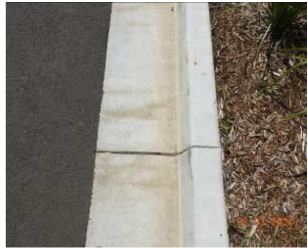
Figure 2180 – Crack propagation through kerb and gutter
