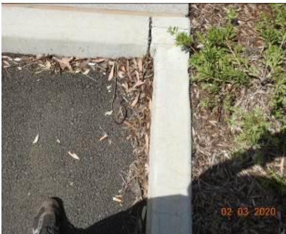
Figure 2061 – Crack propagation and Separation through kerb
