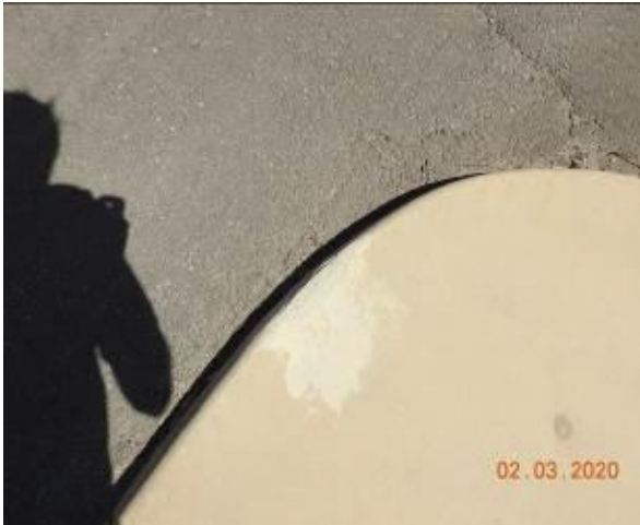
Figure 1546 – Loss of material through kerb
