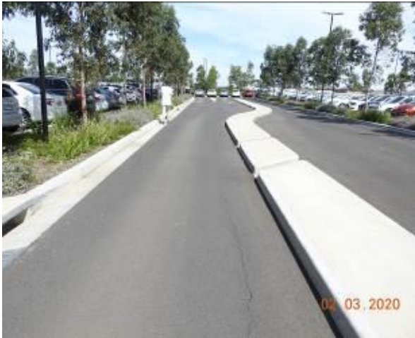
Figure 2886 – Crack propagation through carpark pavement
