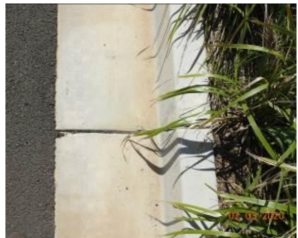
Figure 1990 – Loss of material through gutter
