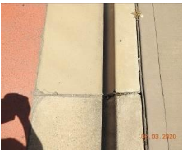
Figure 1682 – Crack propagation and loss of material through kerb and gutter
