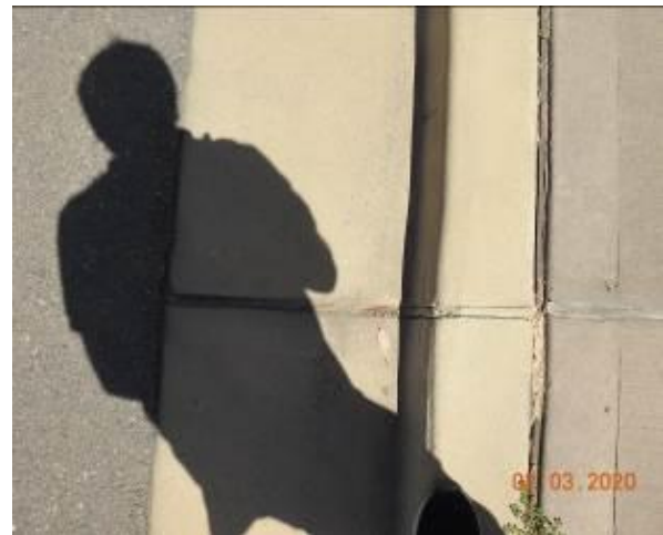
Figure 1561 – Crack propagation through kerb and gutter
