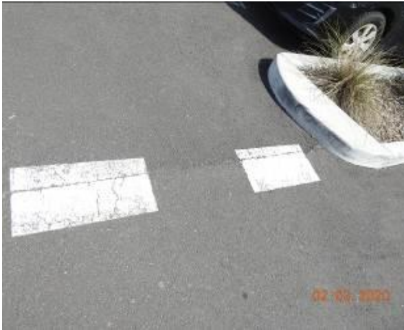
Figure 2952 – Crack propagation through carpark pavement
