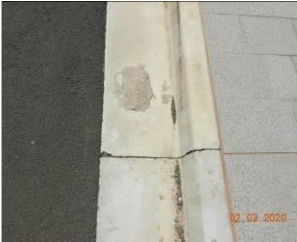
Figure 2165 – Crack propagation and loss of material through kerb and gutter
