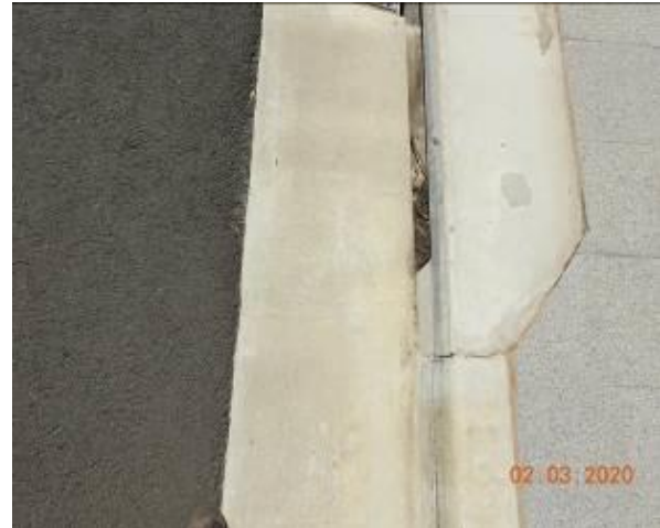
Figure 2166 – Crack propagation through kerb and gutter
