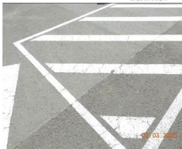
Figure 2745 – Crack propagation through carpark pavement
