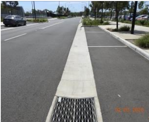
Figure 2023 – General Condition of gutter
