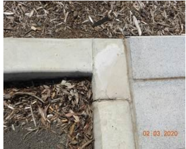
Figure 2112 – Crack propagation through kerb
