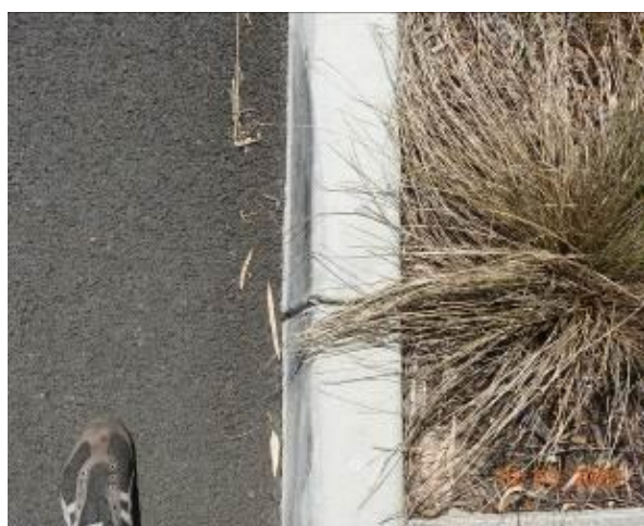
Figure 2071 – Loss of material through kerb
