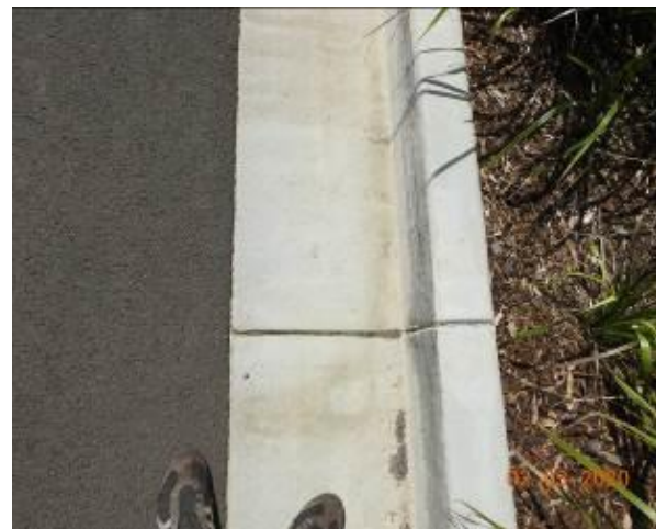
Figure 2170 – Crack propagation through kerb
