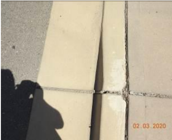
Figure 1624 – Loss of material through kerb
