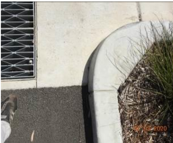
Figure 2077 – Crack propagation through kerb
