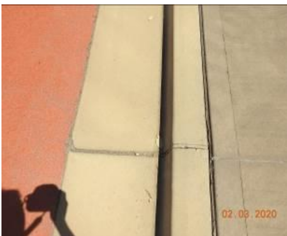
Figure 1676 – Crack propagation and loss of material through kerb and gutter
