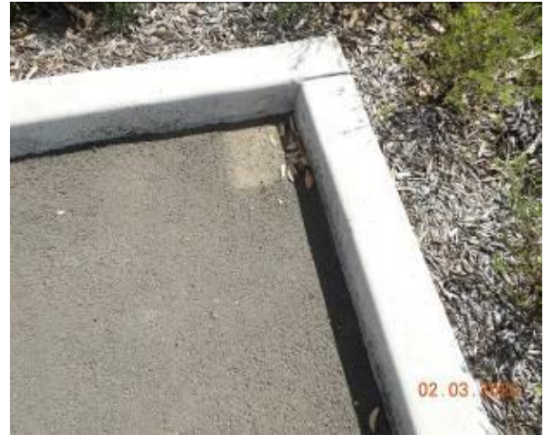
Figure 2757 – Loss of material through carpark pavement
