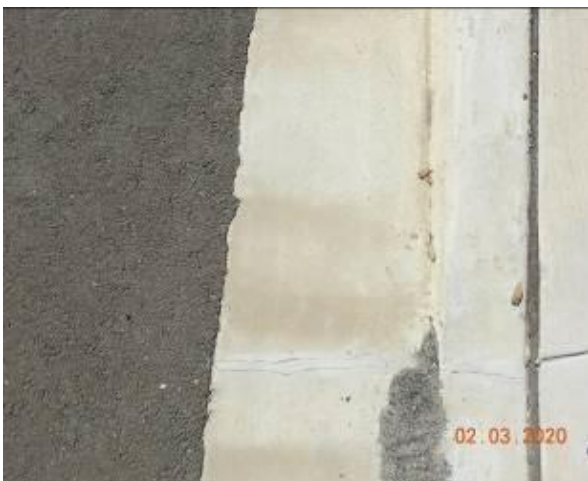
Figure 2043 – Evidence of patchwork through layback and gutter
