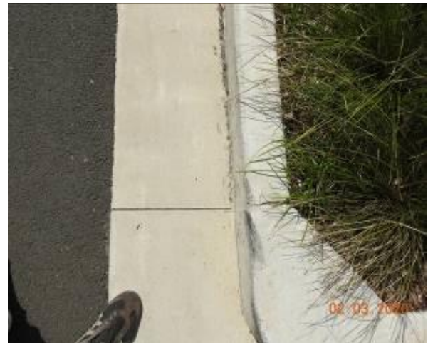
Figure 2096 – Crack propagation through kerb
