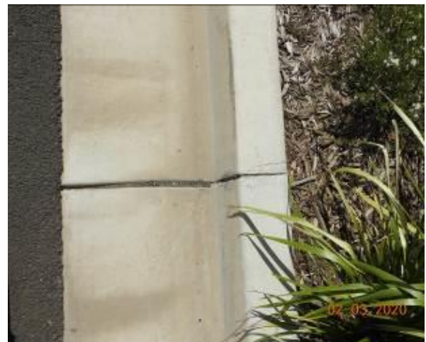
Figure 1978 – Crack propagation through kerb
