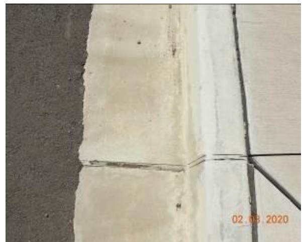
Figure 2044 – Loss of material through gutter
