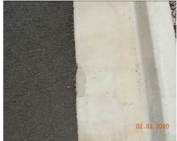
Figure 1962 – Evidence of patchwork through gutter
