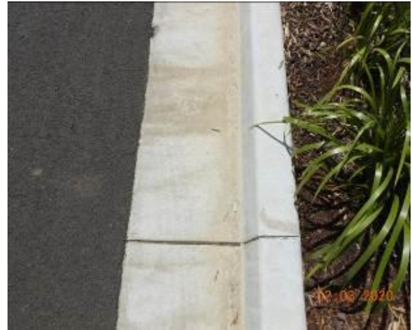
Figure 2178 – Crack propagation through kerb and gutter
