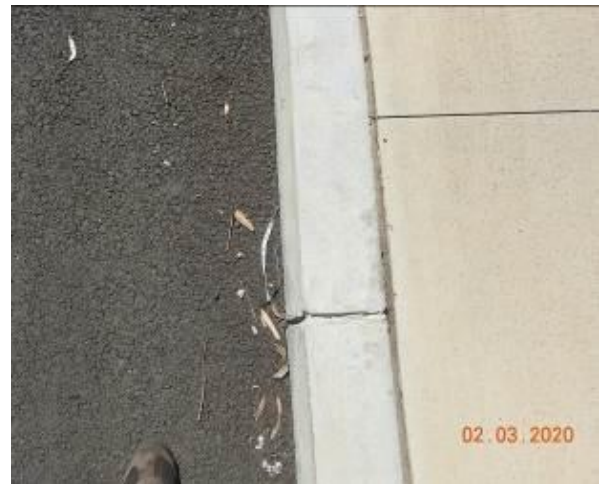
Figure 2012 – Loss of material through kerb
