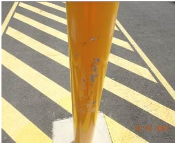
Figure 2442 – Physical damage traffic bollard
