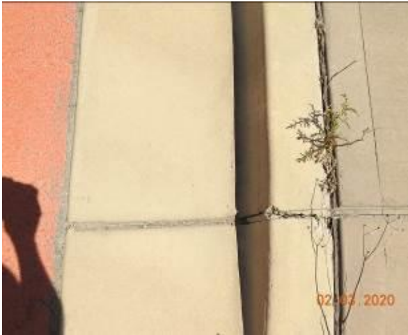
Figure 1690 – Crack propagation and loss of material through kerb
