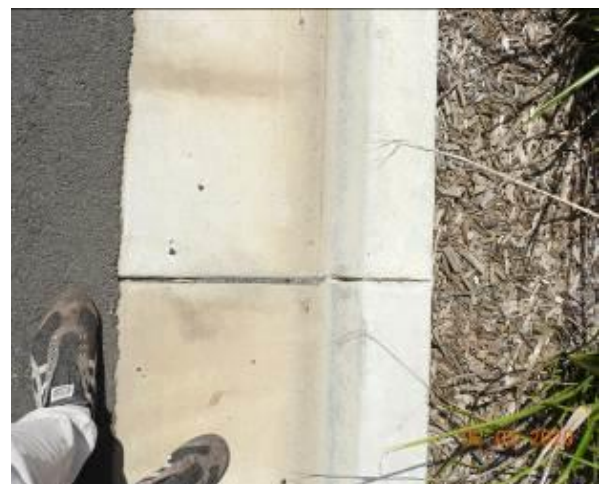
Figure 2032 – Crack propagation through kerb
