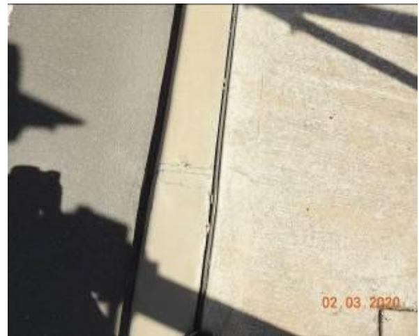
Figure 1543 – Crack propagation through kerb
