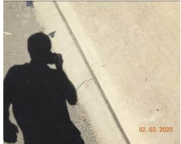
Figure 1535 – Crack propagation through kerb
