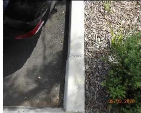
Figure 2507 – Crack propagation and loss of material through kerb
