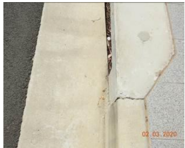
Figure 2158 – Crack propagation through kerb
