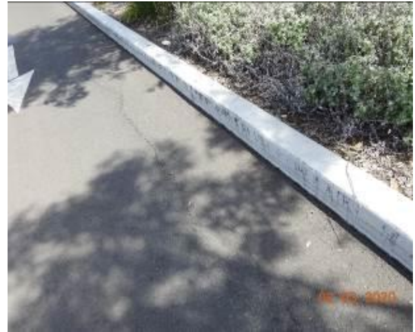
Figure 2875 – Crack propagation through carpark pavement
