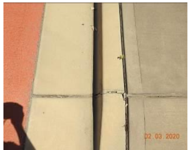
Figure 1701 – Crack propagation through kerb and gutter
