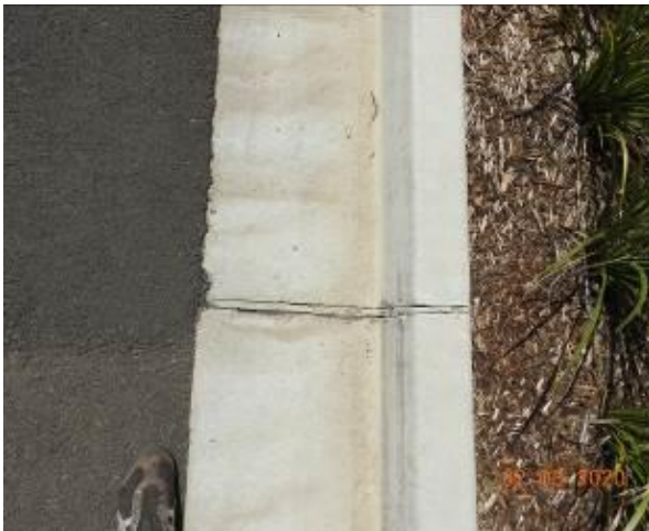
Figure 2173 – Crack propagation through kerb and gutter
