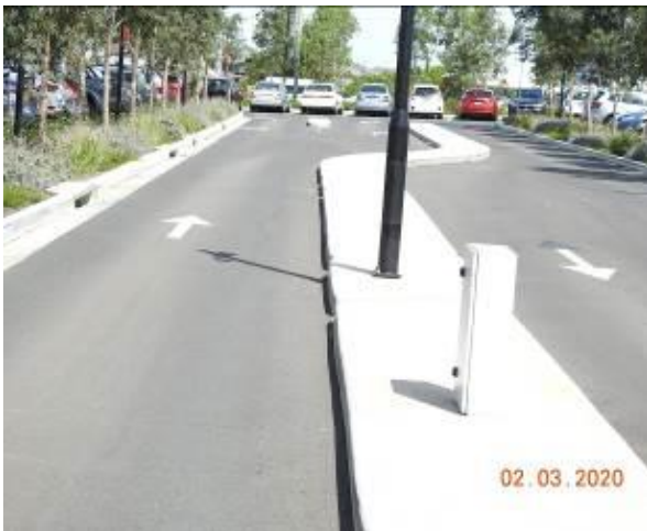
Figure 3074 – General Condition of traffic island kerb
