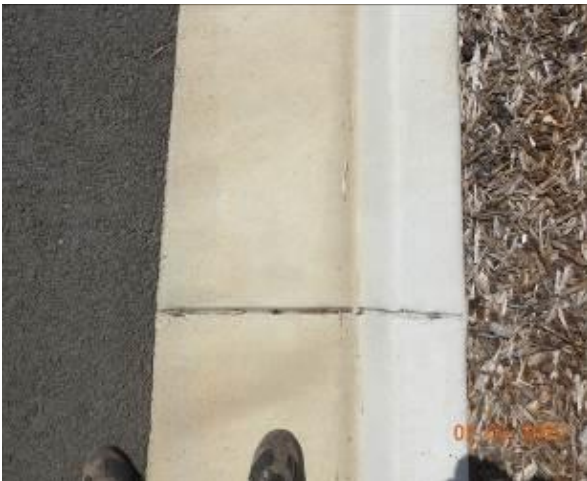
Figure 2191 – Crack propagation through kerb and gutter
