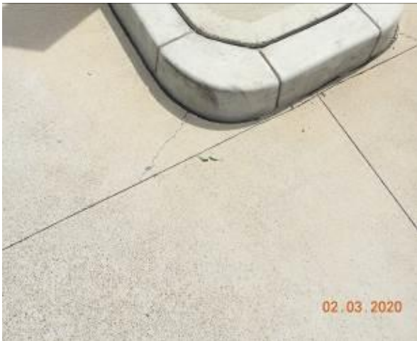
Figure 2518 – Crack propagation through driveway pavement
