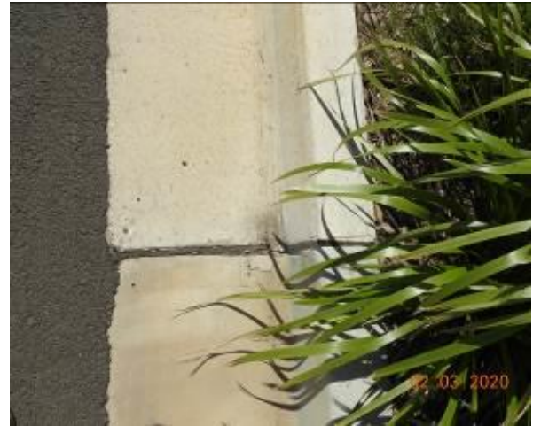
Figure 1992 – Loss of material through gutter
