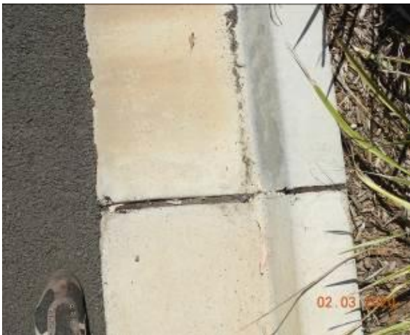
Figure 1995 – Loss of material through kerb and gutter
