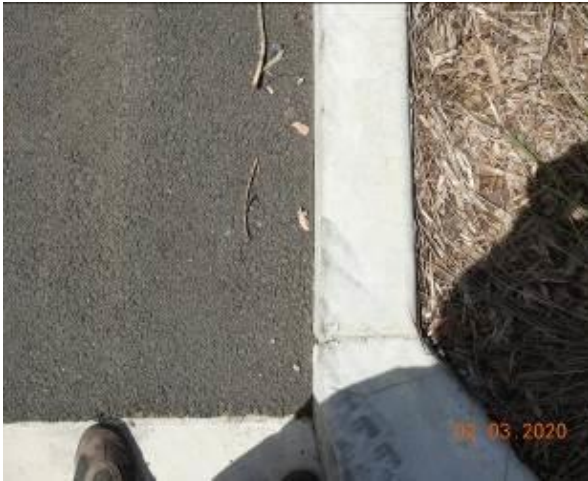
Figure 2081 – Loss of material through kerb
