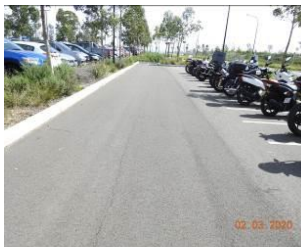
Figure 2749 – Crack propagation through carpark pavement
