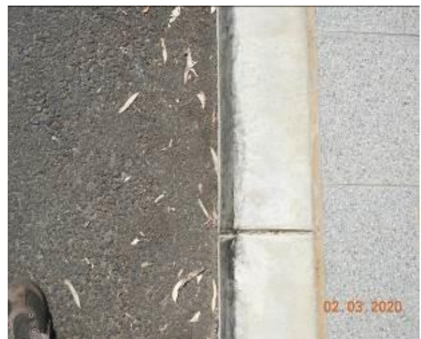
Figure 2140 – Crack propagation through kerb
