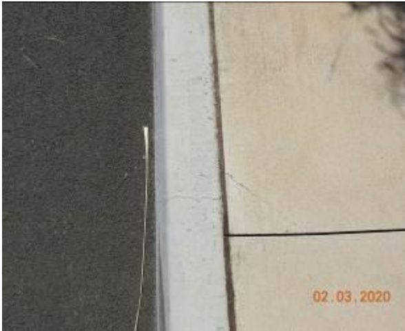
Figure 2009 – Crack propagation through kerb
