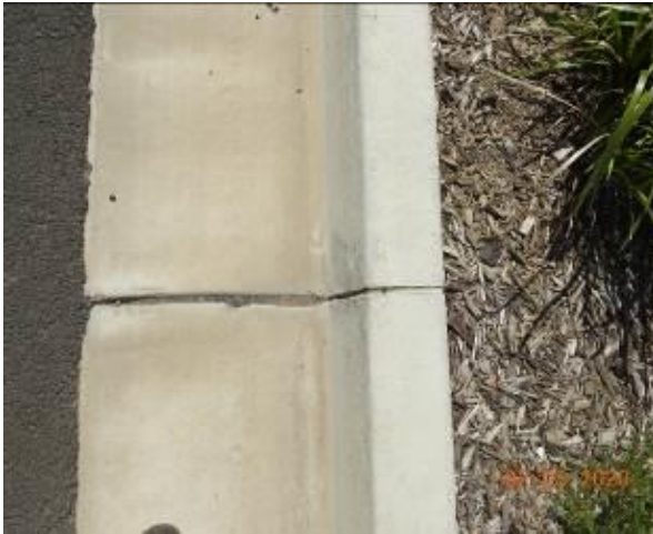
Figure 1979 – Loss of material through kerb and gutter
