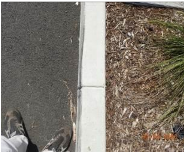
Figure 2107 – Crack propagation through kerb
