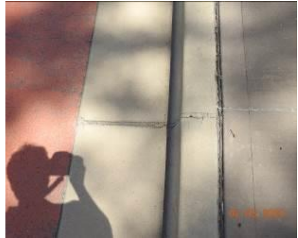
Figure 1661 – Crack propagation and loss of material through kerb and gutter
