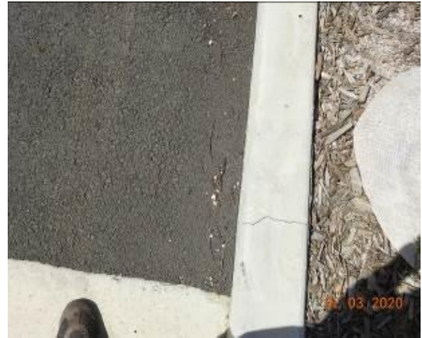
Figure 2004 – Crack propagation through curb
