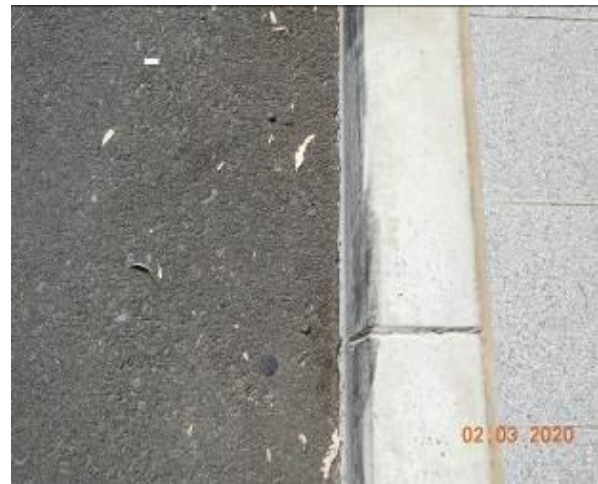
Figure 2132 – Crack propagation through kerb
