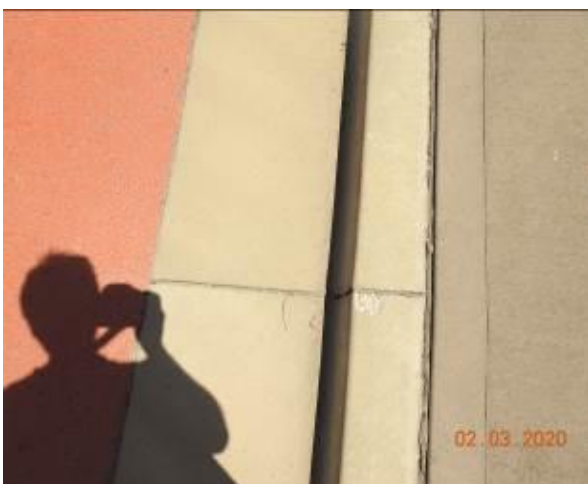
Figure 1664 – Loss of material through kerb
