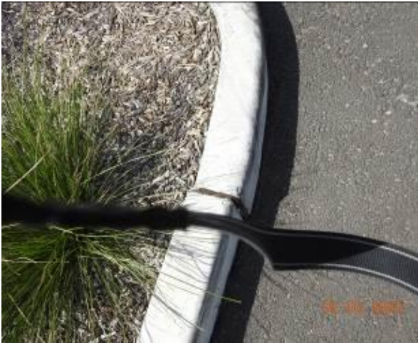
Figure 3120 – Displacement through kerb
