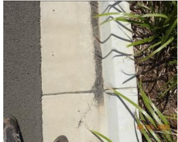
Figure 2058 – Crack propagation through kerb and gutter
