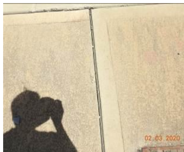
Figure 1489 – Crack propagation through footpath pavement
