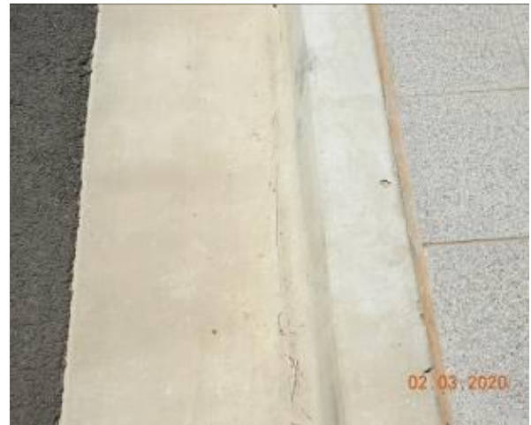
Figure 2156 – Crack propagation through kerb
