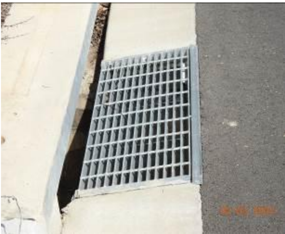
Figure 3080 – Crack propagation through stormwater inlet pit
