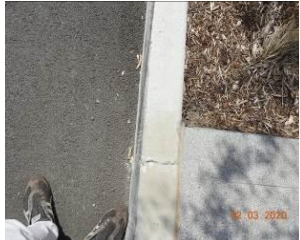
Figure 2106 – Crack propagation through kerb
