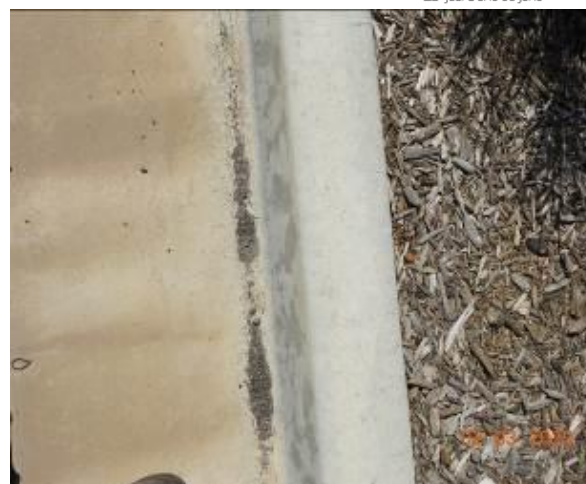
Figure 1998 – Crack propagation through kerb and gutter
