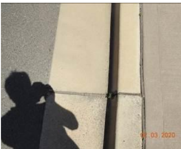
Figure 1610 – Crack propagation and loss of material through kerb and gutter
