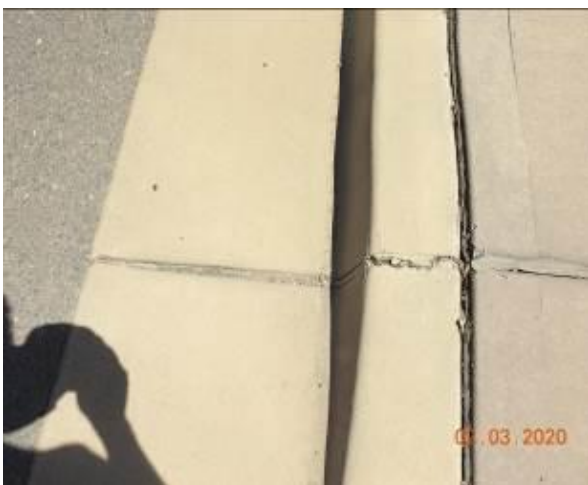
Figure 1626 – Crack propagation through kerb
