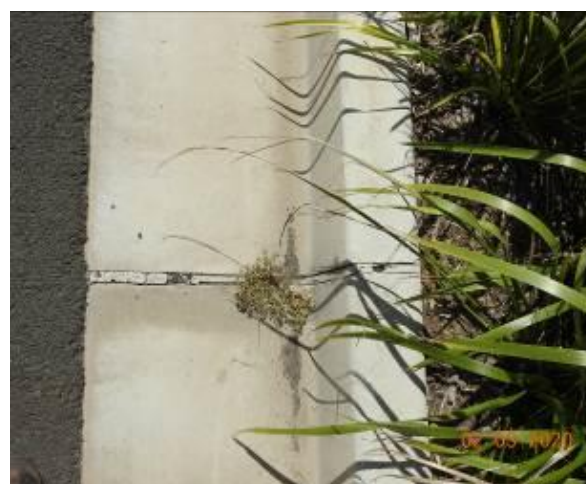
Figure 1970 – Crack propagation through kerb and gutter
