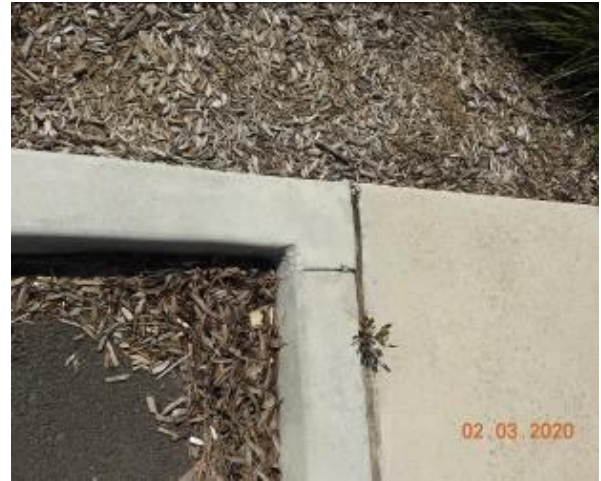
Figure 2028 – Crack propagation through kerb
