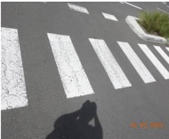
Figure 2650 – Crack propagation through carpark pavement
