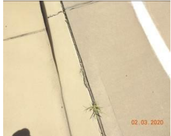
Figure 1625 – Loss of material through layback
