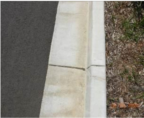
Figure 2179 – Crack propagation through kerb
