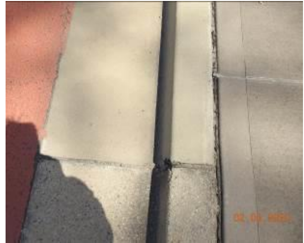
Figure 1643 – Loss of material through kerb
