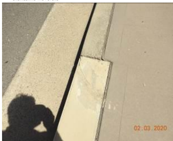
Figure 1600 – Crack propagation through stormwater inlet pit
