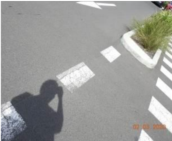
Figure 2656 – Crack propagation through carpark pavement
