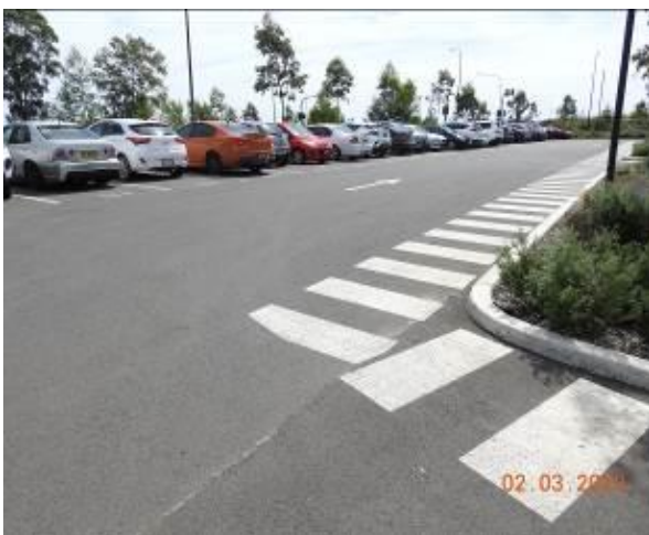
Figure 2620 – Crack propagation through carpark pavement
