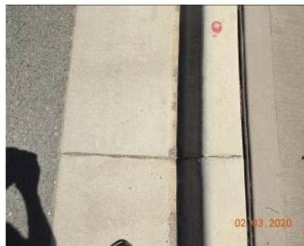
Figure 1503 – Crack propagation through kerb
