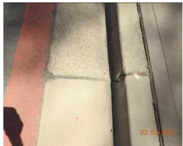
Figure 1641 – Loss of material through kerb and gutter
