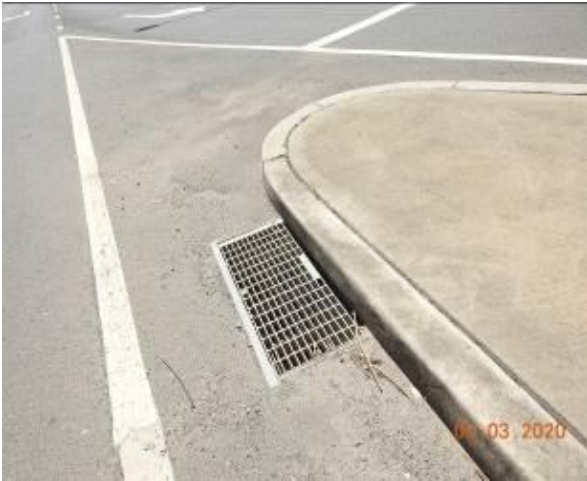
Figure 1528 – General Condition of stormwater inlet pit
