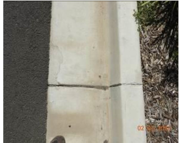
Figure 1974 – Crack propagation through kerb and gutter
