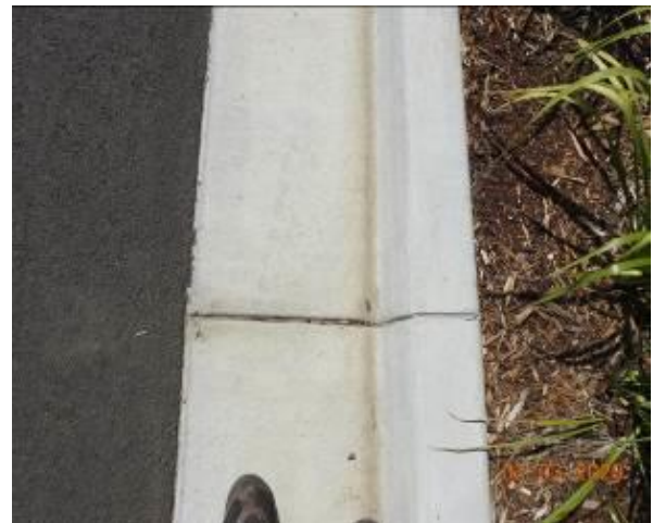
Figure 2188 – Crack propagation through kerb and gutter
