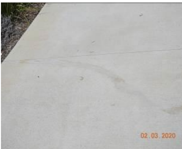
Figure 1941 – Crack propagation through footpath pavement
