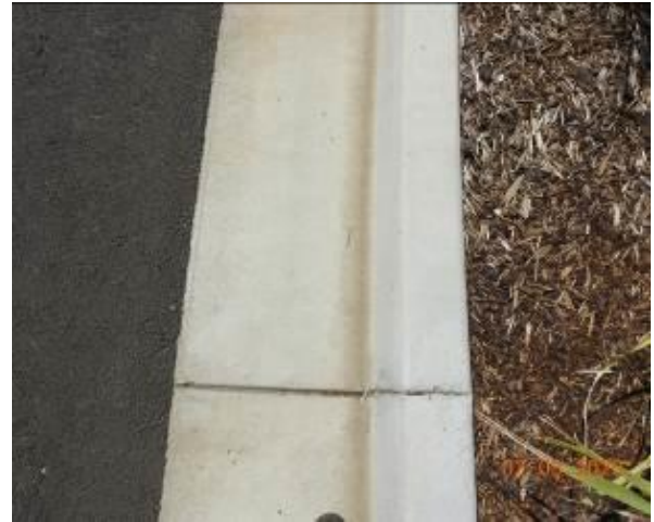
Figure 2190 – Crack propagation through kerb and gutter
