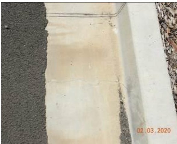
Figure 1989 – Crack propagation through kerb and gutter
