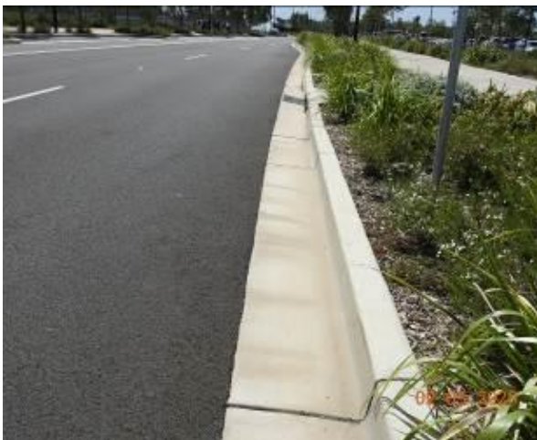
Figure 1977 – General Condition of kerb and gutter
