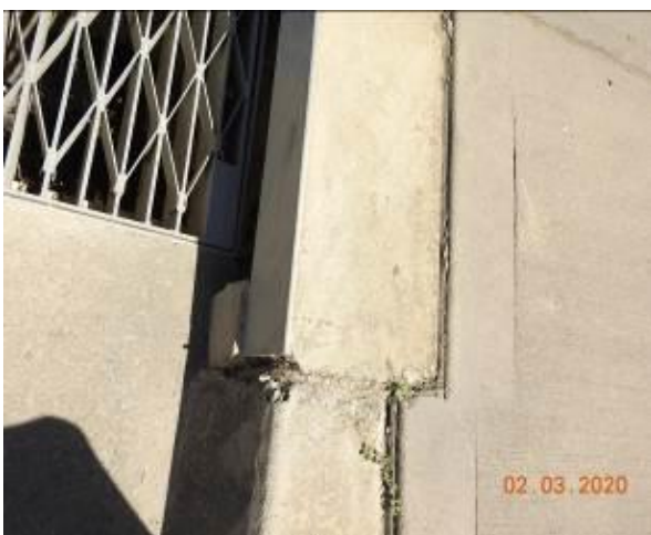
Figure 1574 – Loss of material through stormwater inlet pit
