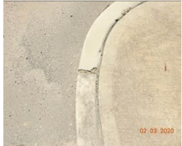
Figure 1529 – Loss of material through kerb
