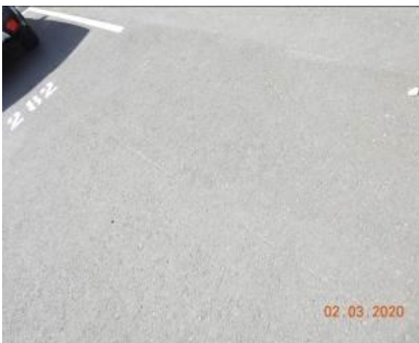
Figure 3058 – Loss of material through carpark pavement
