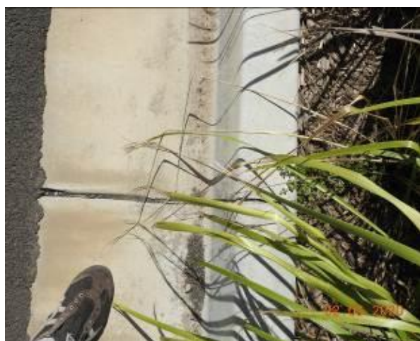
Figure 2001 – Crack propagation through kerb and gutter
