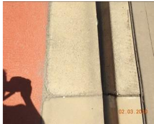
Figure 1693 – Crack propagation and loss of material through gutter
