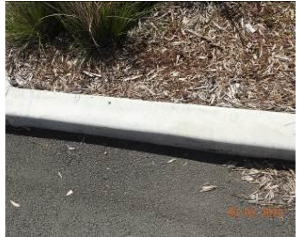
Figure 2076 – Crack propagation through kerb
