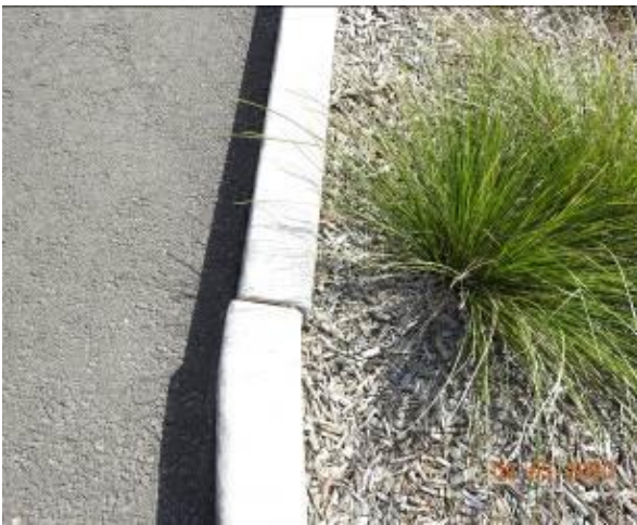
Figure 3122 – Displacement through kerb
