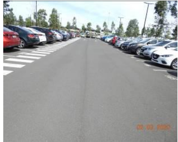
Figure 2959 – Crack propagation through carpark pavement
