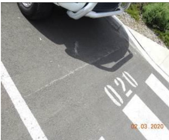
Figure 2566 – Crack propagation through carpark pavement
