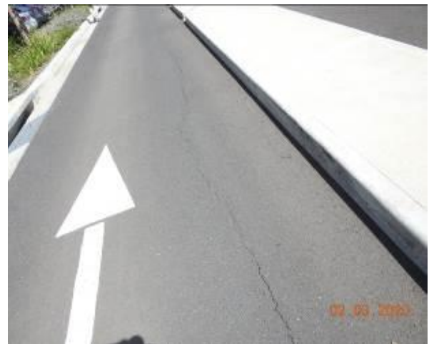
Figure 2885 – Crack propagation through carpark pavement
