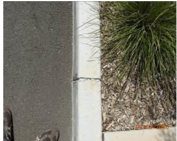
Figure 2024 – Crack propagation through kerb
