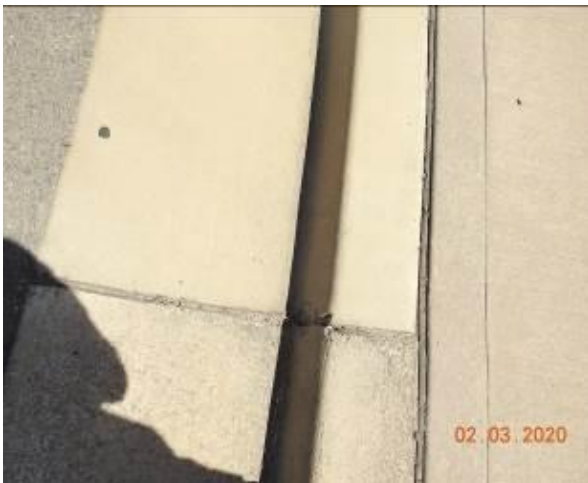
Figure 1620 – Loss of material through kerb
