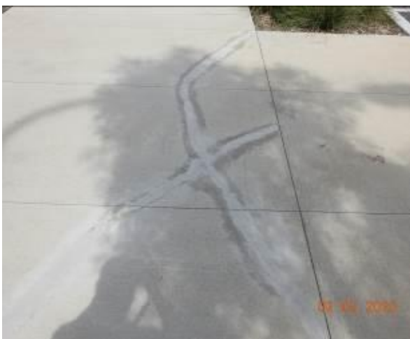
Figure 1929 – Crack propagation through footpath pavement
