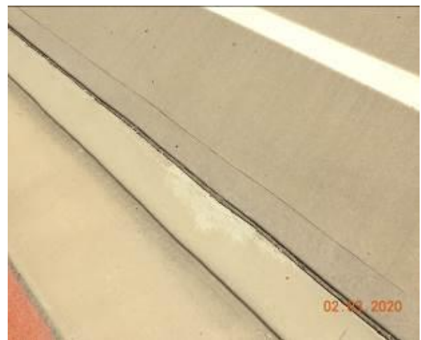
Figure 1699 – Loss of material through layback
