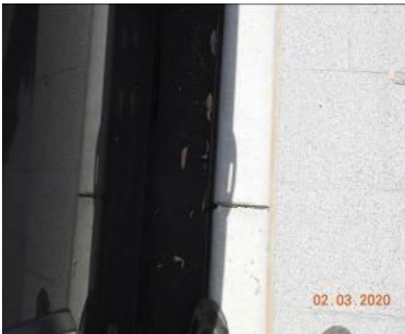
Figure 2065 – Crack propagation through kerb
