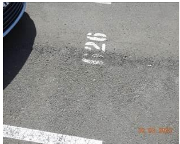
Figure 2939 – Loss of material through carpark pavement
