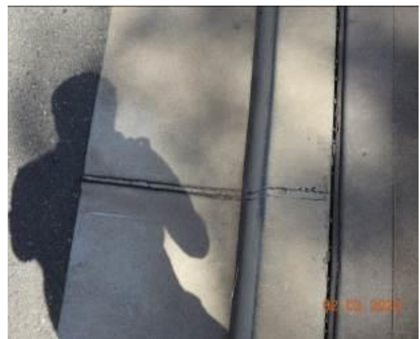
Figure 1579 – Crack propagation through kerb and gutter
