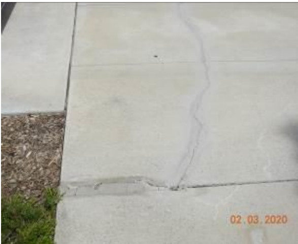
Figure 1933 – Crack propagation and loss of material through footpath pavement
