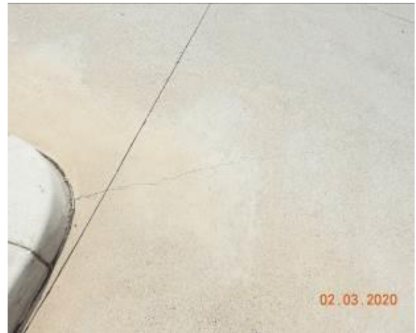
Figure 2519 – Crack propagation through driveway pavement
