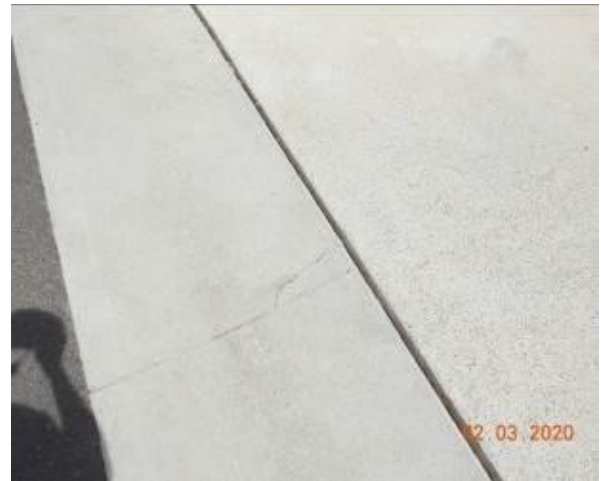
Figure 2513 – Crack propagation through layback and gutter
