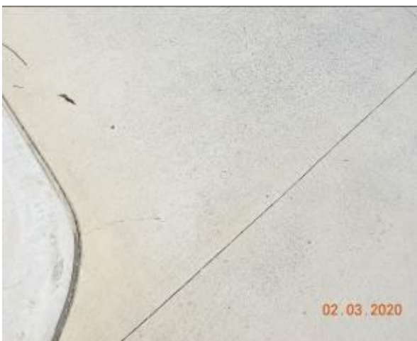
Figure 2860 – Crack propagation through driveway pavement
