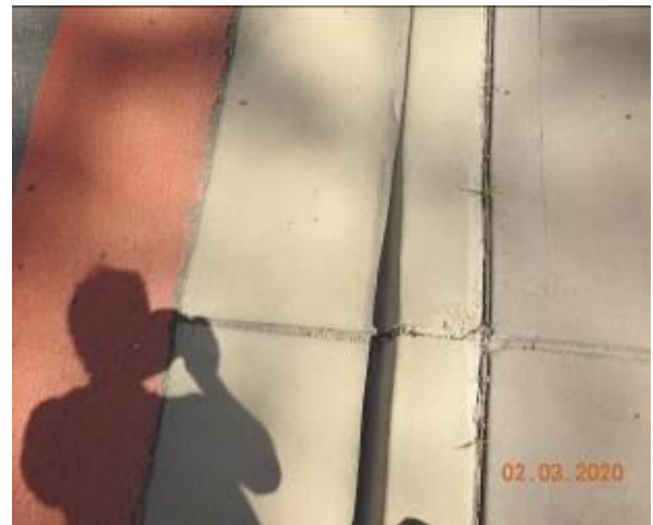
Figure 1645 – Loss of material through kerb
