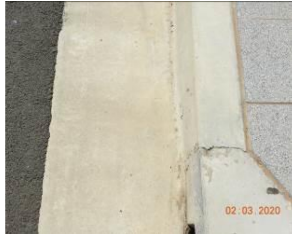
Figure 2160 – Crack propagation through kerb
