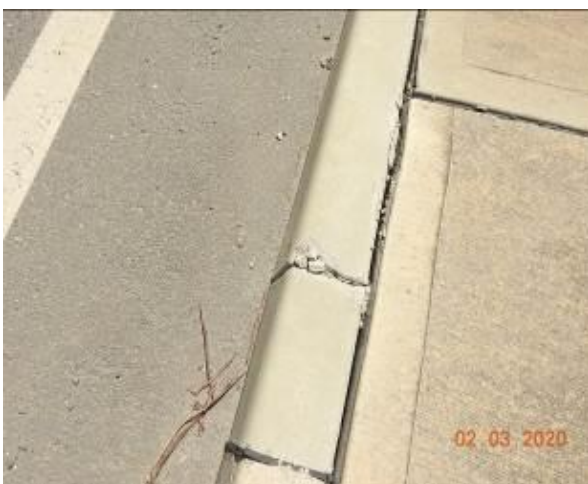
Figure 1526 – Crack propagation and loss of material through kerb
