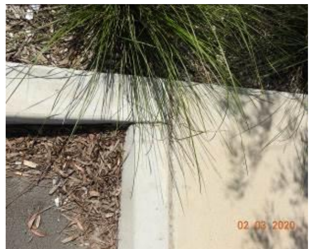
Figure 2014 – Crack propagation through kerb
