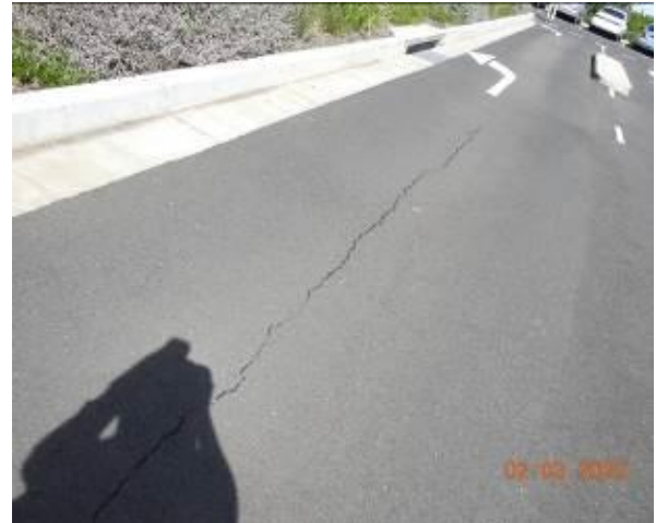
Figure 2899 – Crack propagation through carpark pavement
