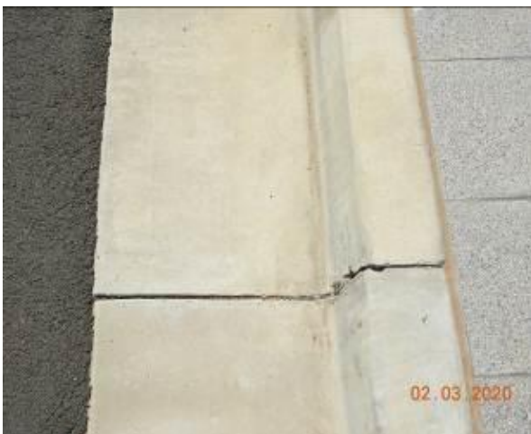
Figure 2157 – Loss of material through kerb and gutter
