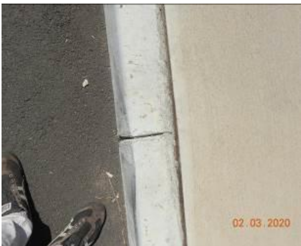
Figure 2025 – Crack propagation through kerb
