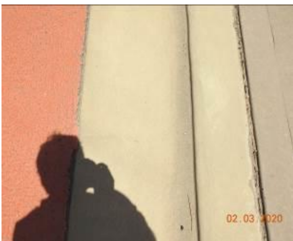
Figure 1646 – Crack propagation through layback and gutter
