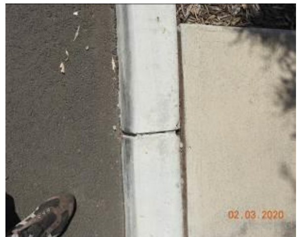
Figure 2026 – Crack propagation through kerb
