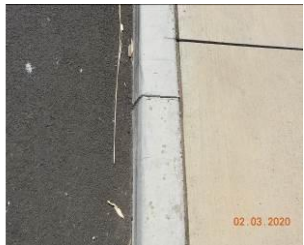
Figure 2008 – Crack propagation through curb
