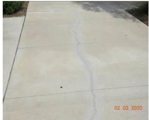
Figure 1934 – Crack propagation through footpath pavement
