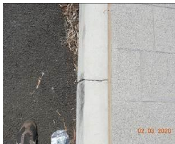
Figure 2072 – Crack propagation through kerb
