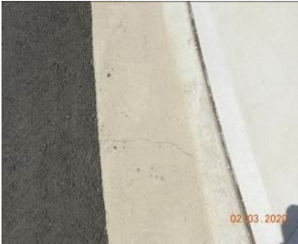
Figure 2195 – Crack propagation through layback and gutter
