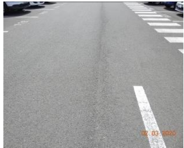
Figure 2377 – Loss of material through carpark pavement
