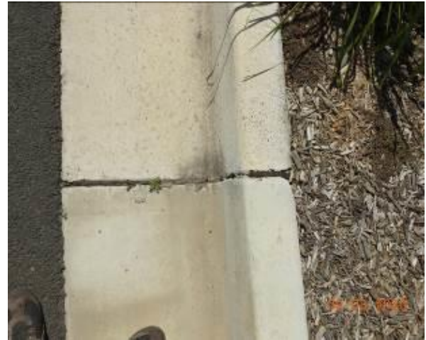
Figure 1980 – Loss of material through kerb and gutter
