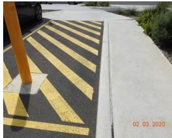
Figure 2467 – Crack propagation through footpath pavement
