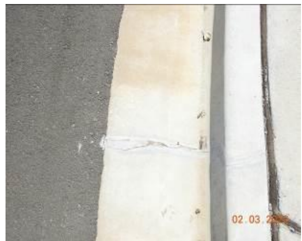
Figure 2050 – Crack propagation through kerb and gutter
