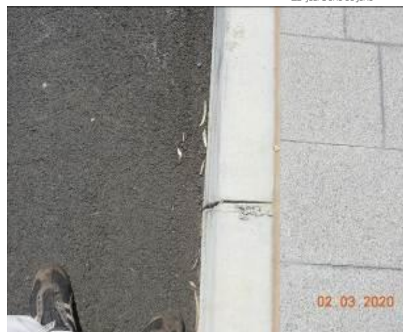
Figure 2070 – Crack propagation and loss of material through kerb
