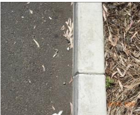
Figure 2139 – Crack propagation through kerb
