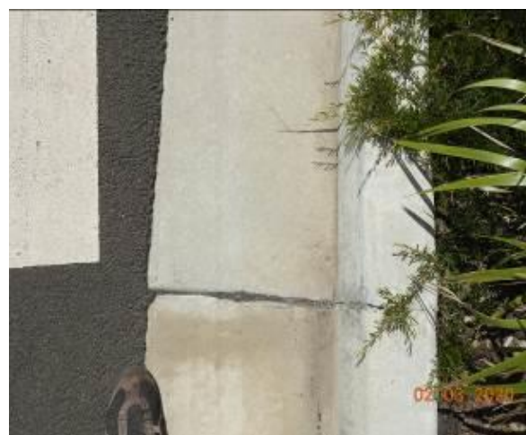
Figure 2036 – Crack propagation and loss of material through kerb and gutter
