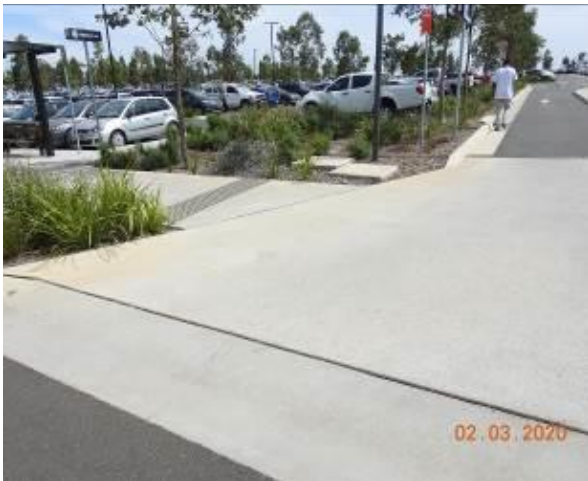
Figure 2512 – Crack propagation through layback and gutter
