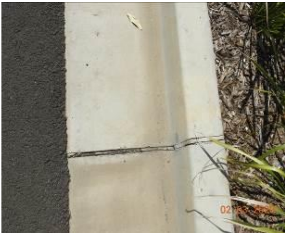
Figure 1975 – Crack propagation through kerb and gutter
