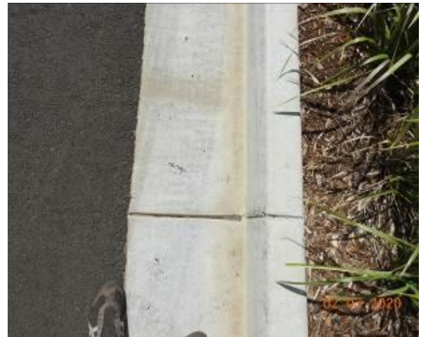
Figure 2174 – Crack propagation through kerb and gutter
