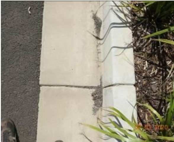
Figure 2057 – Crack propagation through kerb and gutter
