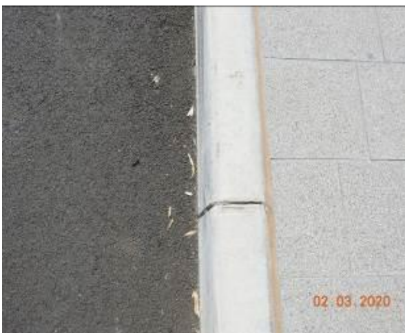
Figure 2067 – Crack propagation through kerb
