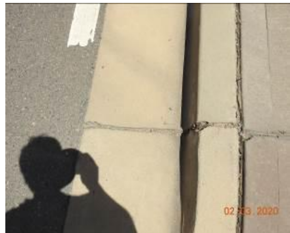
Figure 1635 – Loss of material through kerb
