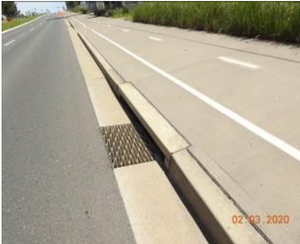
Figure 1618 – General Condition of stormwater inlet pit
