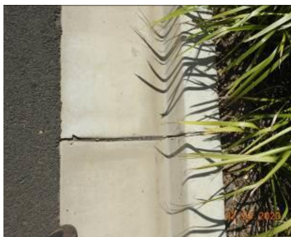
Figure 1971 – Loss of material through gutter
