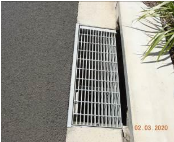
Figure 1981 – General Condition of stormwater inlet pit
