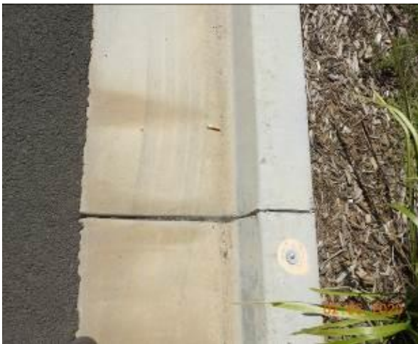
Figure 1987 – Crack propagation and loss of material through kerb
