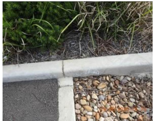
Figure 1232 – Hairline cracking through car park kerb
