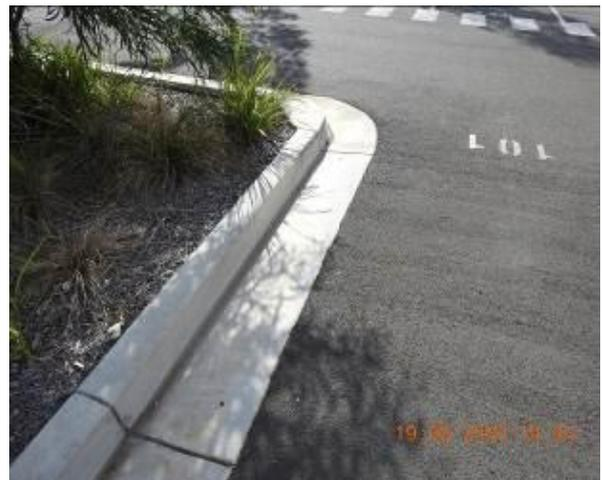
Figure 1262 – Crack propagation through car park kerb
