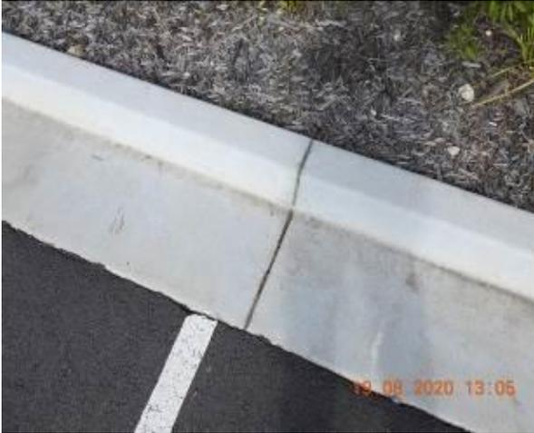
Figure 2271 – Crack propagation through car park kerb
