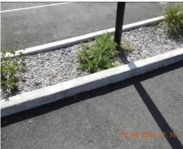
Figure 1735 – Crack propagation through car park kerb
