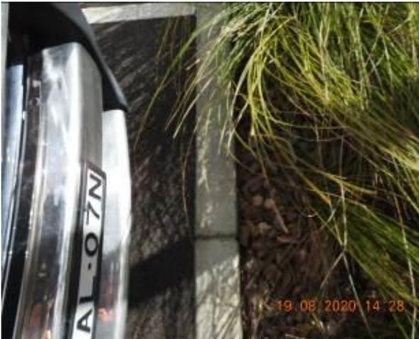
Figure 1213 – Crack propagation through car park kerb
