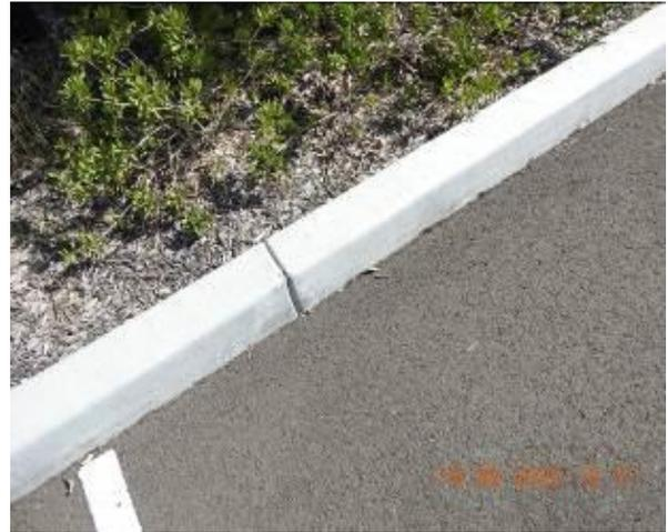
Figure 1744 – Crack propagation through car park kerb
