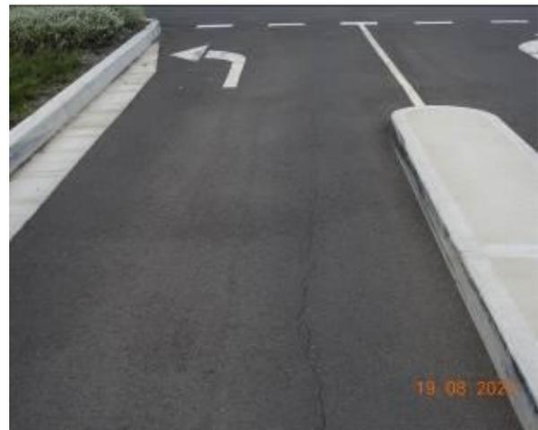
Figure 1412 – Crack propagation through car park pavement
