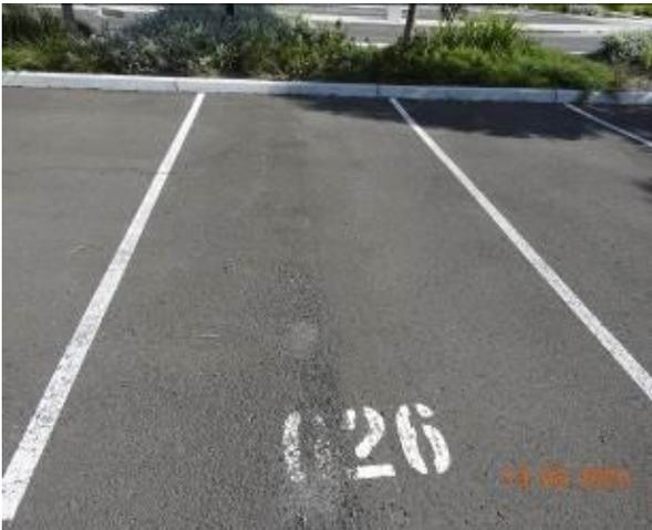
Figure 1457 – Loss of material through car park pavement
