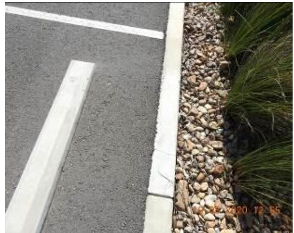
Figure 2136 – Crack propagation through car park kerb
