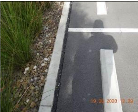
Figure 1861 – Crack propagation through car park kerb
