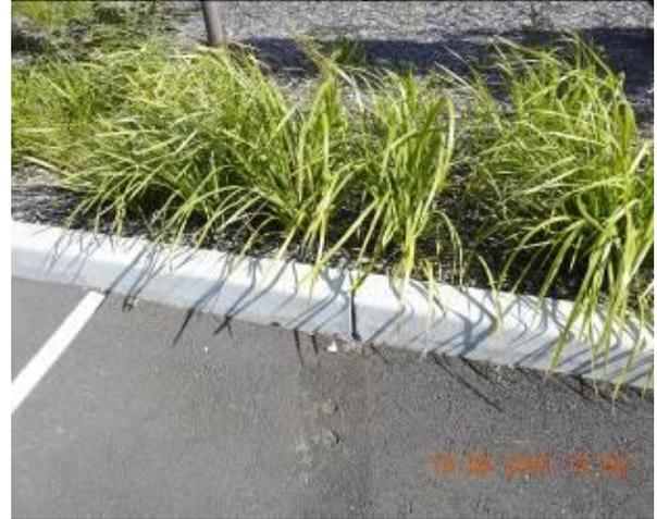
Figure 2164 – Crack propagation through car park kerb
