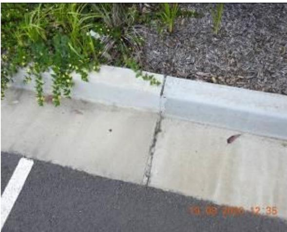
Figure 1921 – Crack propagation through car park kerb and gutter
