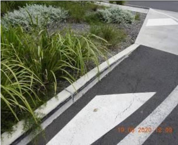
Figure 1701 – Crack propagation through car park kerb
