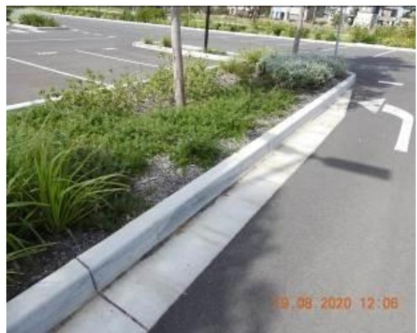
Figure 1670 – Crack propagation through car park kerb
