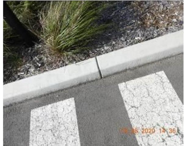
Figure 1306 – Crack propagation through car park kerb
