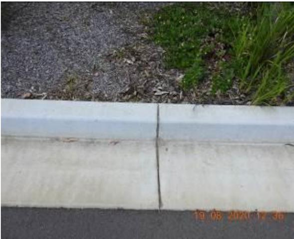
Figure 1925 – Crack propagation through car park kerb
