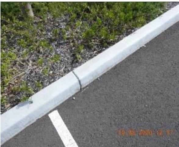
Figure 1741 – Crack propagation through car park kerb
