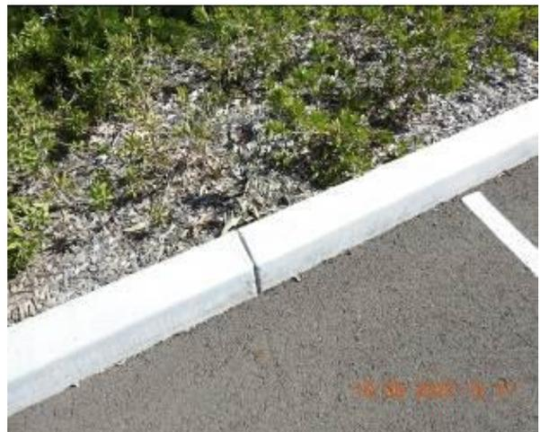
Figure 1754 – Crack propagation through car park kerb
