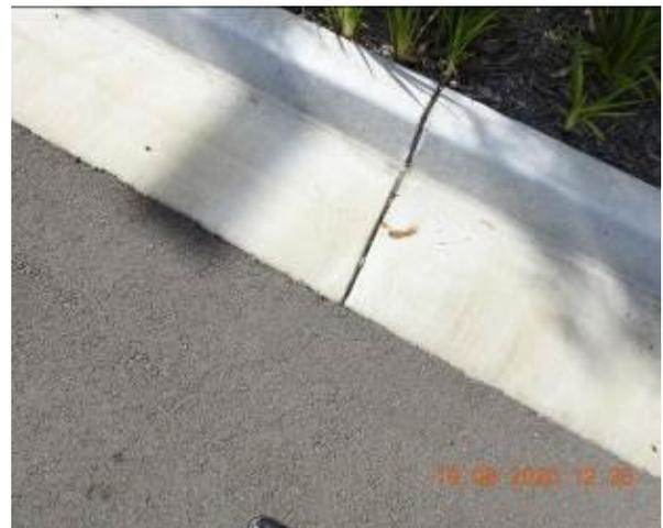
Figure 1934 – Crack propagation through car park kerb
