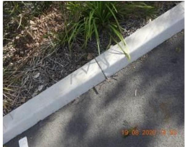
Figure 1284 – Crack propagation through car park kerb
