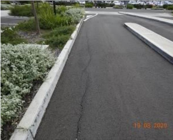
Figure 1425 – Crack propagation through car park pavement
