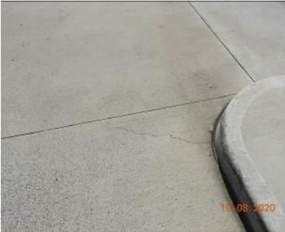
Figure 1431 – Crack propagation through car park pavement
