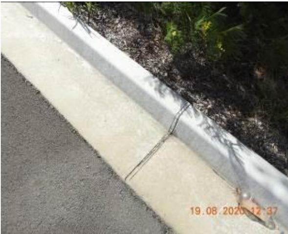
Figure 1943 – Crack propagation through car park gutter
