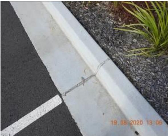
Figure 2273 – Crack propagation through car park kerb
