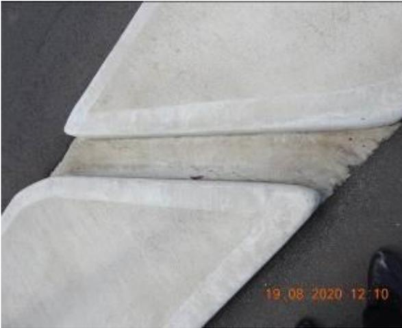
Figure 1713 – Crack propagation through traffic island
