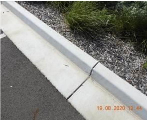
Figure 2009 – Crack propagation through car park kerb and gutter
