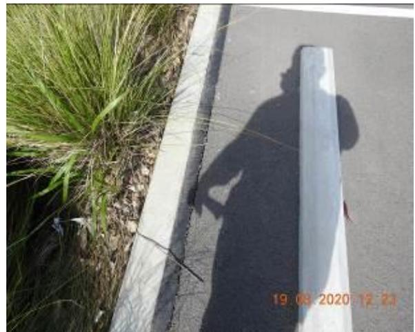
Figure 1800 – Crack propagation through car park kerb
