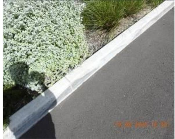
Figure 1876 – Crack propagation through car park kerb
