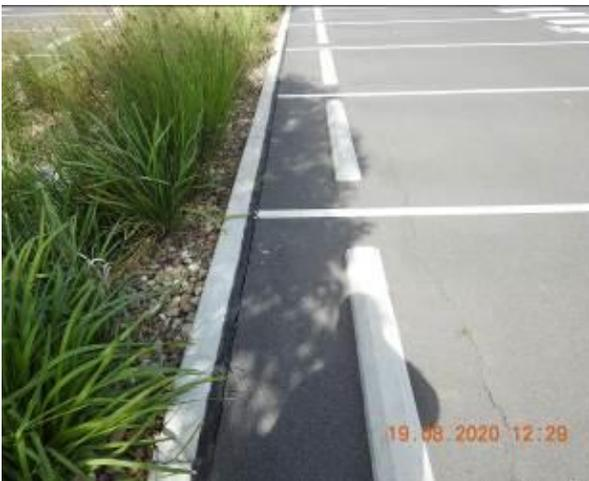
Figure 1859 – Crack propagation through car park kerb
