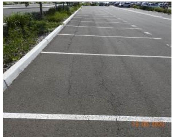
Figure 1442 – Crack propagation through car park pavement
