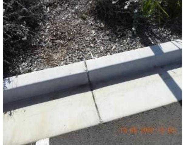
Figure 2218 – Crack propagation through car park kerb
