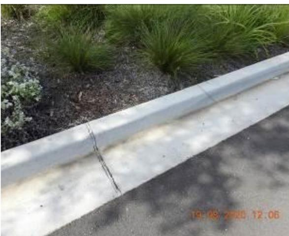
Figure 1669 – Crack propagation and loss of material through car park kerb and gutter
