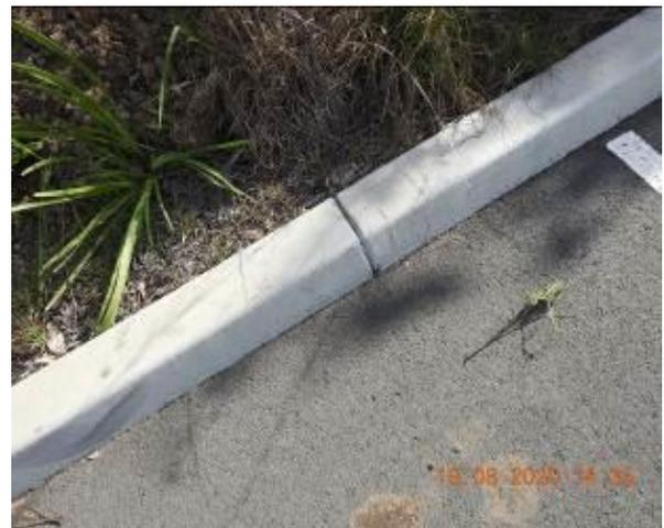
Figure 1280 – Crack propagation through car park kerb
