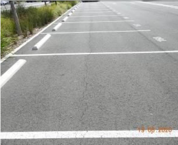
Figure 1515 – Crack propagation through car park pavement
