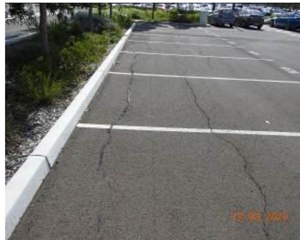
Figure 1454 – Crack propagation and evidence of patchwork through car park pavement
