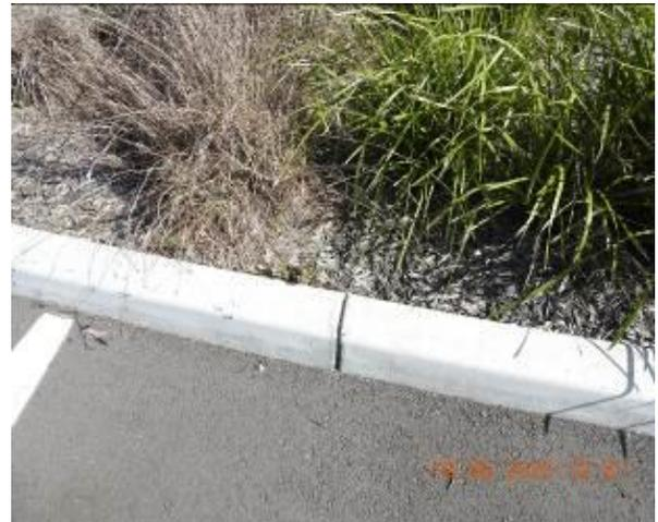
Figure 2166 – Crack propagation through car park kerb
