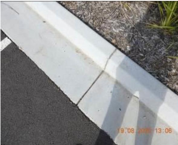
Figure 2279 – Crack propagation through car park kerb
