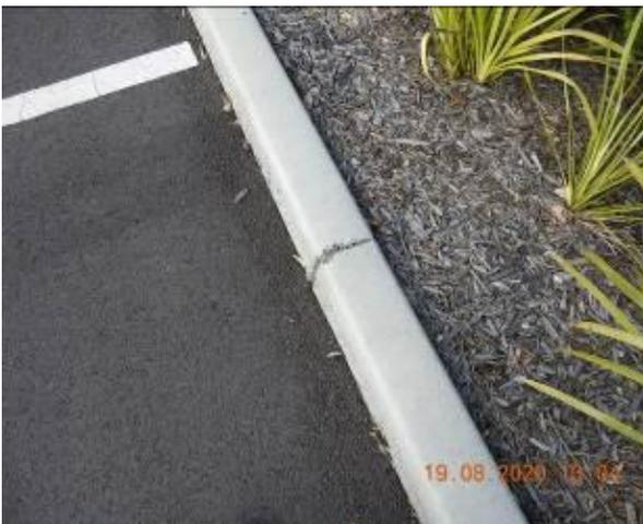
Figure 2245 – Crack propagation through car park kerb
