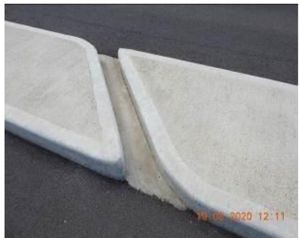
Figure 1718 – Crack propagation through traffic island
