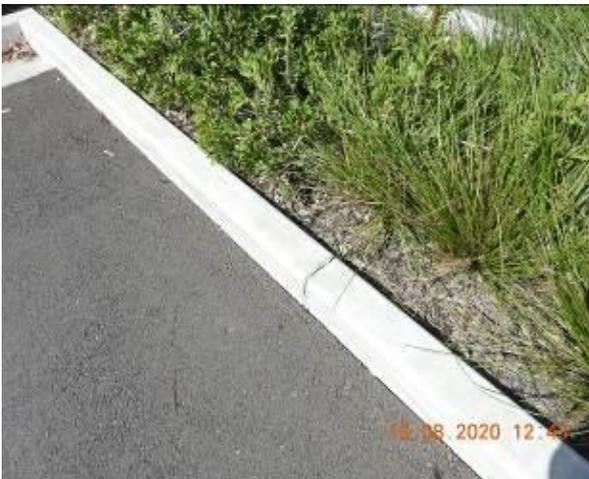
Figure 1991 – Crack propagation through car park kerb
