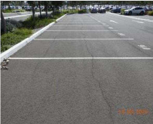
Figure 1451 – Crack propagation through car park pavement
