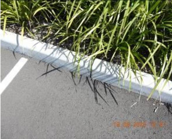
Figure 2169 – Crack propagation through car park kerb
