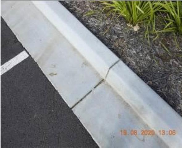
Figure 2277 – Crack propagation through car park kerb
