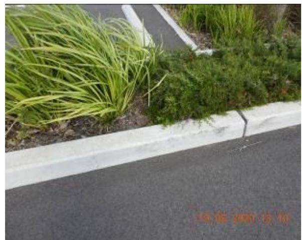
Figure 2192 – Crack propagation through car park kerb
