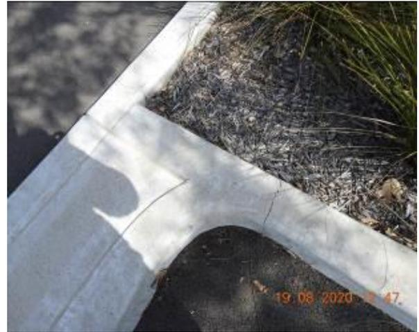
Figure 2050 – Crack propagation through car park kerb
