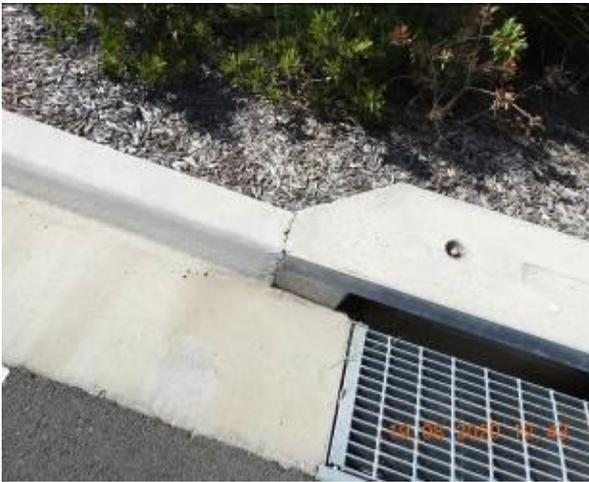
Figure 1997 – Crack propagation through car park kerb
