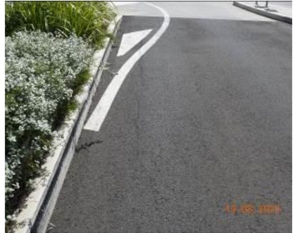
Figure 1426 – Crack propagation through car park pavement
