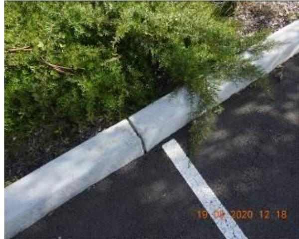
Figure 1768 – Crack propagation through car park kerb
