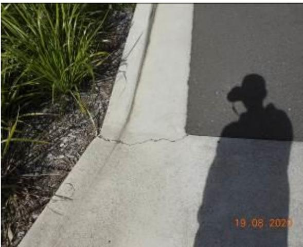
Figure 1399 – Crack propagation through car park pavement
