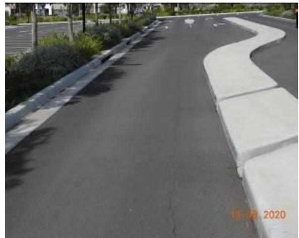
Figure 1406 – Crack propagation through car park pavement
