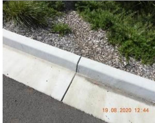
Figure 2008 – Crack propagation through car park kerb and gutter
