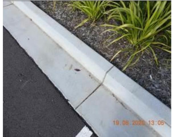
Figure 2266 – Crack propagation through car park kerb
