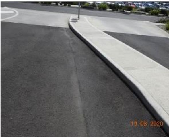
Figure 1429 – Evidence of patchwork through car park pavement
