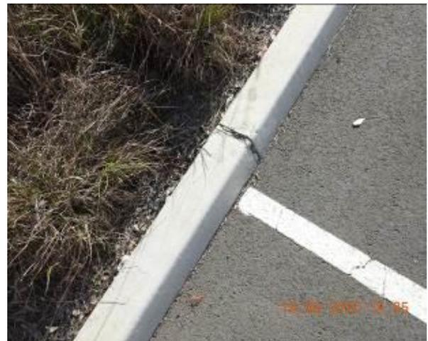
Figure 1290 – Crack propagation and loss of material through car park kerb
