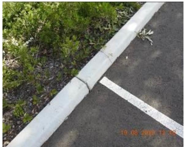
Figure 1766 – Crack propagation through car park kerb
