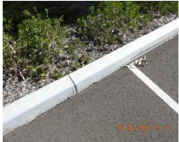
Figure 1758 – Crack propagation through car park kerb
