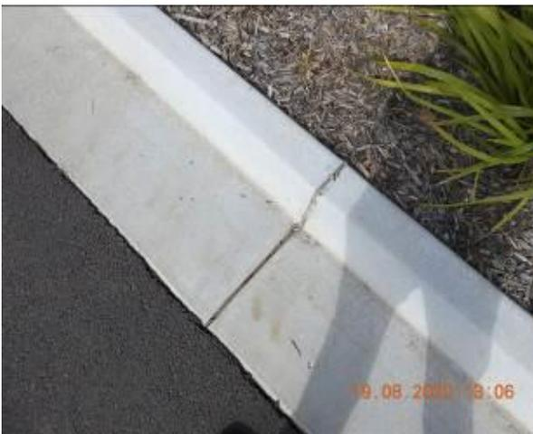
Figure 2281 – Crack propagation through car park kerb
