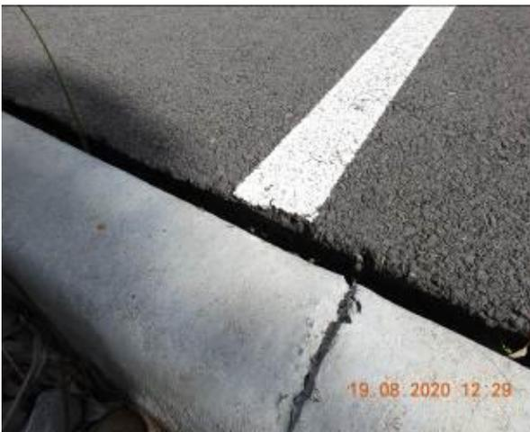
Figure 1867 – Separation through Crack propagation through car park kerb
