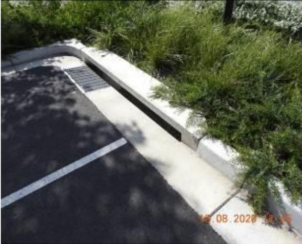
Figure 2019 – General condition of kerb inlet pit and stormwater inlet pit
