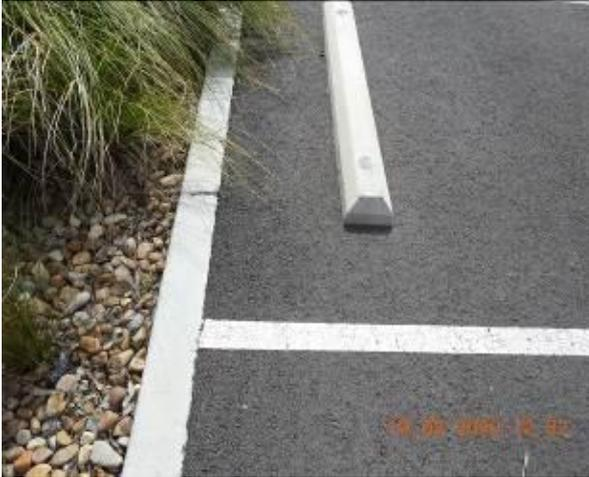
Figure 1893 – Loss of material through car park kerb
