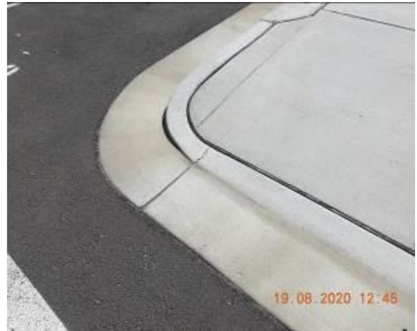
Figure 2022 – Crack propagation through car park kerb layback
