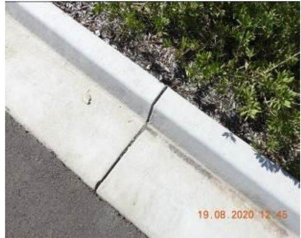
Figure 2018 – Crack propagation through car park kerb
