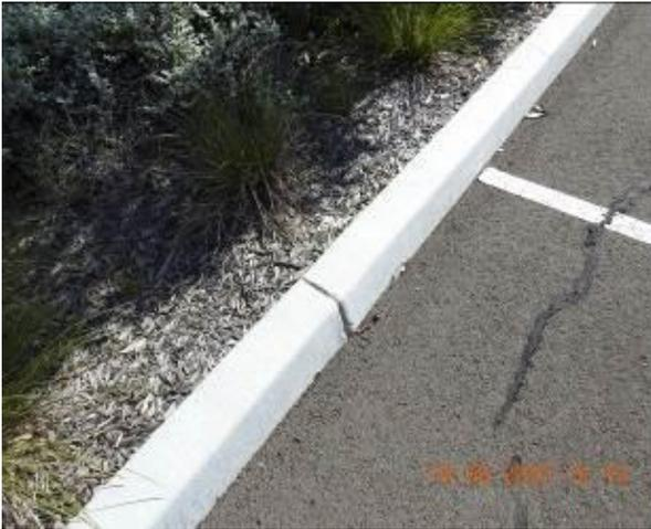
Figure 1761 – Crack propagation through car park kerb
