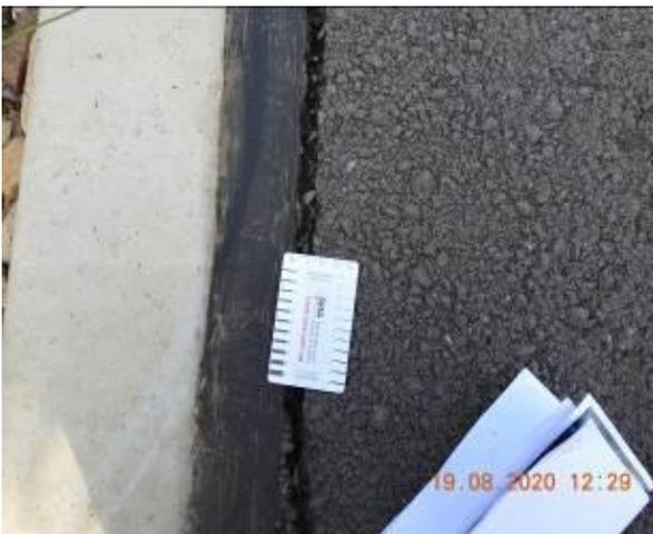
Figure 1855 – Separation through car park kerb approx. 15 mm
