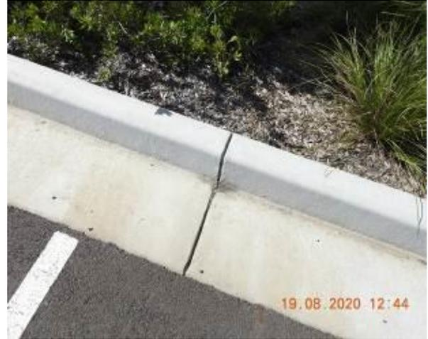
Figure 2002 – Crack propagation through car park kerb
