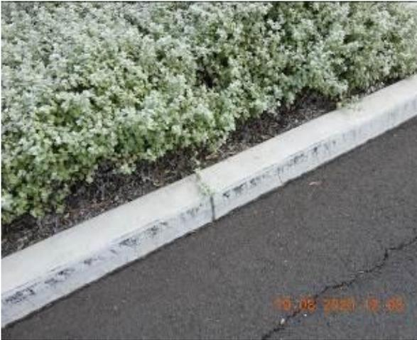
Figure 1695 – Crack propagation through car park kerb
