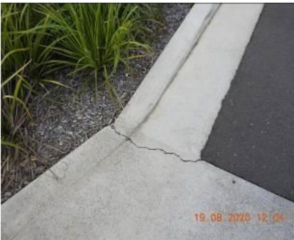
Figure 1651 – Crack propagation through car park kerb and gutter
