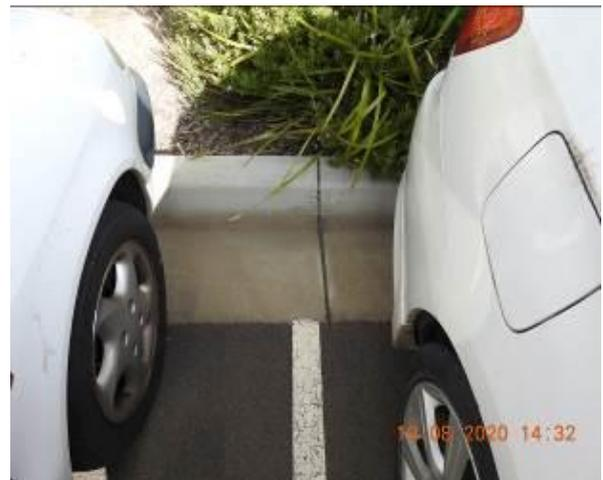
Figure 1244 – Crack propagation through car park kerb
