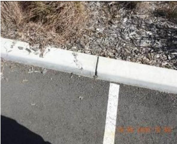
Figure 2159 – Crack propagation through car park kerb
