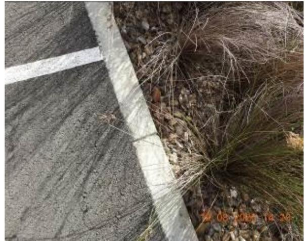
Figure 1214 – Crack propagation through car park kerb
