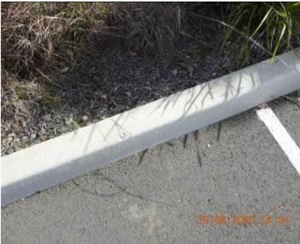
Figure 1277 – Loss of material through car park kerb
