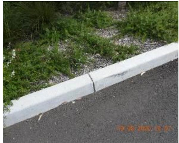
Figure 1674 – Crack propagation through car park kerb
