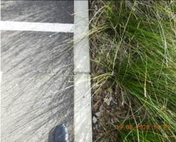
Figure 1221 – Crack propagation through car park kerb
