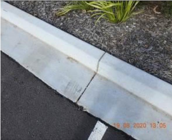
Figure 2265 – Crack propagation through car park kerb
