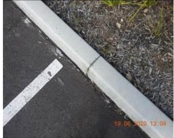
Figure 2248 – Crack propagation through car park kerb
