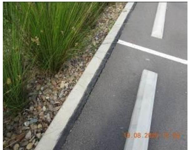
Figure 1850 – Crack propagation through car park kerb
