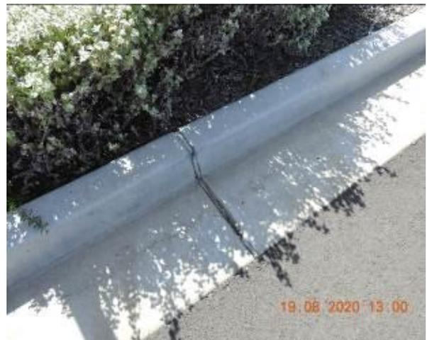
Figure 2216 – Crack propagation and loss of material through car park kerb and gutter
