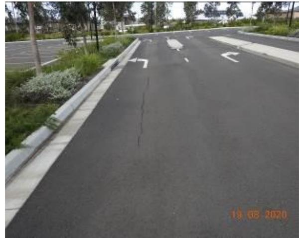
Figure 1410 – Crack propagation through car park pavement
