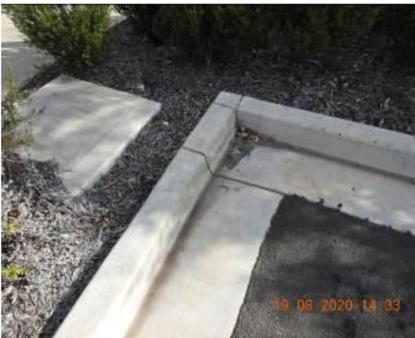
Figure 1261 – Crack propagation through car park kerb
