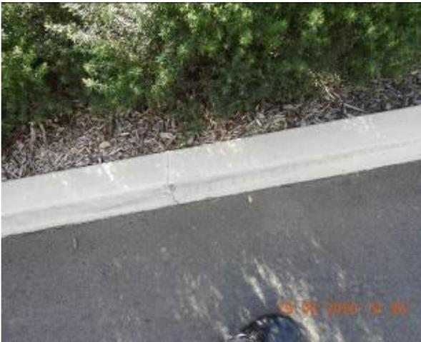
Figure 1301 – Crack propagation through car park kerb
