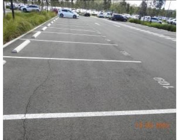
Figure 1486 – Crack propagation through car park pavement
