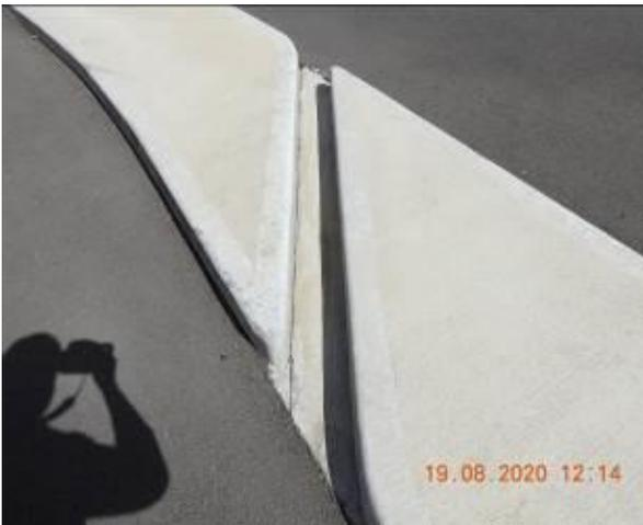
Figure 1721 – Crack propagation through traffic island
