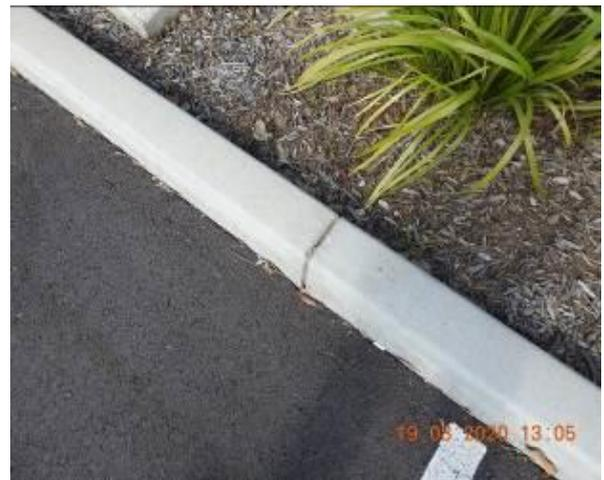
Figure 2258 – Crack propagation through car park kerb
