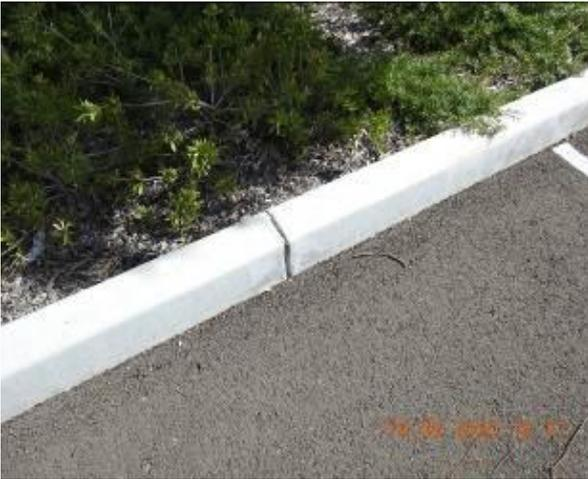
Figure 1749 – Crack propagation through car park kerb
