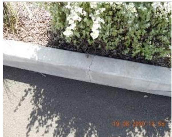
Figure 2144 – Crack propagation through car park kerb
