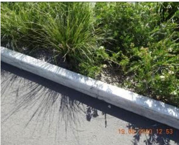
Figure 2119 – Crack propagation through car park kerb
