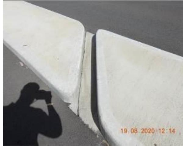
Figure 1726 – Crack propagation through traffic island
