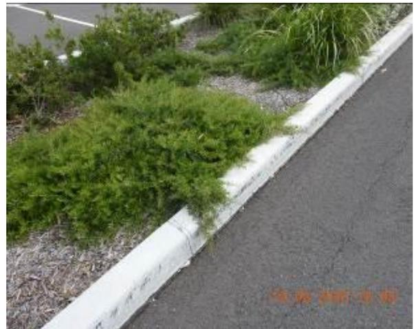
Figure 1692 – Crack propagation through car park kerb
