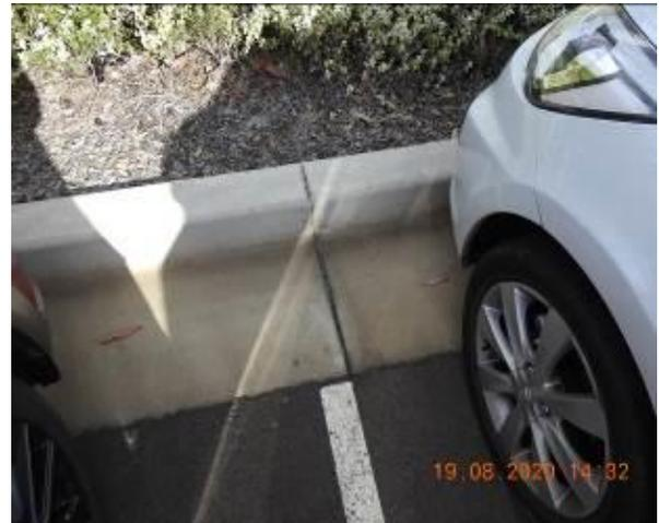
Figure 1242 – Crack propagation through car park kerb
