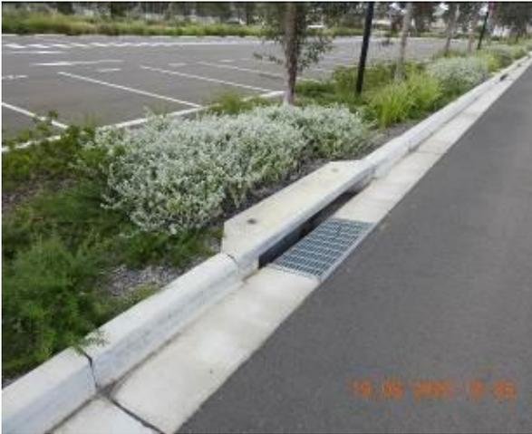
Figure 1659 – General condition of kerb inlet pit and stormwater inlet pit
