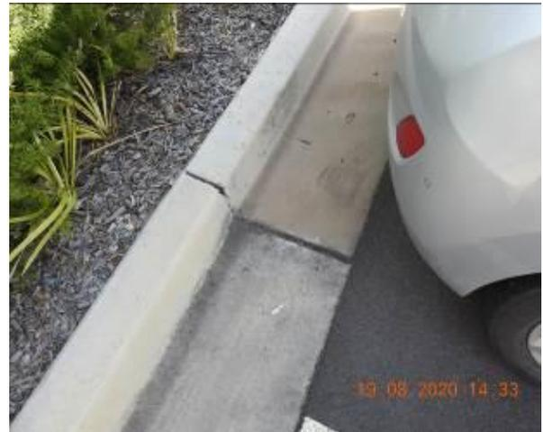
Figure 1254 – Crack propagation and loss of material through car park kerb
