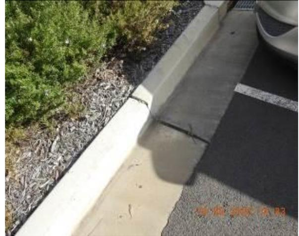
Figure 1252 – Crack propagation and loss of material through car park kerb
