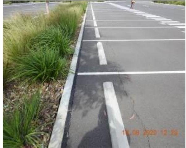
Figure 1858 – Crack propagation through car park kerb
