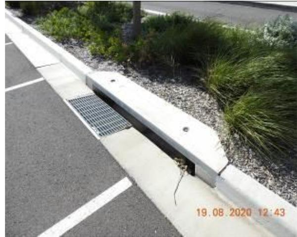
Figure 1996 – General condition of kerb inlet pit and stormwater inlet pit
