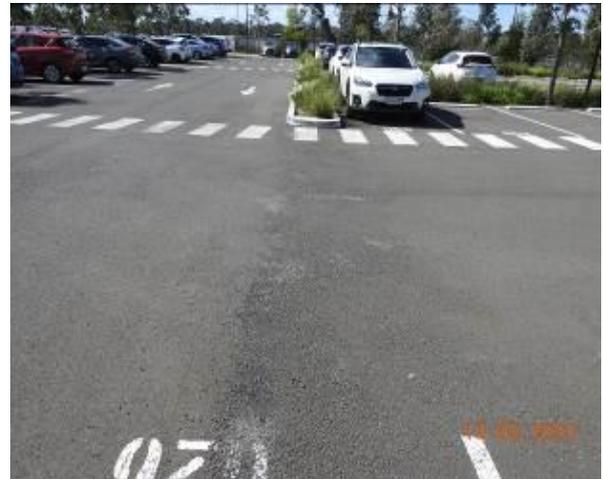
Figure 1458 – Loss of material through car park pavement
