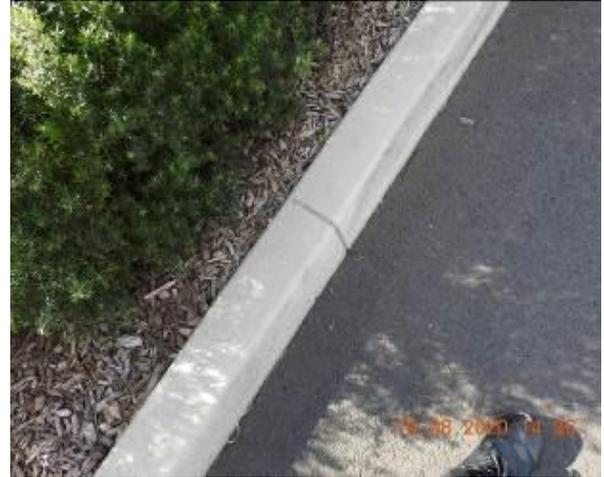
Figure 1300 – Crack propagation through car park kerb
