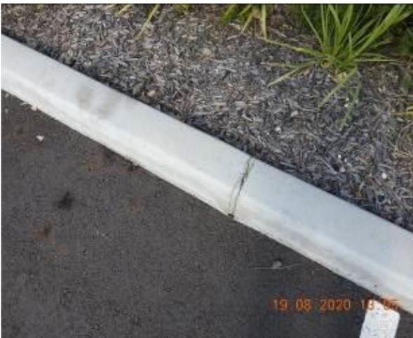
Figure 2255 – Crack propagation through car park kerb
