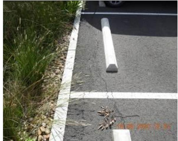
Figure 1906 – General condition of car park kerb and evidence of patchwork through carpark pavement
