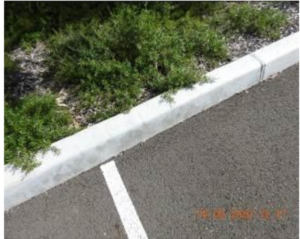
Figure 1750 – Crack propagation through car park kerb
