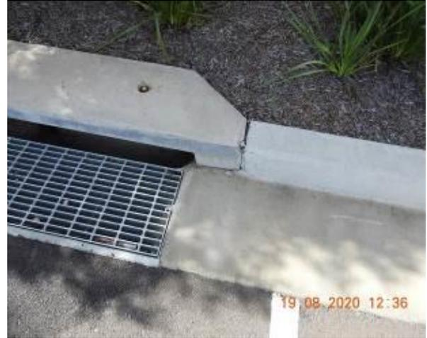
Figure 1936 – Crack propagation and loss of material through car park kerb
