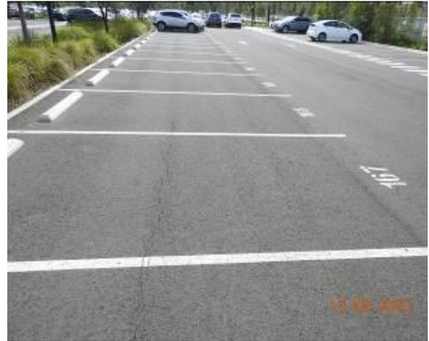
Figure 1516 – Crack propagation through car park pavement
