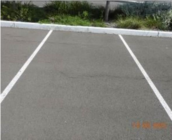
Figure 1449 – Crack propagation through car park pavement
