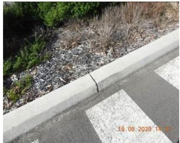
Figure 1316 – Crack propagation through car park kerb
