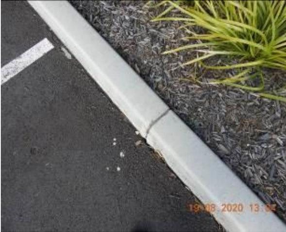
Figure 2247 – Crack propagation through car park kerb
