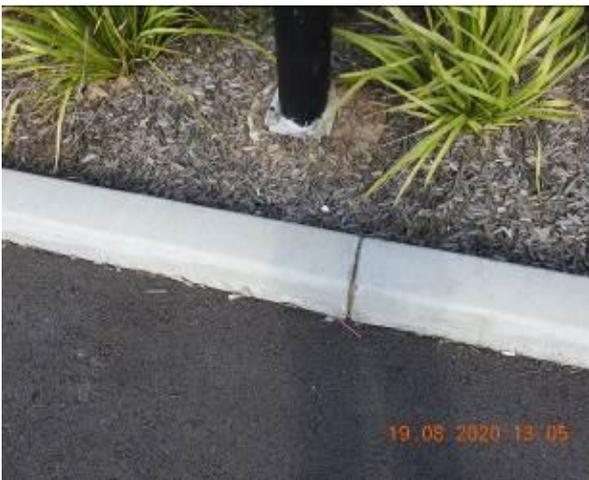
Figure 2257 – Crack propagation through car park kerb
