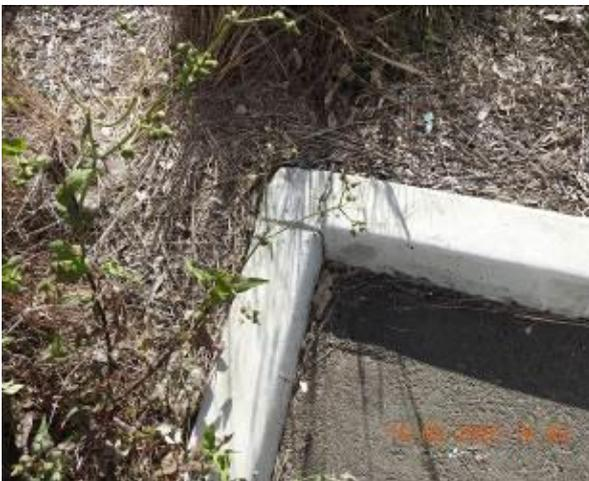
Figure 1295 – Crack propagation through car park kerb
