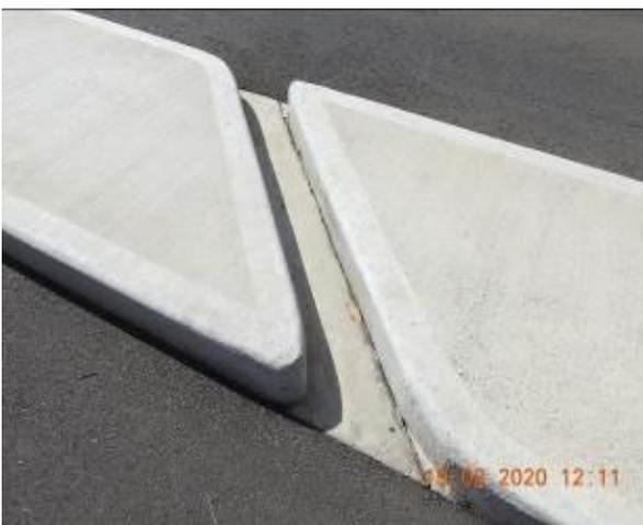
Figure 1717 – Crack propagation through traffic island
