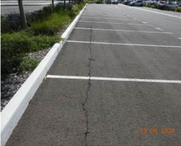
Figure 1443 – Crack propagation and evidence of patchwork through car park pavement
