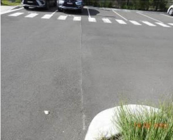
Figure 1527 – Crack propagation through car park pavement
