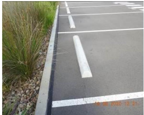
Figure 1782 – Crack propagation through car park kerb
