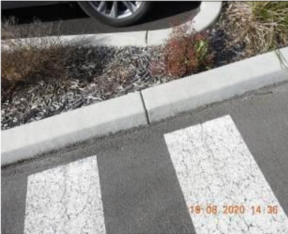
Figure 1305 – Crack propagation through car park kerb
