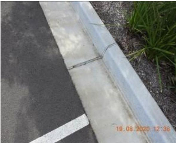
Figure 1931 – Crack propagation through car park kerb and gutter
