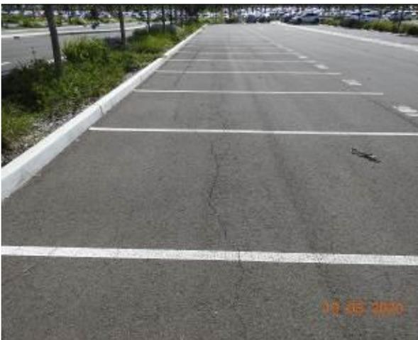
Figure 1441 – Crack propagation through car park pavement
