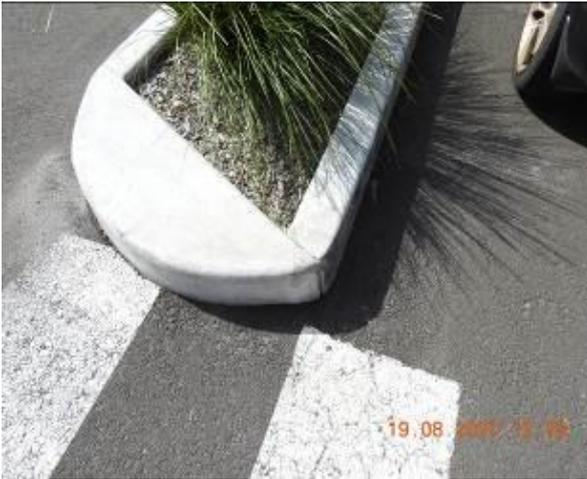
Figure 1845 – Crack propagation through car park kerb
