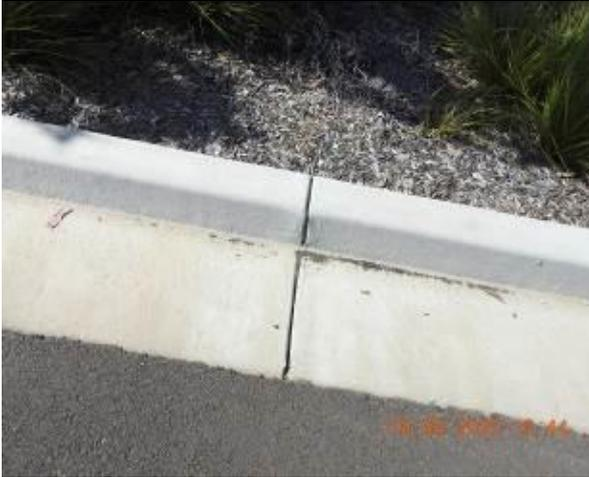
Figure 2001 – Crack propagation through car park kerb
