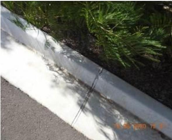
Figure 1949 – Crack propagation through car park kerb
