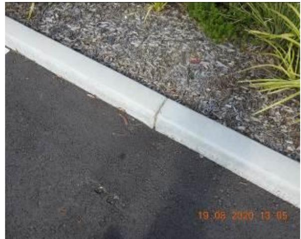
Figure 2262 – Crack propagation through car park kerb
