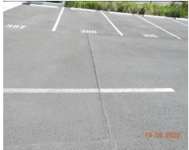
Figure 1560 – Evidence of patchwork through car park pavement
