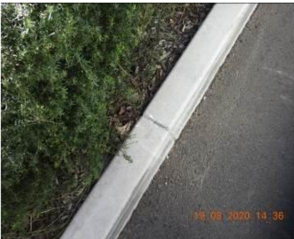
Figure 1297 – Crack propagation through car park kerb
