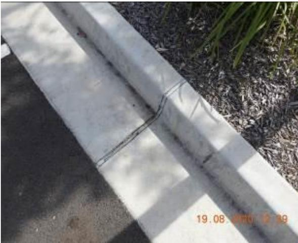
Figure 1967 – Crack propagation through car park kerb and gutter
