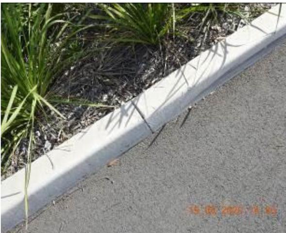
Figure 1279 – Crack propagation through car park kerb
