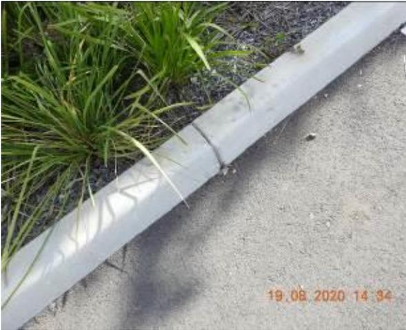
Figure 1275 – Crack propagation through car park kerb
