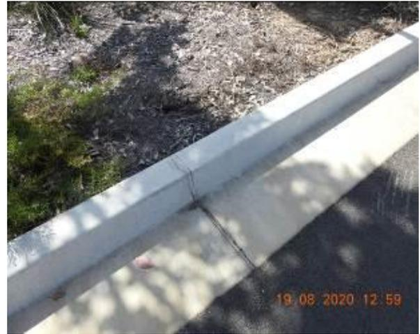
Figure 2206 – Crack propagation through car park kerb
