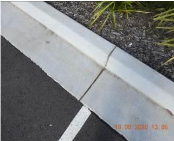
Figure 2267 – Crack propagation through car park kerb
