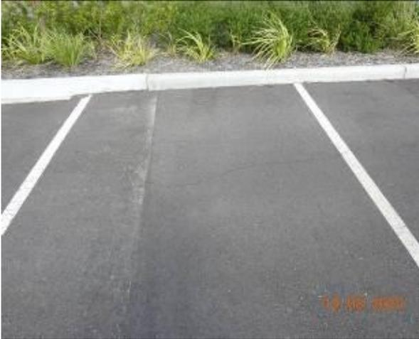
Figure 1641 – Crack propagation through car park pavement
