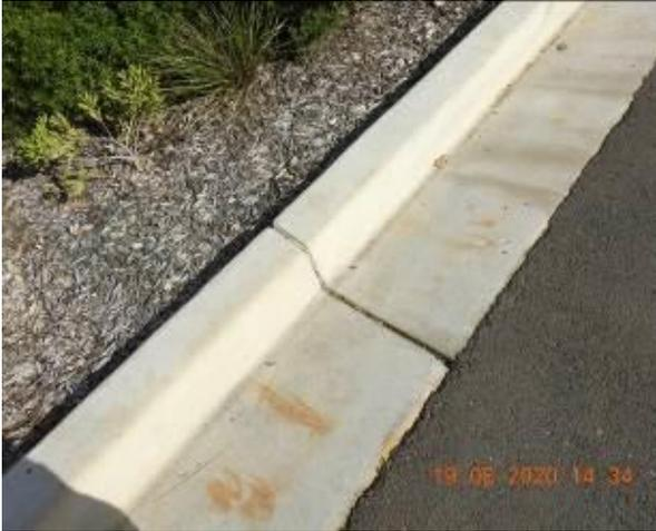
Figure 1269 – Crack propagation through car park kerb
