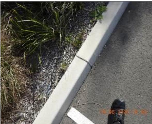
Figure 1291 – Crack propagation through car park kerb
