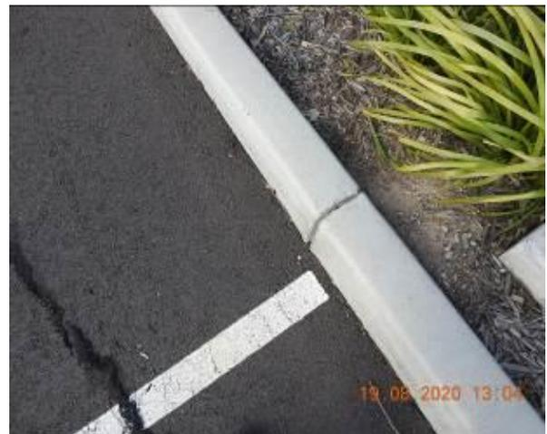
Figure 2252 – Crack propagation through car park kerb
