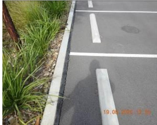
Figure 1852 – Crack propagation through car park kerb
