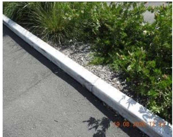
Figure 1988 – Crack propagation through car park kerb
