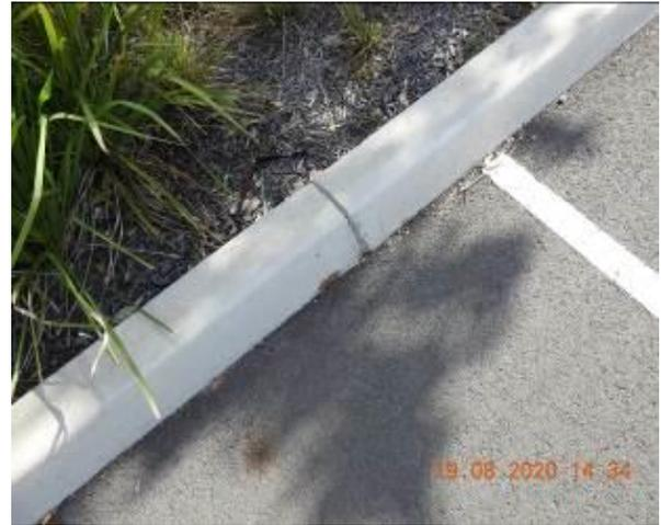
Figure 1276 – Crack propagation through car park kerb
