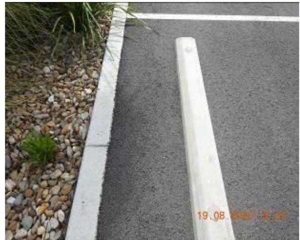
Figure 1896 – Crack propagation through car park kerb
