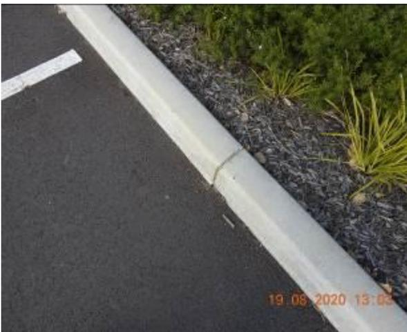
Figure 2227 – Crack propagation through car park kerb
