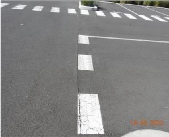
Figure 1587 – Crack propagation through car park pavement
