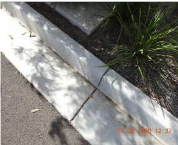
Figure 1951 – Crack propagation through car park kerb
