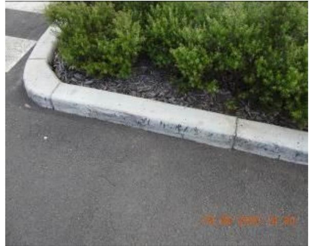
Figure 1234 – Crack propagation through car park kerb
