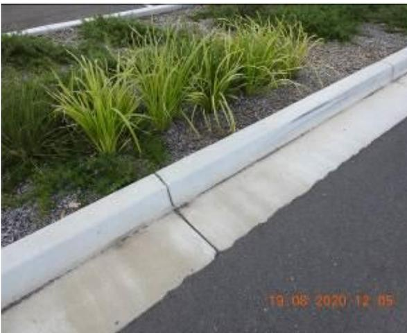
Figure 1657 – Crack propagation through car park kerb
