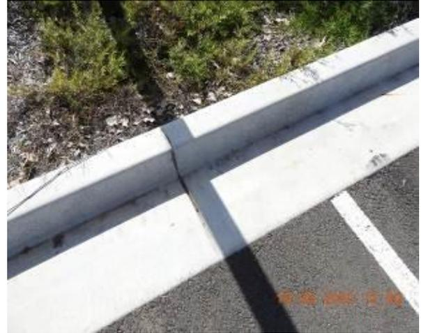
Figure 2200 – Crack propagation through car park kerb
