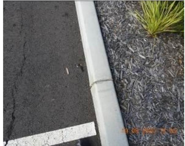
Figure 2254 – Crack propagation through car park kerb
