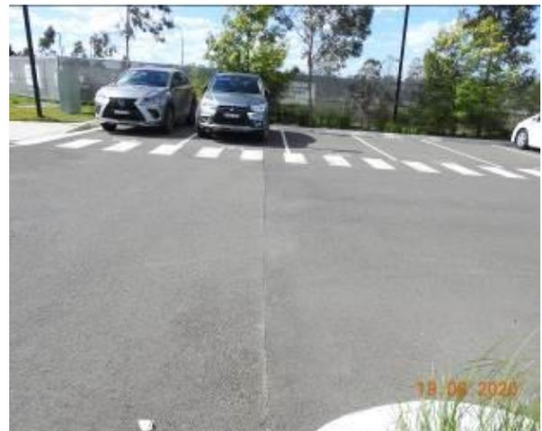
Figure 1526 – Crack propagation through car park pavement
