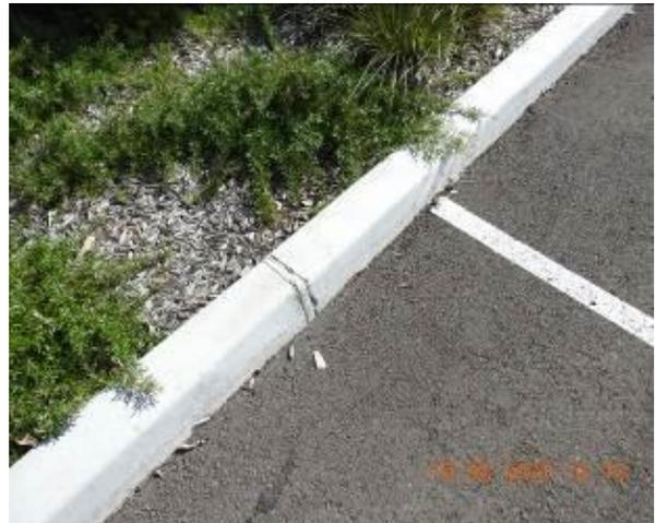
Figure 1764 – Crack propagation and loss of material through car park kerb
