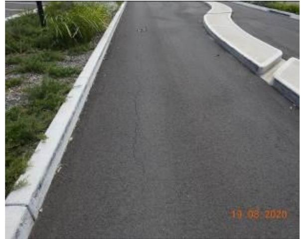
Figure 1420 – Crack propagation through car park pavement
