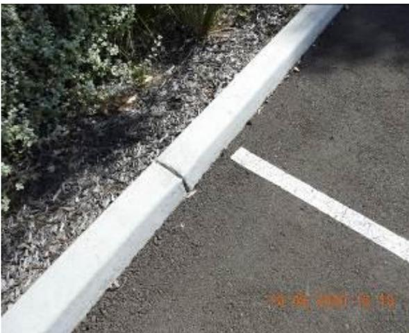
Figure 1765 – Crack propagation through car park kerb
