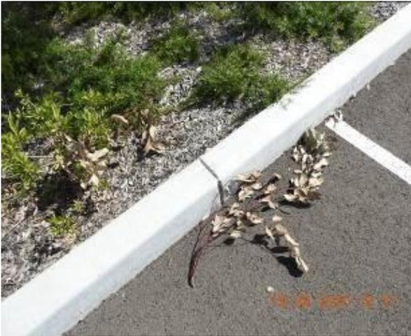
Figure 1755 – Crack propagation through car park kerb
