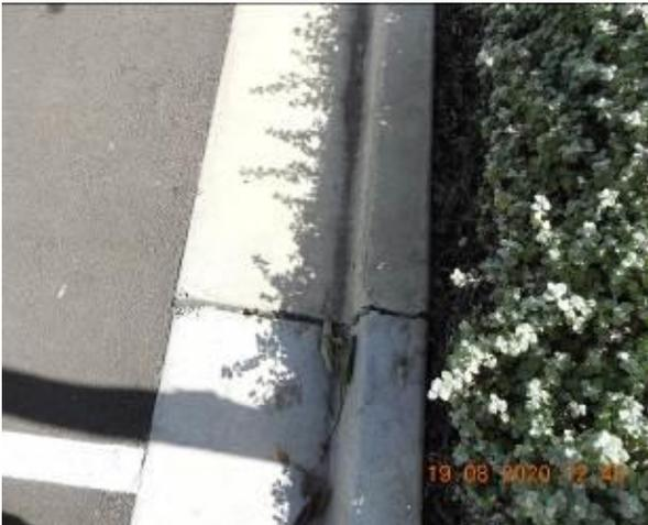
Figure 1975 – Crack propagation and loss of material through car park kerb and gutter
