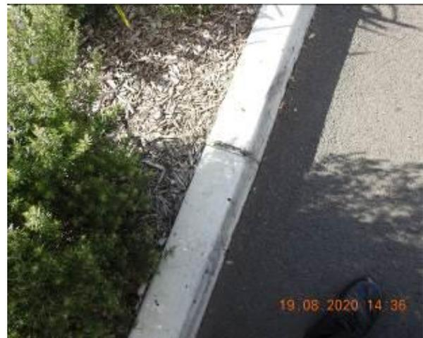
Figure 1298 – Crack propagation and loss of material through car park kerb
