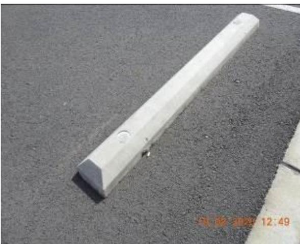
Figure 2065 – Loss of material through car park kerb
