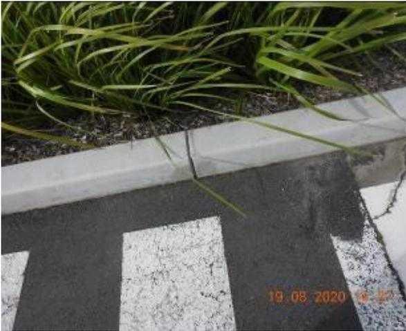
Figure 1197 – Crack propagation through car park kerb
