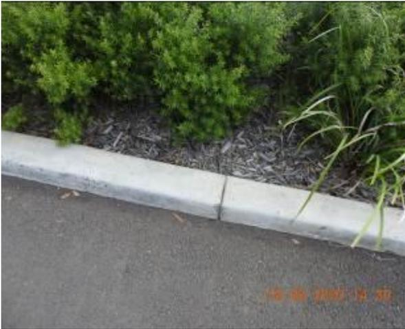
Figure 1233 – Hairline cracking through car park kerb
