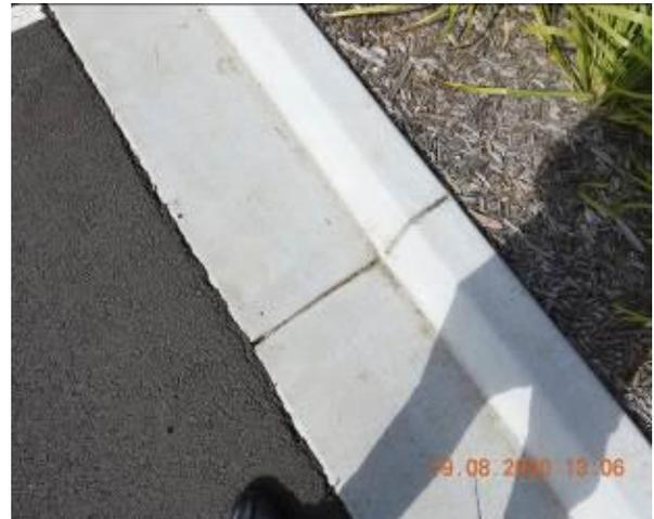
Figure 2280 – Crack propagation through car park kerb
