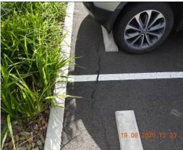
Figure 1907 – General condition of car park kerb and evidence of patchwork through carpark pavement
