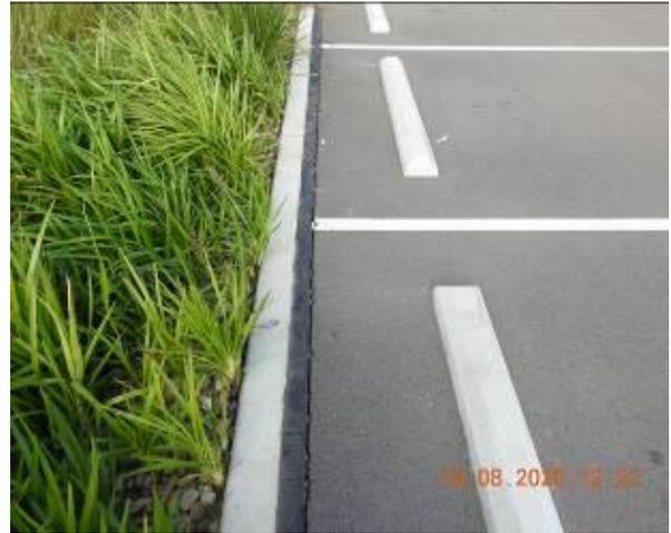
Figure 1786 – Crack propagation through car park kerb
