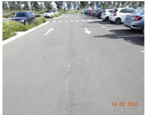
Figure 1544 – Loss of material through car park pavement
