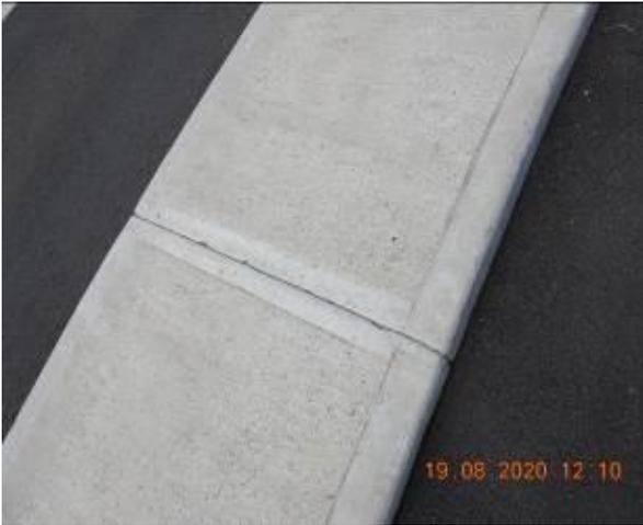
Figure 1707 – Crack propagation through traffic island
