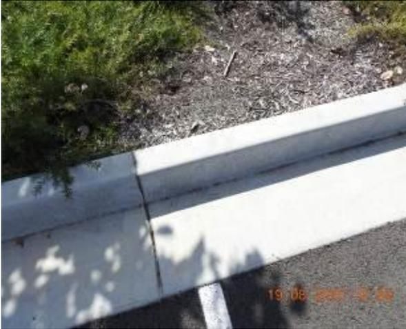
Figure 2199 – Crack propagation through car park kerb
