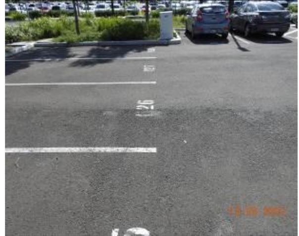
Figure 1456 – Loss of material through car park pavement
