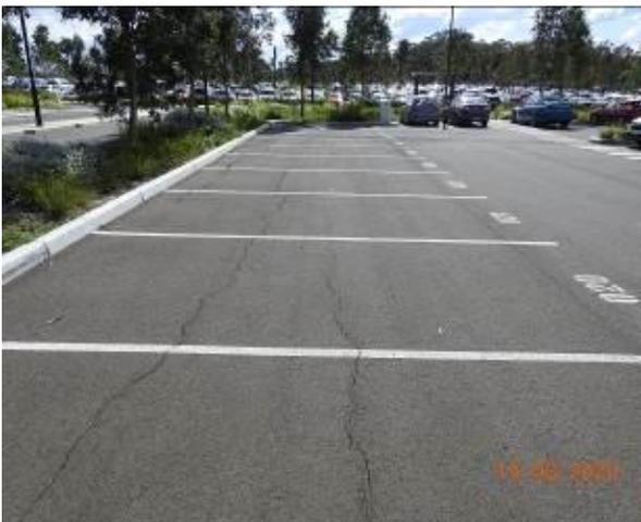
Figure 1453 – Crack propagation through car park pavement
