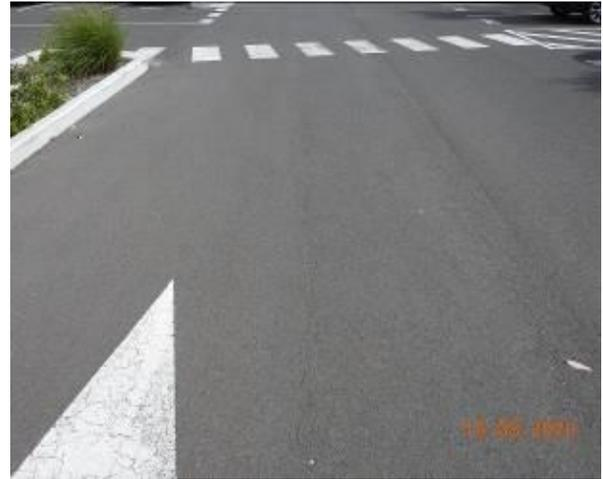
Figure 1546 – Crack propagation through car park pavement
