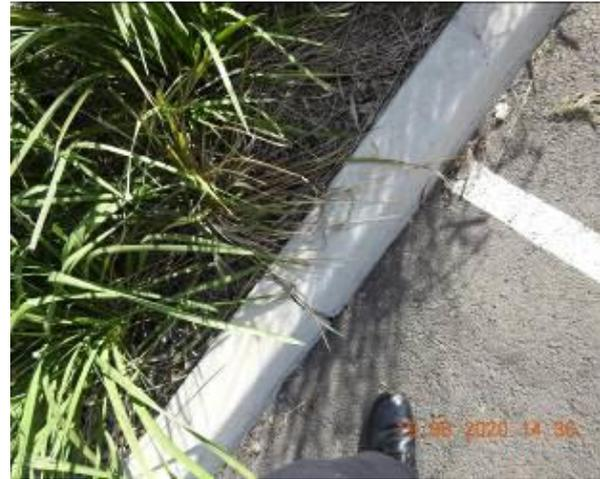
Figure 1294 – Crack propagation through car park kerb
