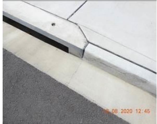
Figure 2026 – Crack propagation through car park gutter
