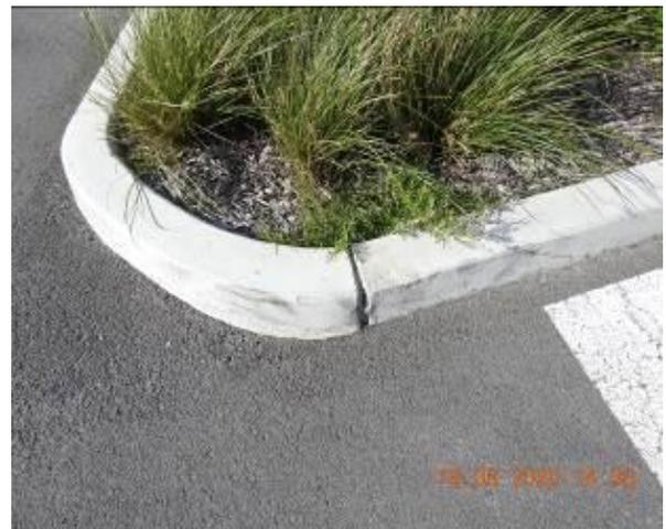
Figure 1304 – Crack propagation and loss of material through car park kerb
