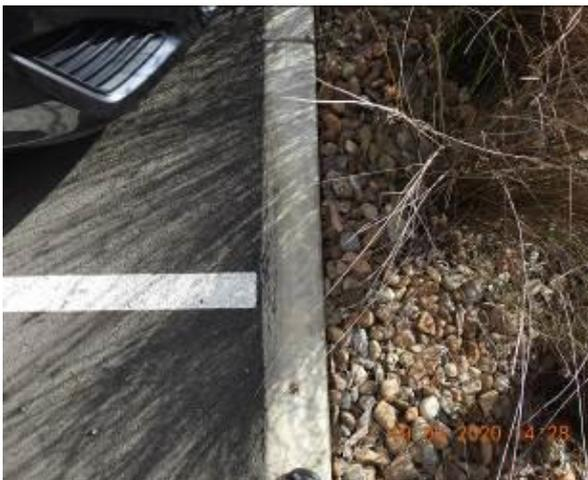
Figure 1207 – Crack propagation and loss of material through car park kerb
