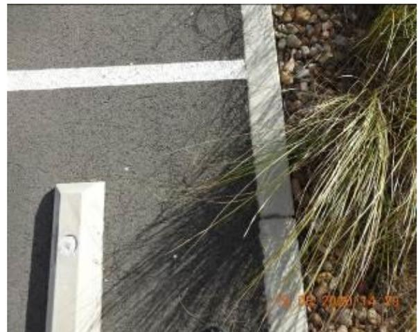
Figure 1226 – Crack propagation through car park kerb
