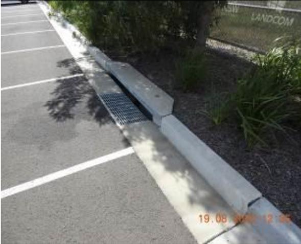
Figure 1935 – General condition of kerb inlet pit and stormwater inlet pit
