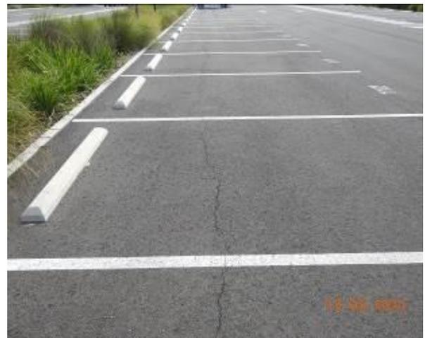
Figure 1484 – Crack propagation through car park pavement
