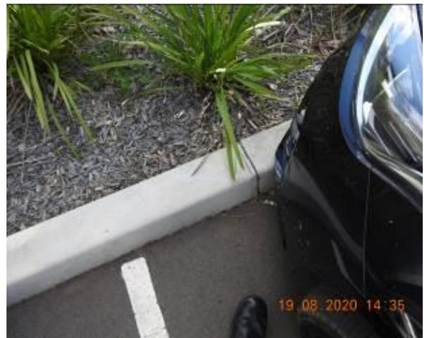
Figure 1286 – Crack propagation through car park kerb
