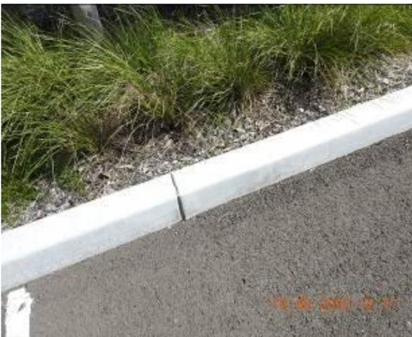
Figure 1747 – Crack propagation through car park kerb
