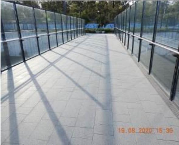
Figure 2400 – General condition of RailCorp overbridge pavement
