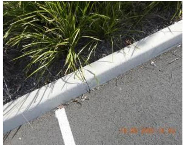
Figure 1278 – Crack propagation through car park kerb
