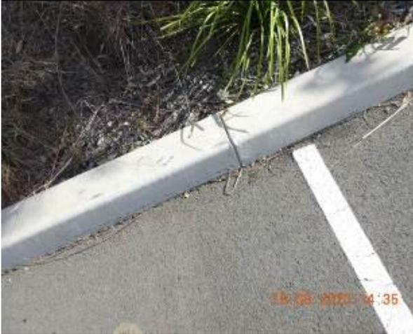
Figure 1281 – Crack propagation through car park kerb
