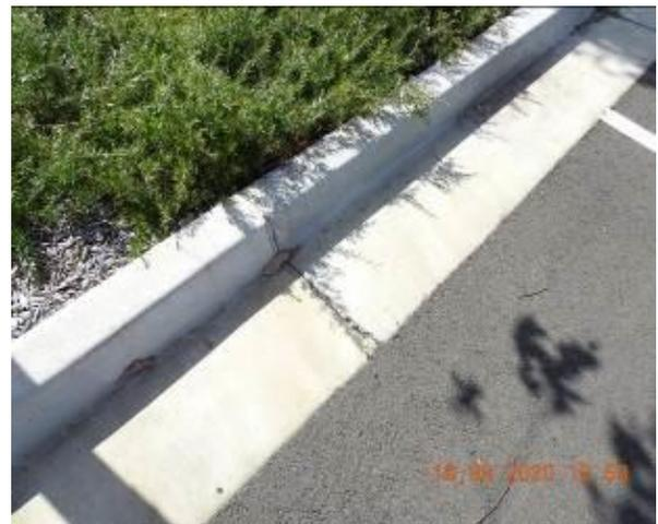
Figure 2210 – Crack propagation and loss of material through car park kerb and gutter
