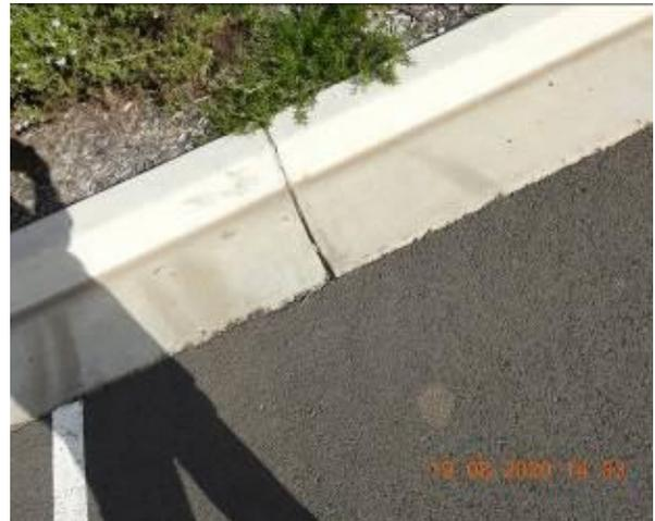
Figure 1260 – Crack propagation through car park kerb
