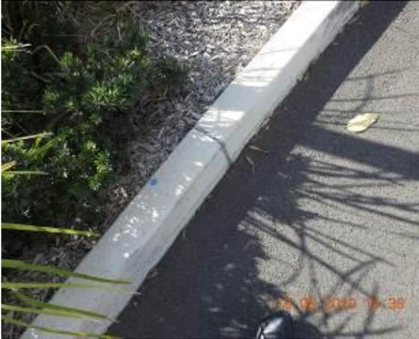
Figure 1299 – Crack propagation through car park kerb
