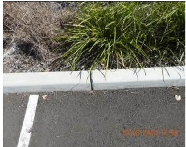
Figure 2154 – Crack propagation through car park kerb
