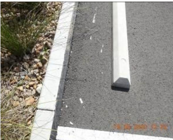
Figure 1831 – Crack propagation through car park kerb
