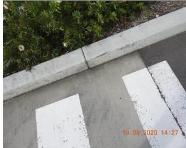
Figure 1198 – Crack propagation through car park kerb
