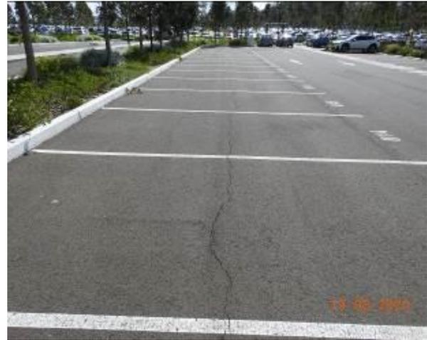
Figure 1450 – Crack propagation through car park pavement
