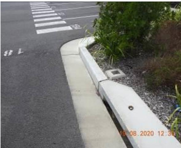
Figure 1913 – General condition of service pit and crack propagation through car park gutter
