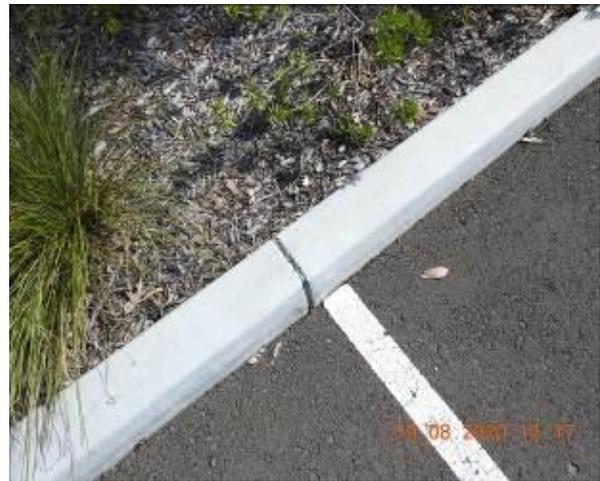
Figure 1740 – Crack propagation through car park kerb
