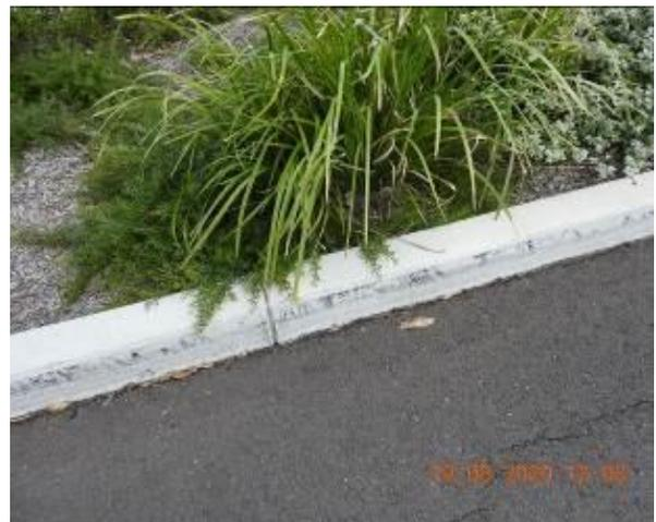
Figure 1694 – Crack propagation through car park kerb
