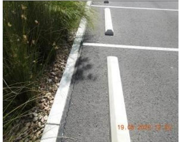
Figure 1834 – Crack propagation through car park kerb
