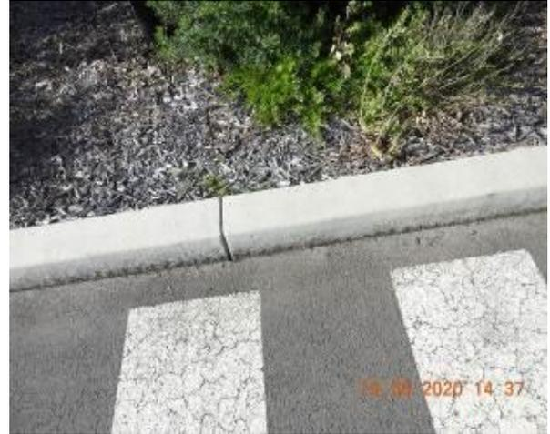
Figure 1312 – Crack propagation through car park kerb
