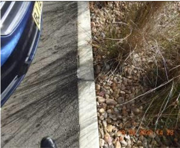
Figure 1205 – Crack propagation and loss of material through car park kerb
