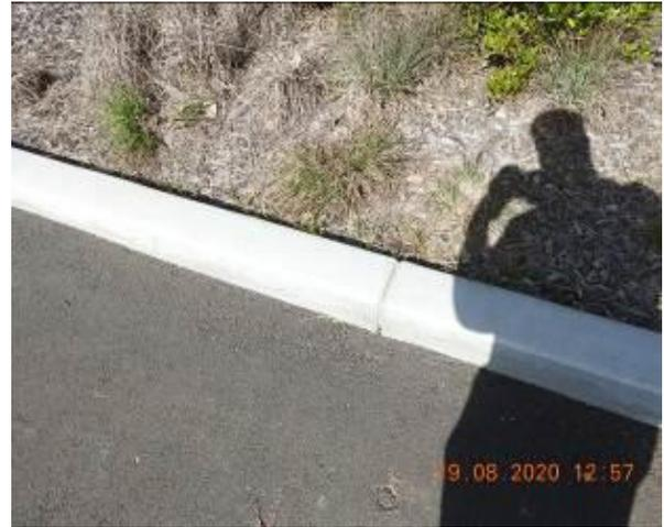
Figure 2182 – Crack propagation through car park kerb
