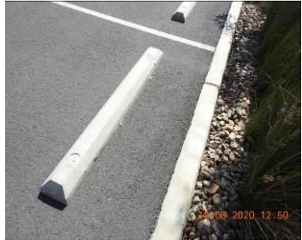
Figure 2074 – Loss of material through car park kerb
