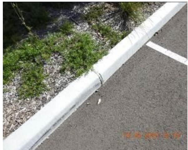
Figure 1760 – Crack propagation through car park kerb
