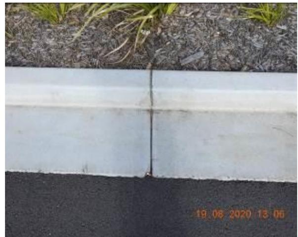
Figure 2276 – Crack propagation through car park kerb
