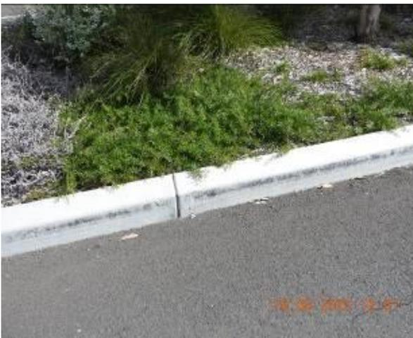
Figure 1681 – Crack propagation through car park kerb
