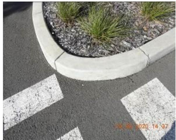
Figure 1310 – Crack propagation through car park kerb
