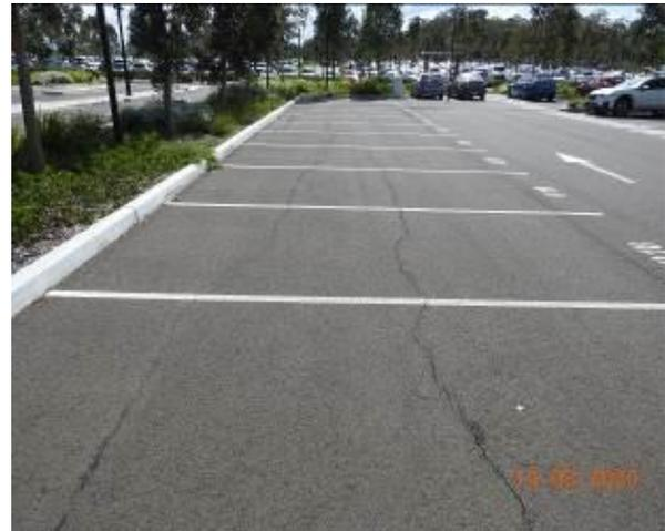
Figure 1452 – Crack propagation through car park pavement t
