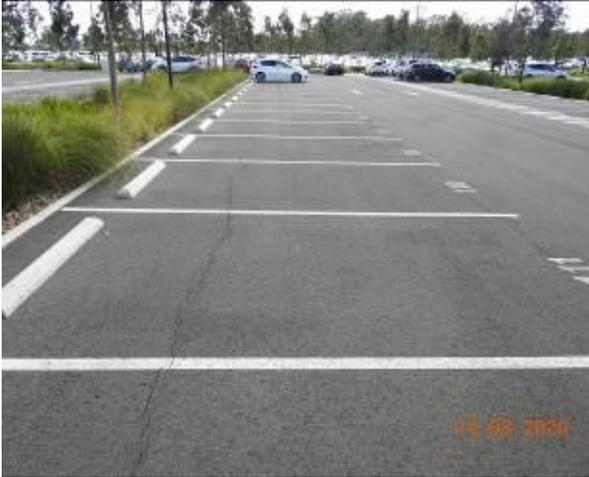
Figure 1485 – Crack propagation through car park pavement
