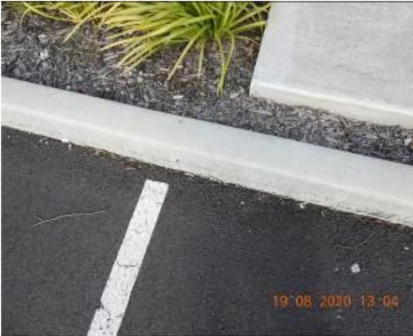
Figure 2241 – Crack propagation through car park kerb
