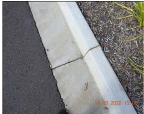
Figure 2282 – Crack propagation through car park kerb
