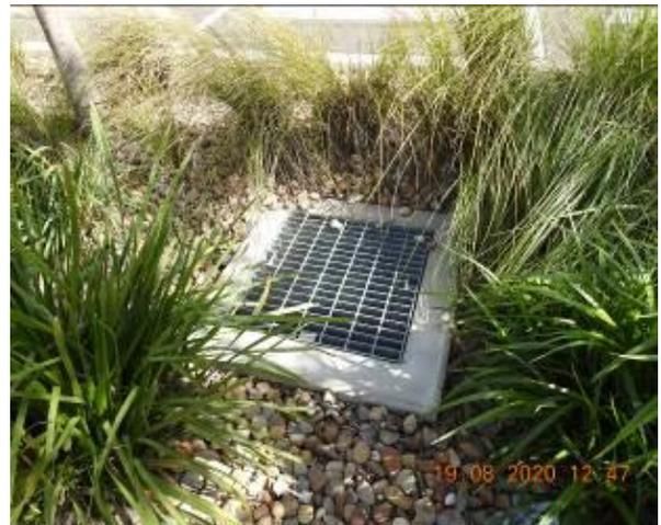
Figure 2040 – General condition of stormwater inlet pit
