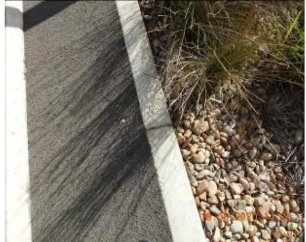
Figure 1210 – Crack propagation through car park kerb
