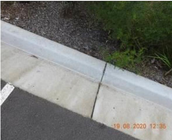
Figure 1919 – Crack propagation through car park kerb
