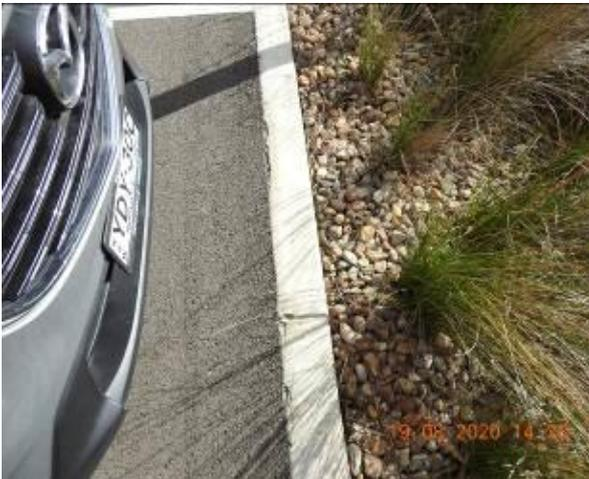
Figure 1211 – Crack propagation and loss of material through car park kerb
