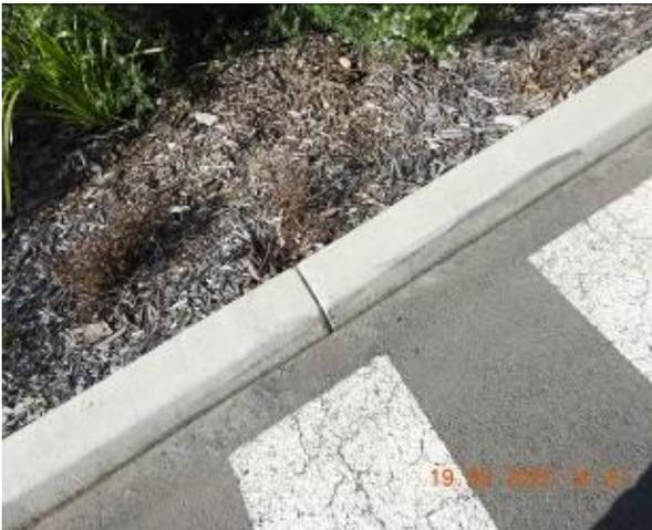
Figure 1313 – Crack propagation through car park kerb
