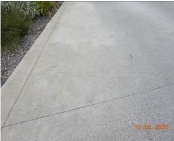
Figure 1397 – Crack propagation through car park pavement
