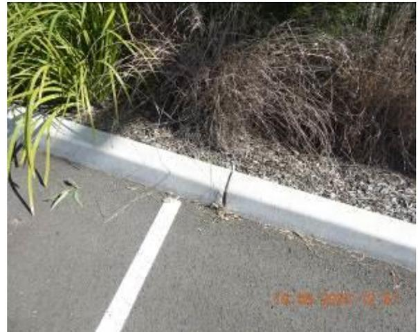
Figure 2172 – Crack propagation through car park kerb
