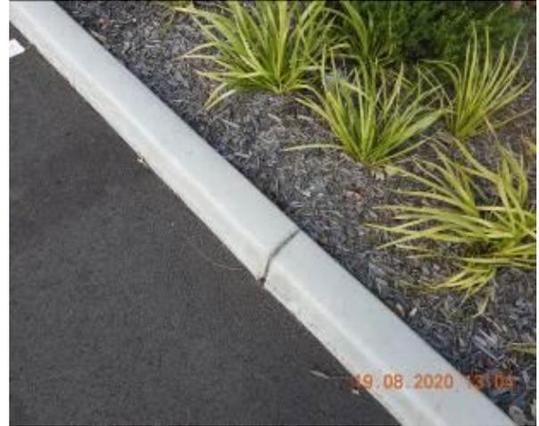
Figure 2236 – Crack propagation through car park kerb
