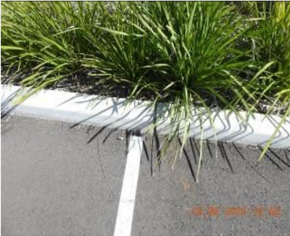
Figure 2157 – Crack propagation through car park kerb
