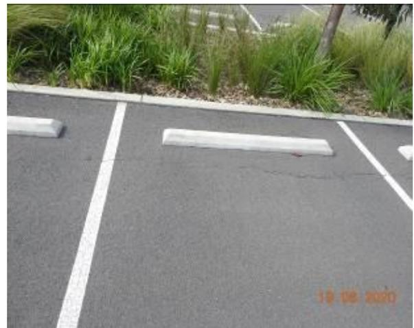
Figure 1502 – Crack propagation through car park pavement
