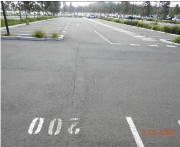
Figure 1643 – Crack propagation through car park pavement
