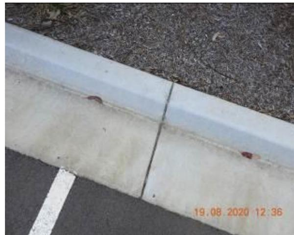
Figure 1928 – Crack propagation through car park kerb
