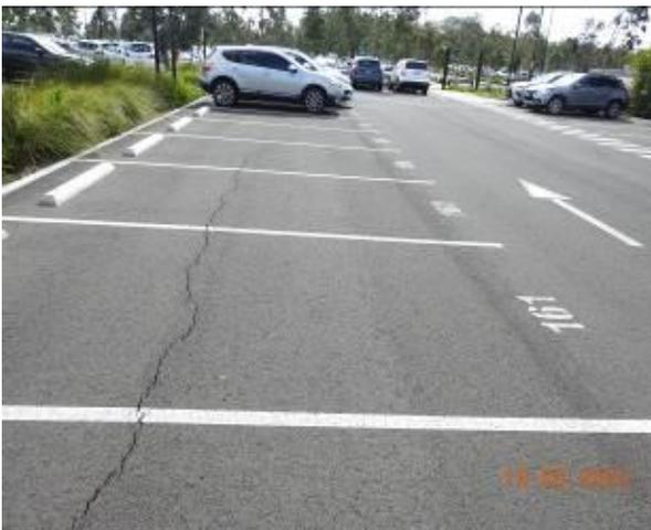
Figure 1519 – Crack propagation through car park pavement
