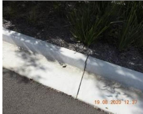
Figure 1942 – Crack propagation through car park kerb
