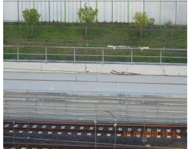
Figure 2385 – Crack propagation and efflorescence through RailCorp retaining wall
