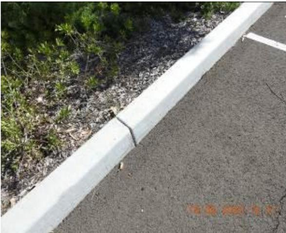
Figure 1745 – Crack propagation through car park kerb
