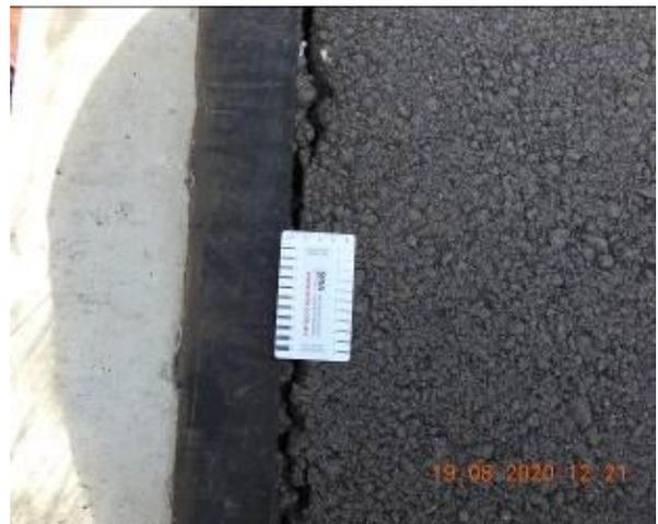
Figure 1784 – Crack propagation through car park kerb approx. 10 mm in width
