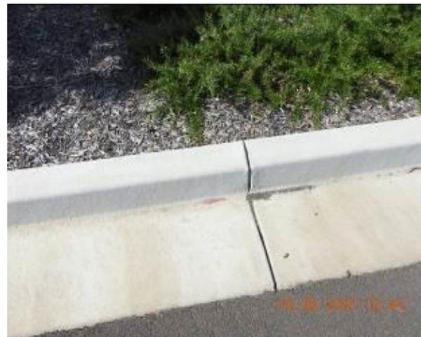
Figure 2000 – Crack propagation through car park kerb
