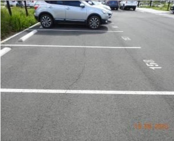
Figure 1521 – Crack propagation through car park pavement
