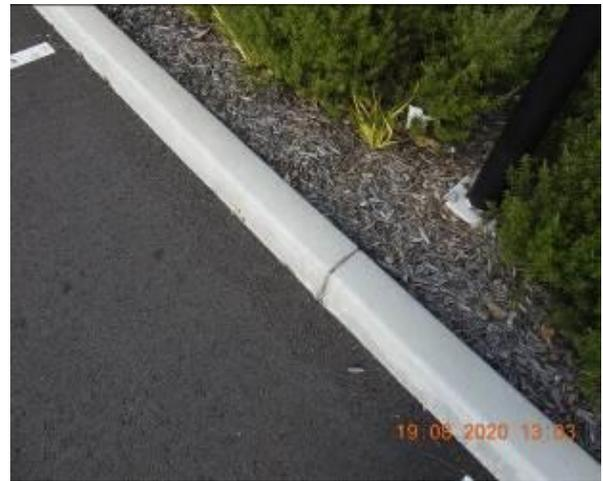
Figure 2226 – Crack propagation through car park kerb
