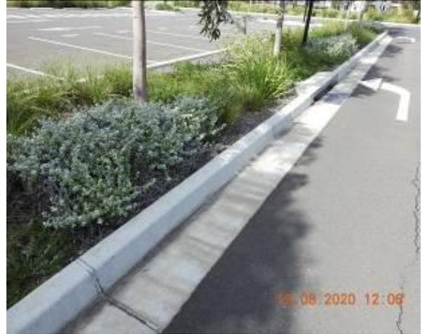
Figure 1666 – Crack propagation through car park kerb
