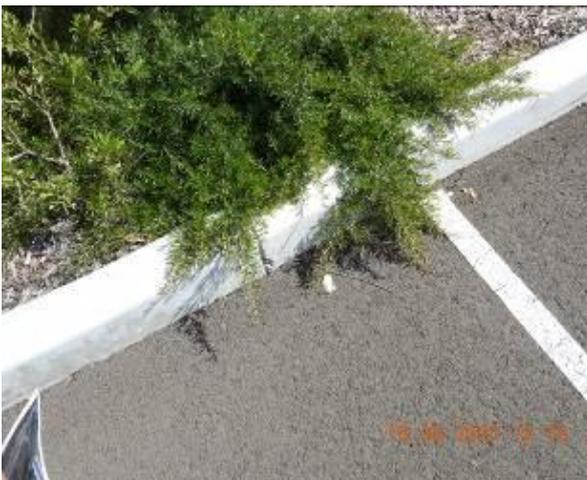
Figure 1759 – Crack propagation through car park kerb
