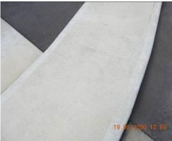
Figure 1703 – Hairline cracking through traffic island
