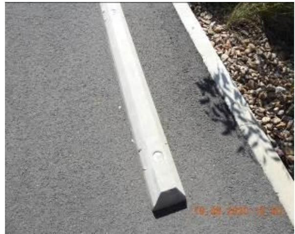
Figure 2076 – Loss of material through car park kerb
