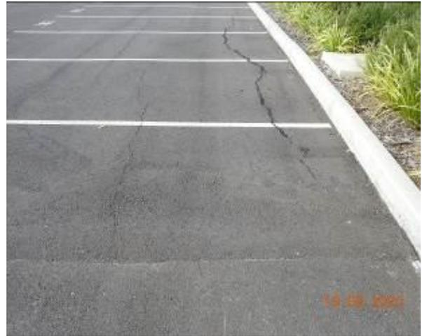
Figure 1632 – Crack propagation and Evidence of patchwork through car park pavement
