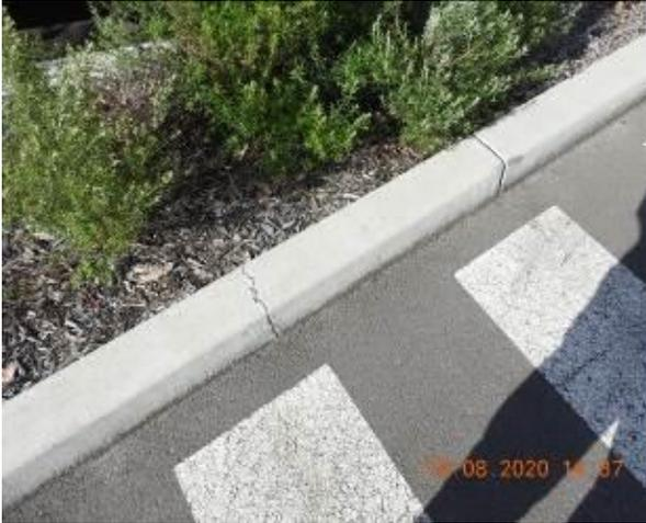
Figure 1311 – Crack propagation through car park kerb
