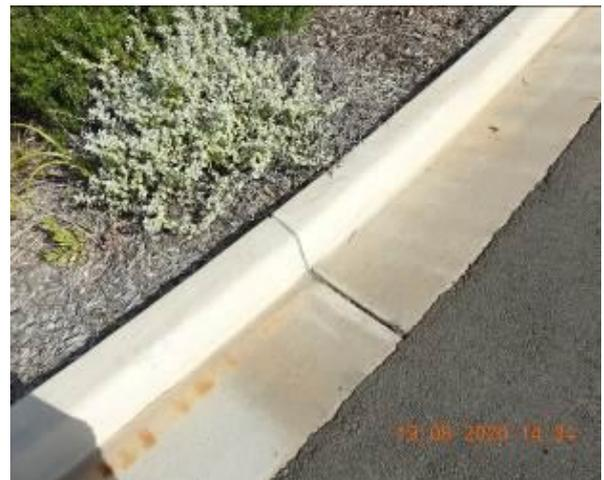
Figure 1268 – Crack propagation through car park kerb
