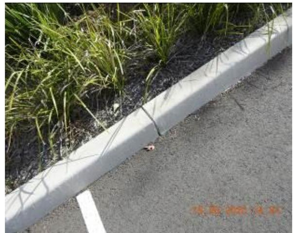
Figure 1274 – Crack propagation through car park kerb
