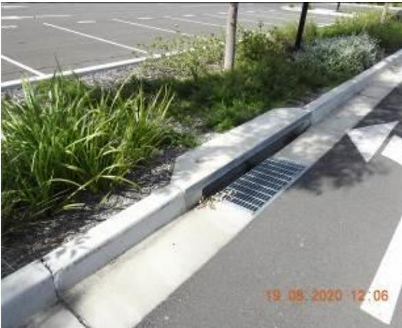
Figure 1667 – Crack propagation and loss of material through car park kerb and general condition of stormwater inlet pit
