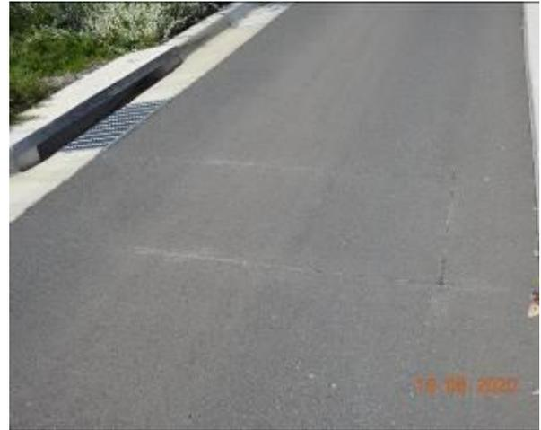
Figure 1402 – Crack propagation through car park pavement
