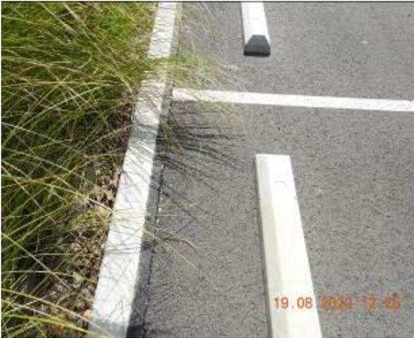
Figure 1833 – Crack propagation through car park kerb
