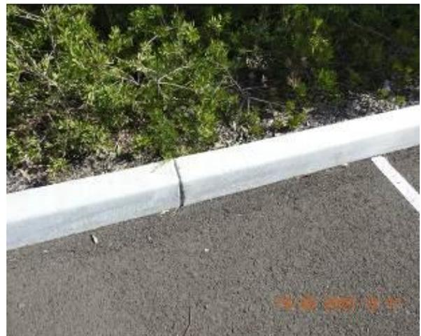
Figure 1748 – Crack propagation through car park kerb
