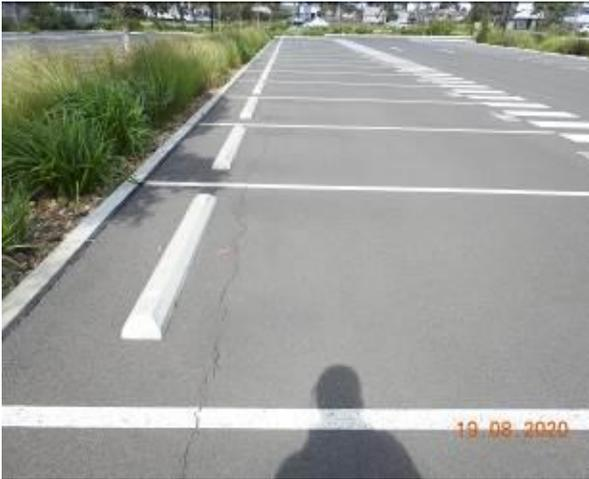
Figure 1503 – Crack propagation through car park pavement
