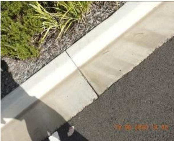
Figure 1259 – Crack propagation through car park kerb
