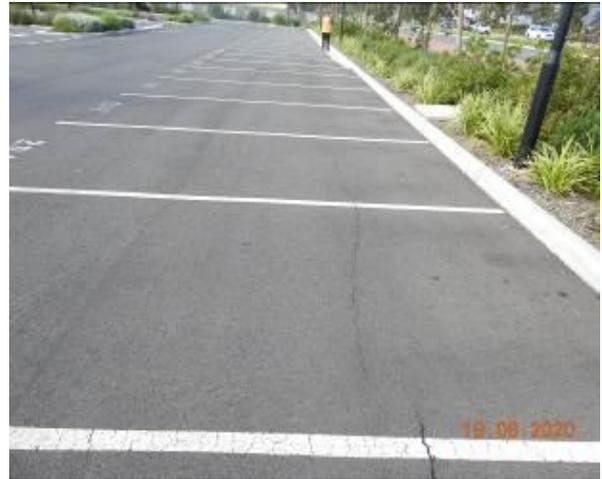
Figure 1638 – Crack propagation through car park pavement
