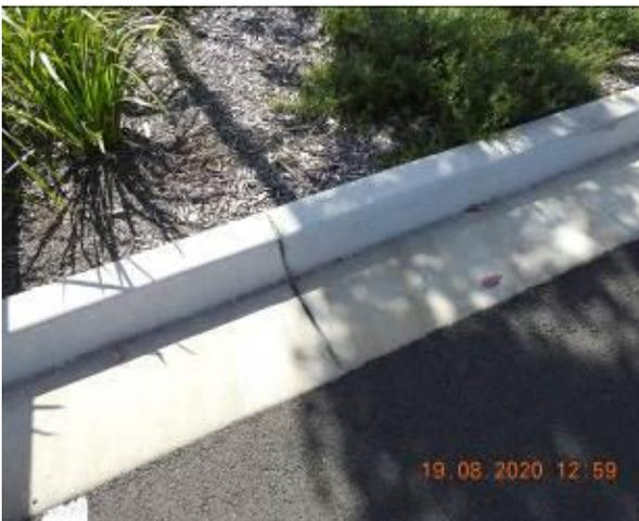
Figure 2209 – Crack propagation through car park kerb
