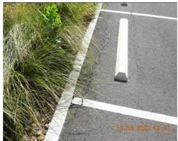
Figure 1904 – General condition of car park kerb and evidence of patchwork through carpark pavement
