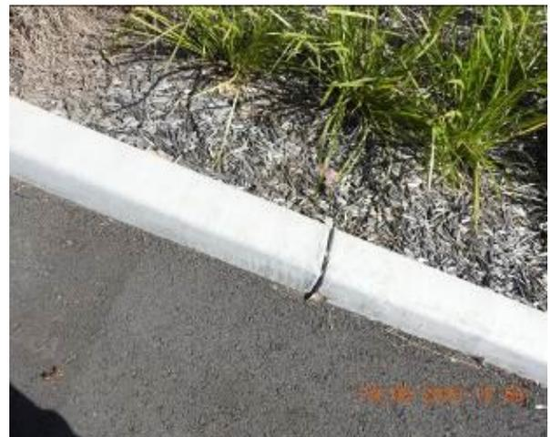
Figure 2162 – Crack propagation through car park kerb
