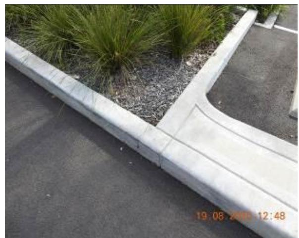
Figure 2054 – Crack propagation through car park kerb
