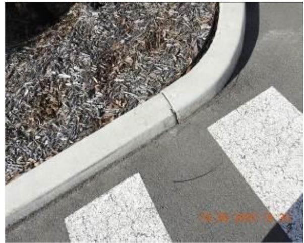
Figure 1308 – Crack propagation through car park kerb
