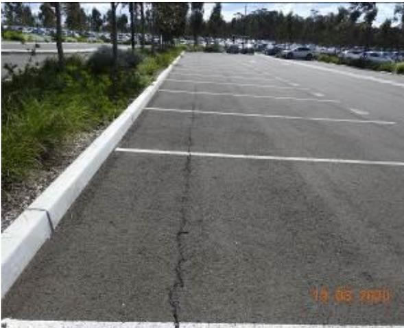
Figure 1445 – Crack propagation and evidence of patchwork through car park pavement
