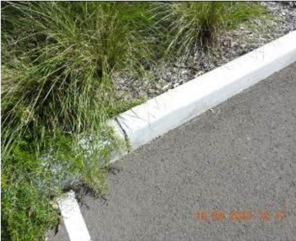
Figure 1743 – Crack propagation through car park kerb
