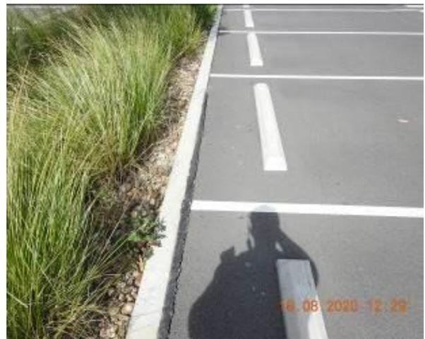
Figure 1862 – Crack propagation through car park kerb
