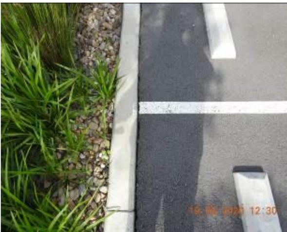
Figure 1873 – Crack propagation through car park kerb
