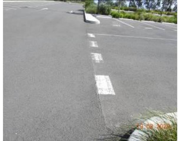
Figure 1558 – Crack propagation through car park pavement
