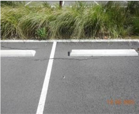
Figure 1523 – Evidence of patchwork through car park pavement
