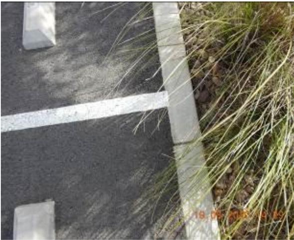
Figure 1229 – Crack propagation through car park kerb
