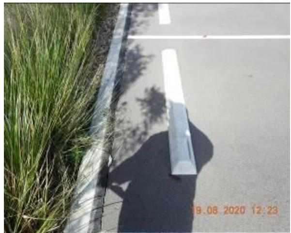
Figure 1796 – Crack propagation through car park kerb
