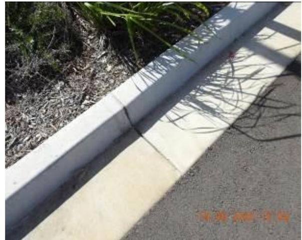
Figure 2208 – Crack propagation through car park kerb
