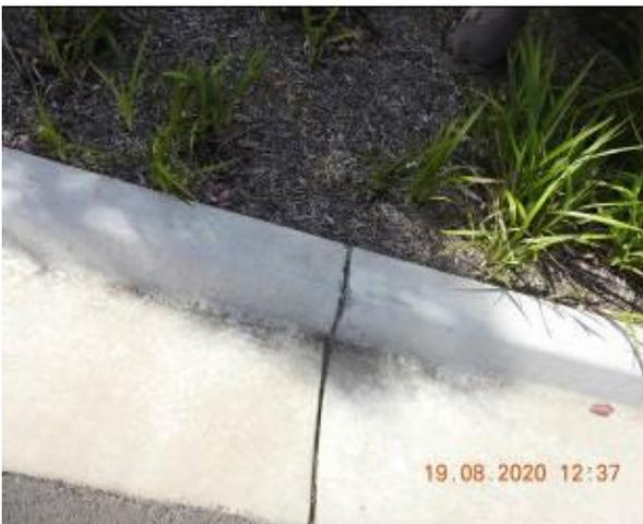
Figure 1945 – Crack propagation through car park gutter
