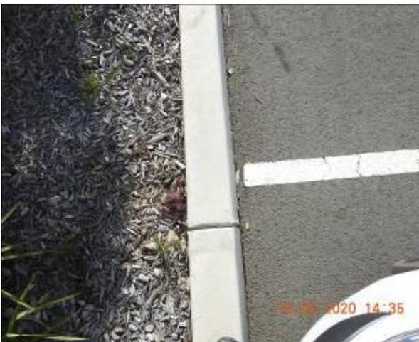
Figure 1289 – Crack propagation through car park kerb
