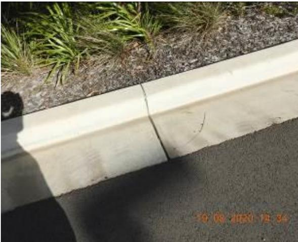
Figure 1265 – Crack propagation through car park kerb
