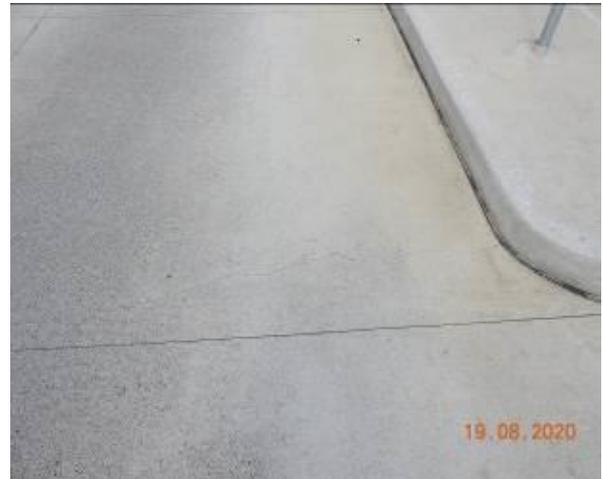
Figure 1398 – Crack propagation through car park pavement
