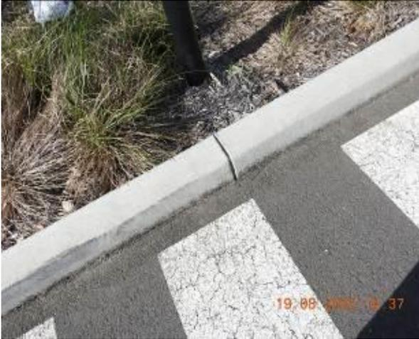
Figure 1317 – Crack propagation through car park kerb
