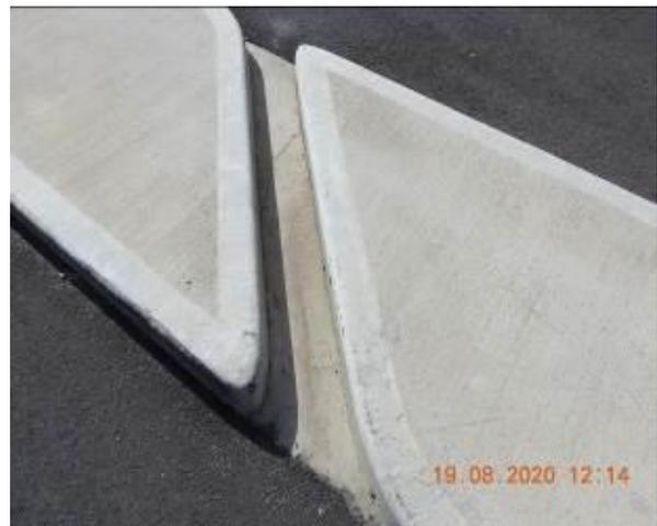
Figure 1724 – Crack propagation through traffic island
