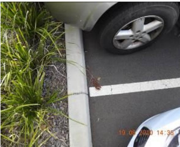
Figure 1285 – Crack propagation through car park kerb
