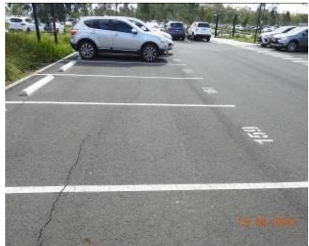
Figure 1520 – Crack propagation through car park pavement
