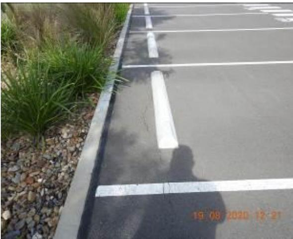
Figure 1781 – Crack propagation through car park kerb
