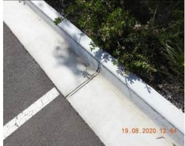
Figure 2014 – Crack propagation and loss of material through car park gutter
