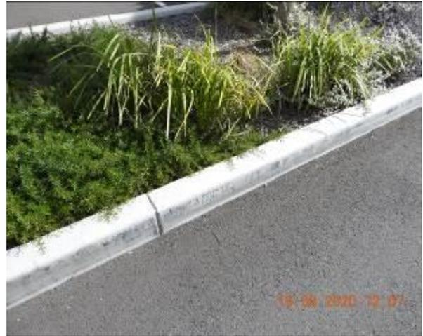
Figure 1678 – Crack propagation through car park kerb
