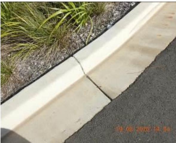
Figure 1267 – Crack propagation through car park kerb
