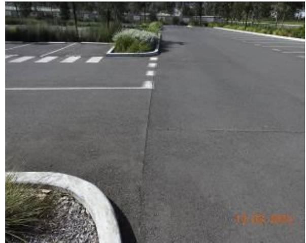
Figure 1434 – Crack propagation through car park pavement
