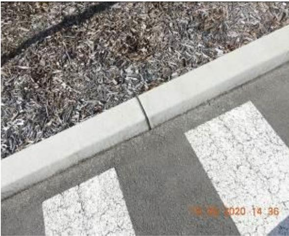
Figure 1307 – Crack propagation through car park kerb
