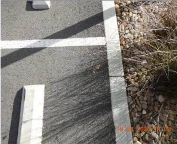
Figure 1227 – Crack propagation through car park kerb
