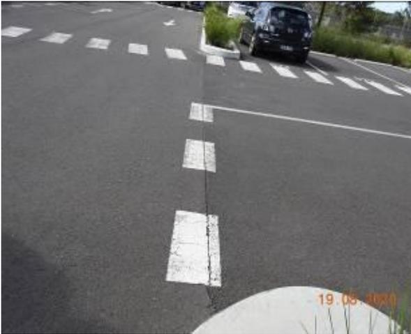
Figure 1497 – Crack propagation through car park pavement
