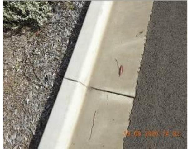
Figure 1246 – Crack propagation through car park kerb
