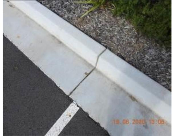
Figure 2272 – Crack propagation through car park kerb
