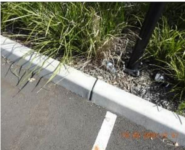
Figure 2179 – Crack propagation through car park kerb
