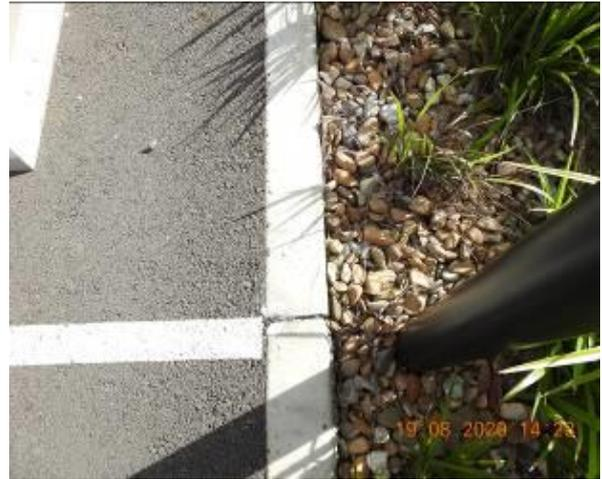
Figure 1204 – Crack propagation through car park kerb
