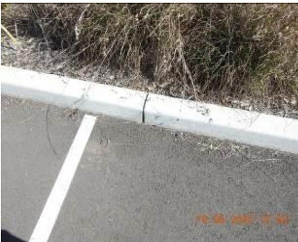
Figure 2155 – Crack propagation through car park kerb
