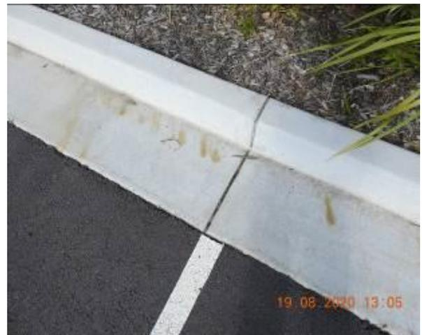
Figure 2270 – Crack propagation through car park kerb
