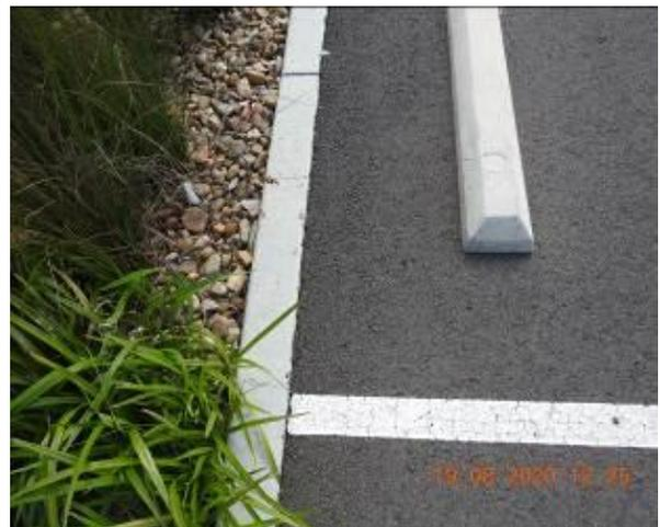
Figure 1820 – Crack propagation through car park kerb
