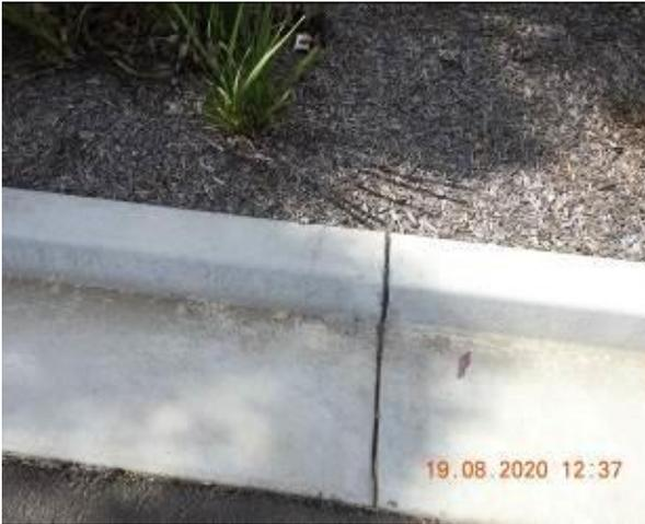
Figure 1941 – Crack propagation through car park kerb
