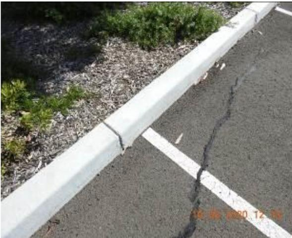
Figure 1763 – Crack propagation through car park kerb
