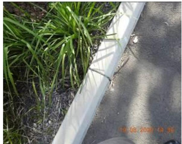
Figure 1292 – Crack propagation through car park kerb
