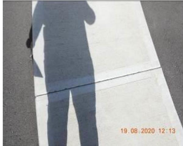
Figure 1720 – Crack propagation through traffic island
