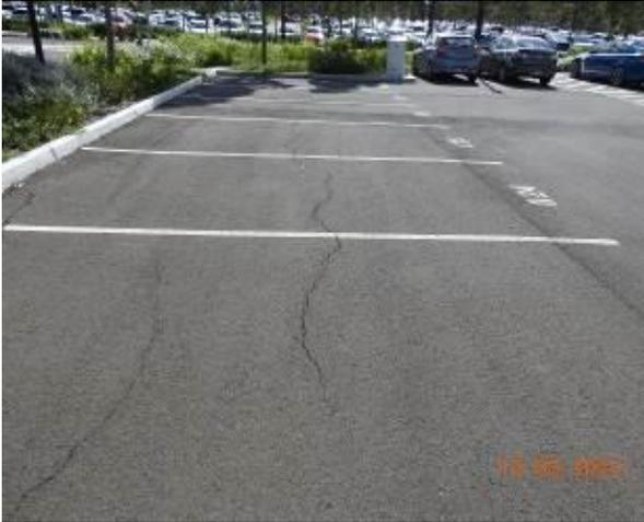
Figure 1455 – Crack propagation through car park pavement
