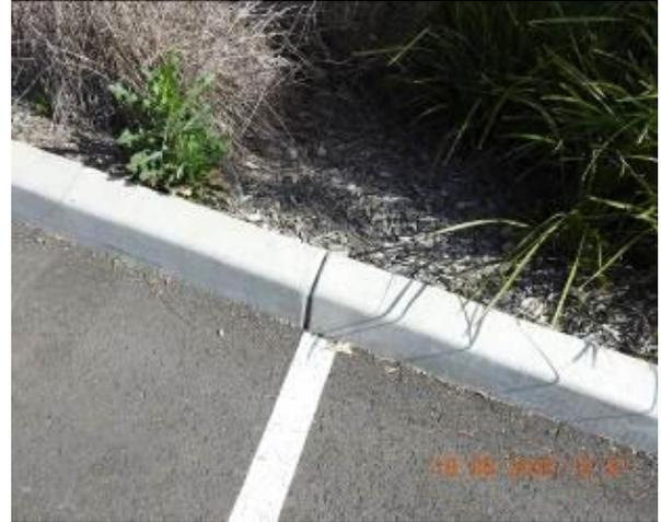
Figure 2176 – Crack propagation through car park kerb
