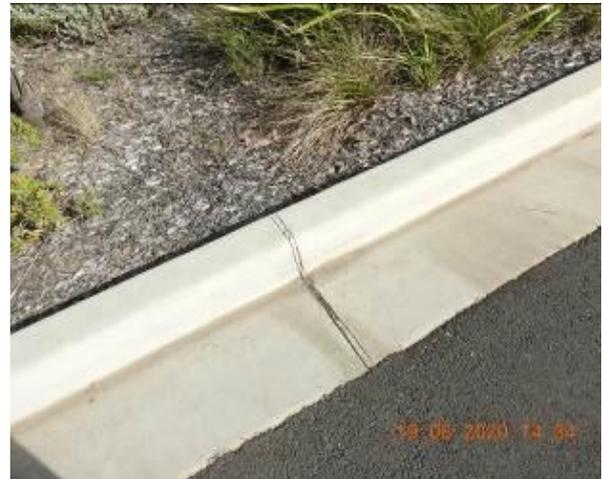
Figure 1266 – Crack propagation through car park kerb
