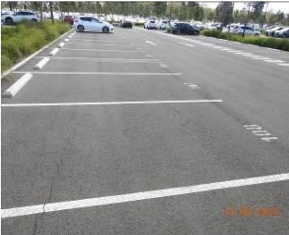
Figure 1487 – Crack propagation through car park pavement
