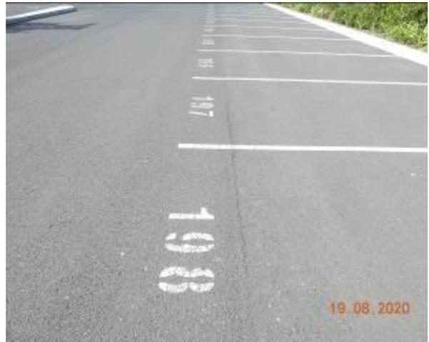
Figure 1644 – Crack propagation through car park pavement
