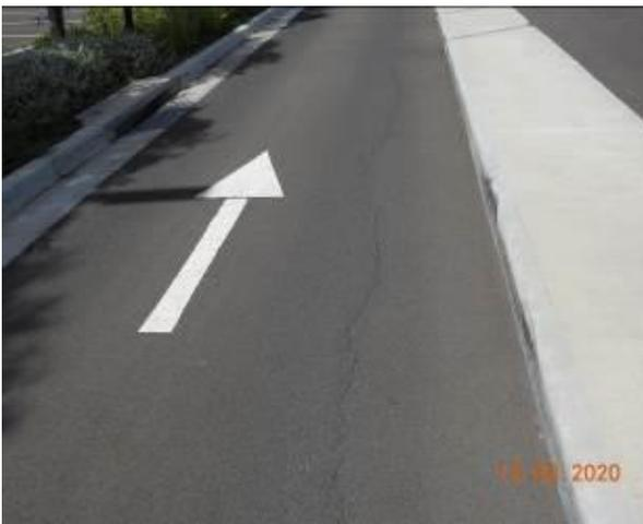
Figure 1405 – Crack propagation through car park pavement
