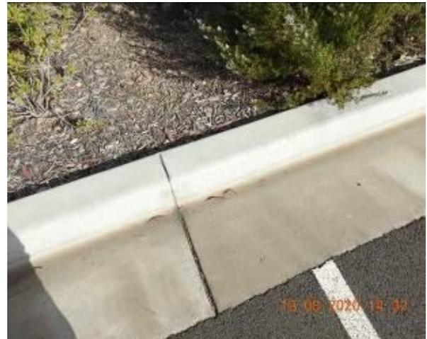
Figure 1248 – Crack propagation through car park kerb
