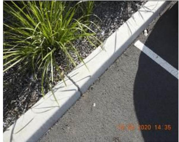
Figure 1288 – Crack propagation through car park kerb
