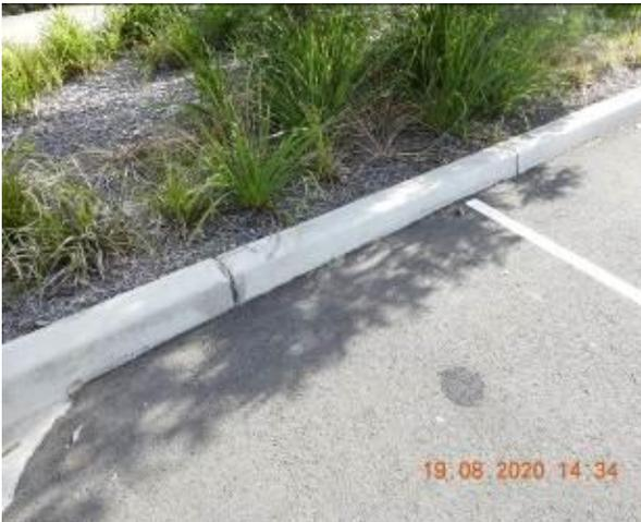
Figure 1271 – Crack propagation through car park kerb
