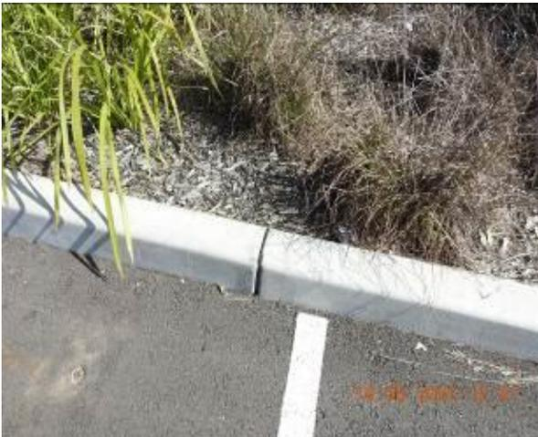
Figure 2177 – Crack propagation through car park kerb
