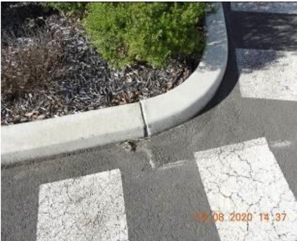
Figure 1319 – Crack propagation through car park kerb
