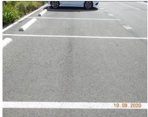
Figure 1494 – Crack propagation through car park pavement
