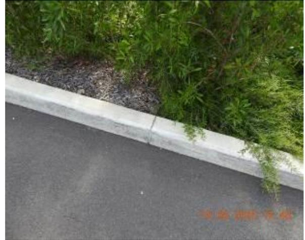
Figure 2056 – Crack propagation through car park kerb
