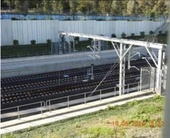
Figure 2382 – General condition of railway corridor, steel portal haunch and overhead power system
