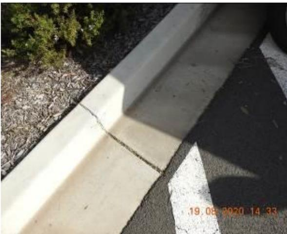
Figure 1255 – Crack propagation through car park kerb
