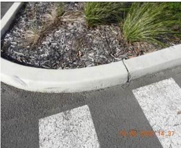
Figure 1315 – Crack propagation through car park kerb
