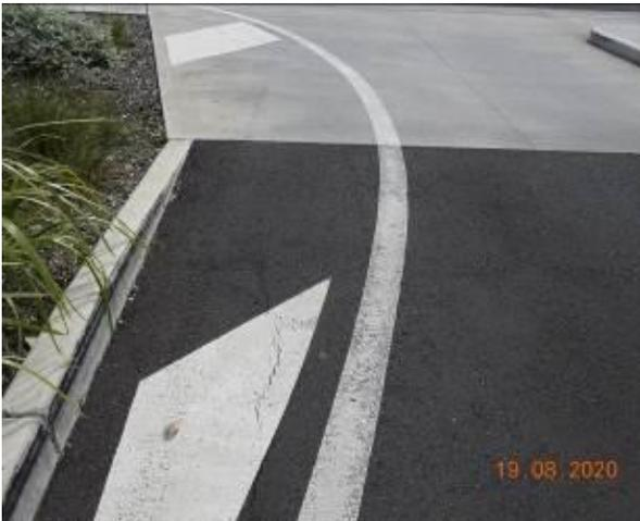
Figure 1427 – Crack propagation through car park pavement
