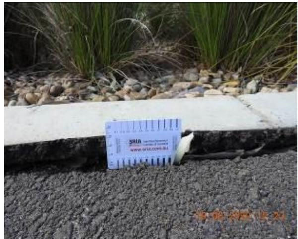
Figure 1794 – Separation through expansion joint approx. 30 mm in height
