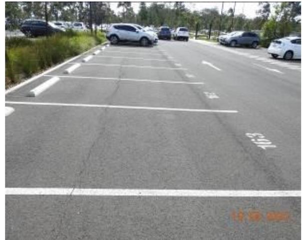
Figure 1518 – Crack propagation through car park pavement
