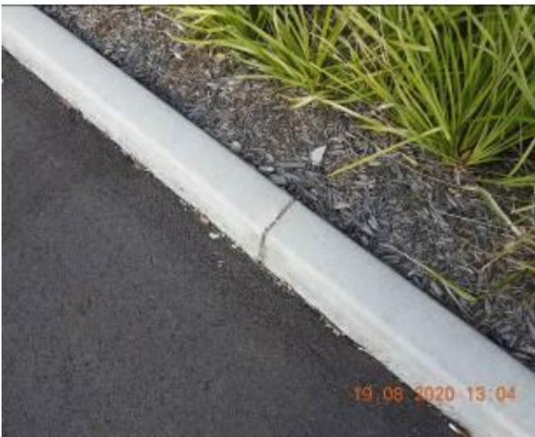
Figure 2243 – Crack propagation through car park kerb
