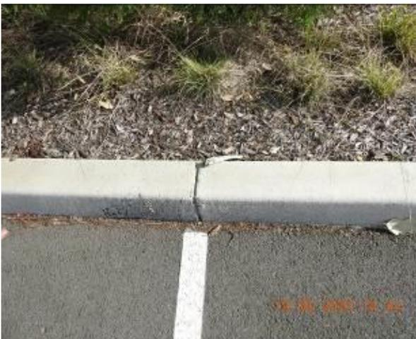
Figure 1273 – Crack propagation through car park kerb
