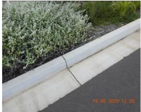
Figure 1656 – Crack propagation through car park kerb
