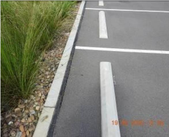
Figure 1851 – Crack propagation through car park kerb
