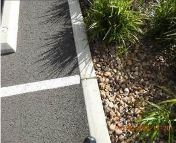
Figure 1215 – Crack propagation through car park kerb
