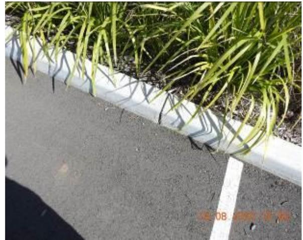
Figure 2160 – Crack propagation through car park kerb
