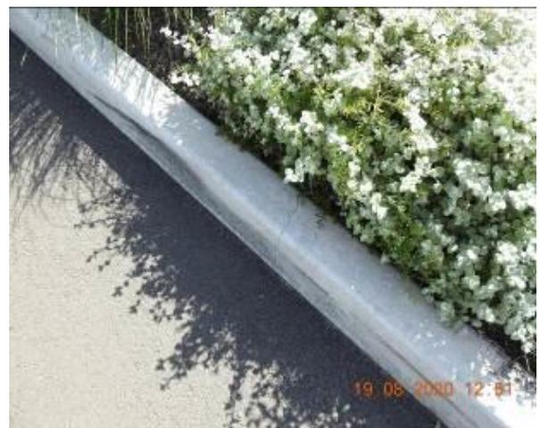
Figure 2084 – Crack propagation through car park kerb
