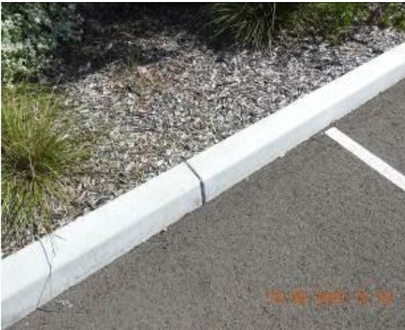
Figure 1757 – Crack propagation through car park kerb
