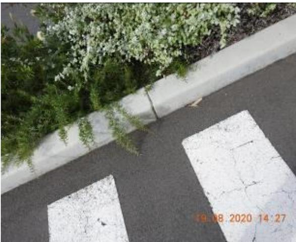
Figure 1199 – Crack propagation through car park kerb
