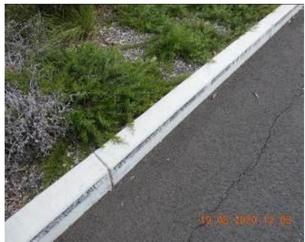
Figure 1688 – Crack propagation through car park kerb
