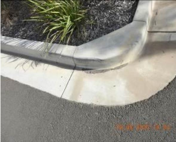
Figure 1263 – Hairline cracking through car park kerb and gutter
