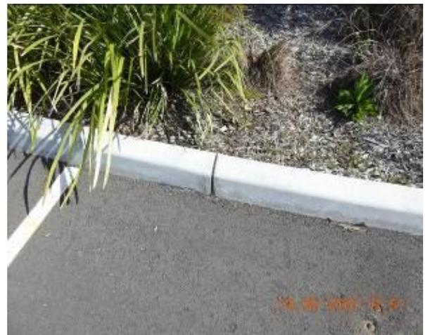
Figure 2168 – Crack propagation through car park kerb
