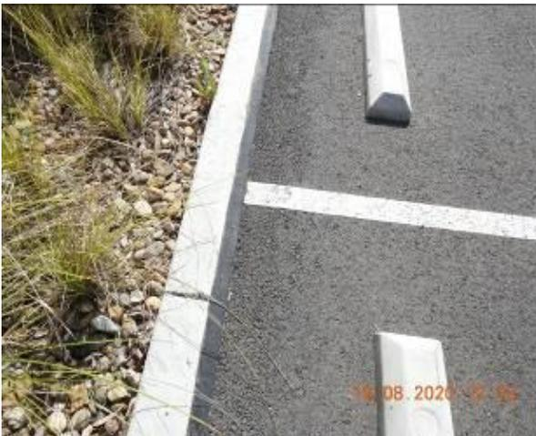
Figure 1829 – Crack propagation through car park kerb
