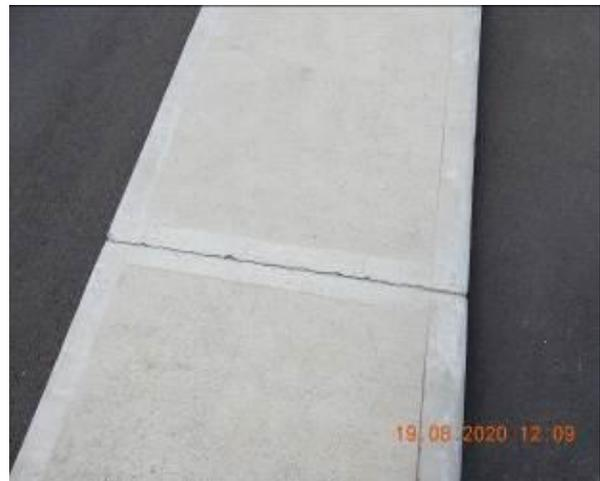
Figure 1704 – Crack propagation through traffic island
