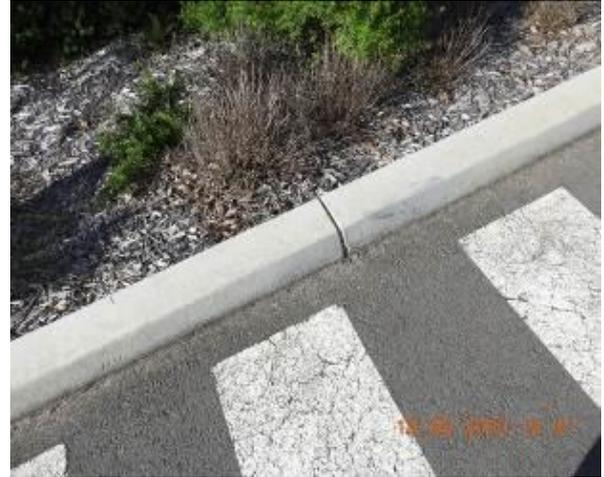
Figure 1318 – Crack propagation through car park kerb
