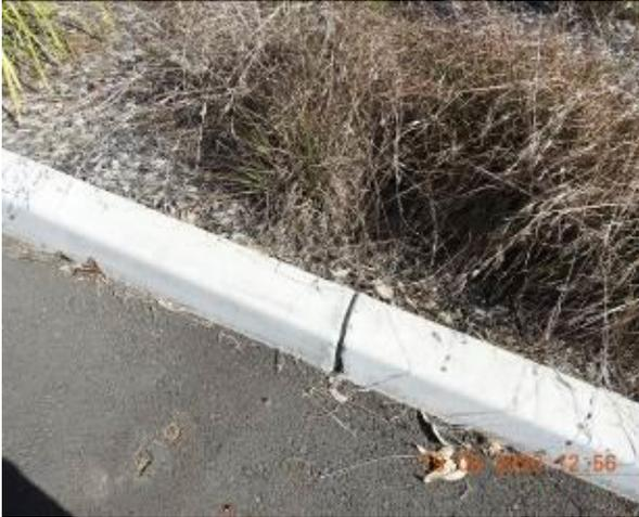
Figure 2163 – Crack propagation through car park kerb
