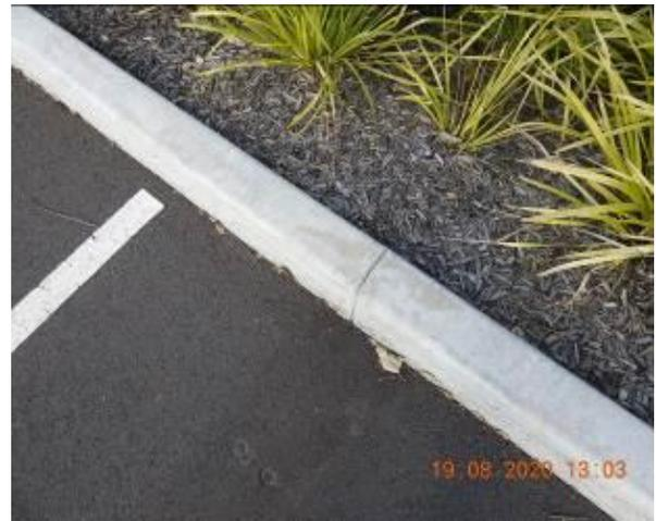
Figure 2232 – Crack propagation through car park kerb
